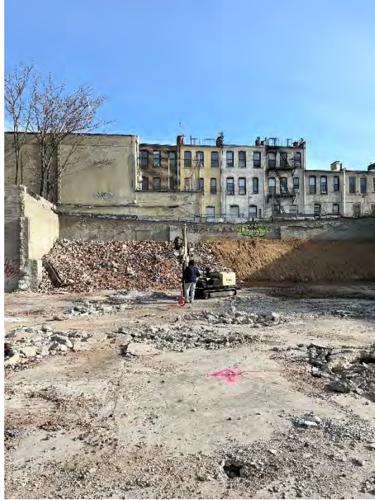
Photo 1: View of drilling activities, facing north.
