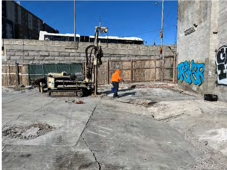
Photo 1: View of drilling activities at SB/SV-02, facing west.
