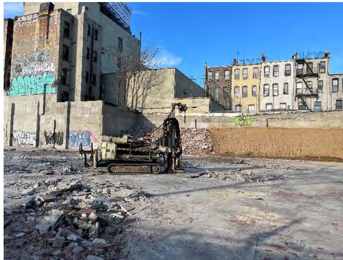
Photo 2: Alternate view of drilling activities, facing north.
