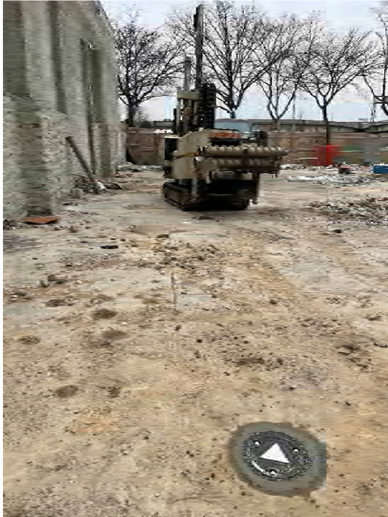
Photo 1: View of installed monitoring well and drilling activities, facing south.
