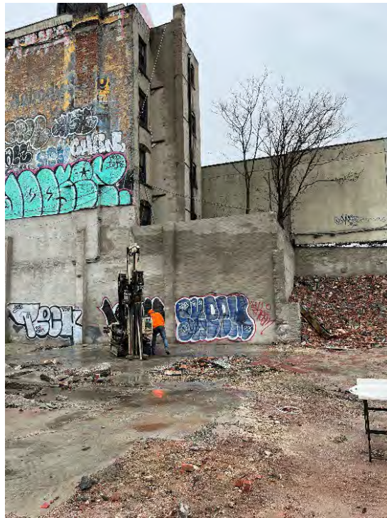
Photo 2: View of drilling activities, facing north.
