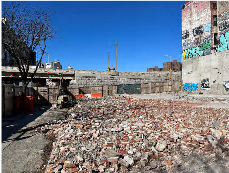
Photo 1: View of drilling activities at SB/MW-01, facing west.
