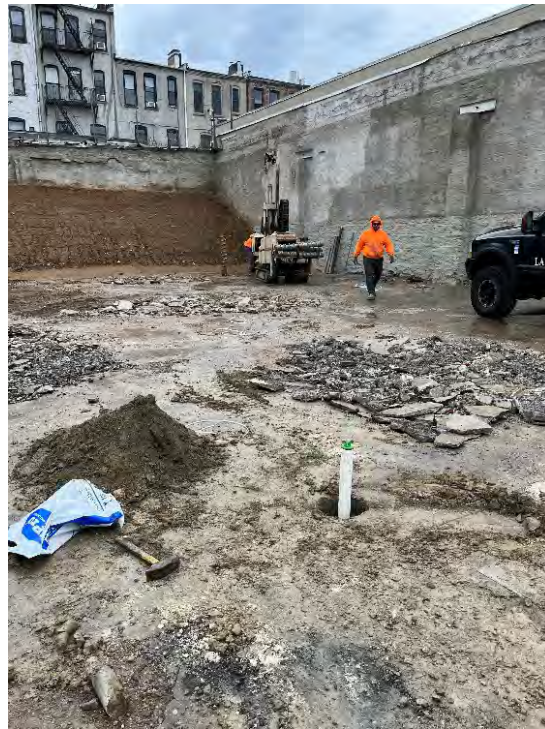
Photo 1: View of drilling activities and monitoring well installation, facing northeast.
