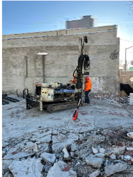
Photo 1: View of drilling activities, facing east.
