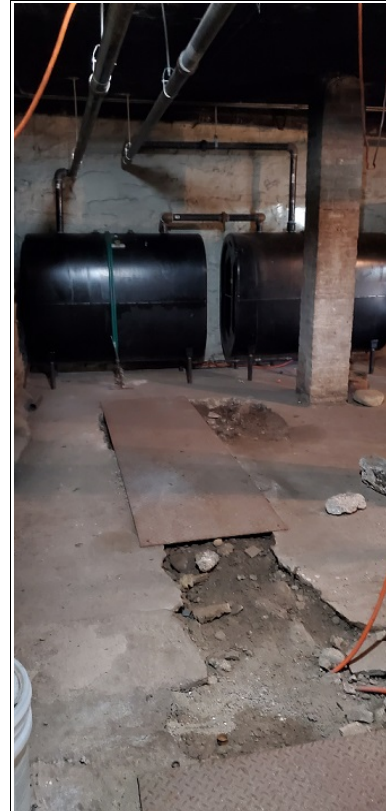
Figure 2. Abandoned UST beneath metal plate.
