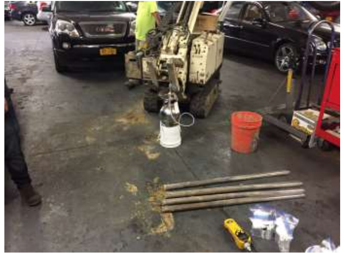
PHOTO 8: Geoprobe Drilling location B-4
