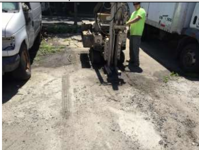
PHOTO 18: Geoprobe Drilling B-10
