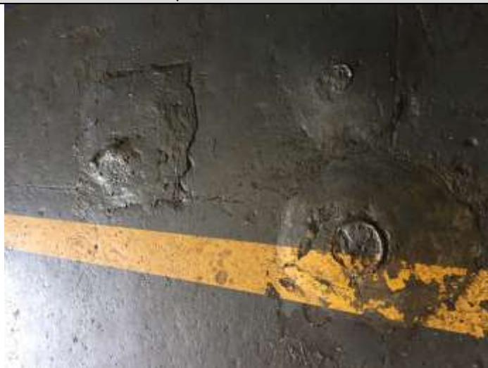
PHOTO 9: Evidence of UST fillports in garage building
