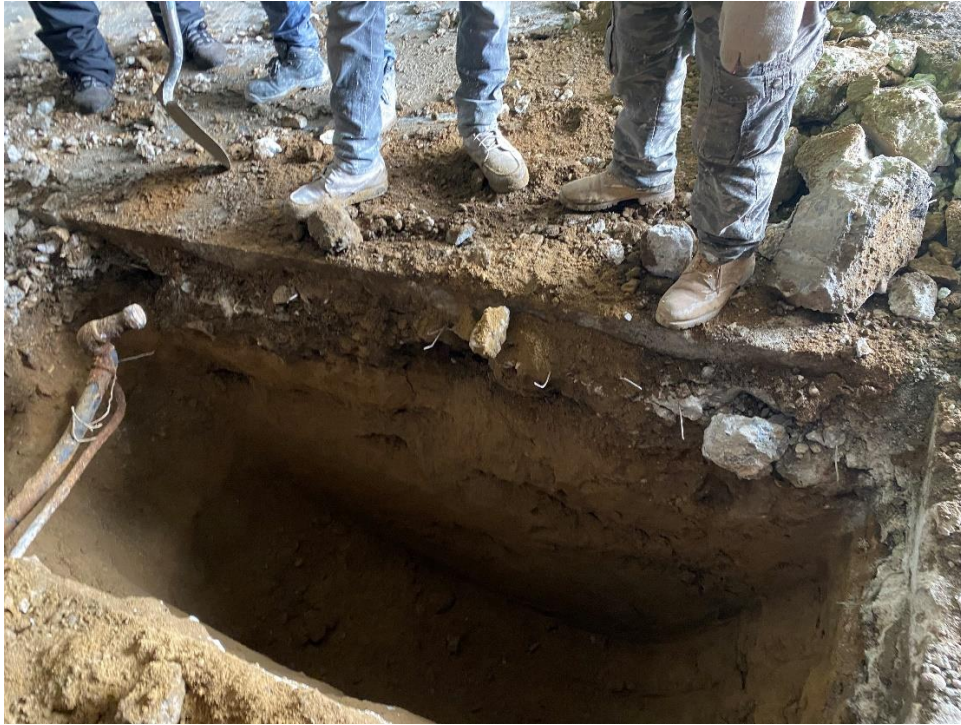
Large Test Pit within the Interior Parking Area, showing corroded below grade piping.
