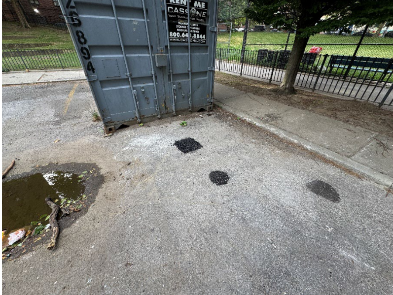
Photo 1: RIMW and RISV – 1 final asphalt patchwork.
