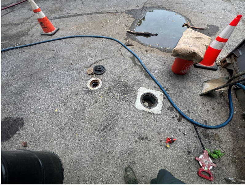
Photo 1: RIMW and RISV – 1 before abandonment.
