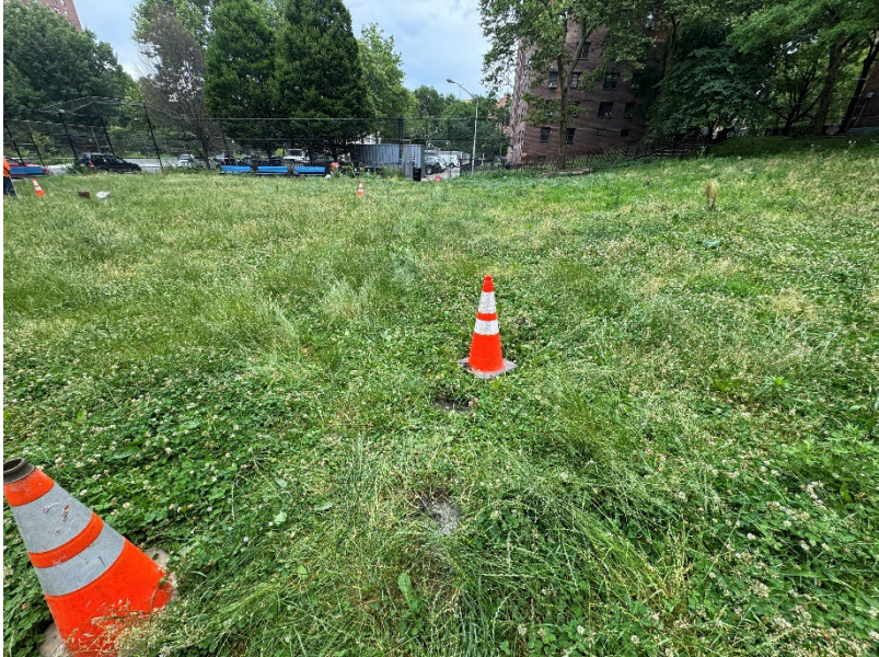
Photo 3: Facing north multiple wells plugged, grouted and coned off.
