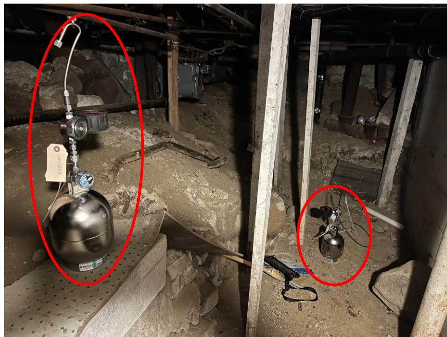
Photo 2 – View of sub-slab vapor (SVI_SSV01) and co-located indoor air (SVI_IA01) samples located in the cellar in the northwestern part of the building on Lot 32 (facing west).
