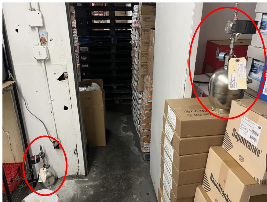
Photo 3 – View of sub-slab vapor (SVI_SSV09) and co-located indoor air (SVI_IA09) samples located in the basement of the one-story supermarket in Lot 16 (facing north).
