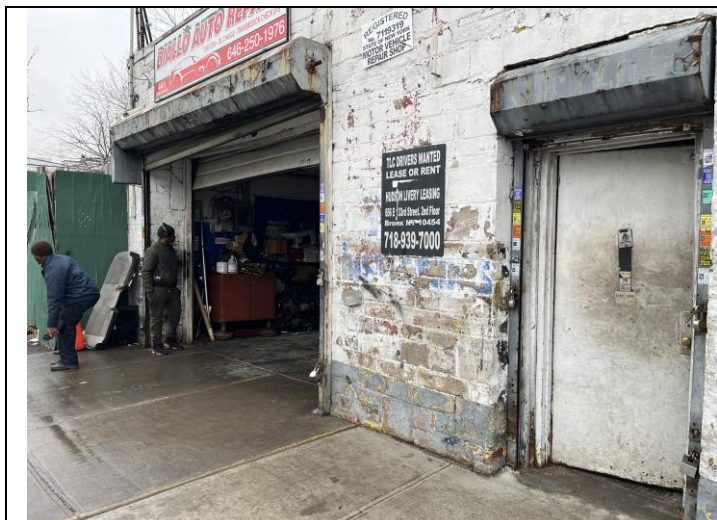
PHOTO 1: Front Entrance of mechanics garage building
