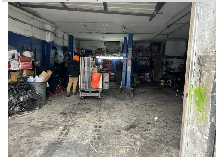
PHOTO 5: View inside garage building
