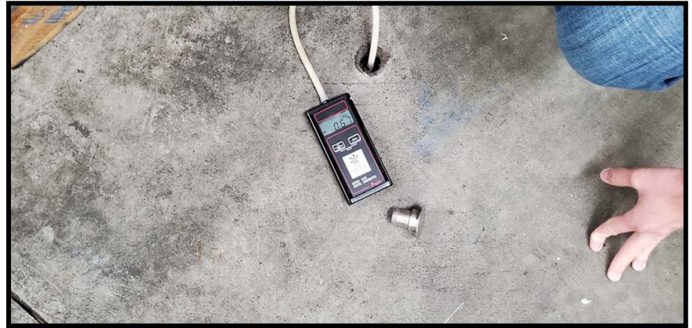
View of monitoring point SP-2, showing a vacuum reading of -0.67 inches water column.
