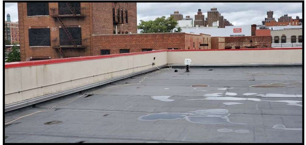
View of the northern blower fan unit on the roof, which read -3.2 inches water column.
