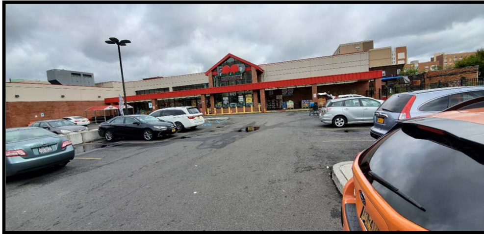
View of the parking lot of the Site. The parking lot's composite cover appeared to be in good condition.
