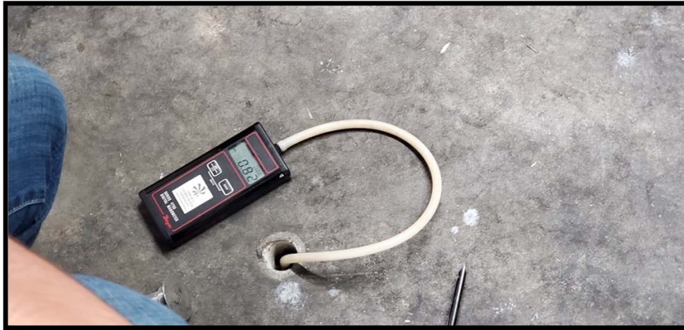
View of monitoring point SP-1, showing a vacuum reading of -0.82 inches water column.
