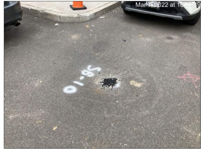
Photograph 10. Location SB-10 on the southern portion of the Site backfilled and surface patched with asphalt following sampling activities.
