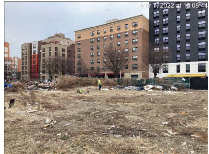
Photograph 2. Geophysical survey of the vacant lot on the eastern portion of the Site, prior to the commencement of drilling activities.
