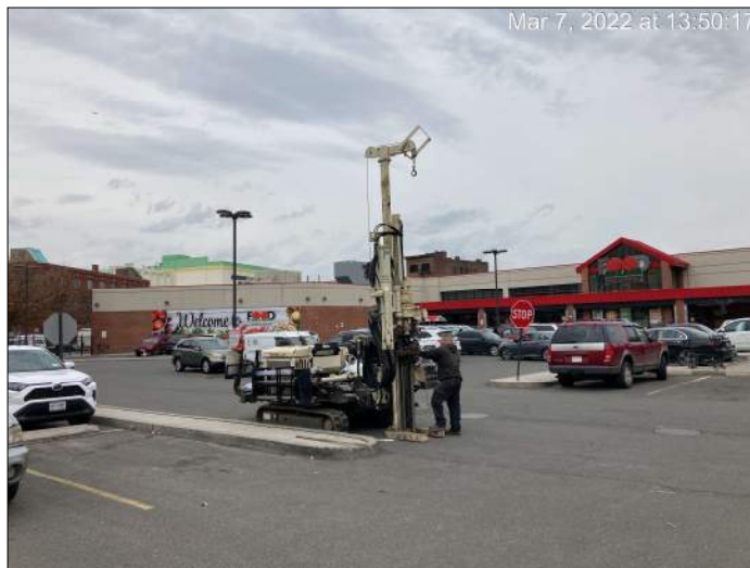
Photograph 3. Drilling activities using Geoprobe® direct push probe at location SB-09 on the central portion of the Site.
