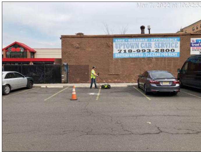
Photograph 1. Geophysical survey of the asphalt parking lot on the eastern-central portion of the Site, prior to the commencement of drilling activities.
