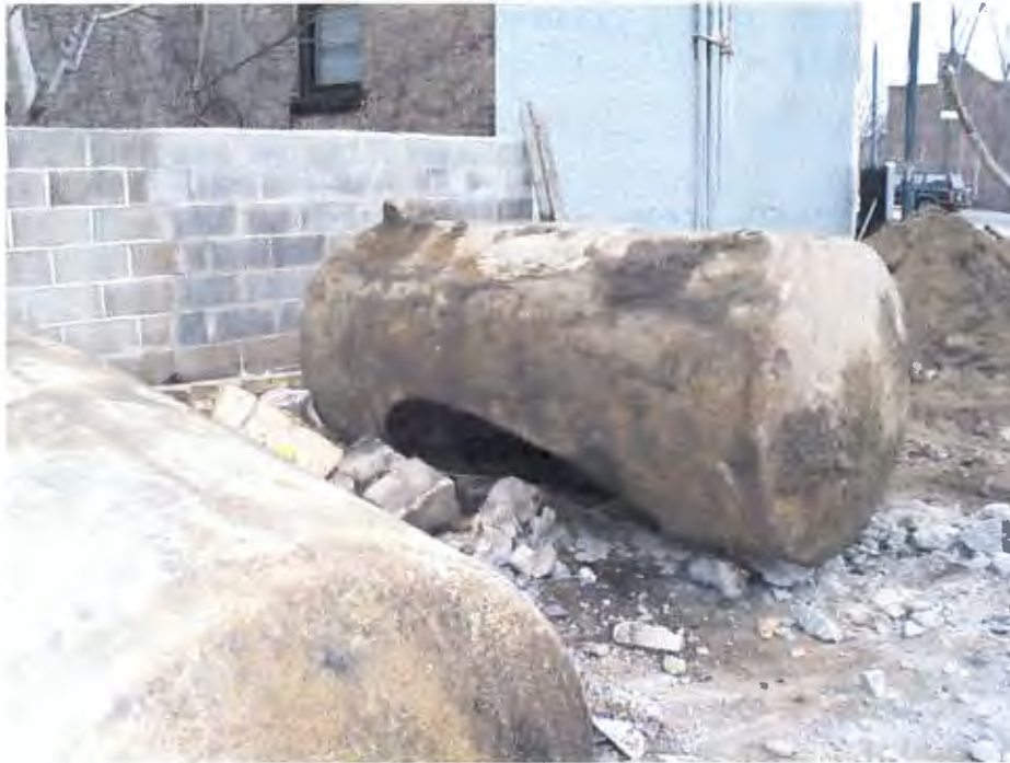
GASOLINE TANKS REMOVED FROM EXCAVATION
