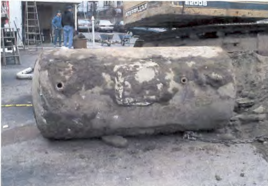
GASOLINE TANK REMOVED FROM EXCAVATION
