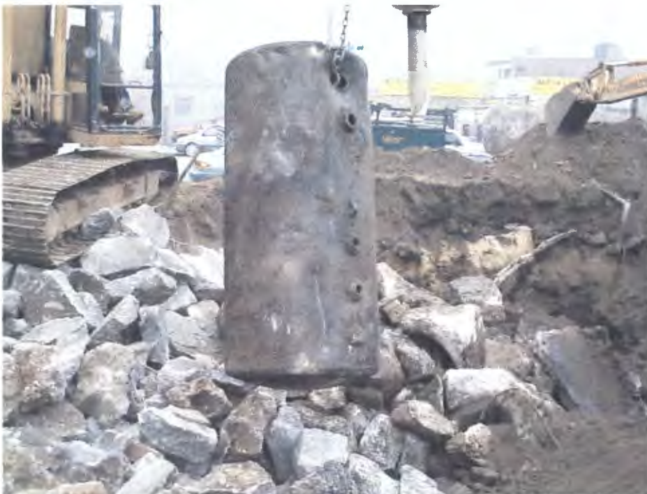
GASOLINE TANK REMOVED FROM EXCAVATION
