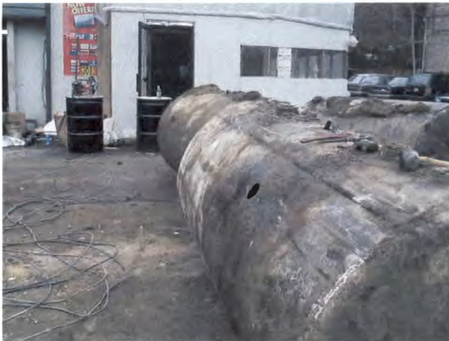
GASOLINE TANKS REMOVED FROM EXCAVATION
