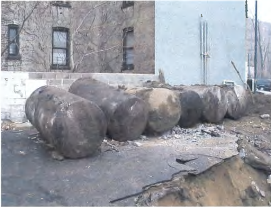
GASOLINE TANKS REMOVED FROM EXCAVATION
