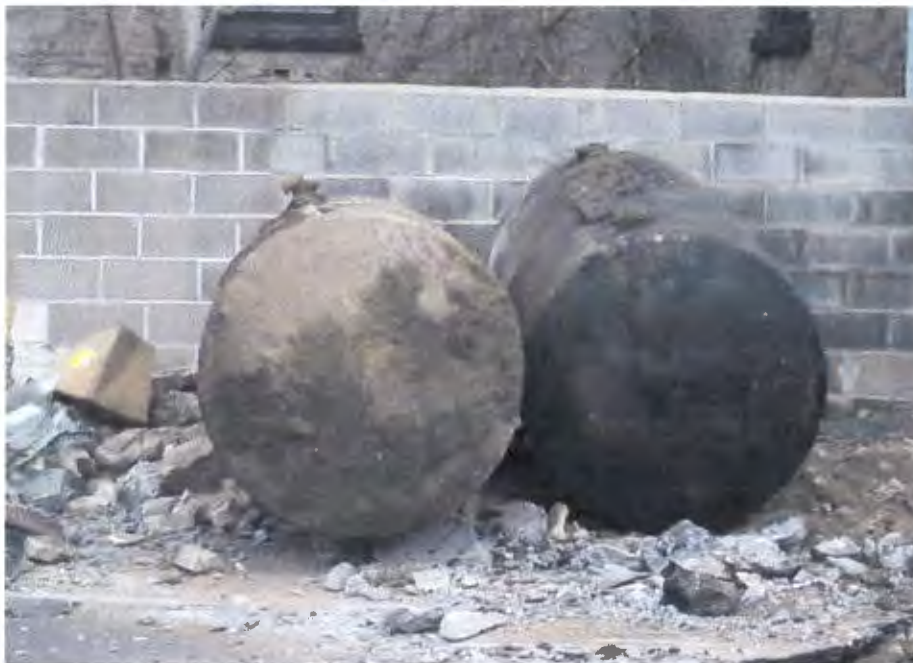
GASOLINE TANKS REMOVED FROM EXCAVATION
