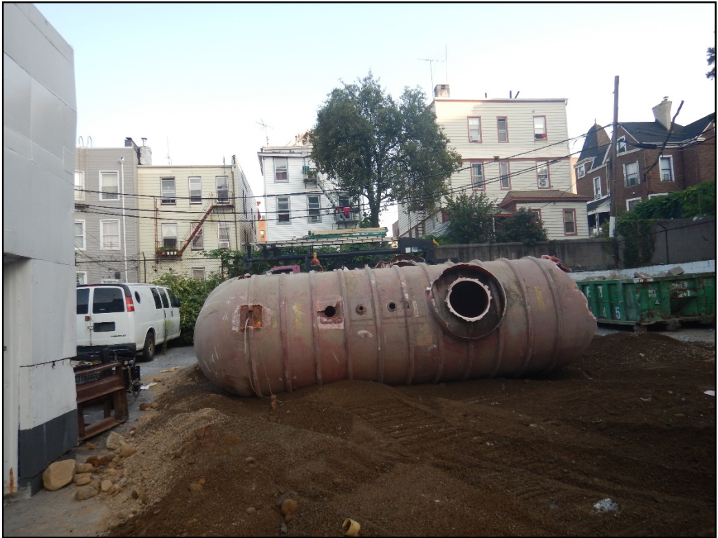
Photo 3: Tank 11 after removal
