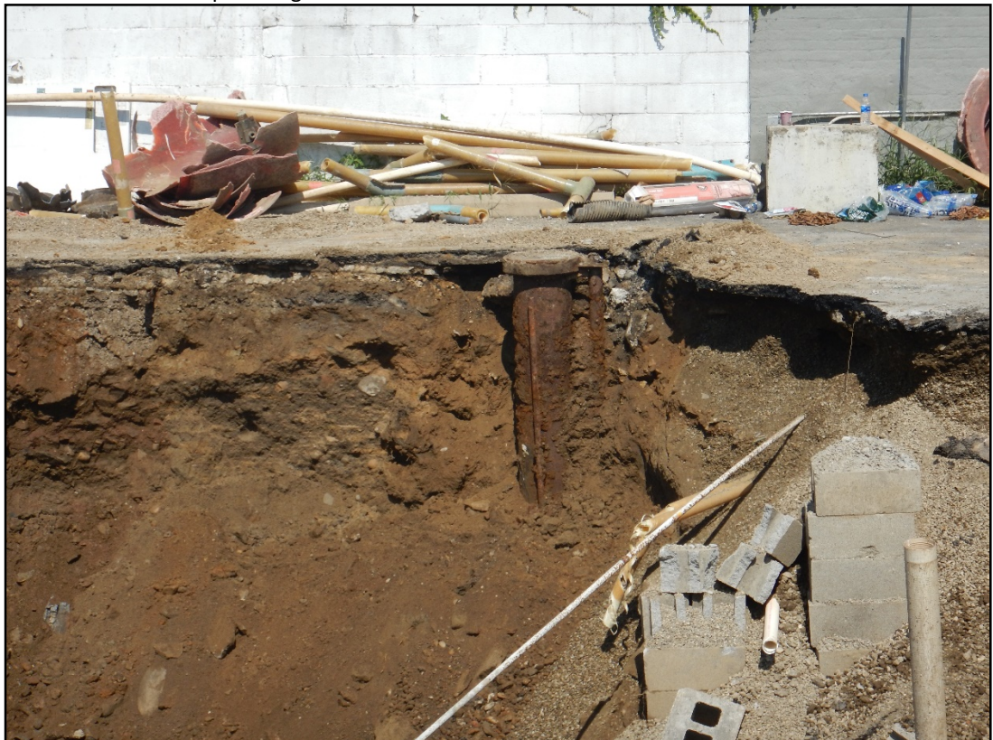
Photo 6: Hydraulic lift during removal
