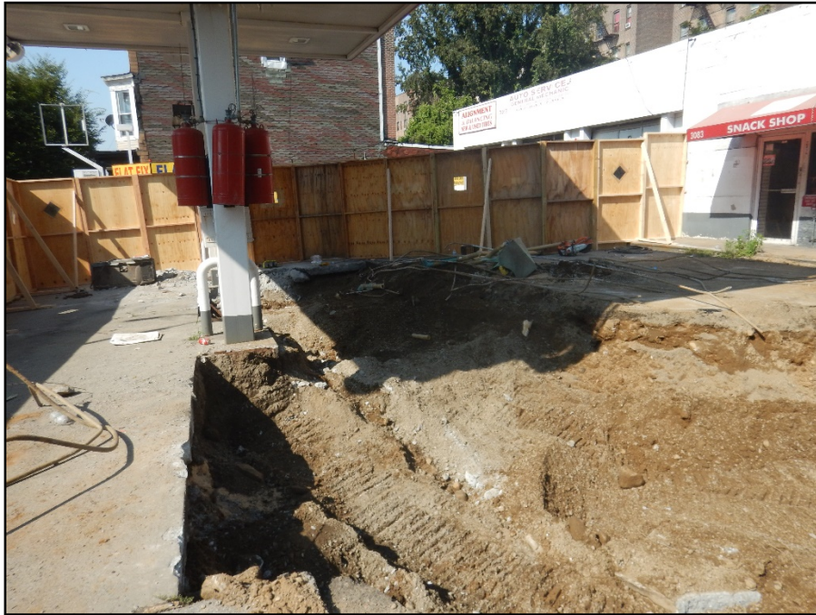
Photo 7: View of area where dispenser sumps removed and product line area DATE: 2021-8-26
