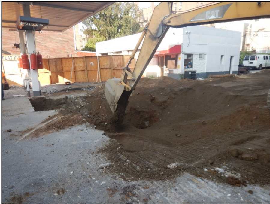
Photo 7: View of area where dispenser sumps removed and product line area DATE: 2021-8-26
