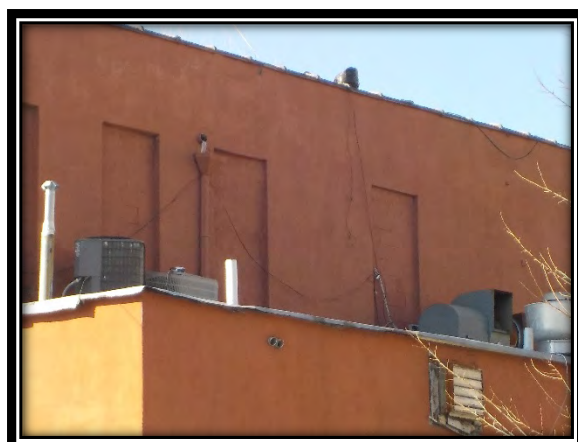
Two AC Compressors & Exhaust Vents
