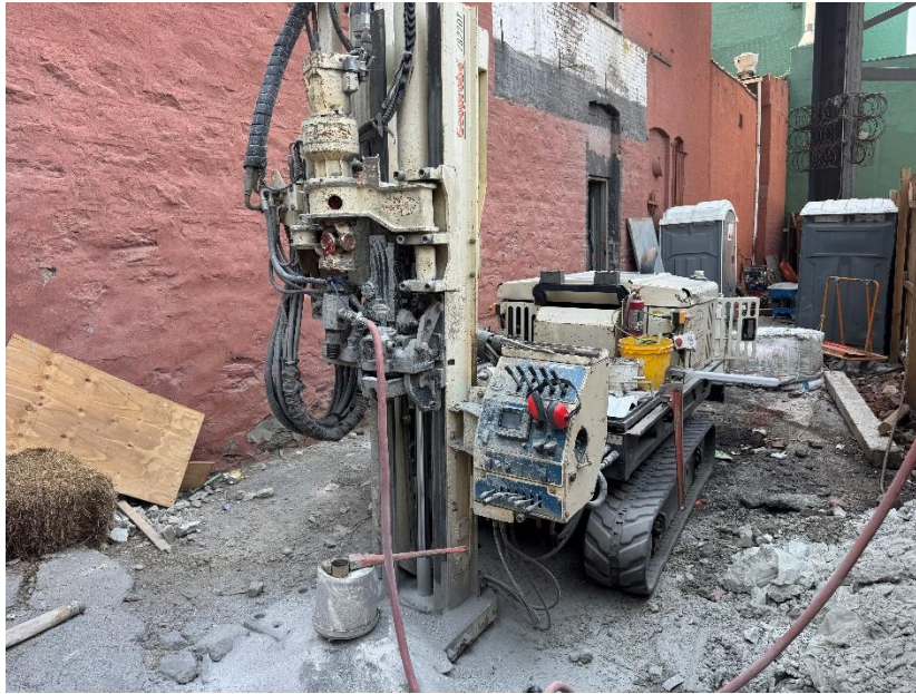
Photo 1: View of monitoring well installation at HA-MW05, facing south.
