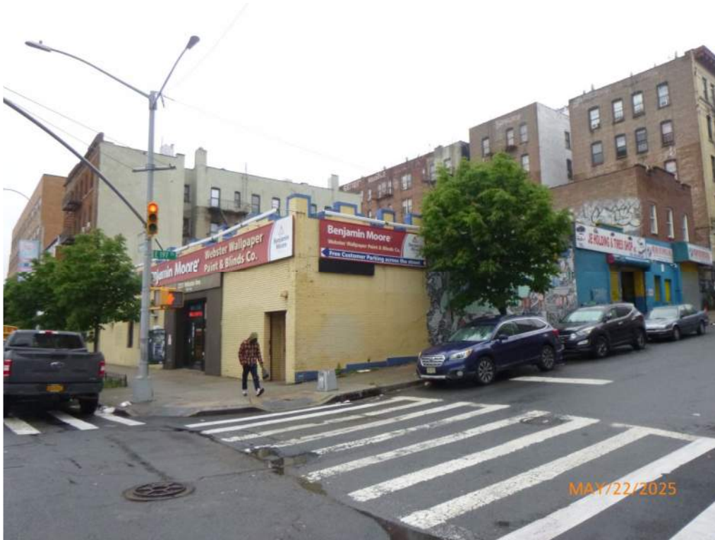
Photograph 1: View of the Site looking southwest from across the intersection of Webster Avenue and E. 197 th Street. The 2737 to 2747 Webster Avenue building visible at foreground. The two smaller attached Site structures are visible at right-background.
