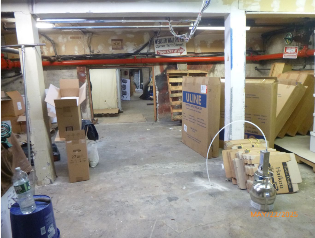
Photograph 3: Typical sub-slab soil vapor sample. SV2 shown.
