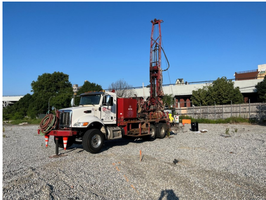
Photo 2: Craig advancing geotechnical boring GB-B-02 (facing northwest)
