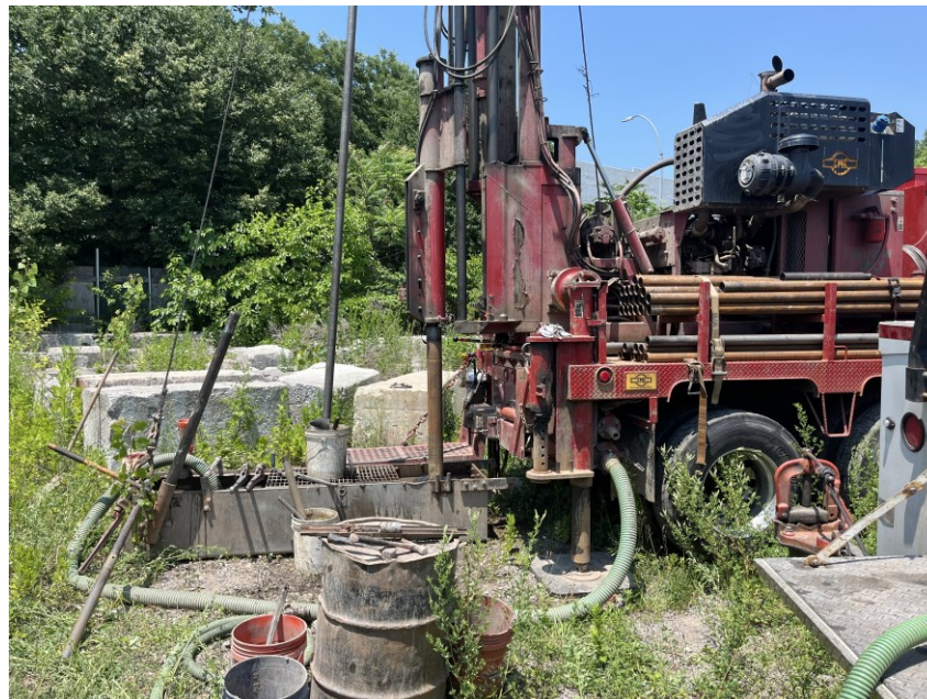
Photo 2: Craig advancing geotechnical boring GB-D-02 (facing west)
