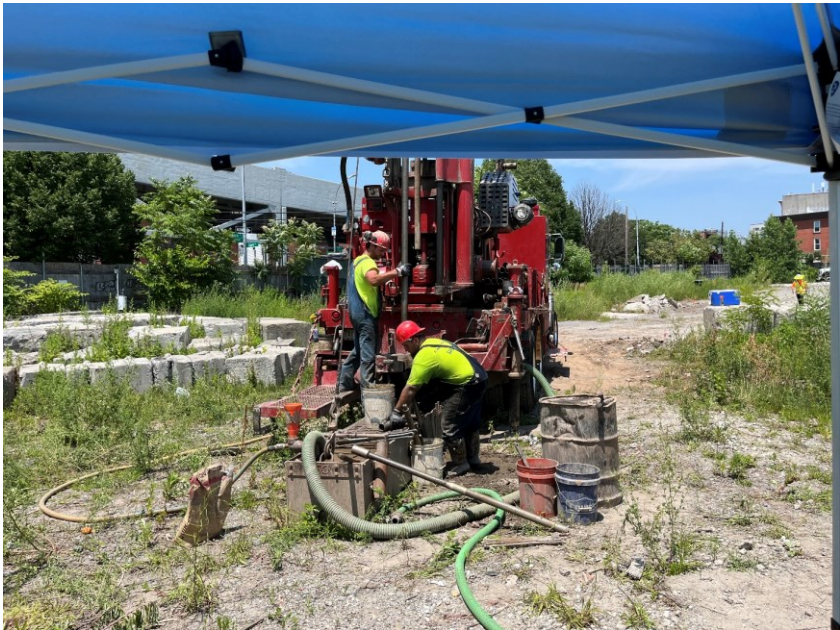
Photo 2: Craig advancing geotechnical boring GB-D-03 (facing northwest)
