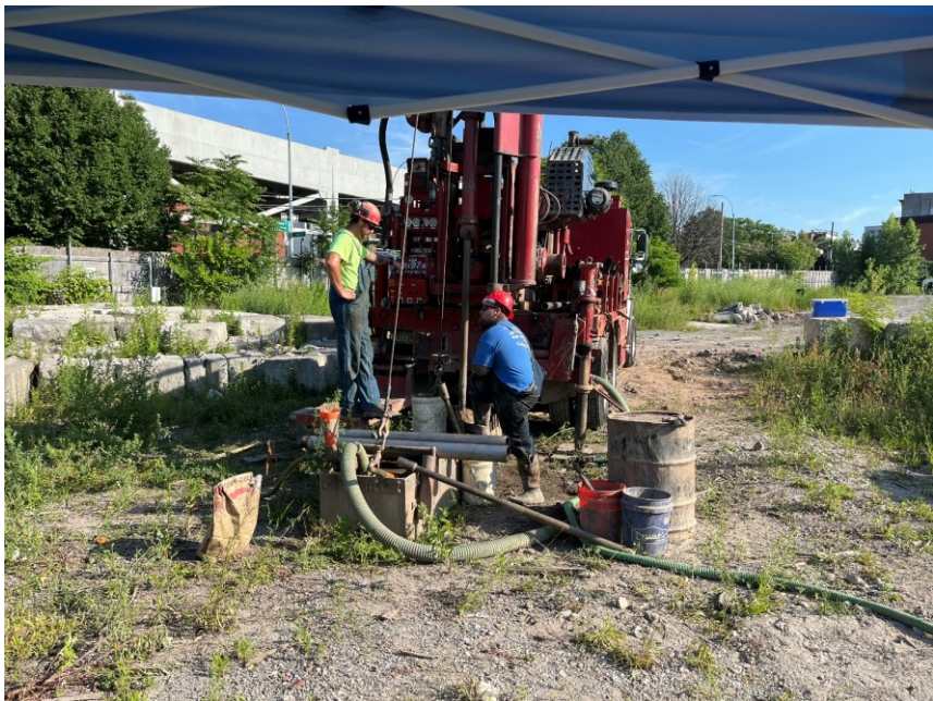
Photo 2: Craig advancing geotechnical boring GB-D-03 (facing north)
