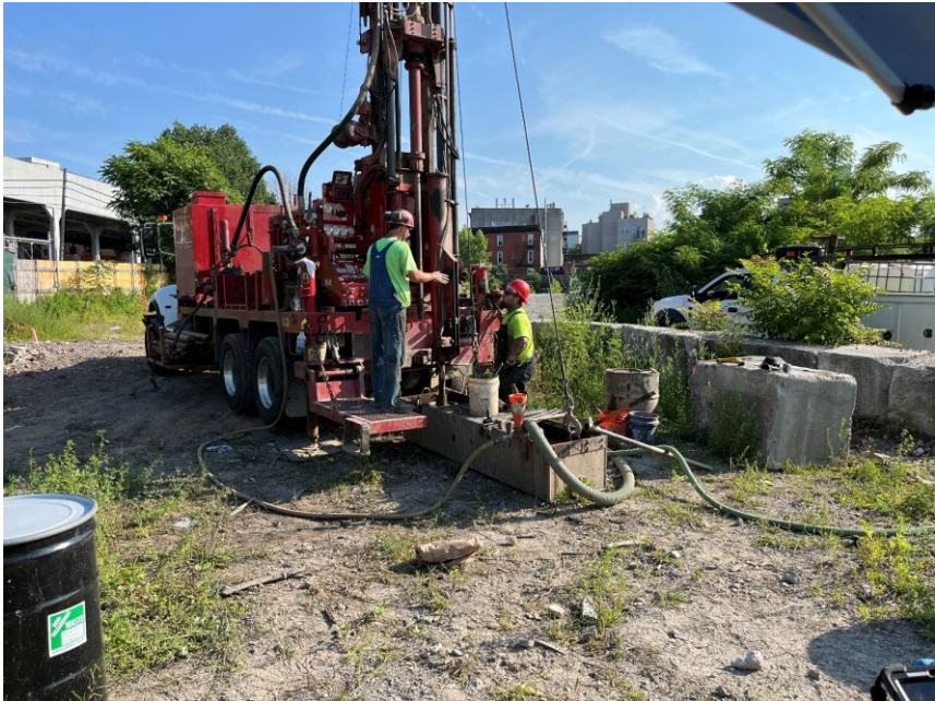
Photo 2: Craig advancing geotechnical boring GB-D-03 (facing north)
