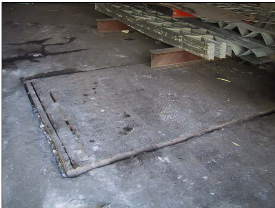
Photograph 6. Metal floor plate noted on the paved area south of the two on-site structures. The place could potentially access a petroleum or chemical storage tank.
