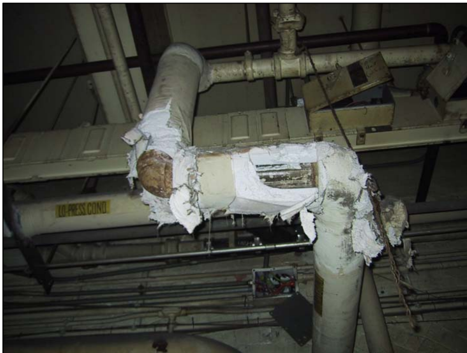
Photograph 4. Suspect asbestos-containing thermal pipe insulation observed in the two-story warehouse structure. Suspect pipe insulation was noted in both on-site structures.
