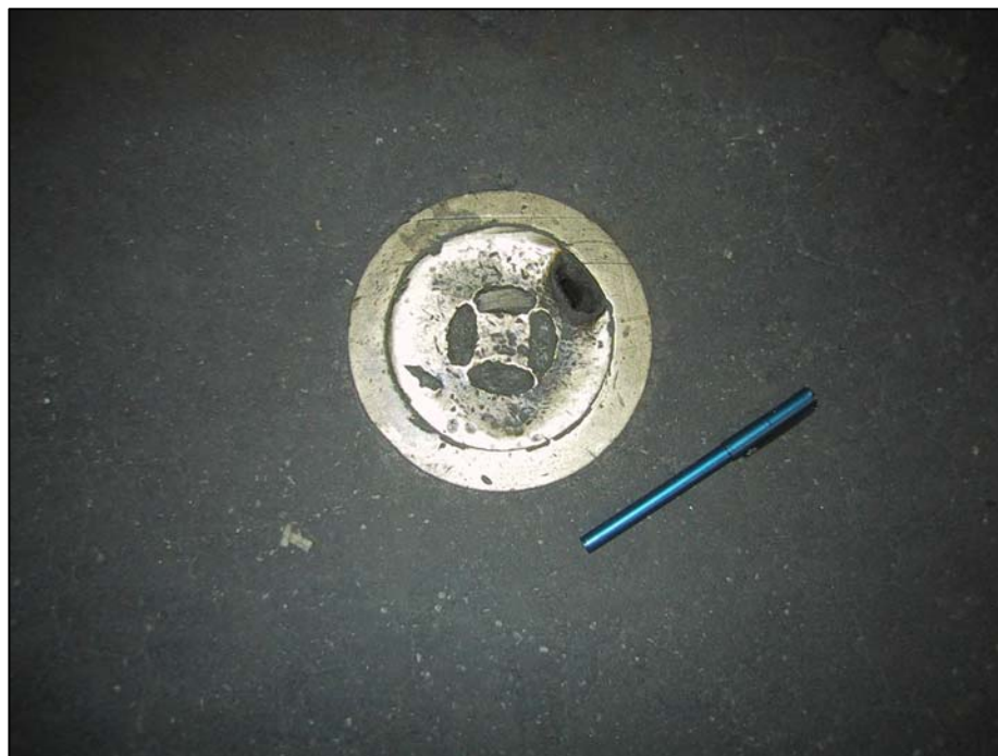
Photograph 7. Suspect fill cap observed in the basement of the three-story warehouse structure. Several such fill caps were noted in the basement of this structure.
