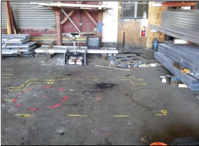
Two UST manhole covers, facing north
