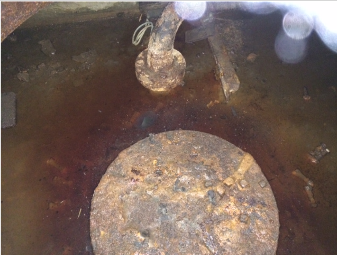
2. Top of UST, in vault
