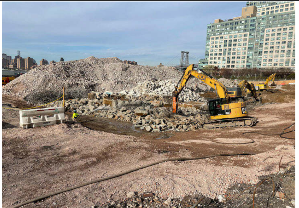
Photo 2: Hammering concrete from former building footings
