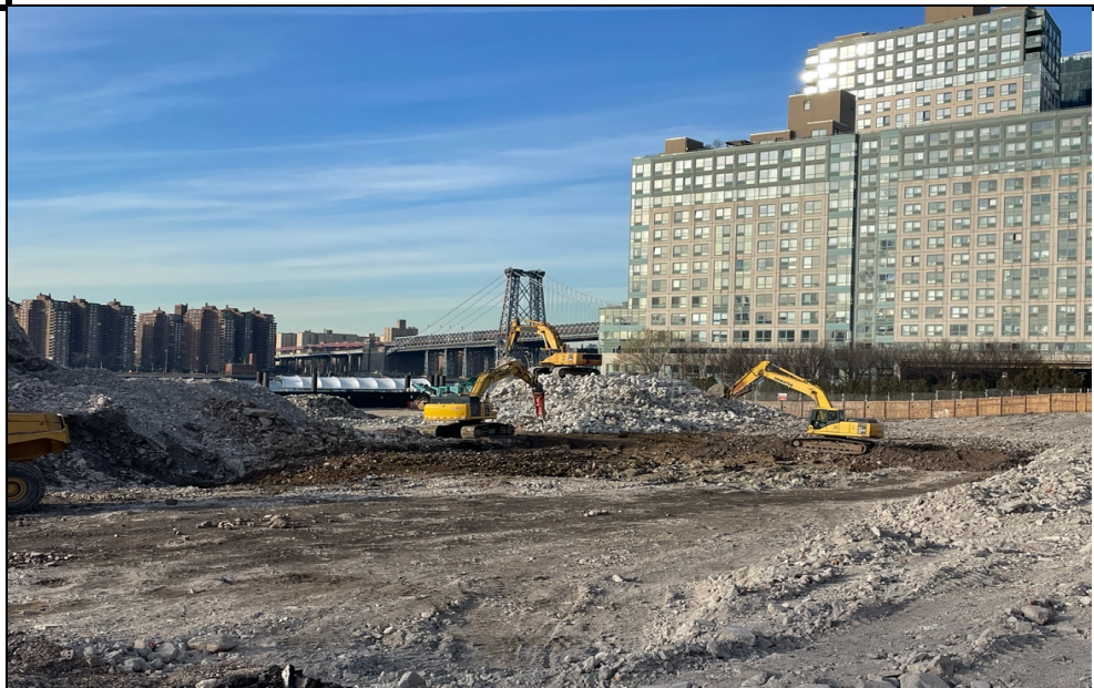
Photo 2: Breaking up concrete debris from the building slab and footings demolition.
