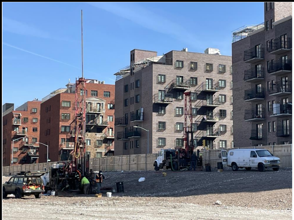
Photo 1: Completing geotechnical boring B-27 and beginning B-25.
