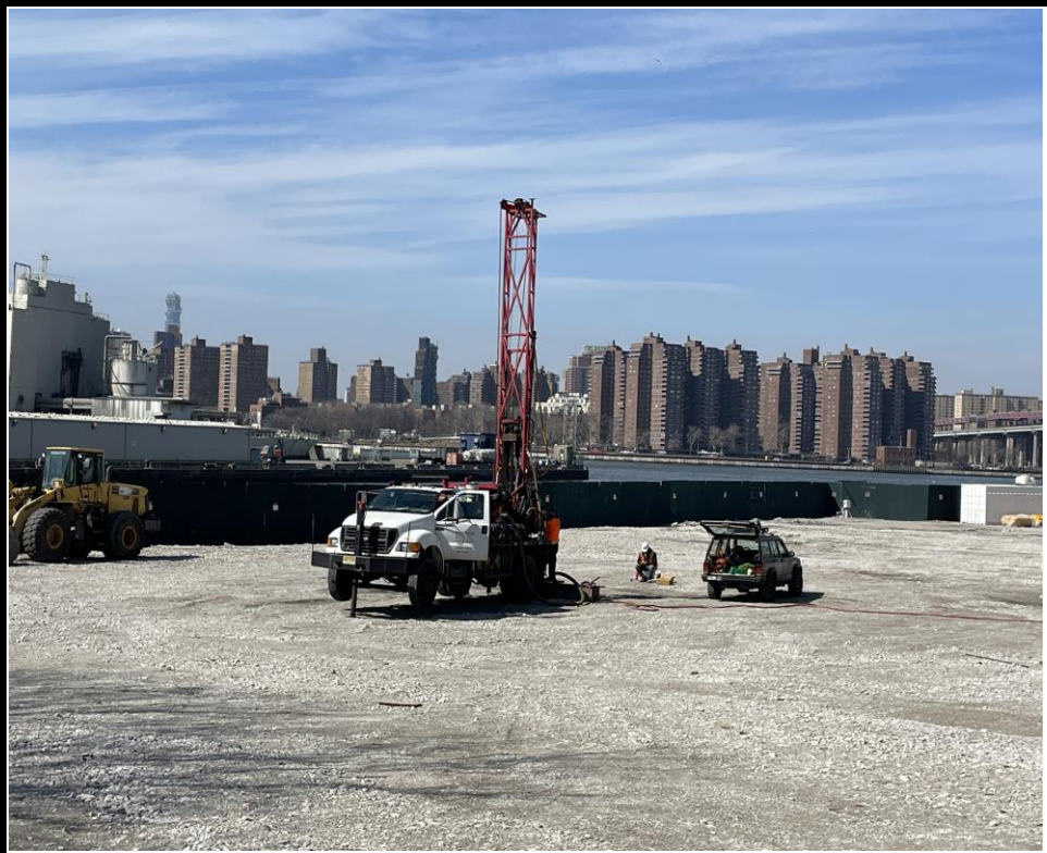
Photo 2: Advancing geotechnical boring B-12.
