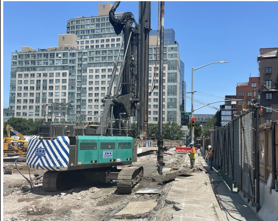
Photo 2: View of pile installation for support of excavation.
