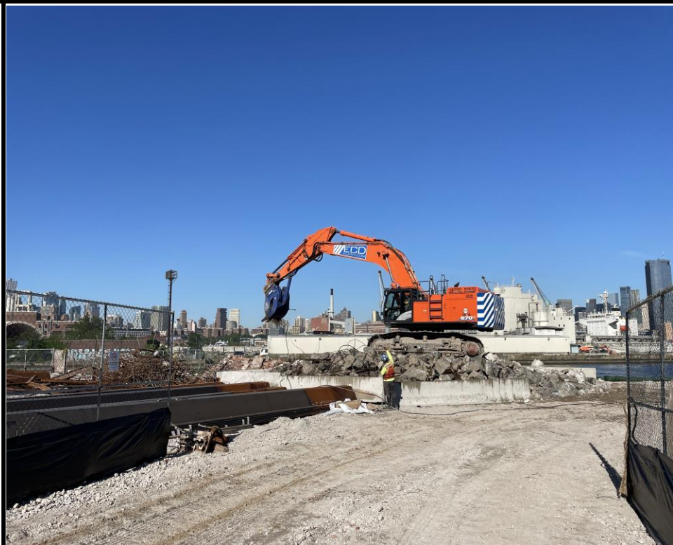
Photo 2: ECD breaking up concrete from marine bulkhead demolition.
