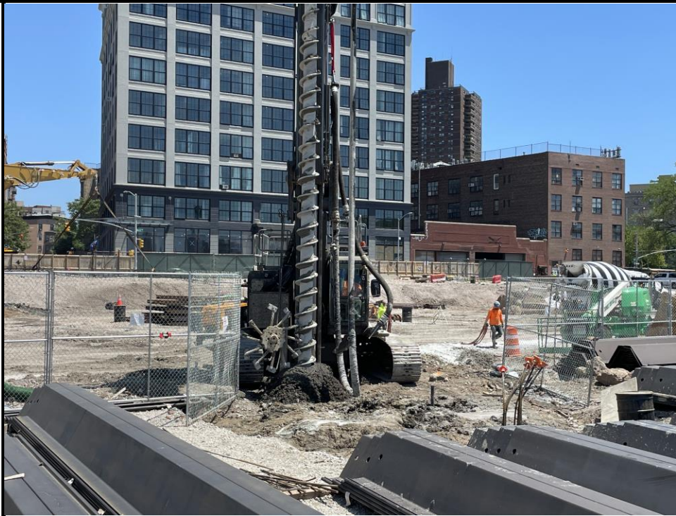
Photo 1: ECD using auger for pile installation.
