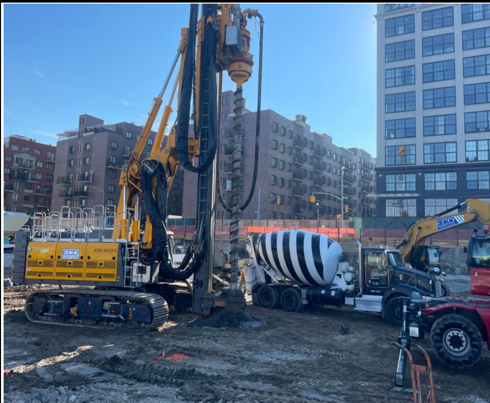
Photo 2: View of pile installation.
