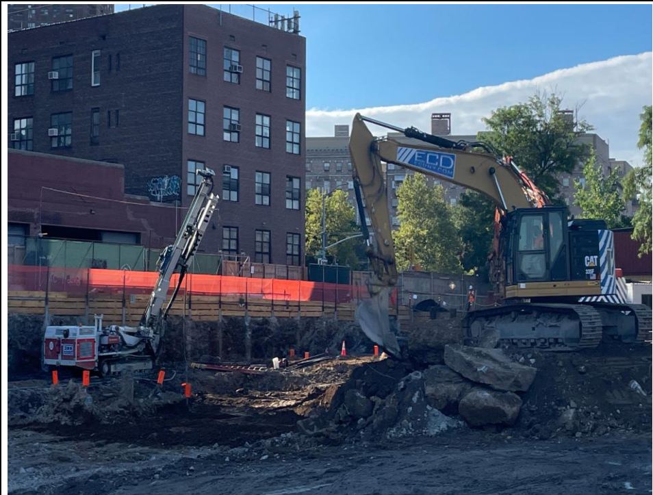
Photo 1: Soil excavation and SOE installation.
