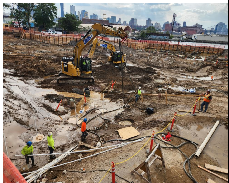
Photo 2: View of dewatering well installation.
