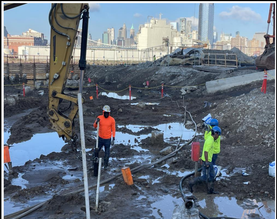
Photo 2: View of dewatering well installation.
