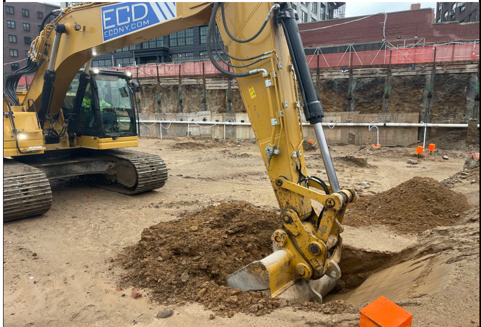
Photo 1: View of excavating test pits.
