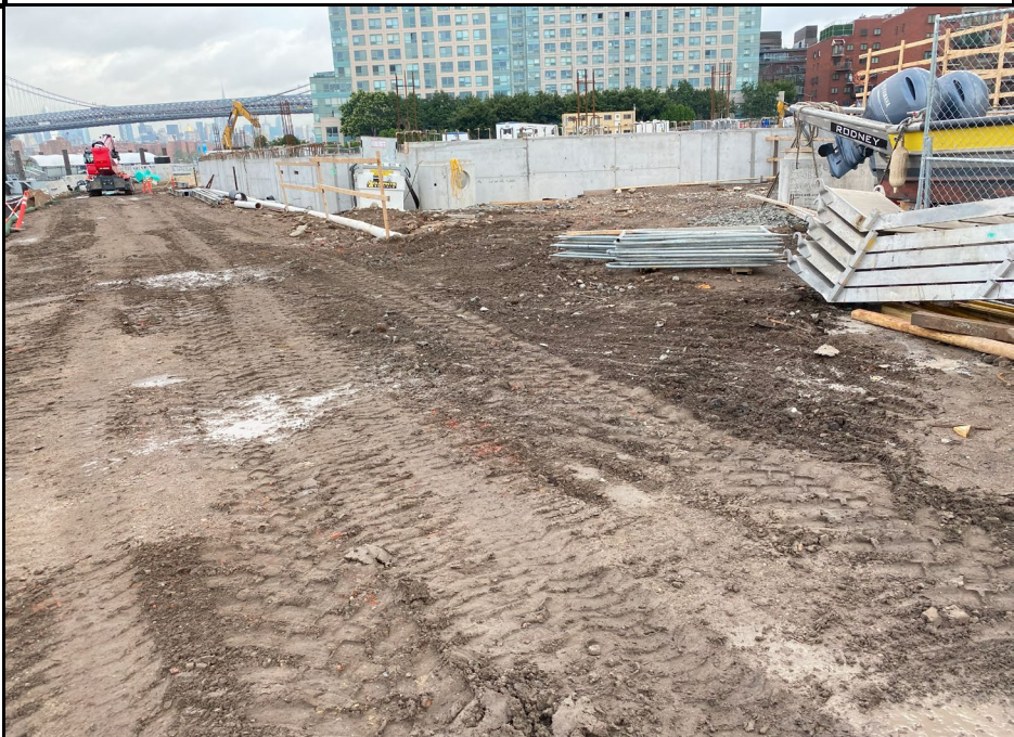
Photo 2: View of Site facing northwest.
