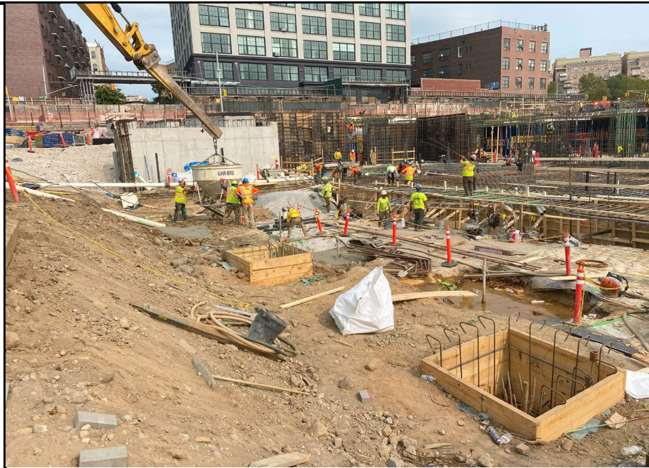
Photo 3: View of excavation and soil work.
