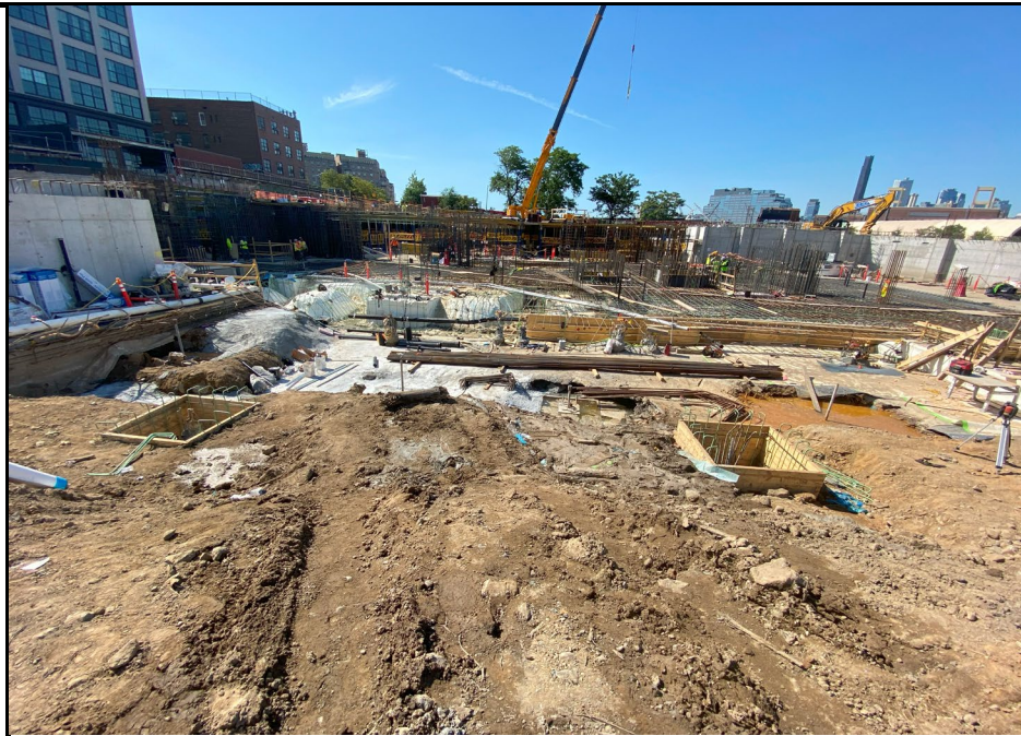
Photo 3: View of excavation and soil work.
