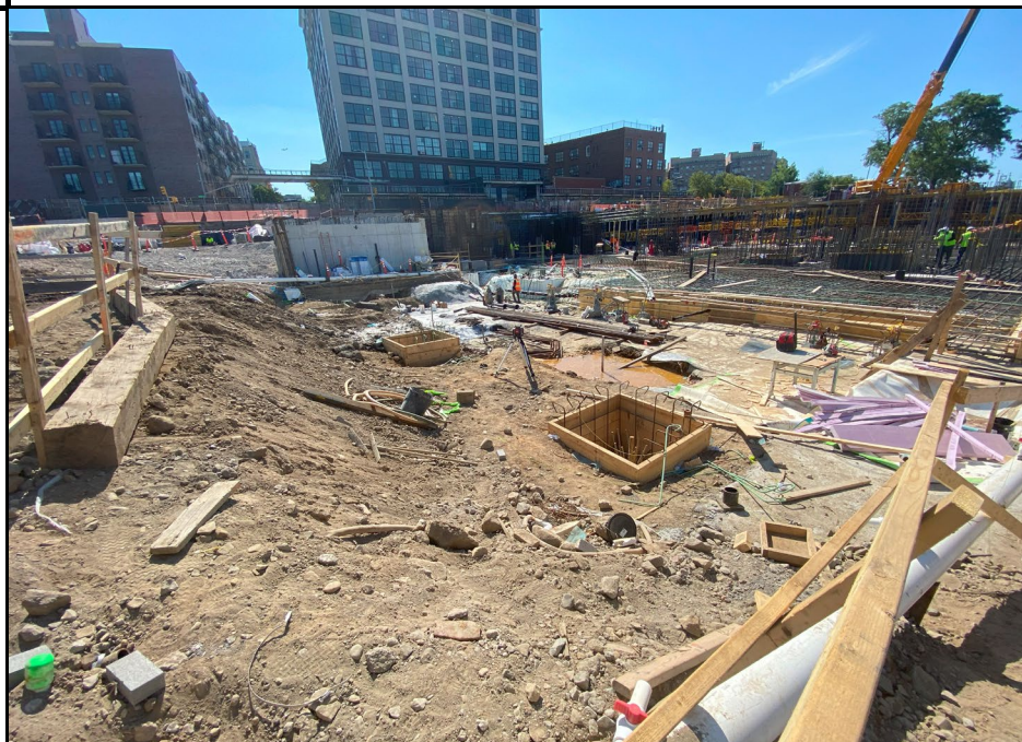
Photo 4: View of rebar and foundation form work.
