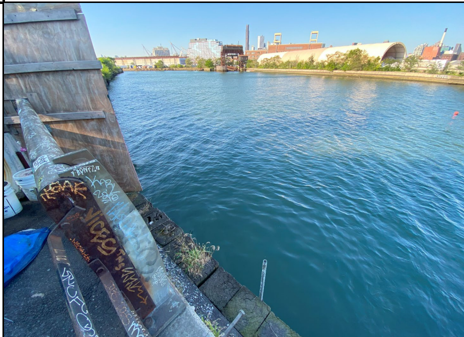
Photo 4: View of outfall on Division Ave facing Wallabout Channel.
