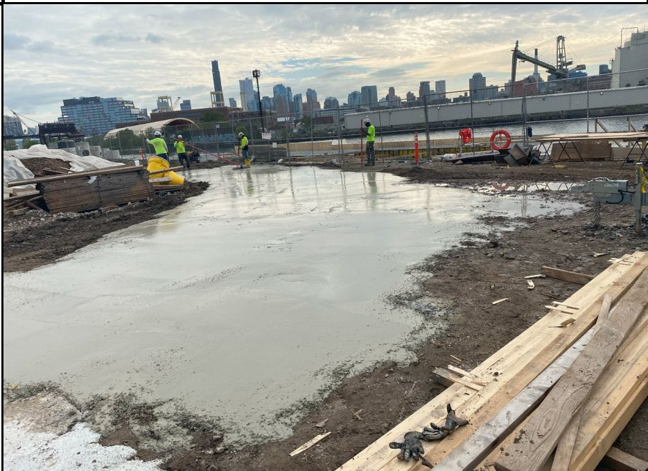
Photo 2: View of the Site facing south.
