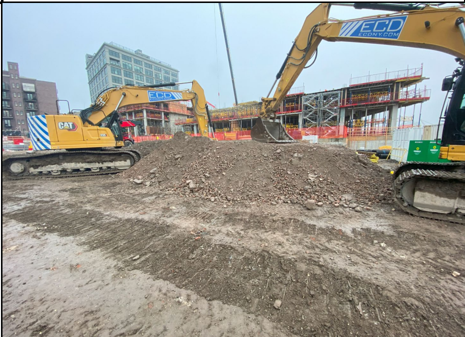
Photo 2: View of the minor soil work on Site.
