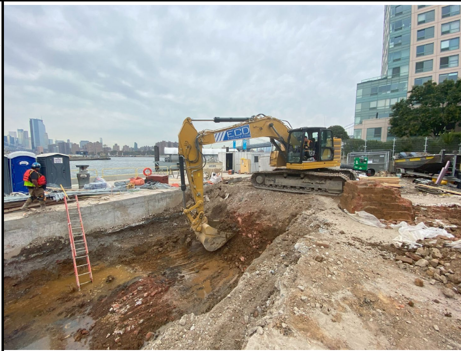
Photo 3: View of ECD continuing to develop the bulhead in the marine area.
