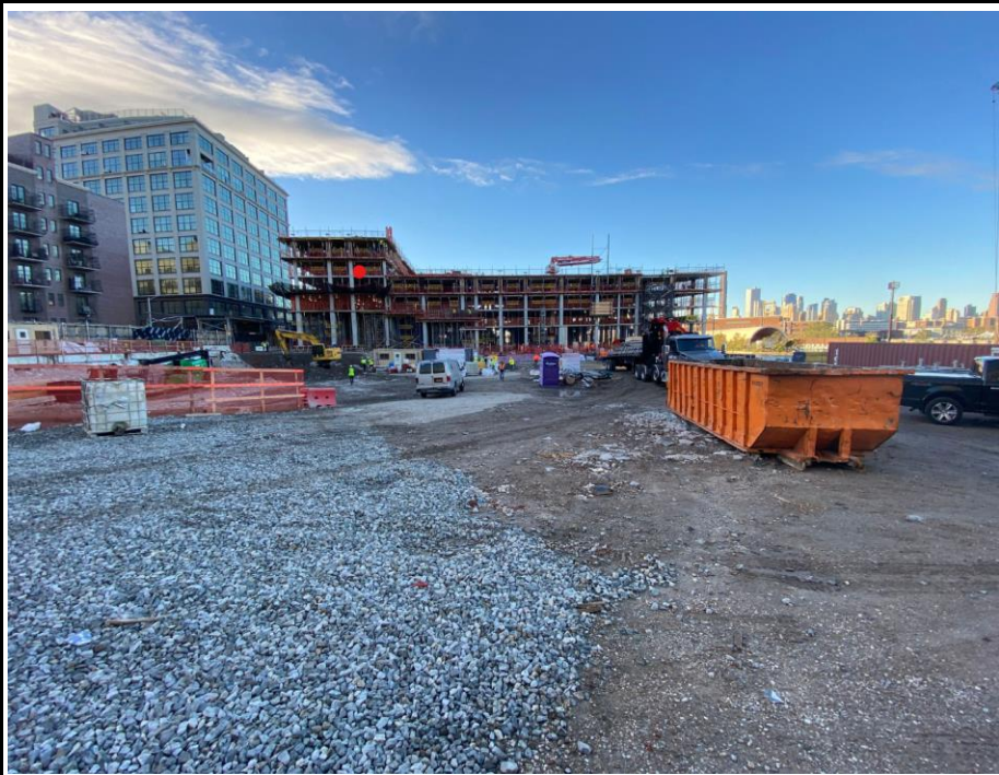
Photo 1: View of the Site facing south.
