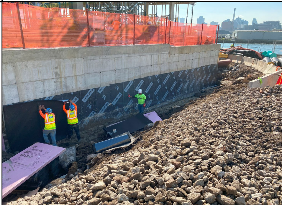
Photo 4: View of the waterproofing work on the foundation wall.
