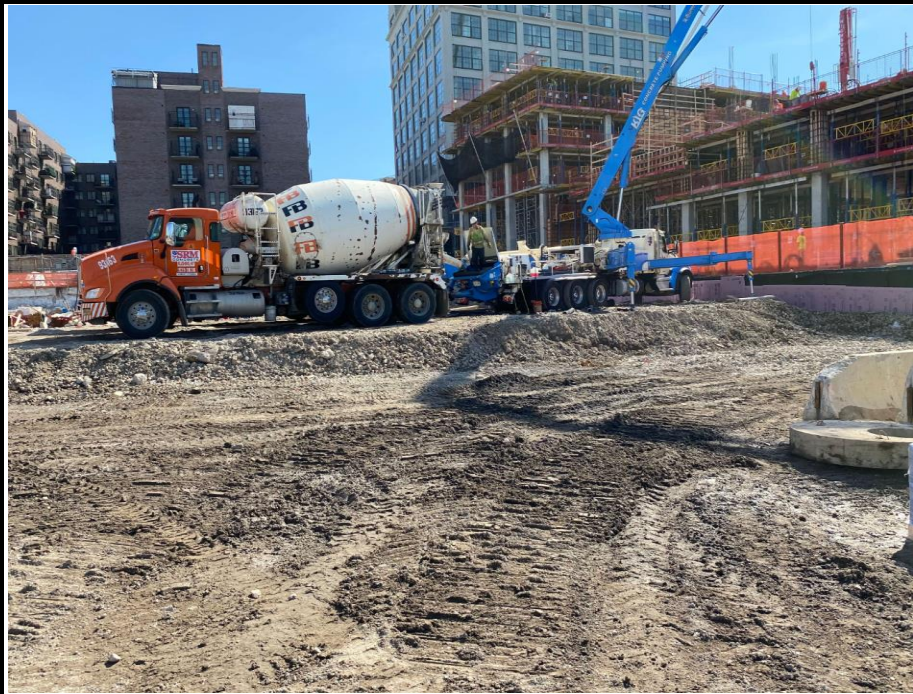
Photo 3: View of the Site facing north.
