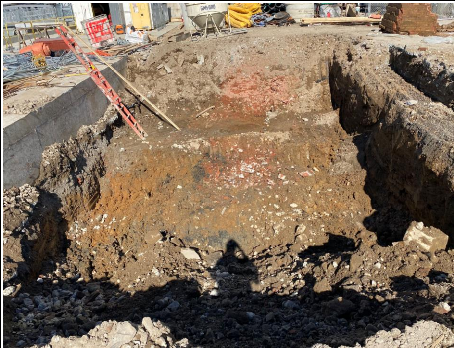
Photo 1: View of the PWSB- 16/PWSB-17 remedial excavation.
