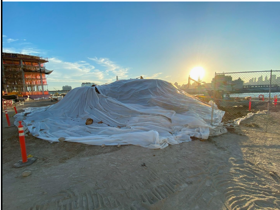
Photo 4: View of covered soil stockpile.
