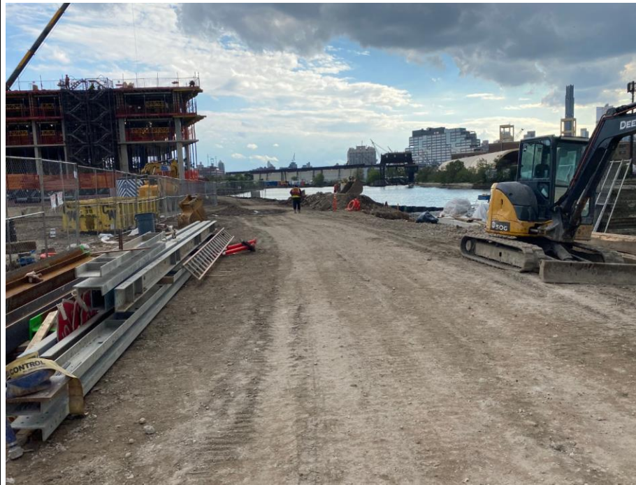
Photo 3: View of the Site facing south.
