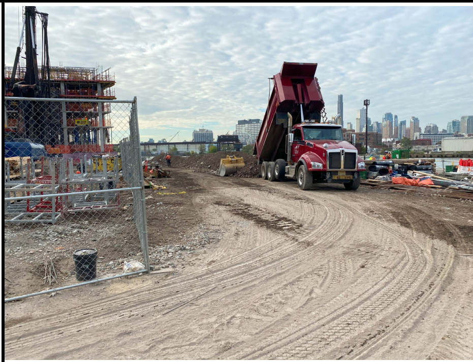
Photo 3: View of Alba stockpiling RCA.
