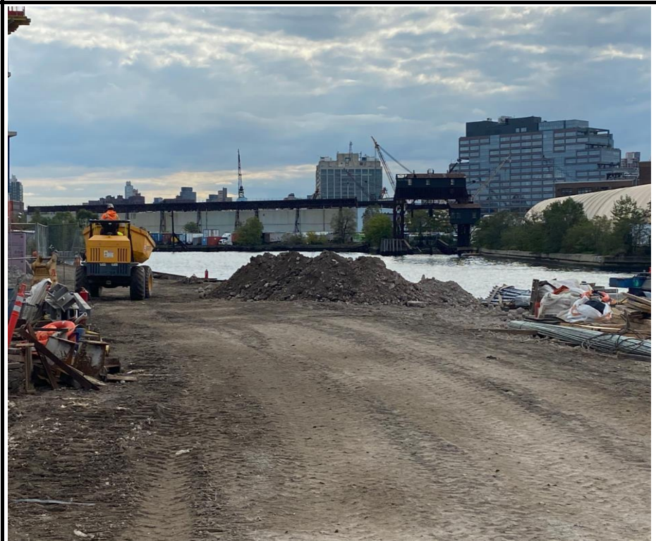
Photo 4: View of Alba stockpiling RCA.
