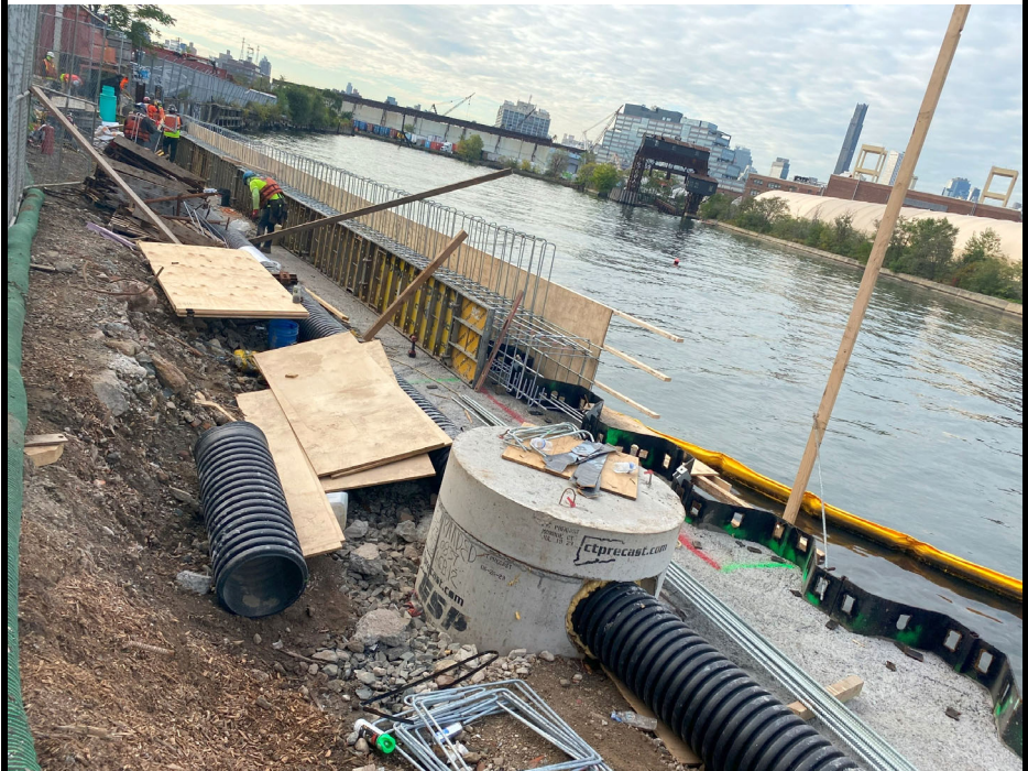
Photo 2: View of ECD continuing bulkhead work in the marine area.
