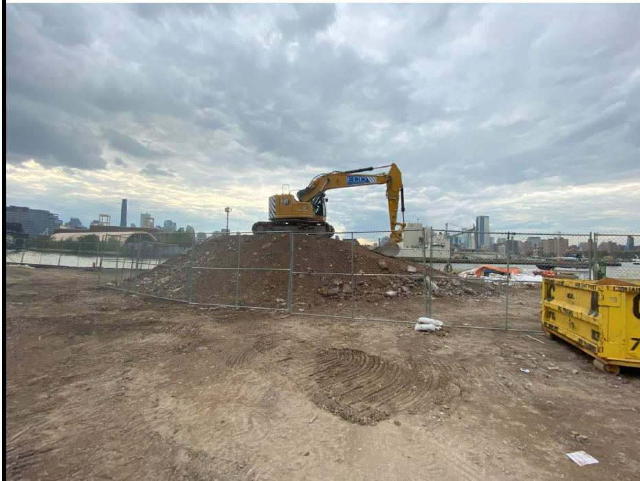
Photo 4: View of Alba stockpiling RCA.
