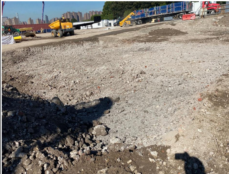
Photo 3: View of RCA in A3 area.
