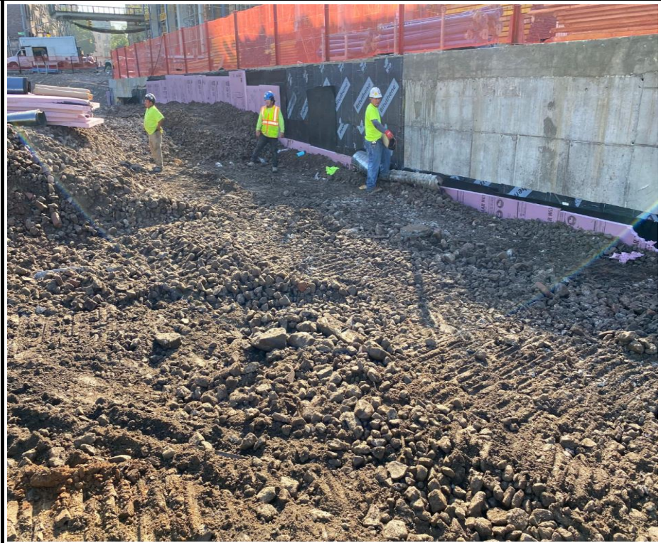
Photo 4: View of the waterproofing work on the sub-grade foundation wall.
