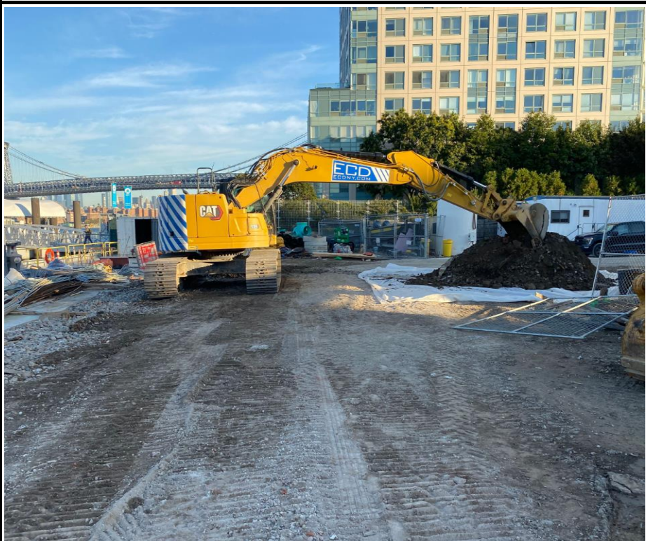
Photo 2: View of PWSB- 16/PWSB-17 remedial excavation.
