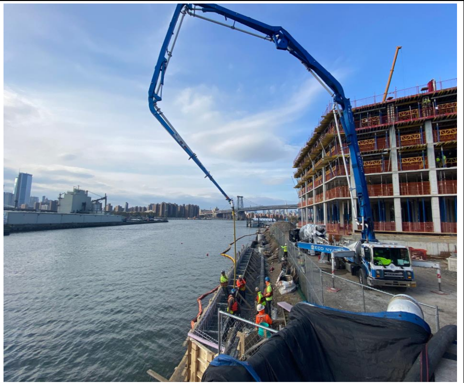
Photo 2: View of ECD continuing bulkhead work in the marine area.
