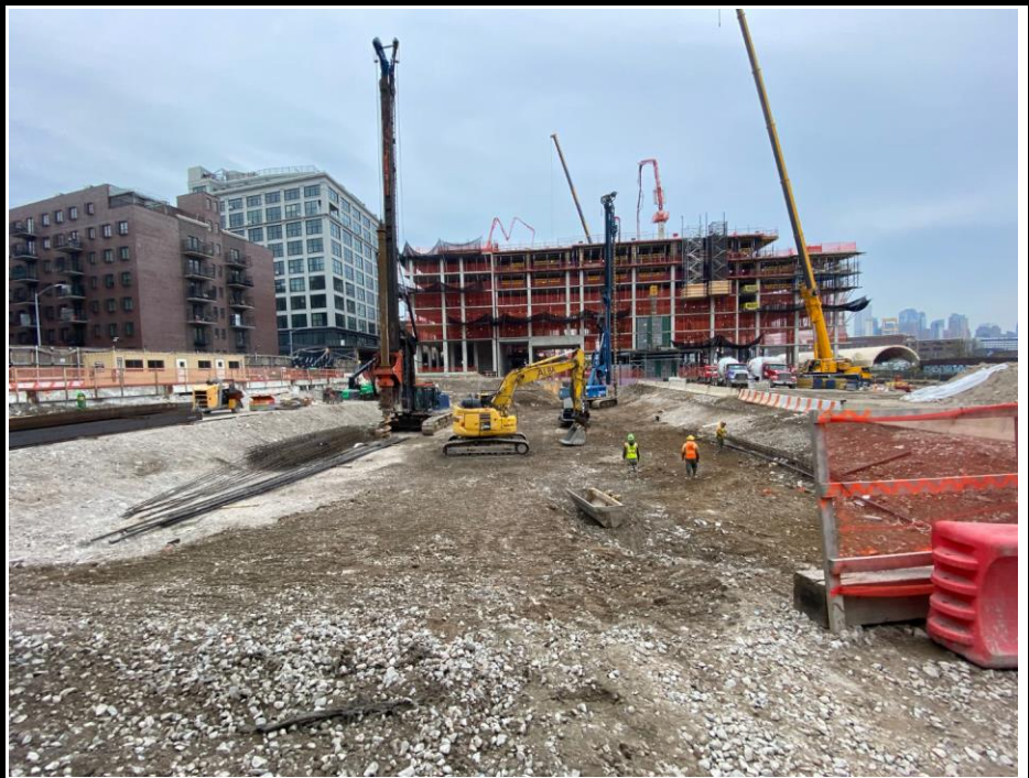
Photo 1: View of the Site facing south,
