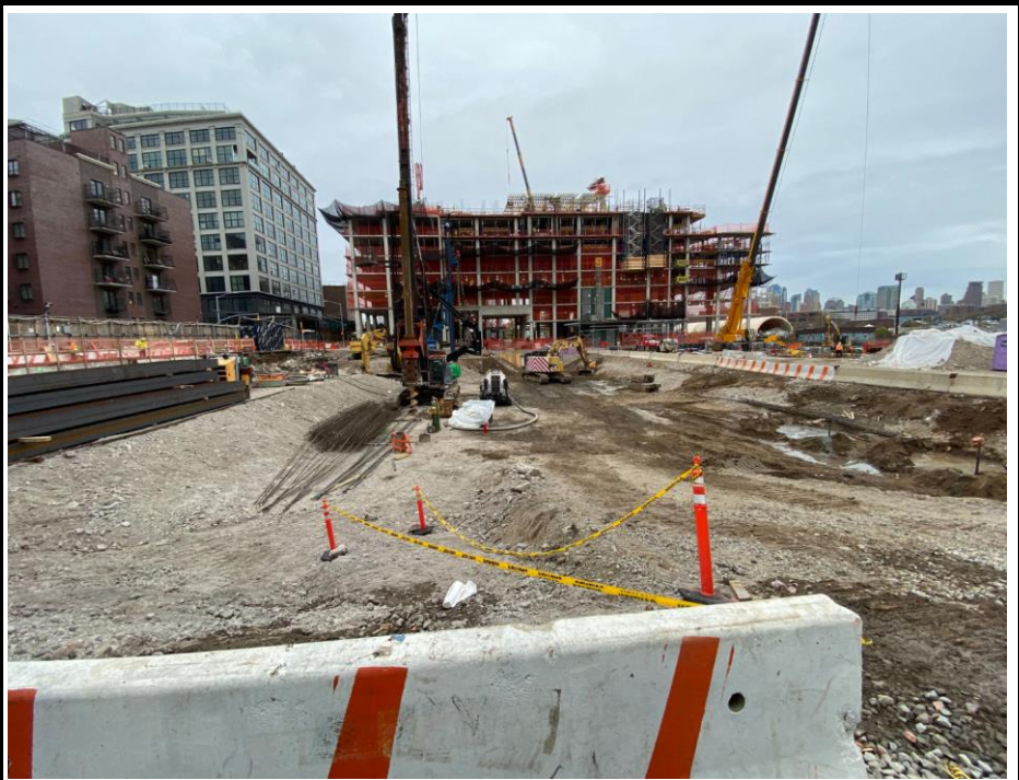
Photo 1: View of the Site facing south.
