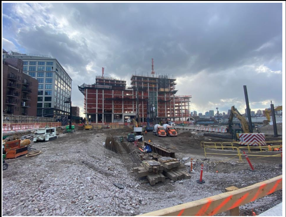
Photo 1: View of the Site facing south.
