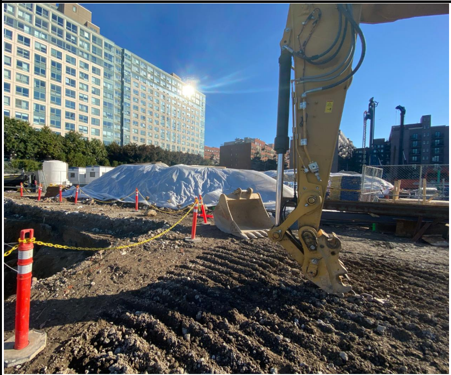
Photo 4: View of covered stockpiles.
