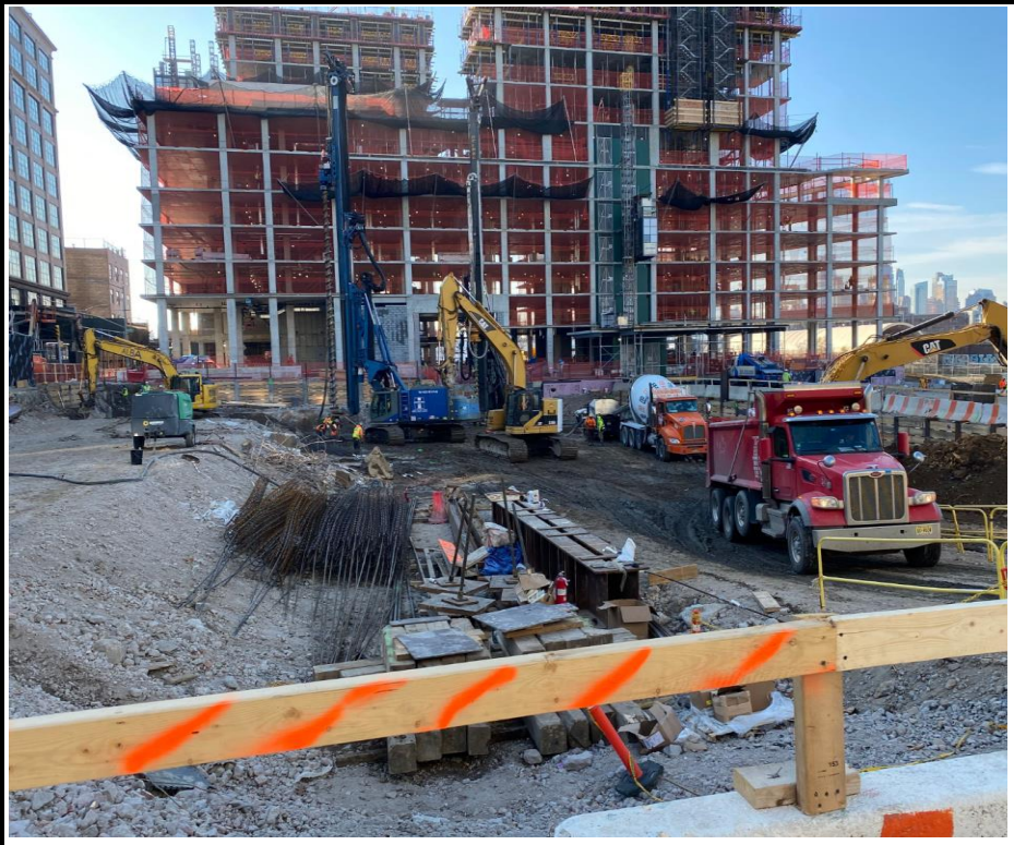
Photo 4: View of site conditions facing south.
