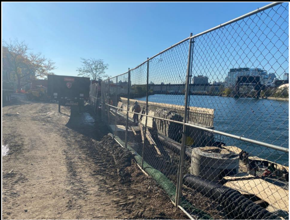
Photo 3: View of continued work in the bulkhead in the marine area.
