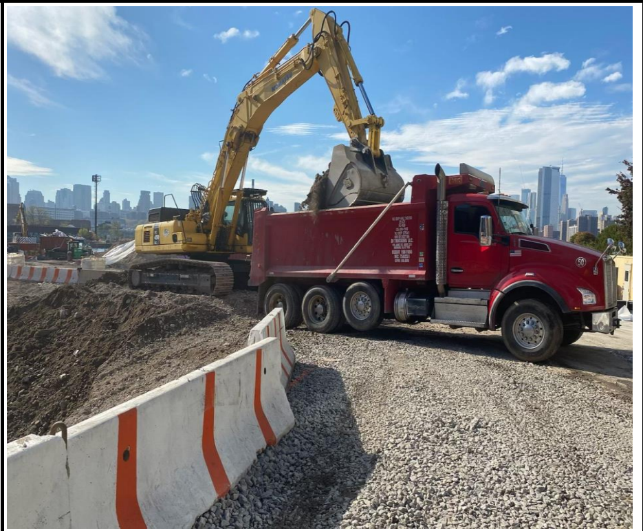
Photo 2: View of truck loading for off-site soil disposal.
