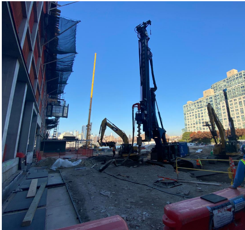
Photo 2: View of drilling and pile installation facing west.
