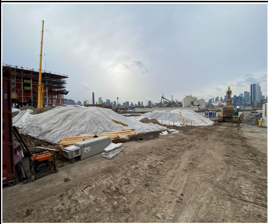
Photo 4: View of covered stockpiles.
