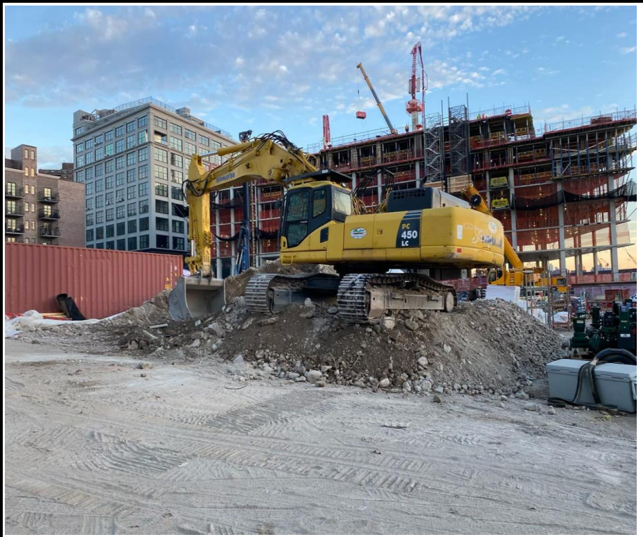
Photo 4: View of staged equipment at the end of the work day.
