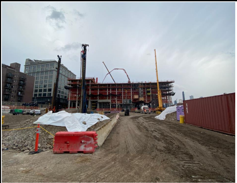
Photo 3: View of the Site facing south.
