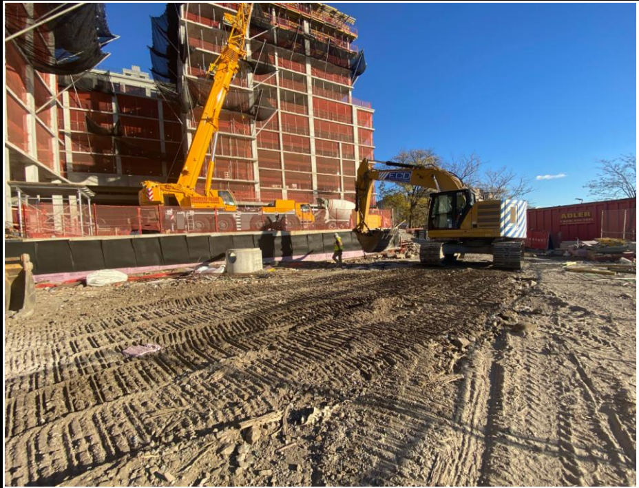
Photo 3: View of continued waterproofing installation and structure development.
