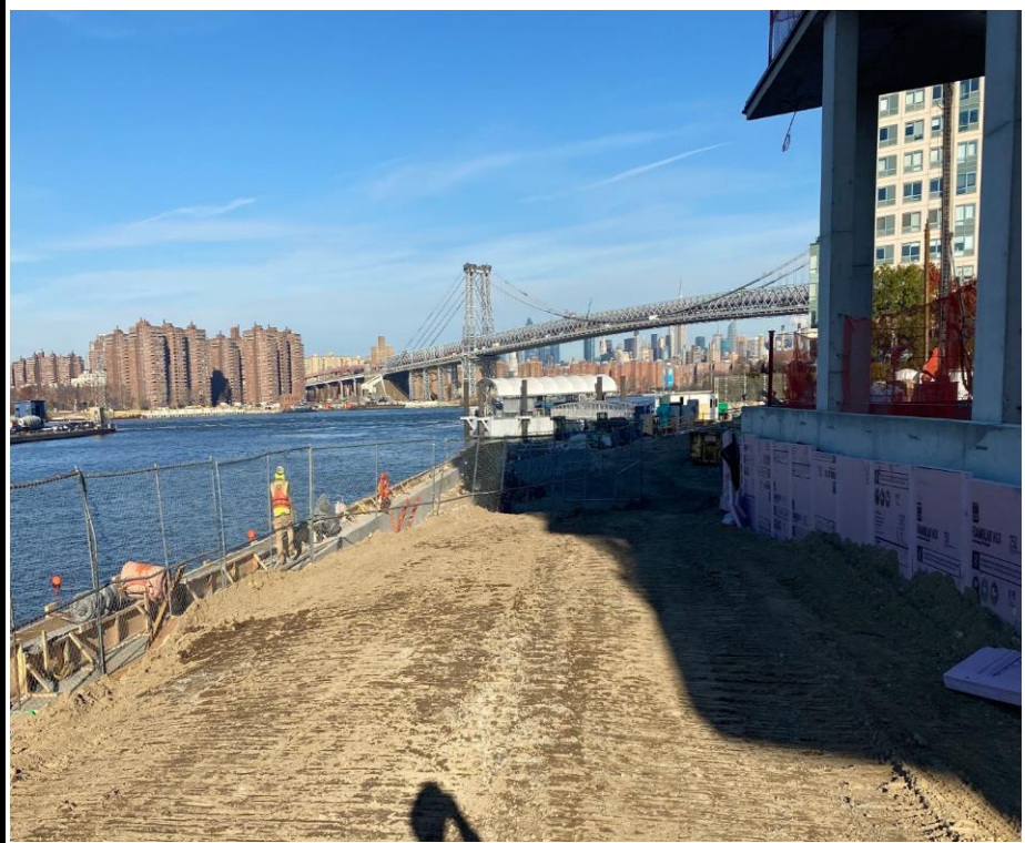
Photo 2: View of the marine area and continued waterproofing installation.
