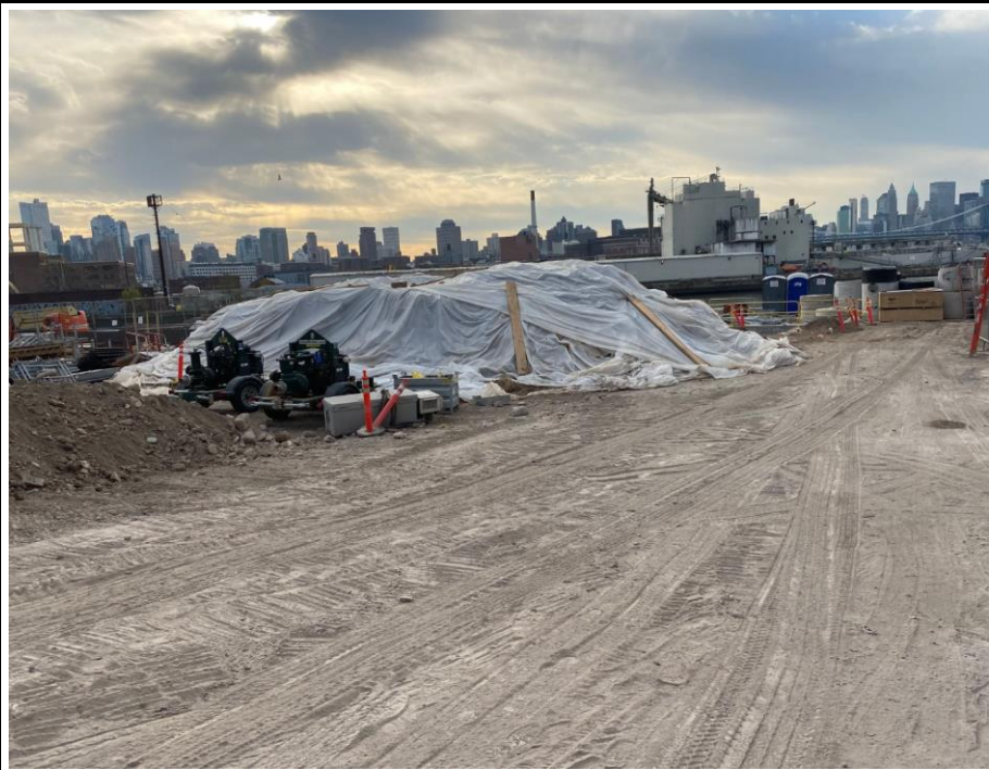
Photo 3: View of covered stockpile.
