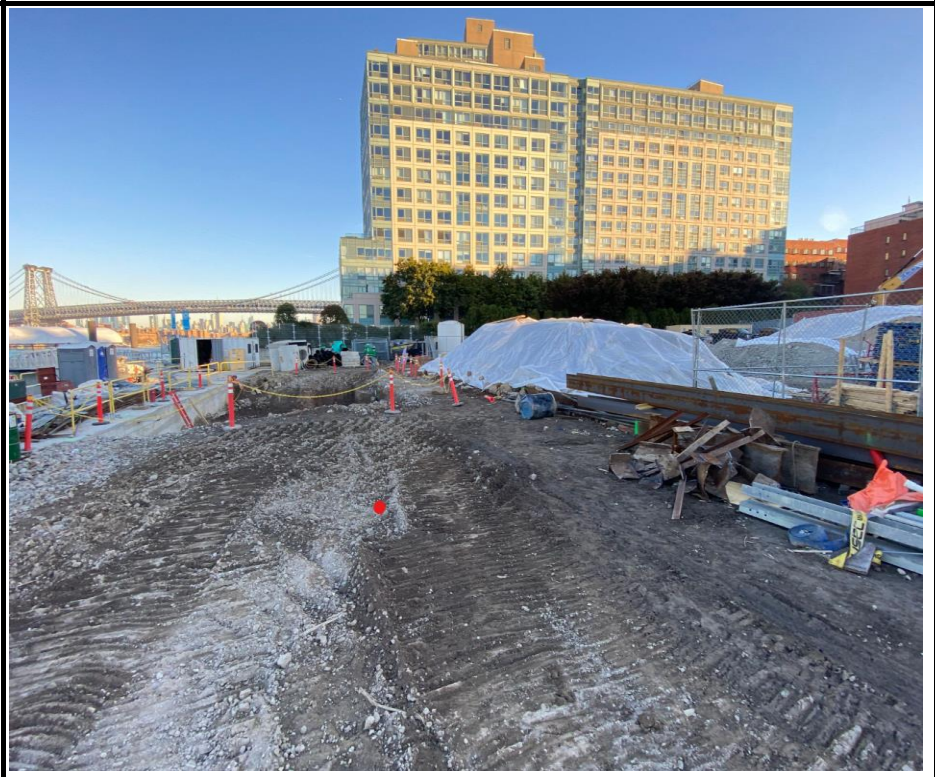
Photo 2: View of the Site facing north.
