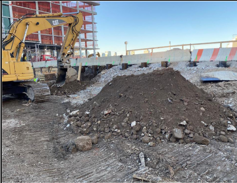
Photo 3: View of soil excavation for off- site disposal.
