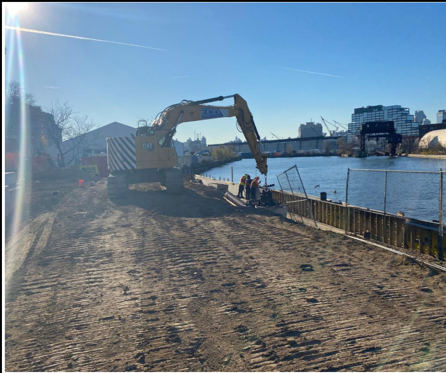
Photo 4: View of continued work on the bulkhead in the marine area.
