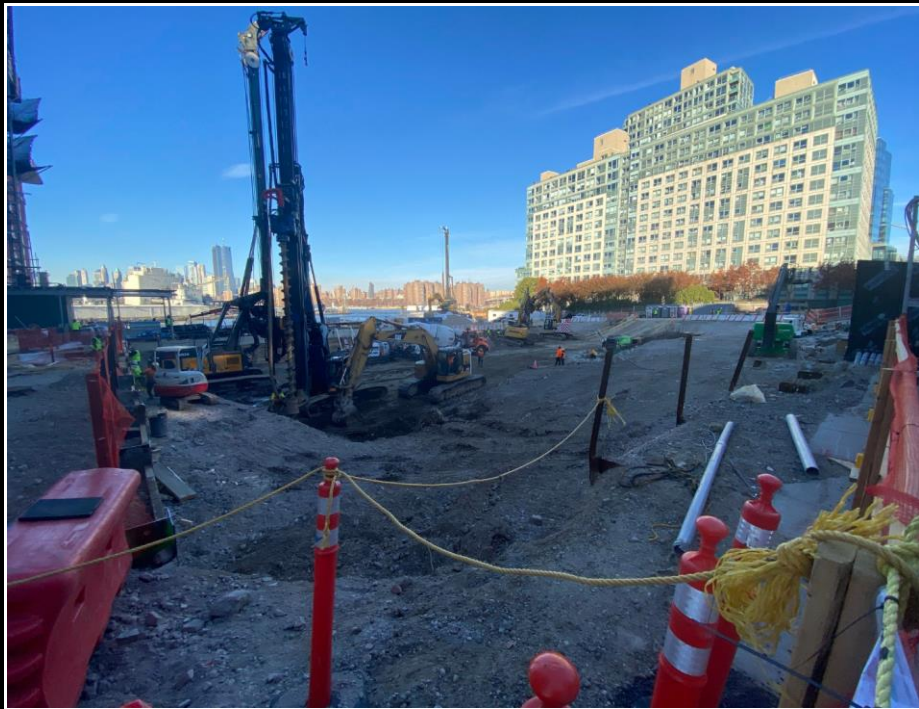
Photo 3: View of soil excavation and pile installation.
