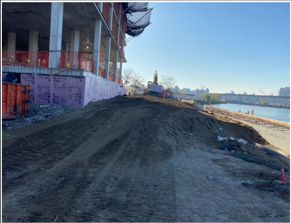
Photo 3: View of imported soil for use as general backfill in the marine area.
