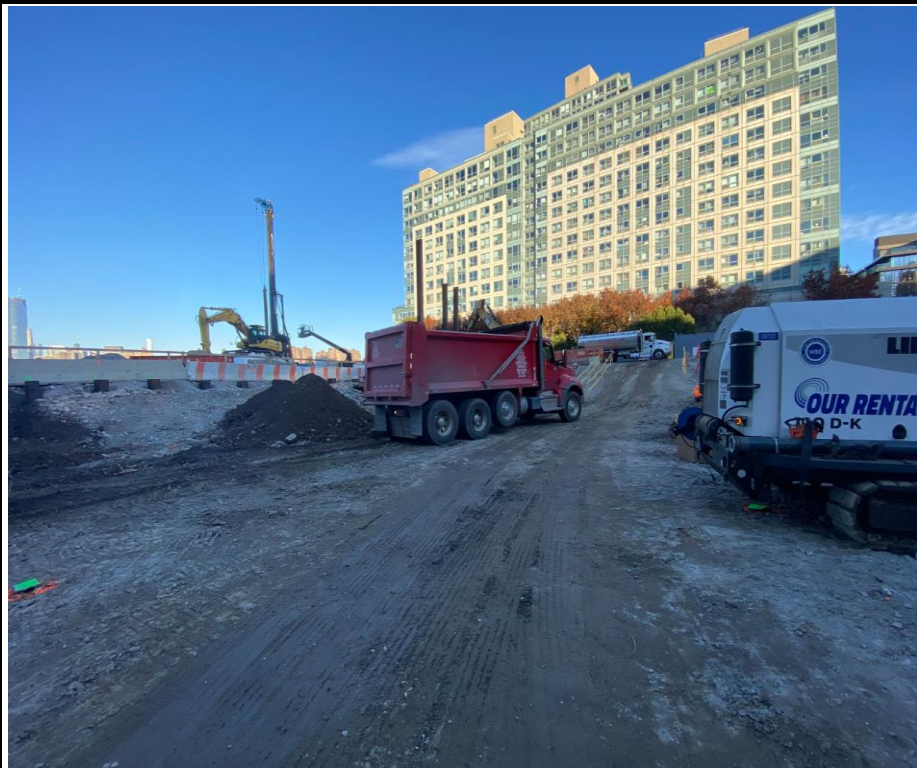
Photo 4: View of the truck loading for off-site disposal of material.
