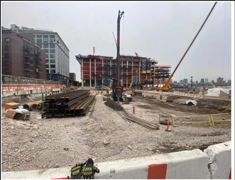
Photo 1: View of the Site facing south.
