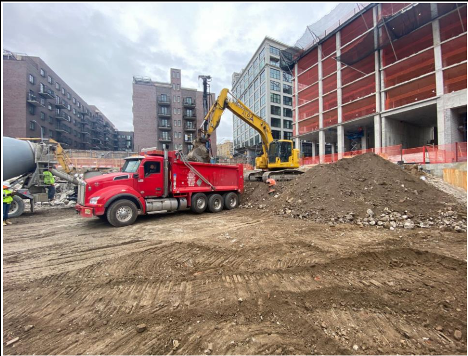
Photo 3: View of truck loading for off-site soil disposal.
