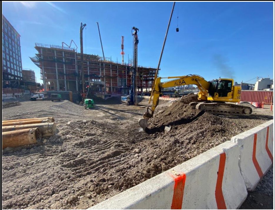
Photo 1: View of the Site facing south.
