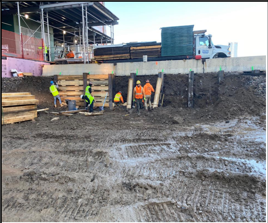
Photo 2: View of lagging installation for SOE.
