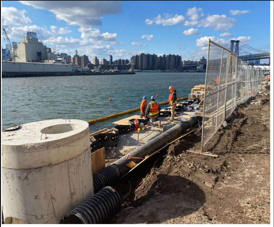
Photo 2: View of the continued bulkhead work in the marine area.
