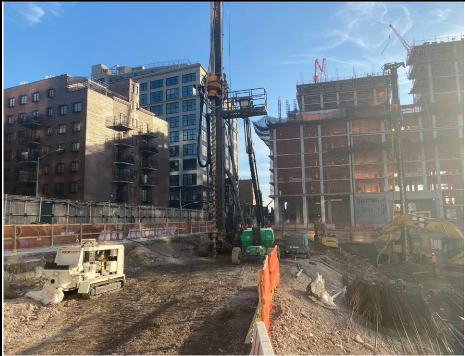
Photo 3: View of soil excavation and pile installation.
