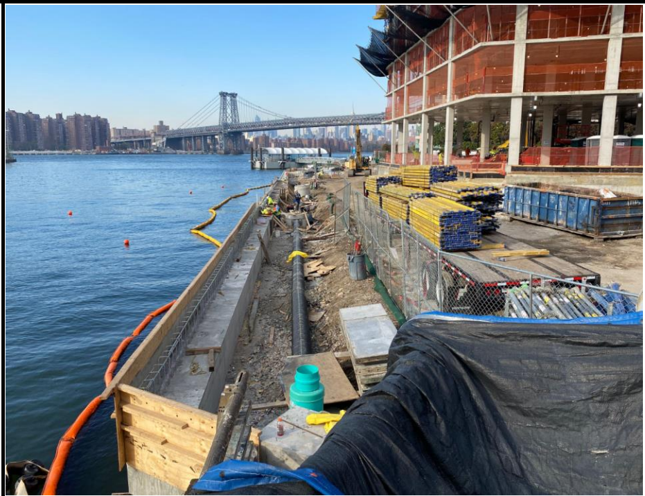
Photo 3: View of the bulkhead development in the marine area.
