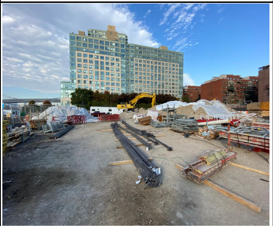
Photo 2: View of the Site facing north.
