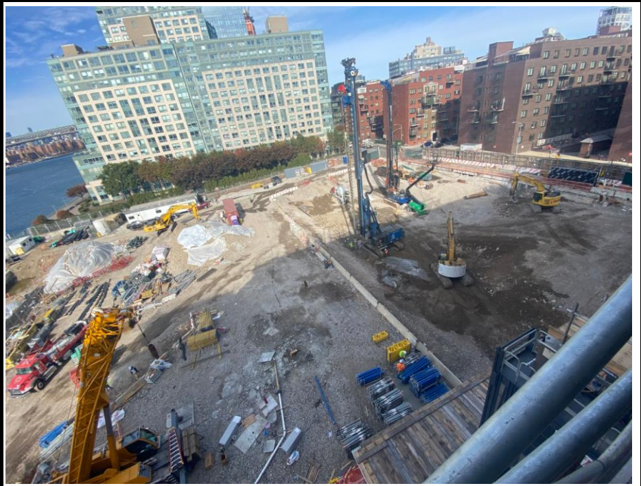
Photo 1: View of the Site facing north,
