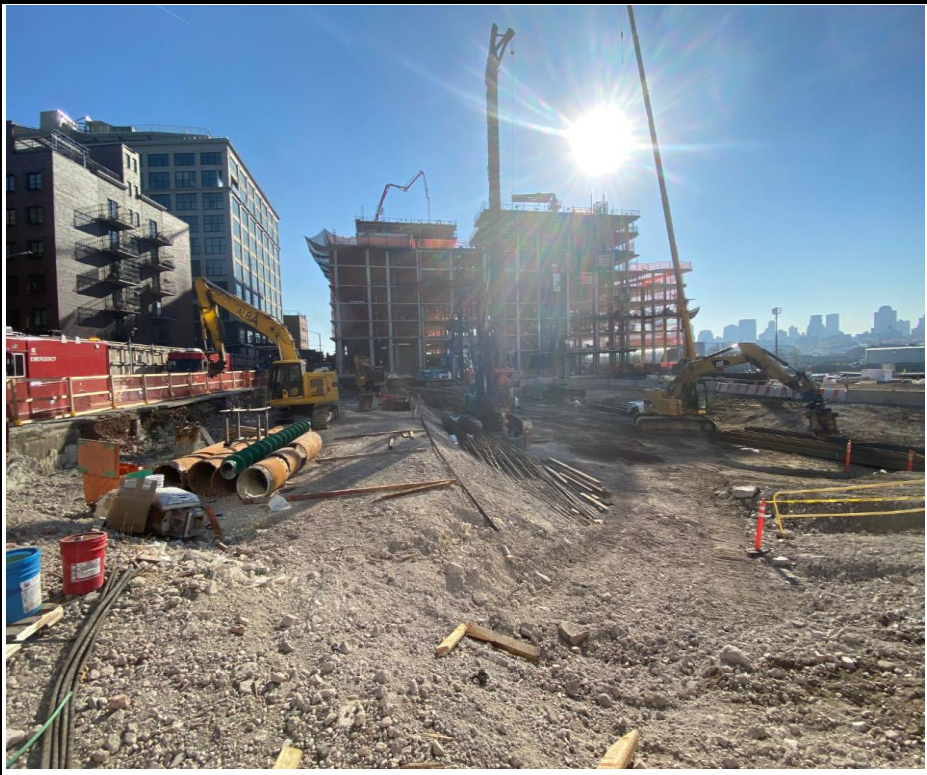
Photo 4: View of the Site facing south.
