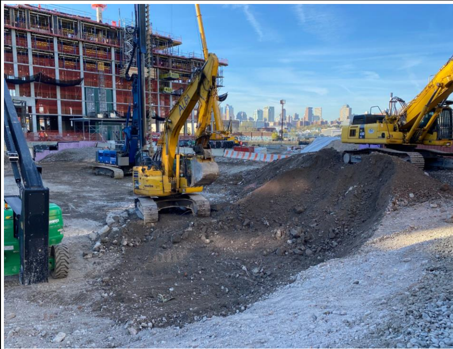
Photo 3: View of Alba continuing soil movement and stockpile relocation.
