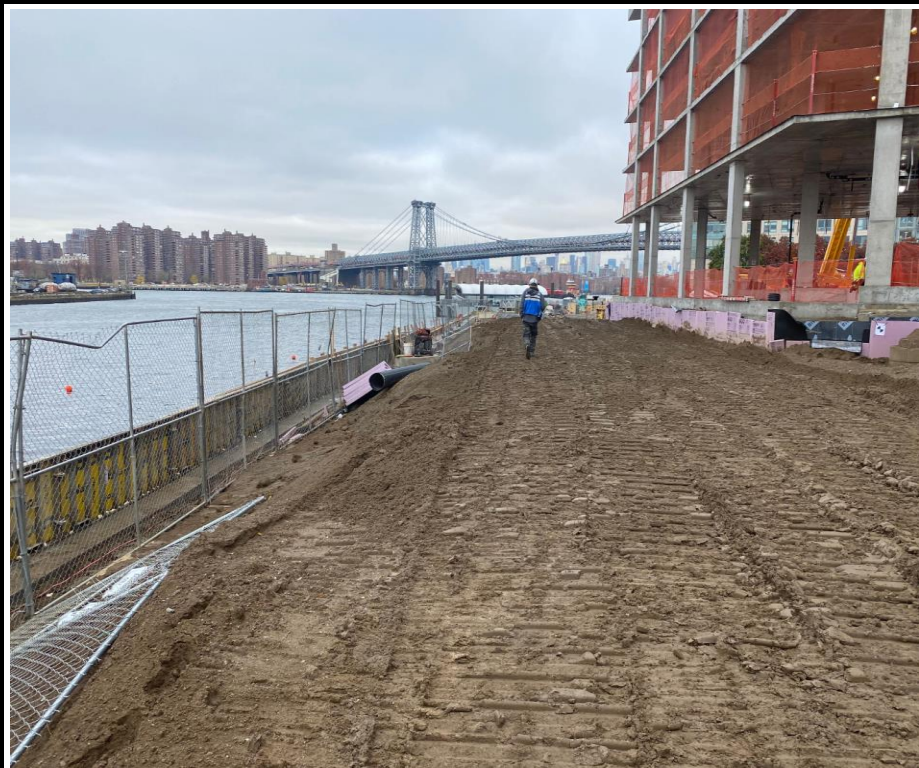
Photo 4: View of continued work on the marine area.
