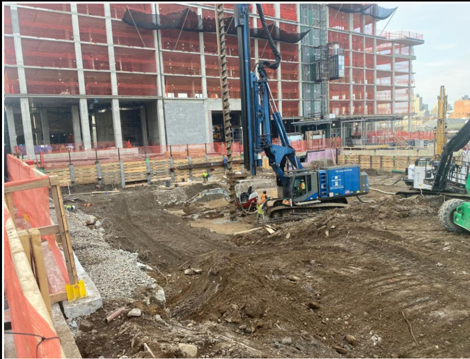
Photo 3: View of soil excavation and pile installation.
