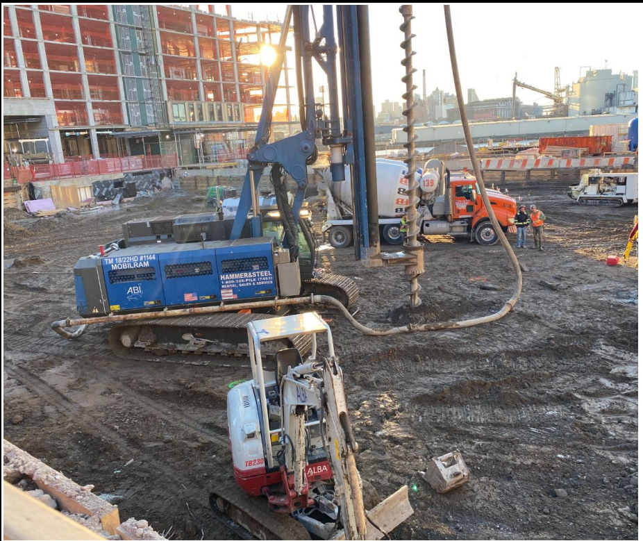
Photo 4: View of drilling for pile installation.
