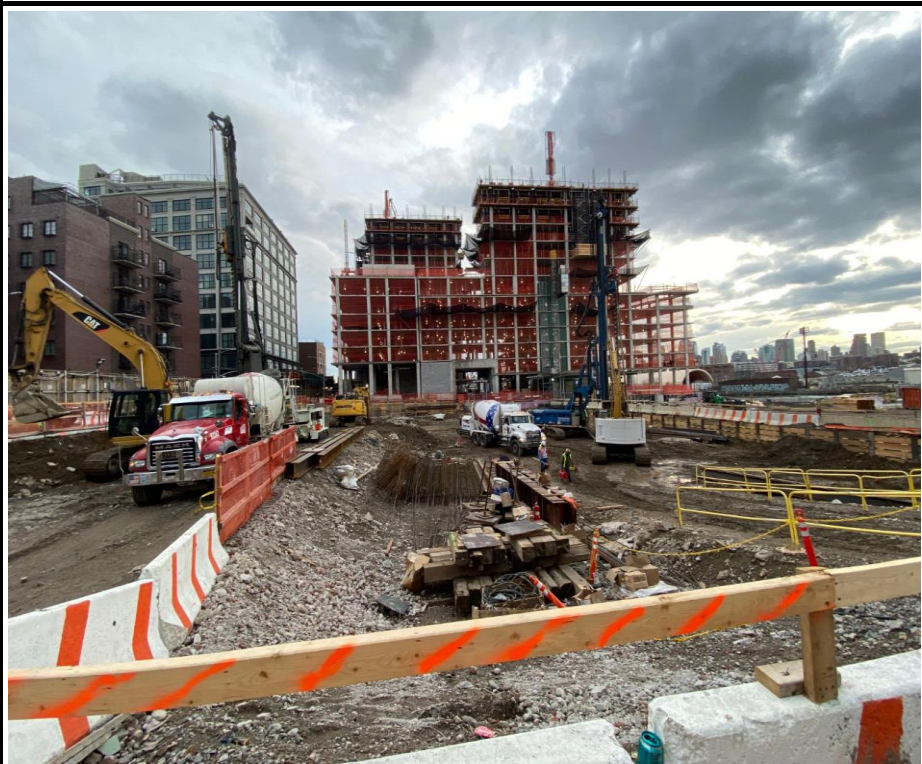
Photo 2: View of site conditions facing south.
