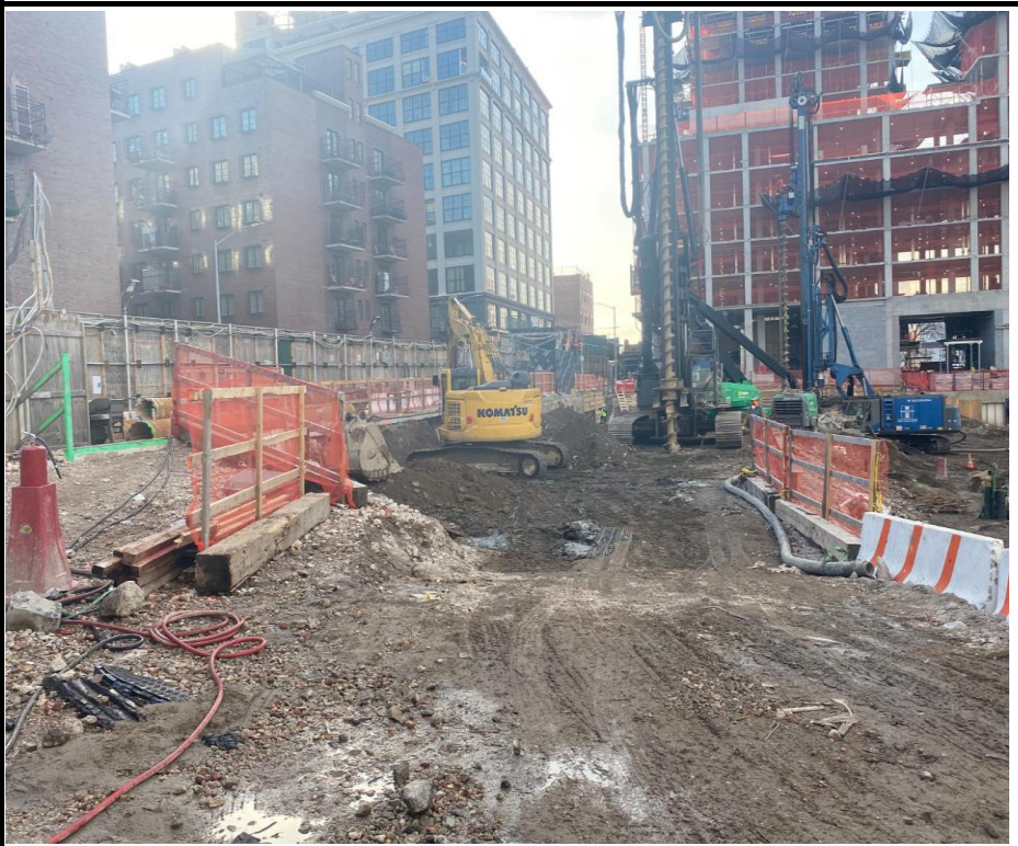
Photo 4: View of soil excavation and pile installation.
