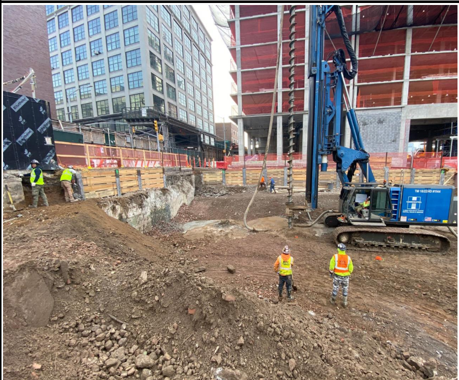
Photo 2: View of drilling and lagging installation for support of excavation.
