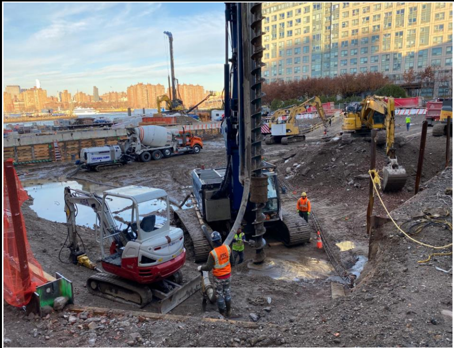
Photo 3: View of soil excavation and pile installation.
