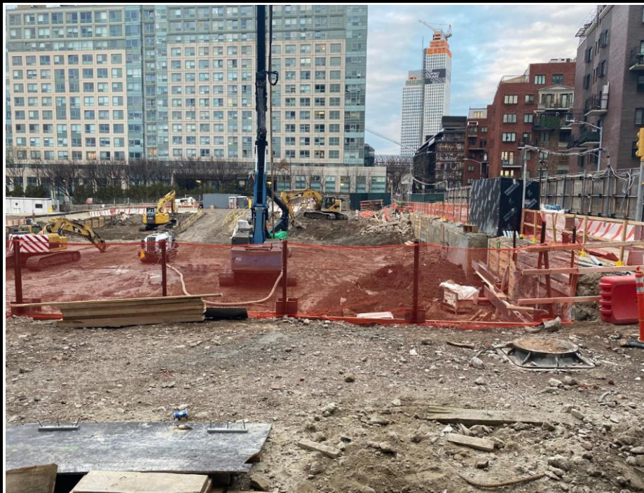
Photo 3: View of the Site facing north.
