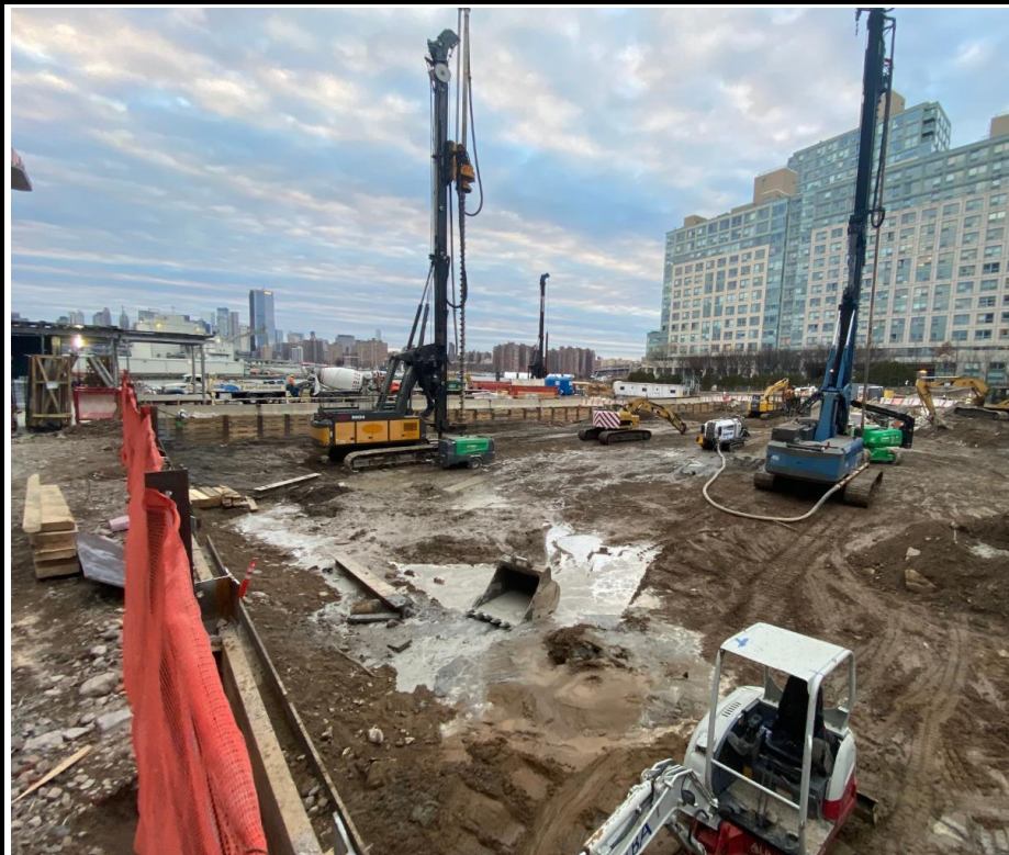
Photo 4: View of drilling for pile installation facing northwest.
