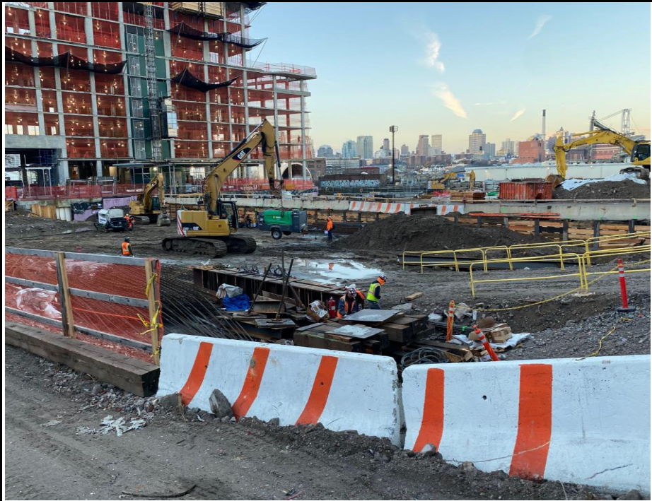
Photo 1: View of the Site facing southwest.
