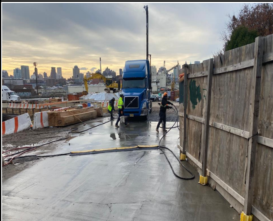
Photo 4: View of vehicle washing prior to leaving the Site.
