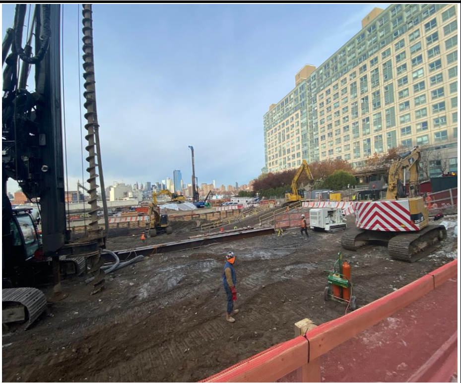
Photo 2: View of site conditions facing northwest.
