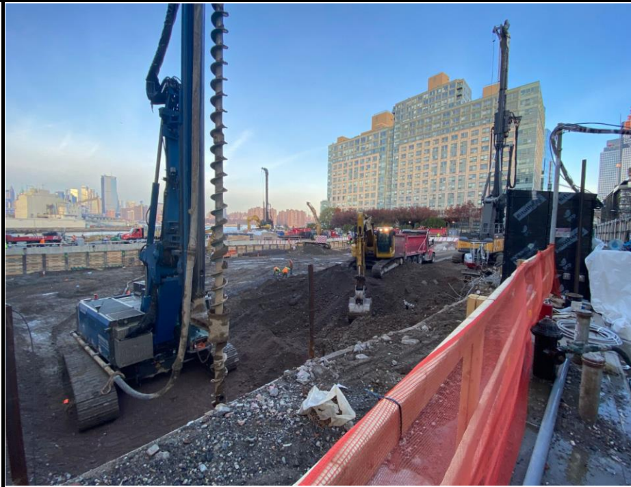
Photo 3: View of soil excavation and pile installation.
