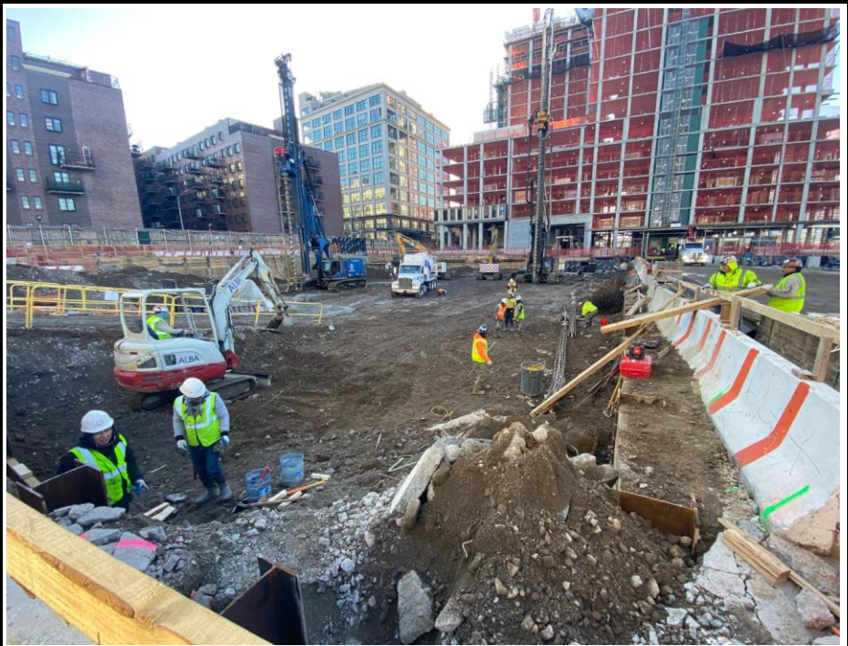
Photo 1: View of drilling for pile installation and site conditions.
