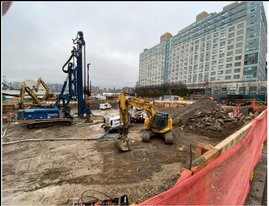
Photo 3: View of site conditions facing northeast.
