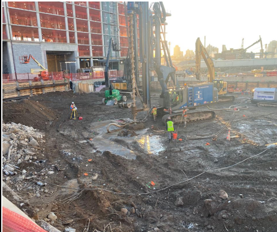
Photo 4: View of drilling for pile installation.
