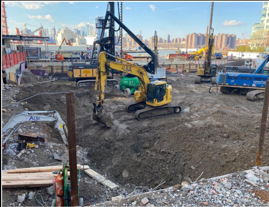
Photo 3: View of soil excavation and pile installation.
