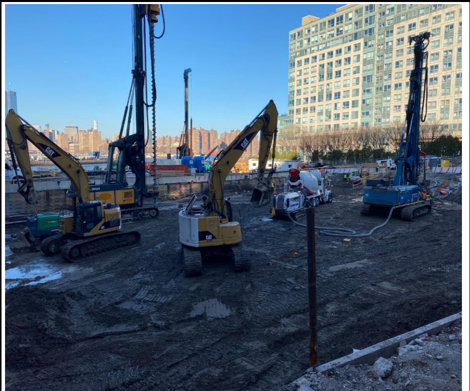
Photo 2: View of excavation and pile installation.
