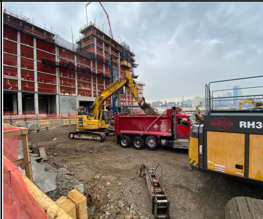
Photo 4: View of truck loading for off-site soil disposal.
