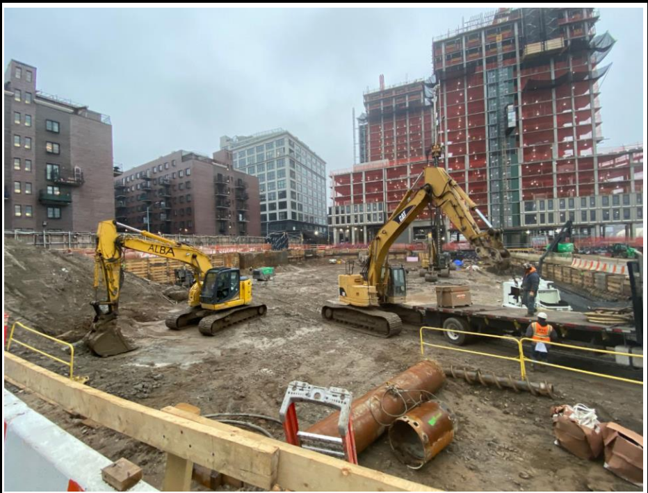
Photo 1: View of Site conditions facing southeast.
