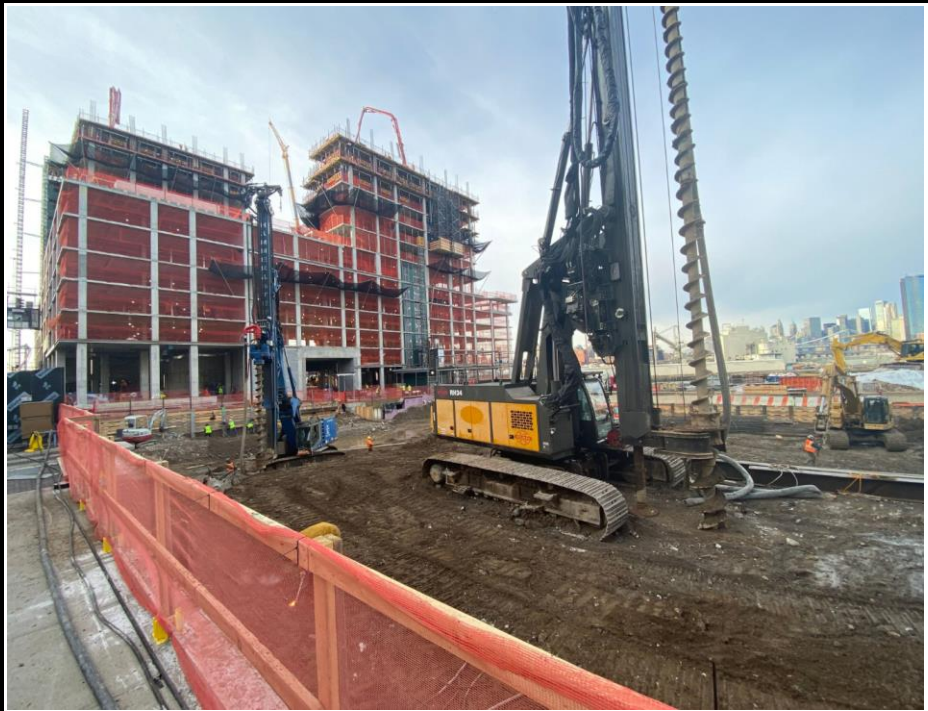
Photo 3: View of soil excavation and pile installation.
