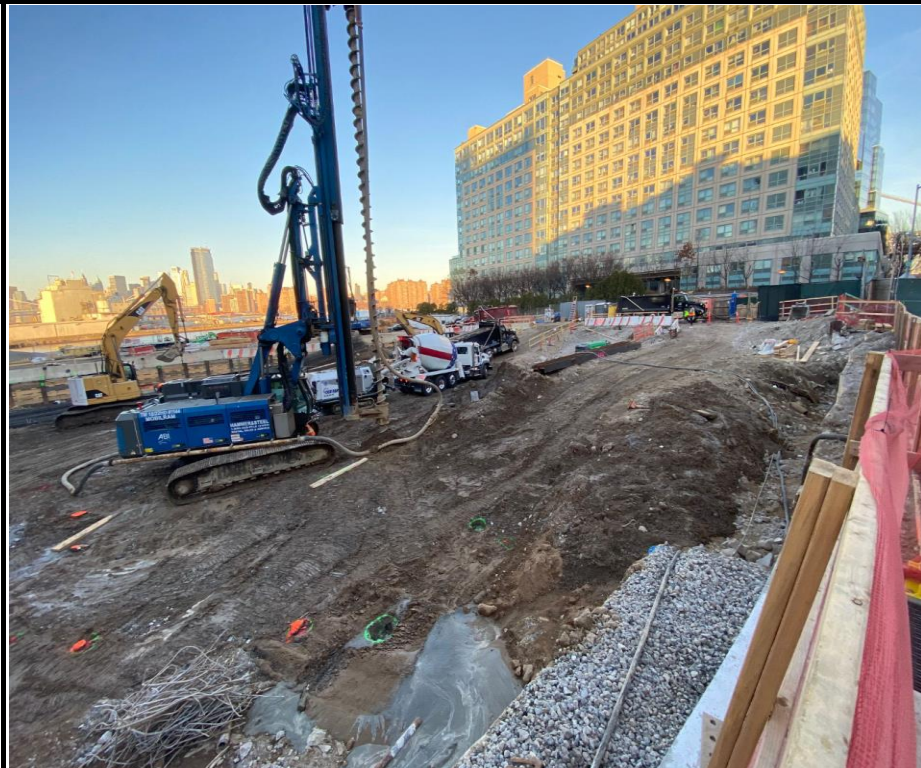
Photo 4: View of drilling for pile installation.
