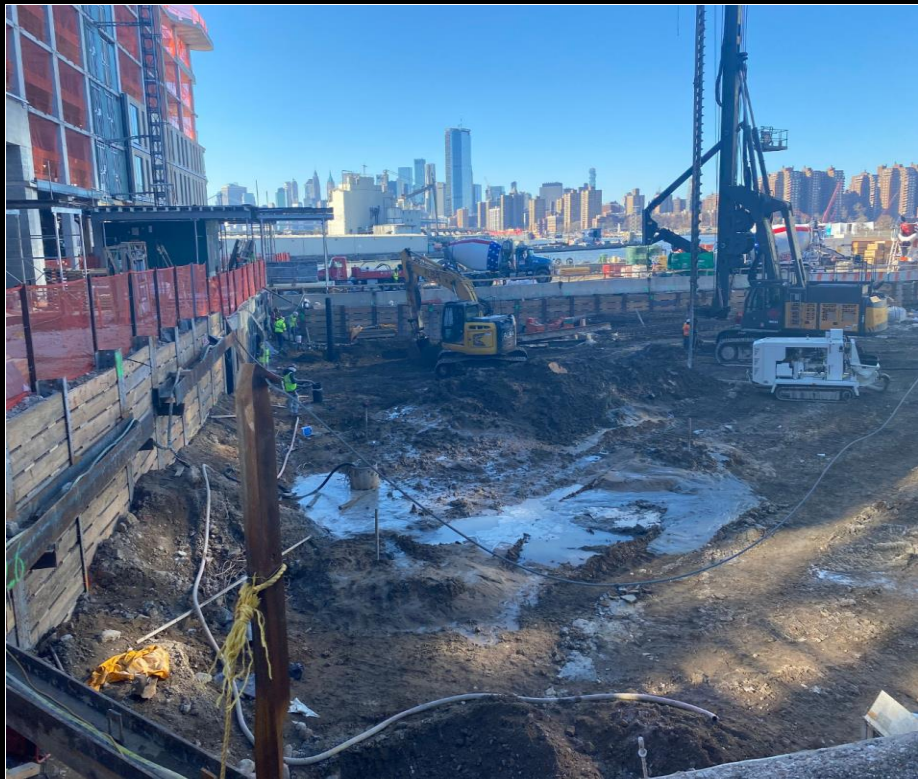
Photo 2: View of excavation and drilling for pile installation and SOE installation.
