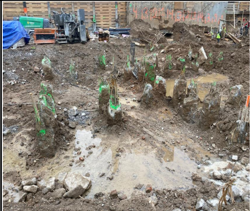
Photo 4: View of exposed piles.
