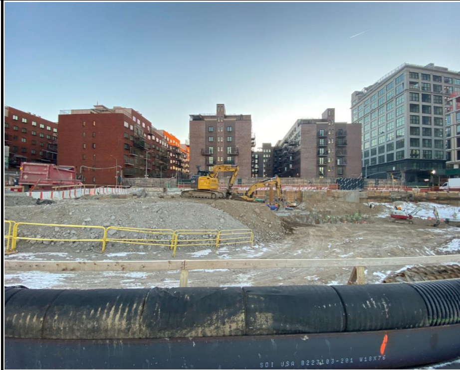
Photo 3: View of Site conditions facing east.
