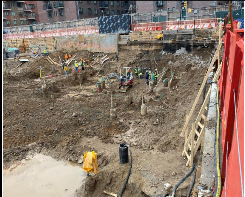
Photo 3: View of Site conditions facing east.
