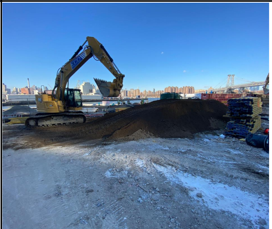
Photo 4: View of soil imported for backfill in the marine area.
