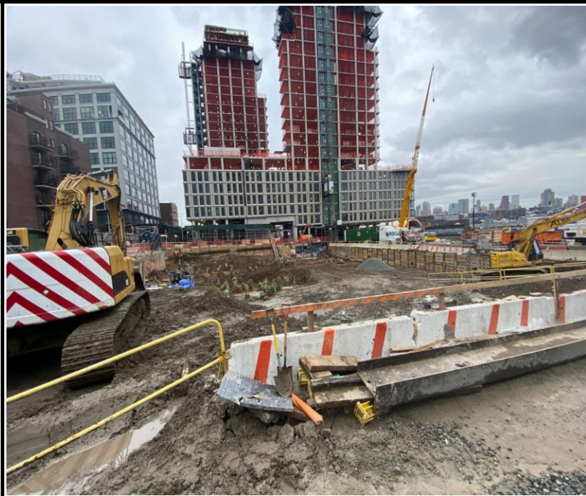
Photo 4: View of Site conditions facing south.
