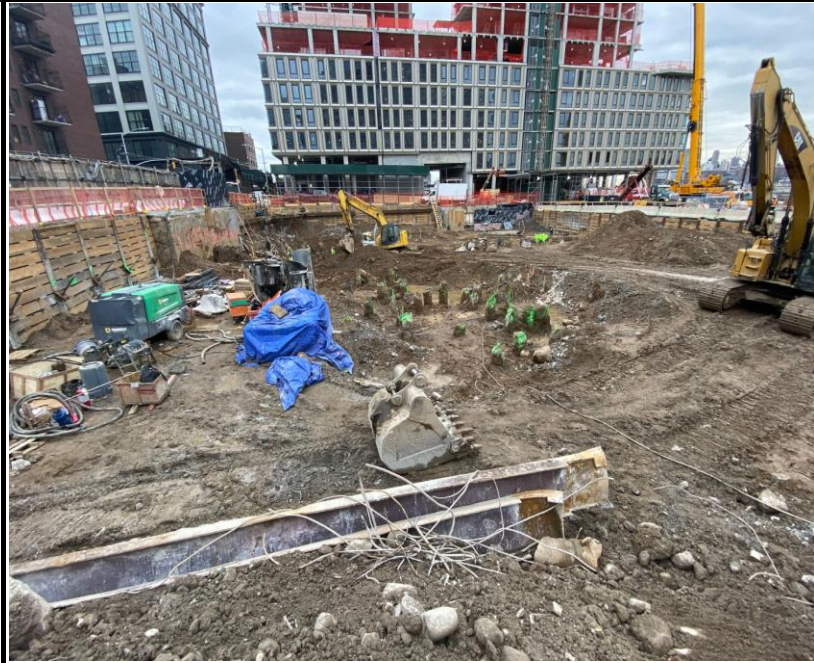
Photo 3: View of Site conditions facing south.
