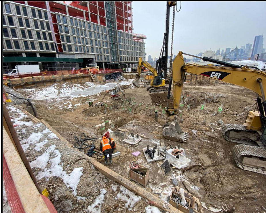
Photo 3: View of soil excavation facing southeast.
