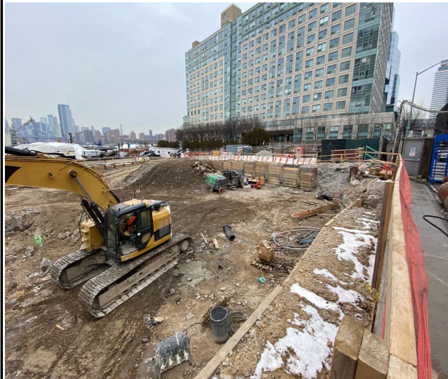
Photo 4: View of Site conditions and activities facing northeast.
