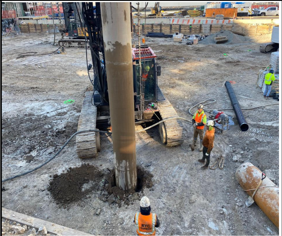
Photo 2: View of excavation and drilling for pile installation and SOE installation.
