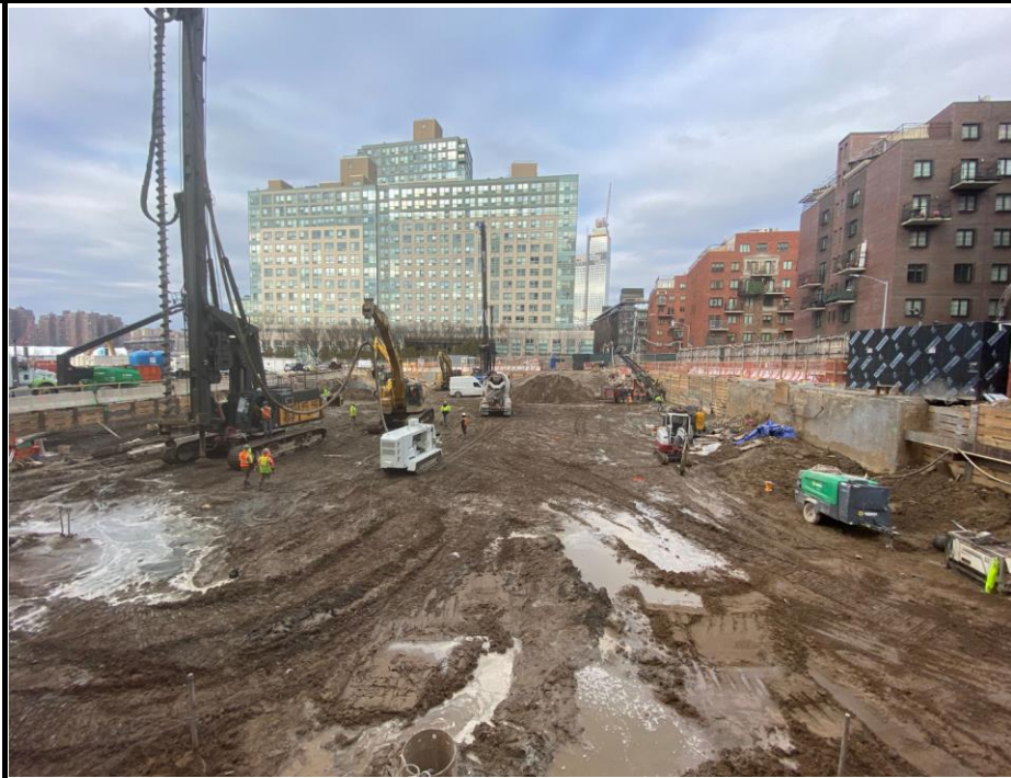
Photo 3: View of Site conditions facing north.
