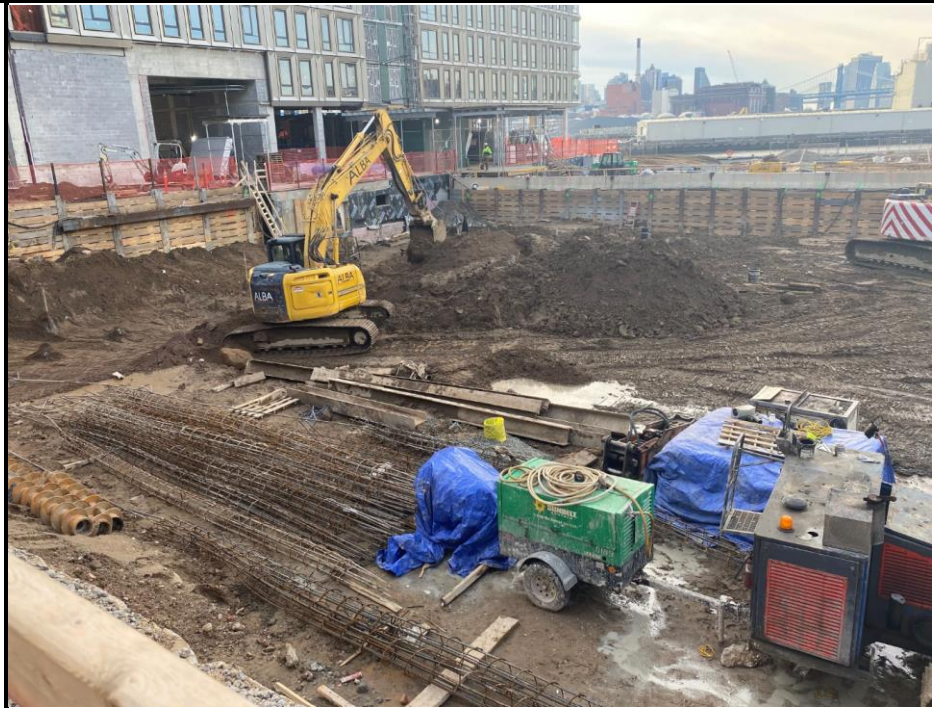
Photo 3: View of soil excavation facing southwest.
