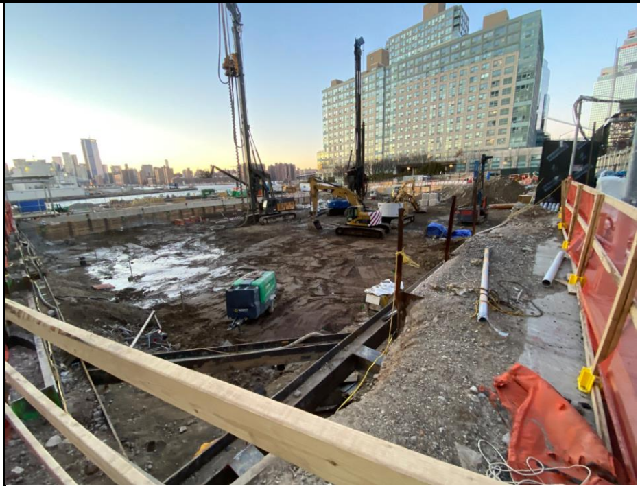
Photo 3: View of Site conditions facing north.
