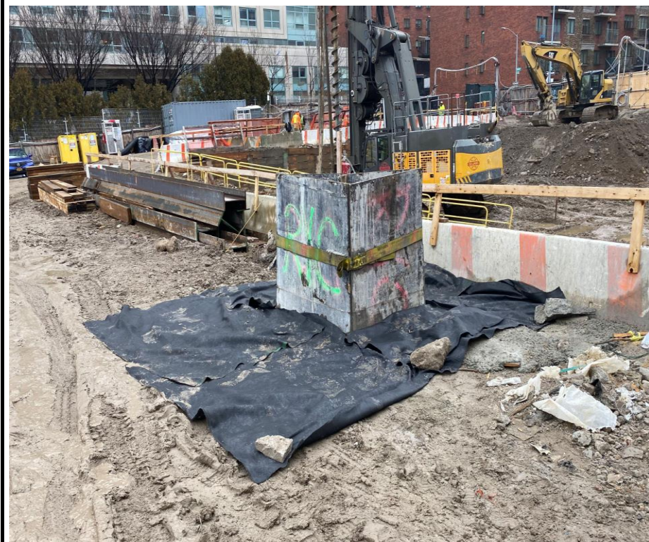
Photo 4: View of forming of a whaler in preparation for development of foundation elements.
