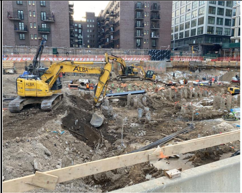
Photo 1: View of soil excavation and Site conditions facing east.
