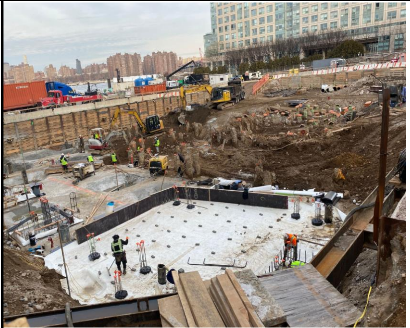
Photo 1: View of Site conditions facing northwest.
