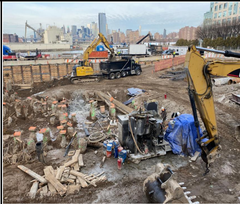
Photo 2: View of Site conditions during truck loading for off-site soil disposal, facing west.
