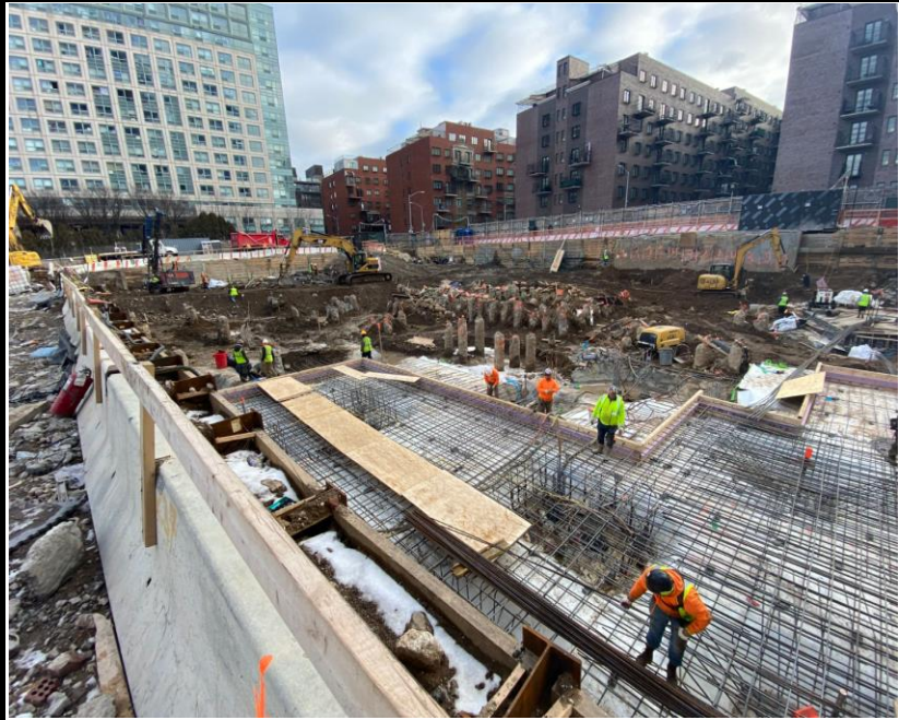
Photo 1: View of Site conditions and rebar installation facing northwest.
