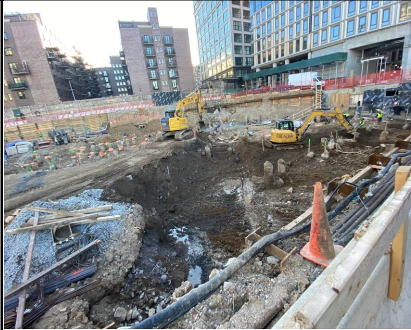
Photo 3: View of excavation and Site conditions facing southeast.
