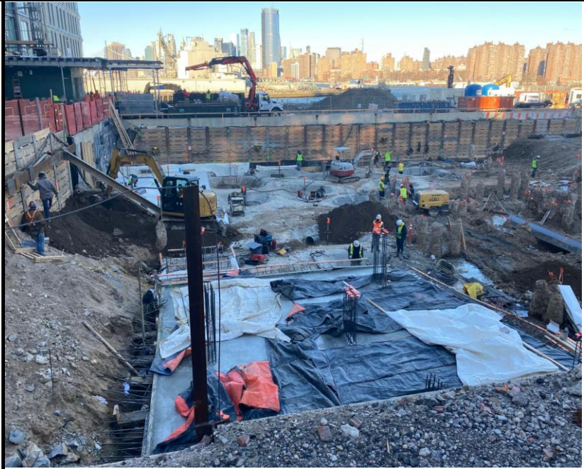
Photo 1: View of Site conditions facing west.
