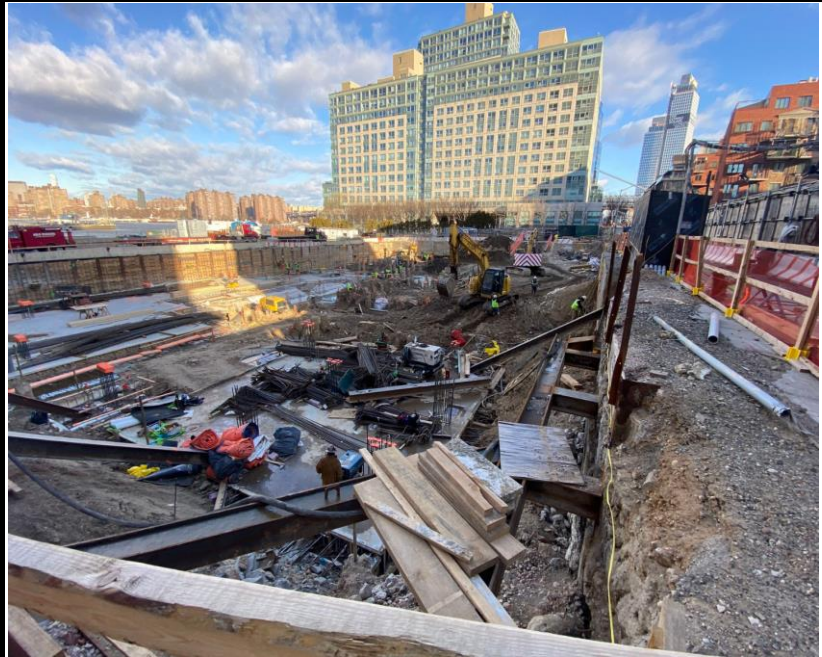
Photo 1: View of Site conditions facing northeast.
