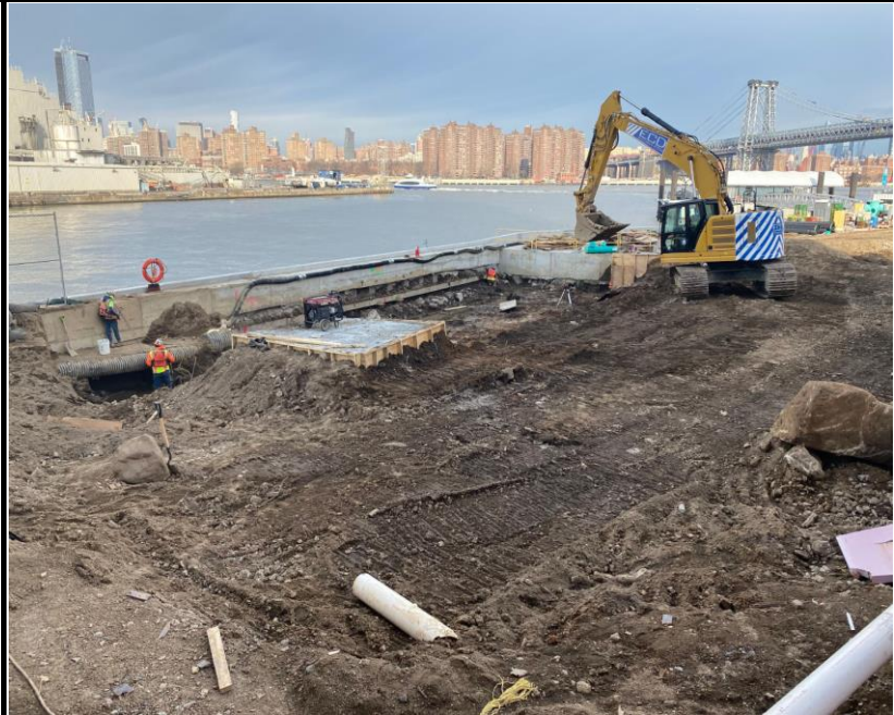
Photo 3: View of the remedial excavation facing west.
