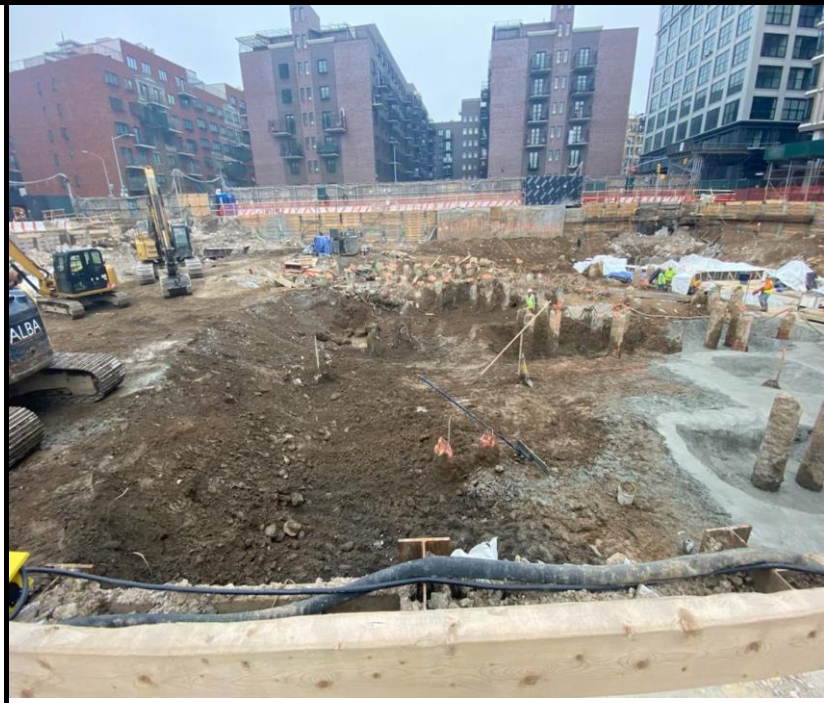
Photo 4: View of soil excavation and waterproofing installation.
