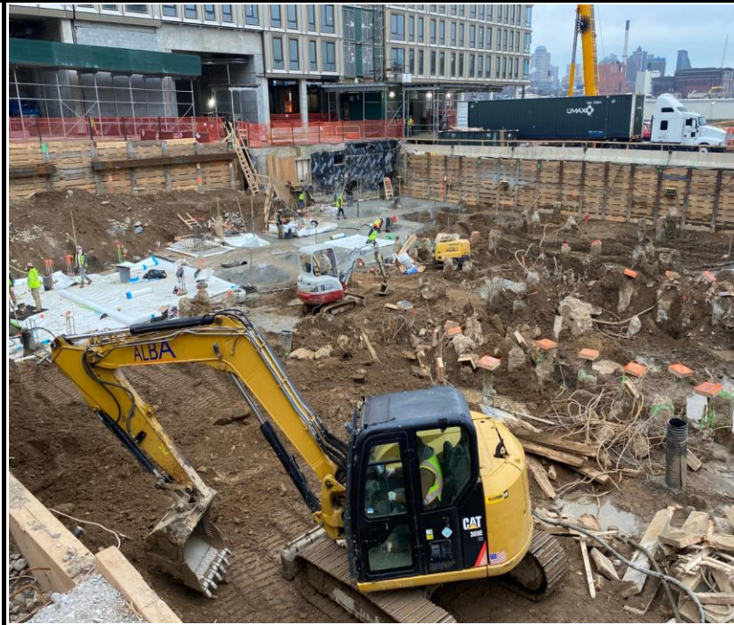
Photo 4: View of soil excavation and waterproofing installation.
