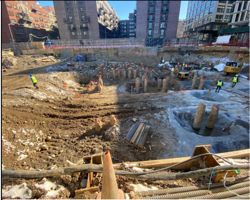
Photo 1: View of Site conditions facing east.
