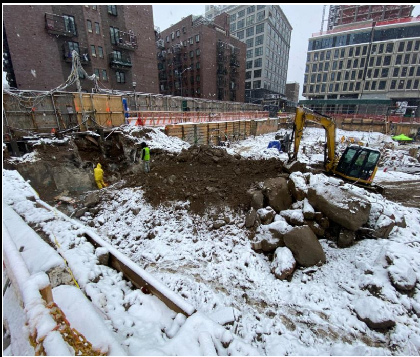
Photo 2: View of excavation in the NE corner of the excavation, facing east.
