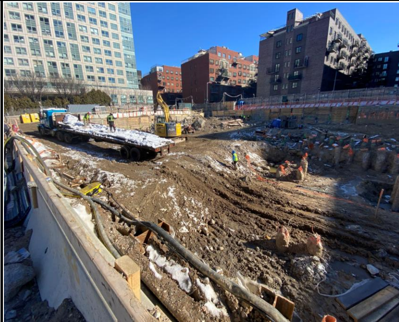
Photo 3: View of Site conditions facing northeast.
