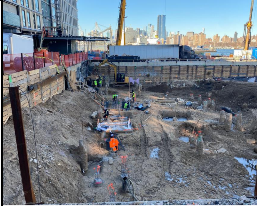
Photo 3: View of foundation footing framing and waterproofing installation.
