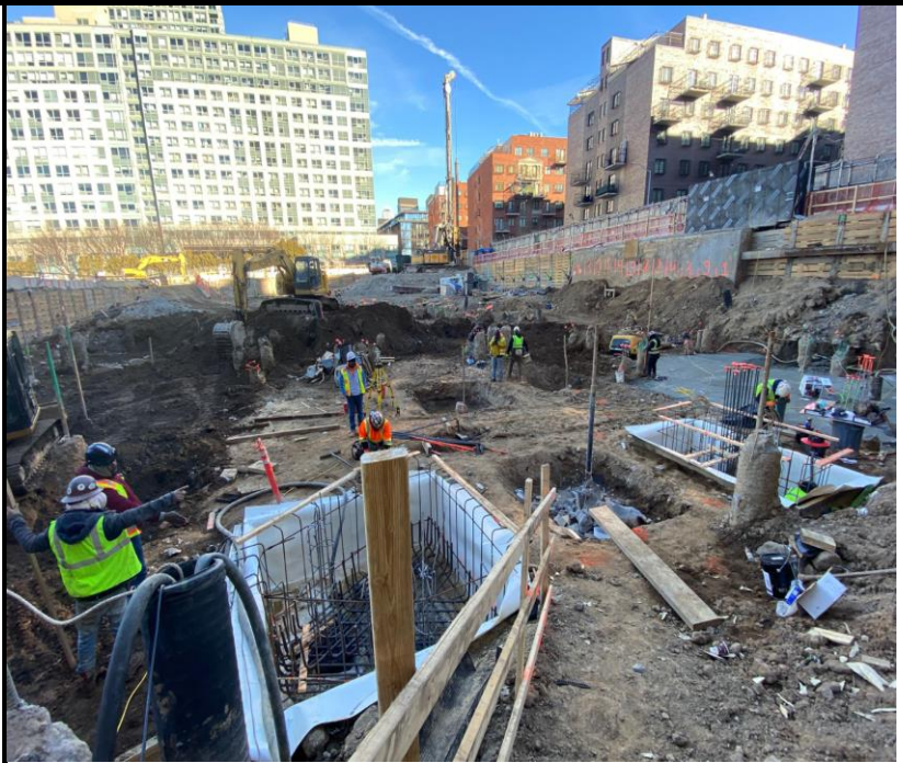
Photo 2: View of Site conditions, waterproofing and rebar installation for foundation development facing northeast.
