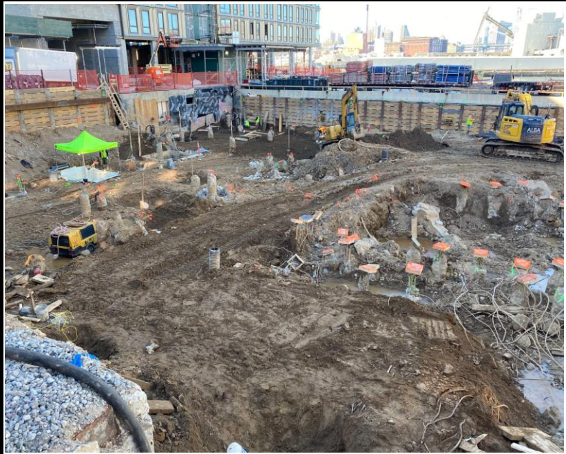
Photo 1: View of Site conditions and soil excavation facing southwest.
