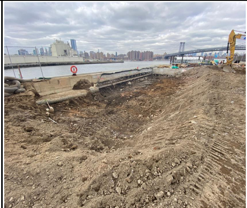
Photo 4: View of Site conditions in the marine waterfront remedial excavation.
