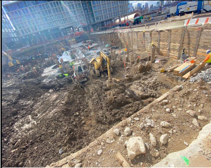
Photo 3: View of Site conditions facing south.
