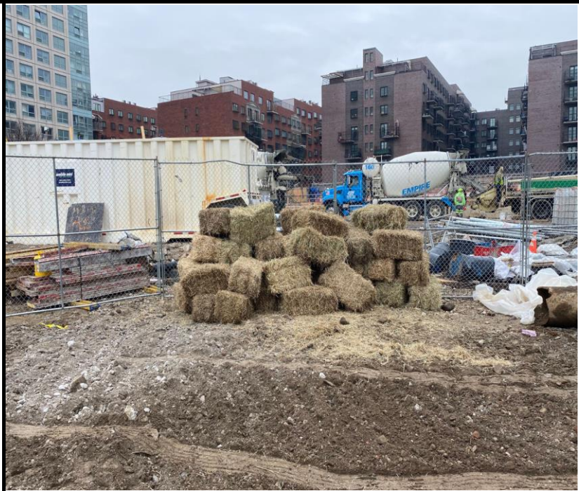
Photo 2: View of hay bales for use to stabilize the remedial excavation soil stockpile.
