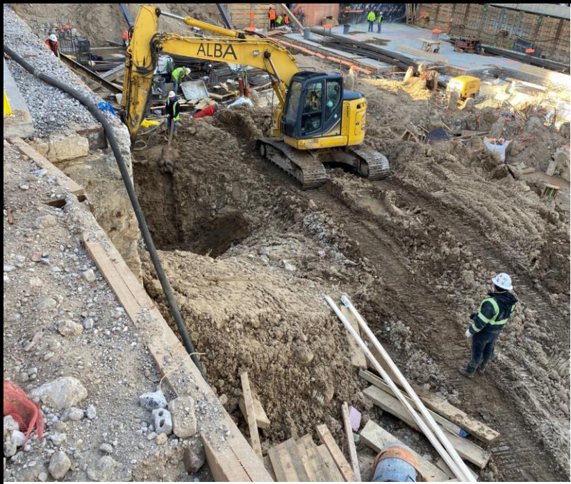
Photo 2: View of soil excavation.
