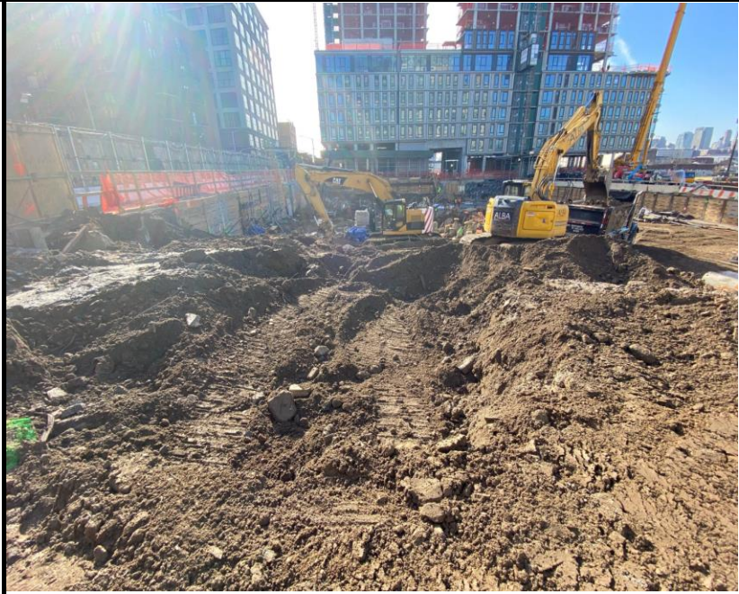
Photo 3: View of Site conditions facing south.
