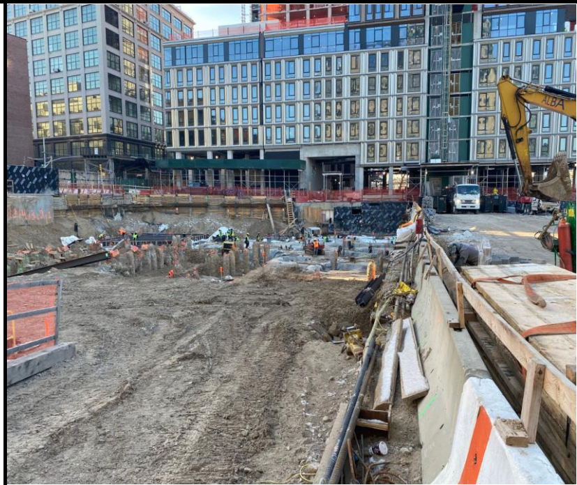
Photo 2: View of Site conditions and waterproofing installation facing east.
