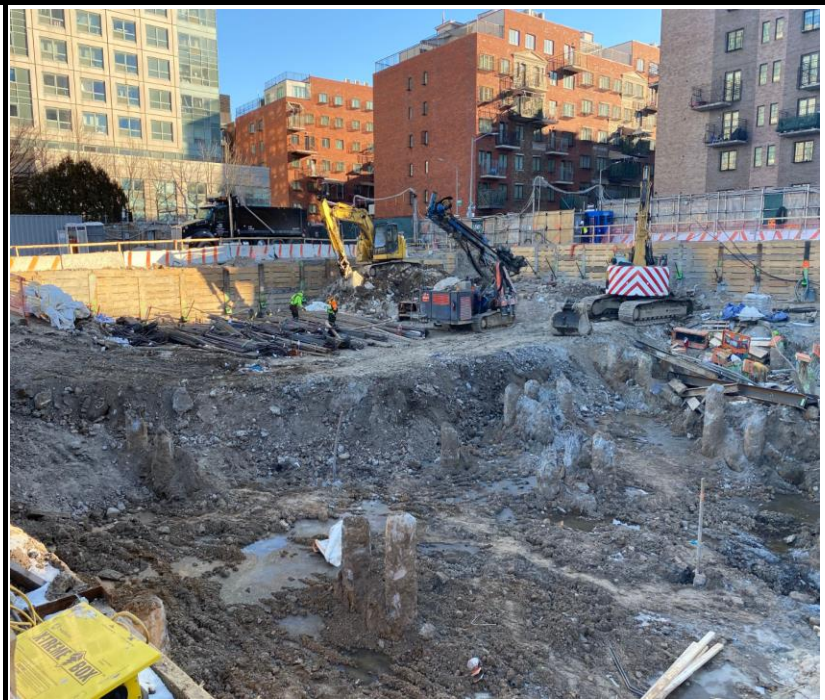
Photo 2: View of excavation and pile installation facing northeast.
