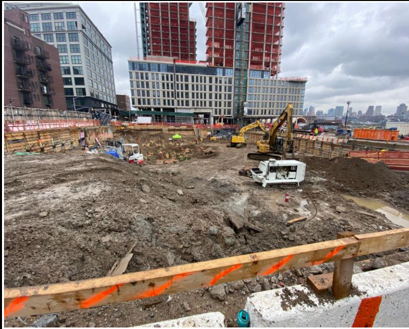
Photo 3: View of Site conditions facing south.
