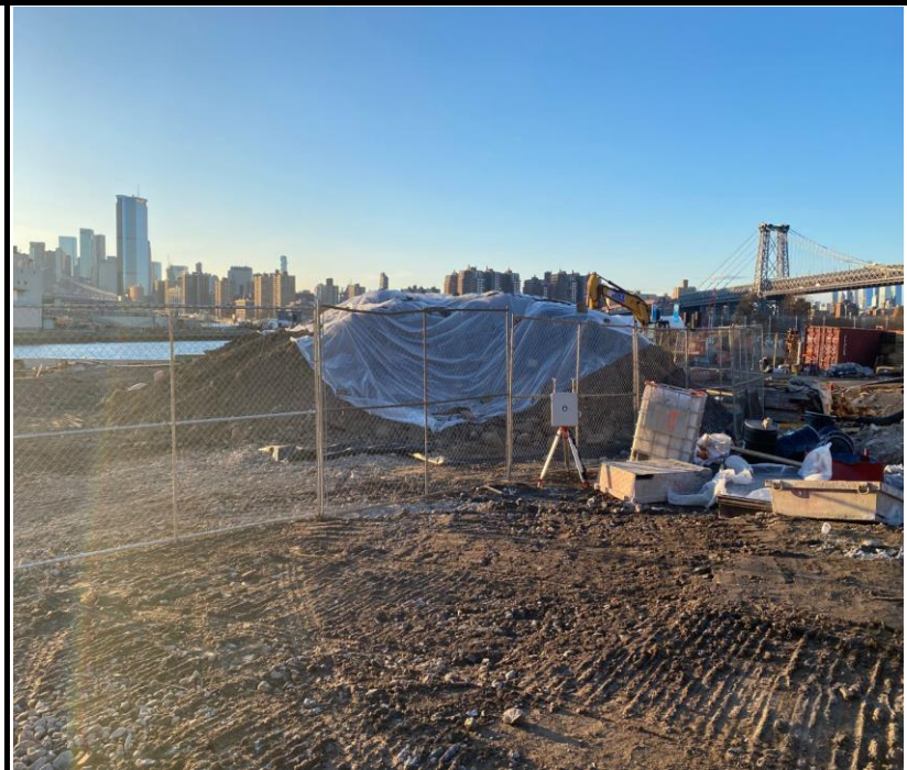
Photo 4: View of stockpiled material from the waterfront remedial excavation facing northwest.
