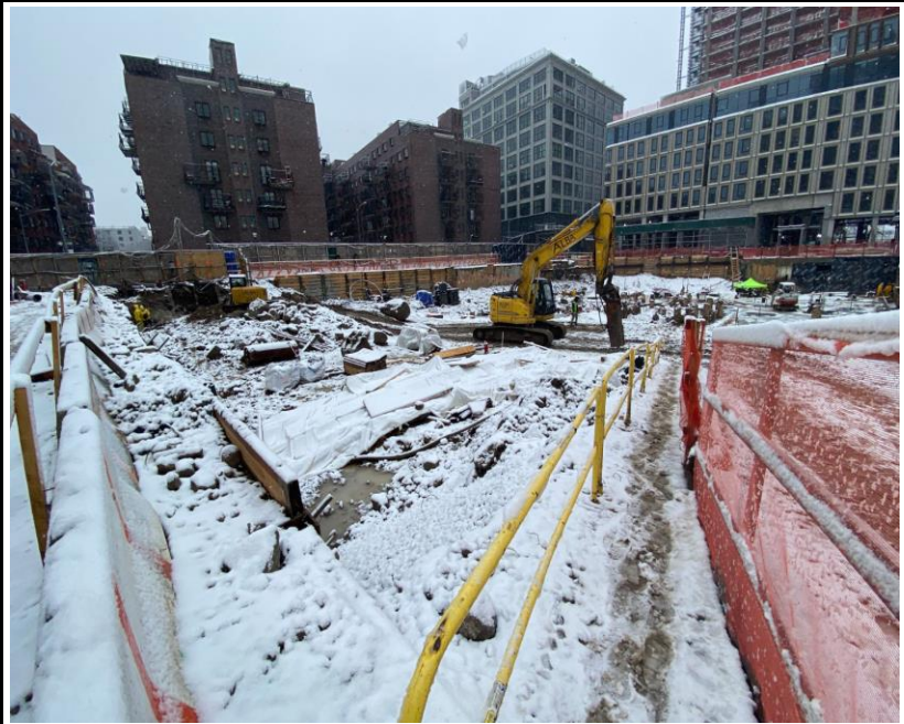
Photo 1: View of Site conditions facing northeast.
