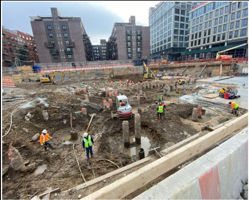
Photo 1: View of Site conditions facing east.
