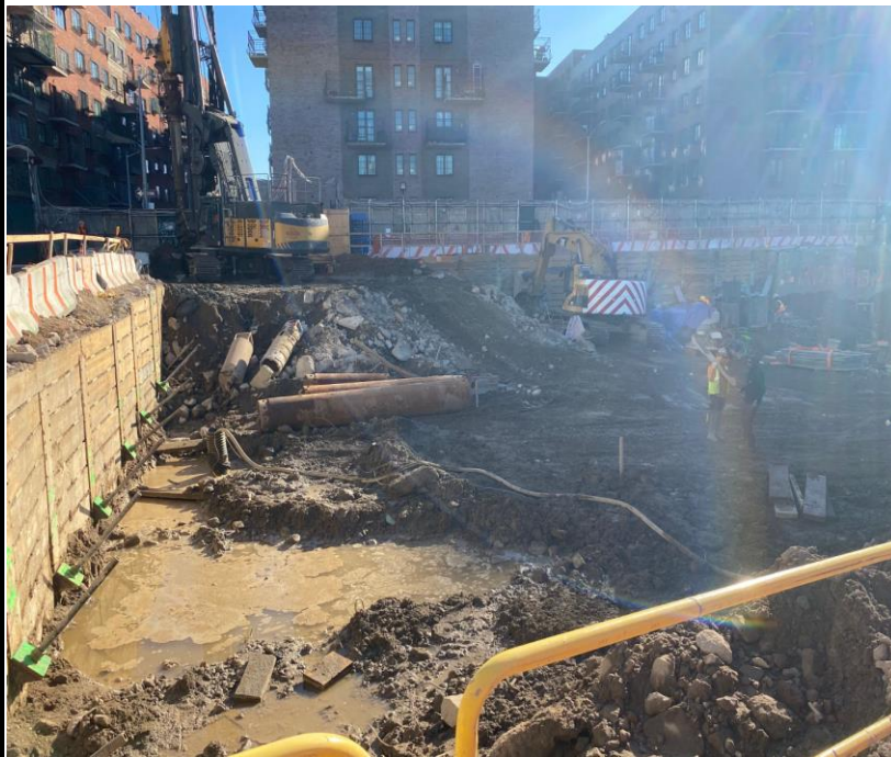
Photo 4: View of soil excavation and pile installation.
