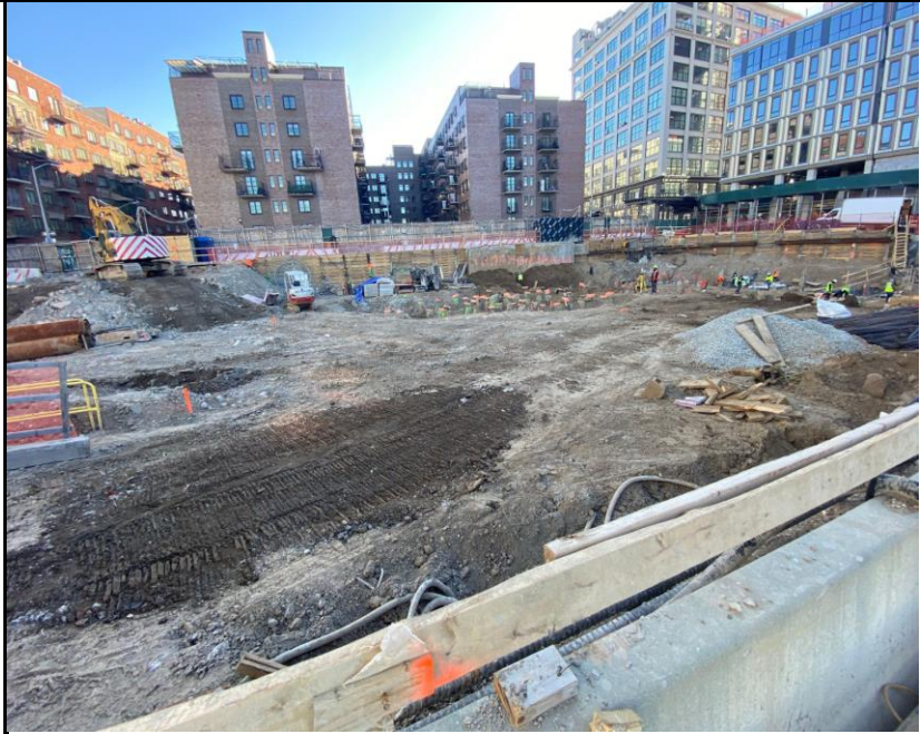
Photo 1: View of Site conditions and soil excavation facing east.
