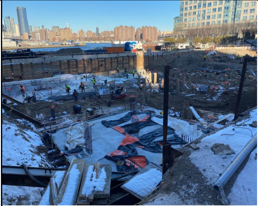
Photo 1: View of Site conditions facing northwest.
