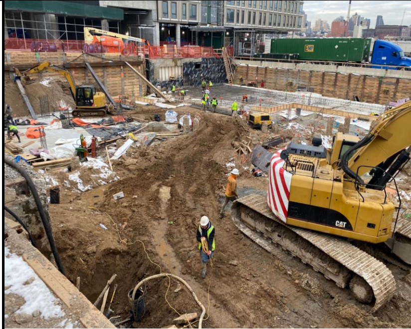
Photo 3: View of Site conditions and rebar instllation for foundation development facing southwest.
