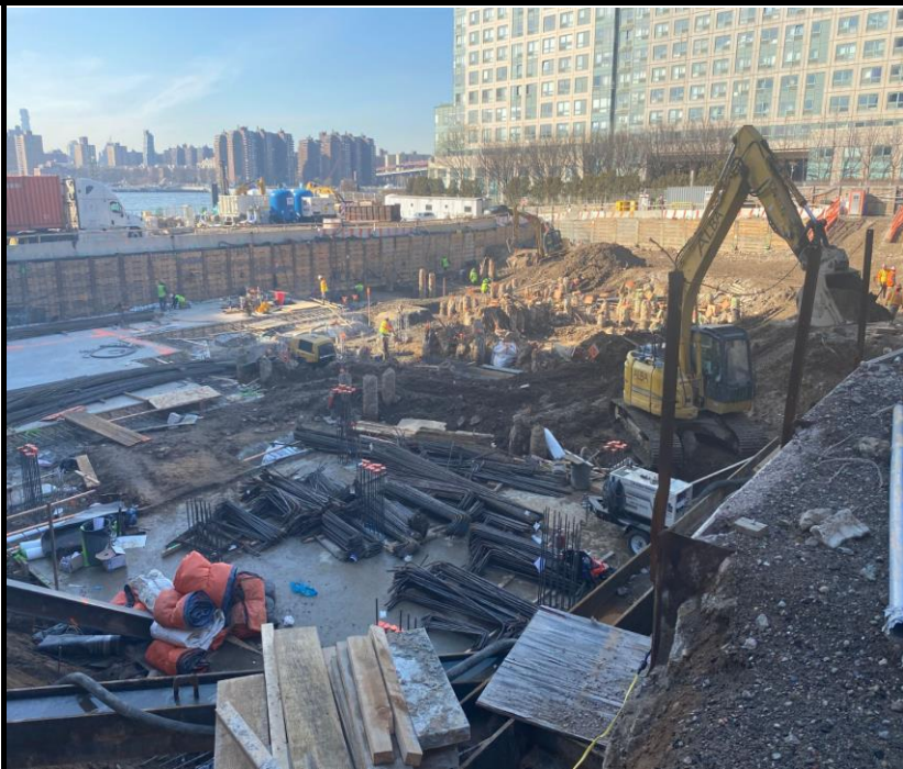
Photo 4: View of Site conditions facing northwest.
