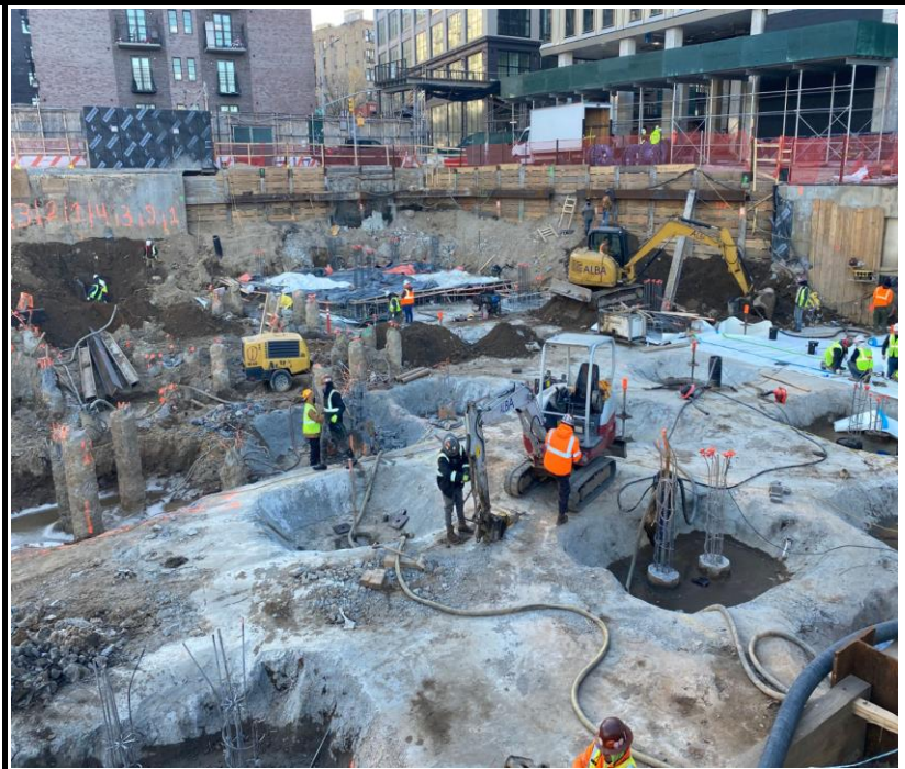
Photo 2: View of Site conditions facing east.
