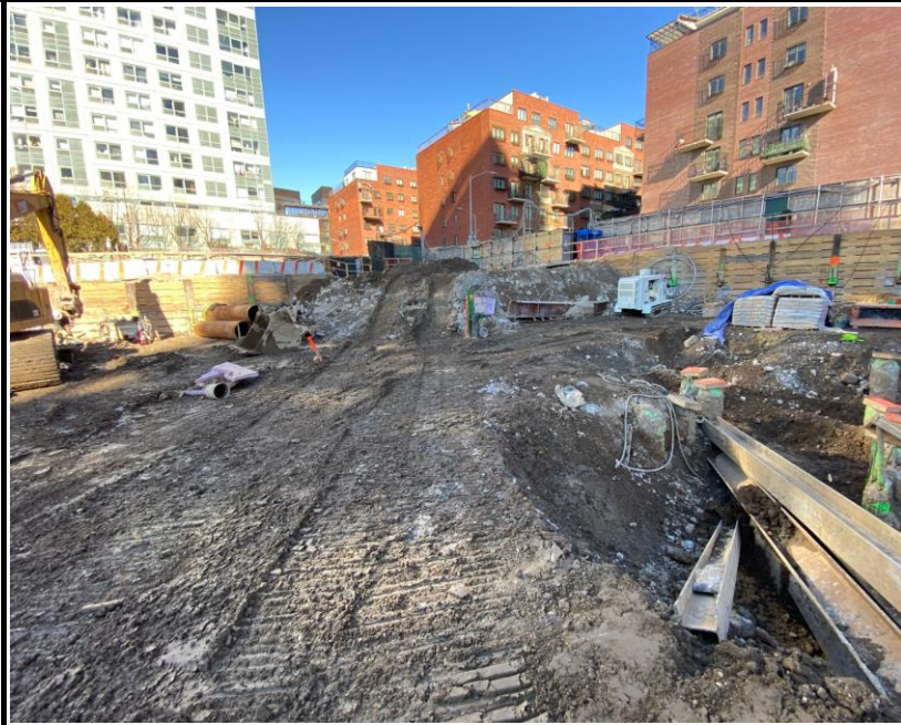
Photo 3: View of Site conditions facing northeast.
