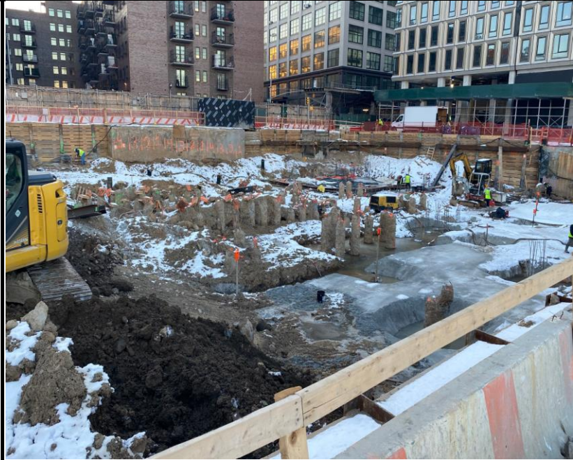
Photo 3: View of Site conditions and exposed piles facing southeast.
