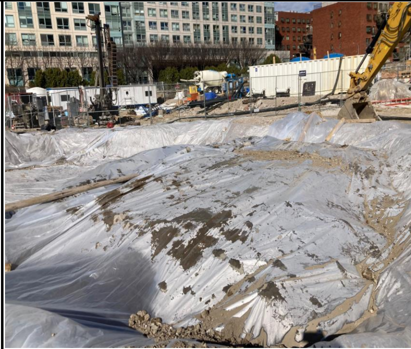
Photo 4: View of the waterfront remedial excavation.
