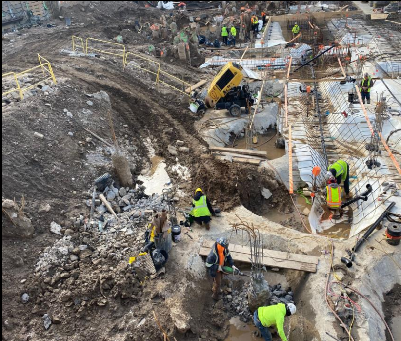
Photo 2: View of Site conditions, framing and rebar installation.
