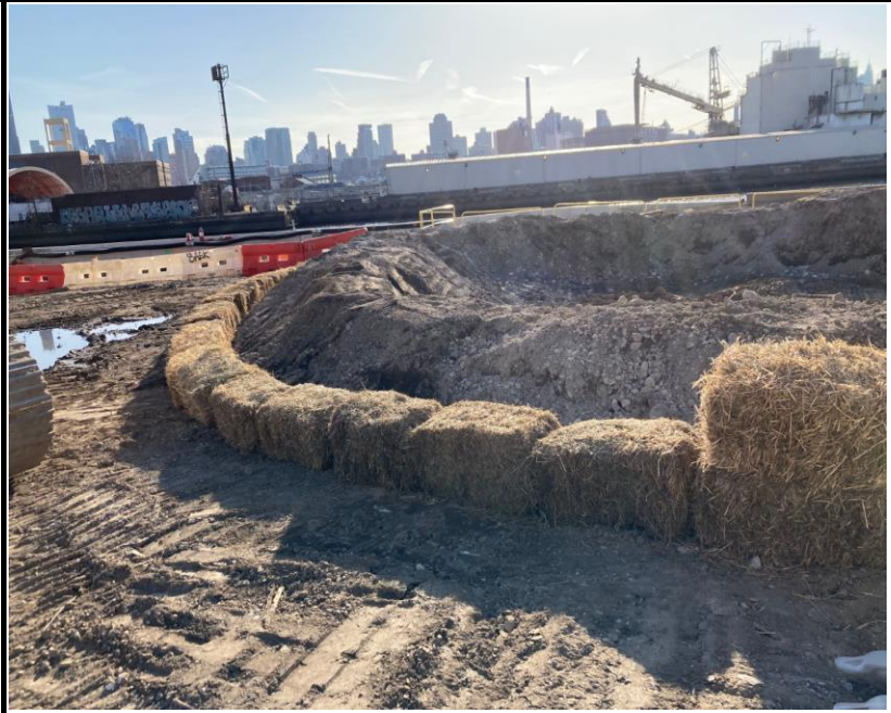
Photo 3: View of haybales surrounding the remedial excavation soil stockpile.
