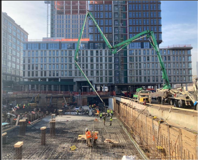
Photo 3: View of concrete pouring for building foundation development, facing south.
