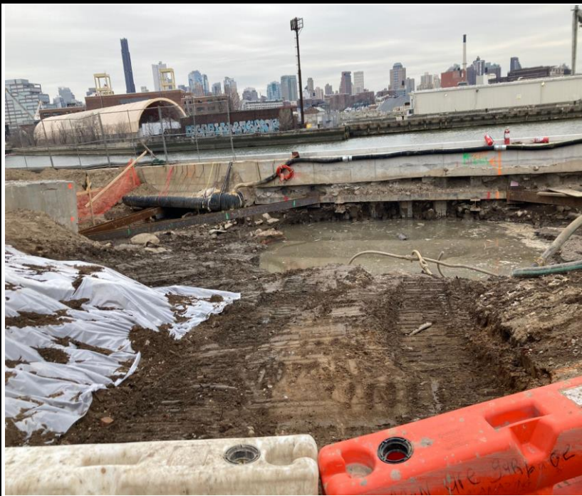
Photo 4: View of the remedial excavation facing west.
