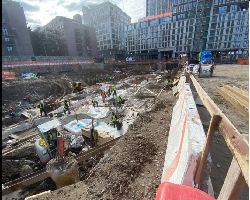
Photo 1: View of Site conditions and activities facing southeast.
