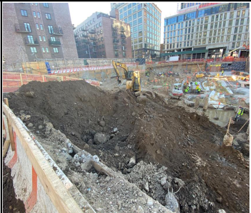
Photo 2: View of soil excavation.
