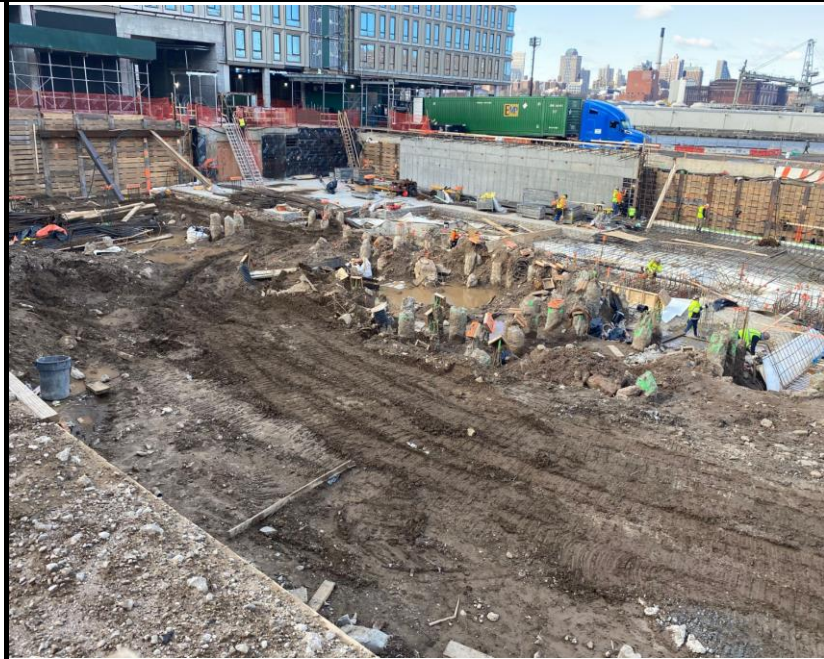
Photo 3: View of Site conditions and waterproofing and rebar installation facing southwest.
