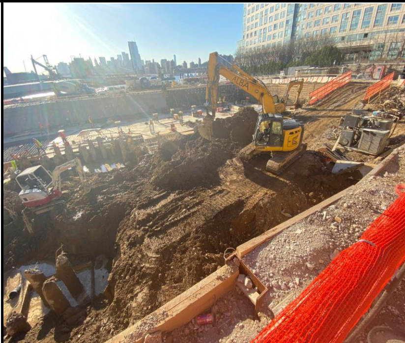
Photo 2: View of soil excavation.
