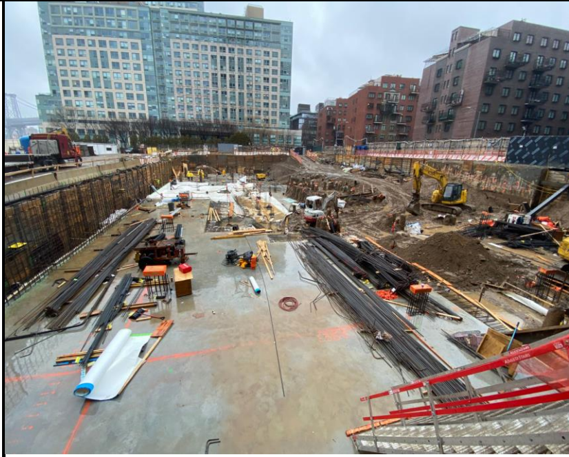
Photo 1: View of Site conditions facing south.
