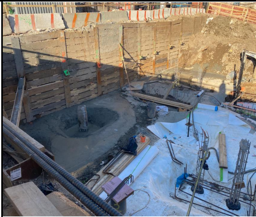
Photo 4: View of concrete pouring and waterproofing installation.
