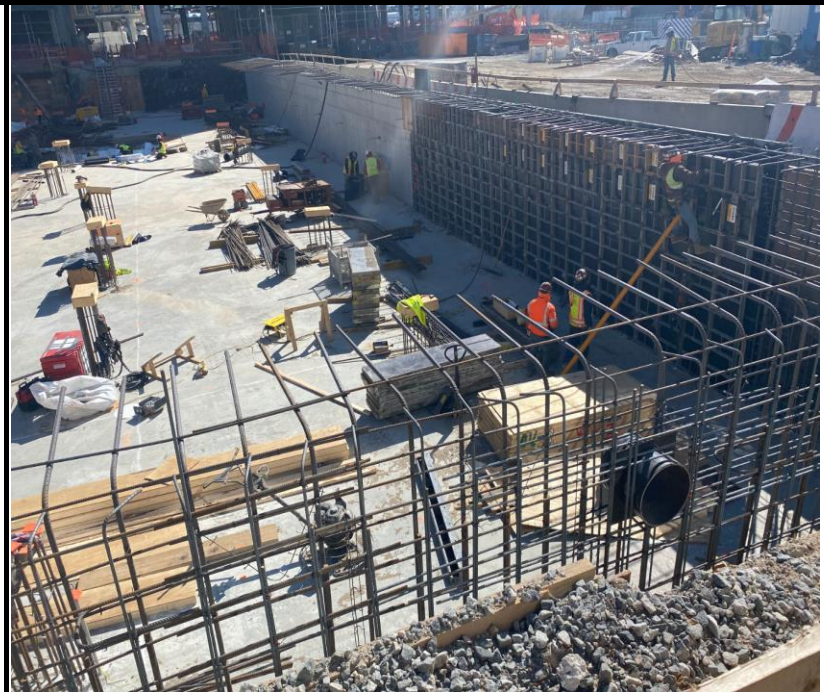
Photo 4: View of rebar installation and foundation framing.
