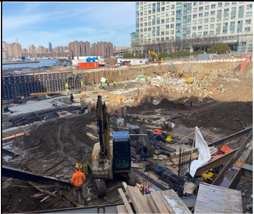
Photo 2: Site conditions, framing and rebar installation facing west.
