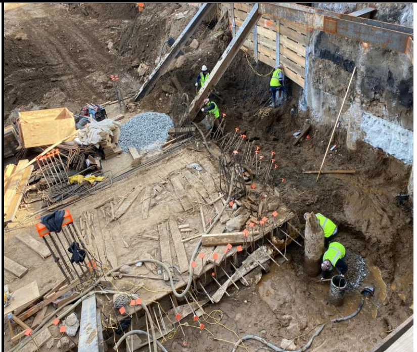
Photo 2: View of soil excavation and lagging installation for SOE.
