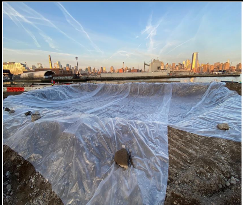
Photo 4: View of the remedial excavation.
