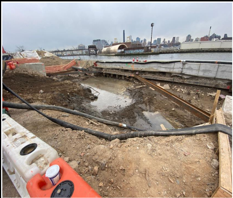
Photo 4: View of the waterfront remedial excavation.
