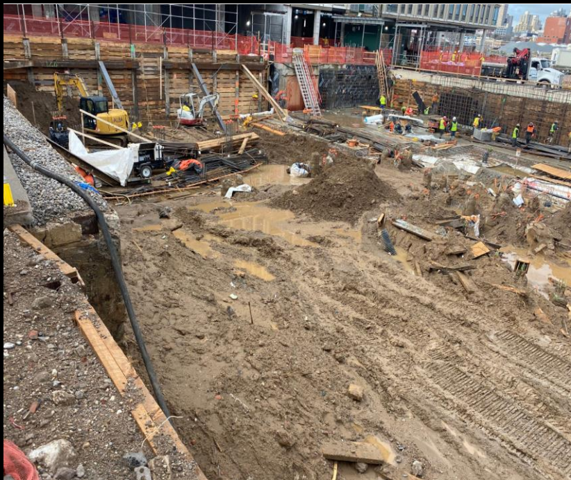
Photo 2: Site conditions and SOE installation facing southwest.
