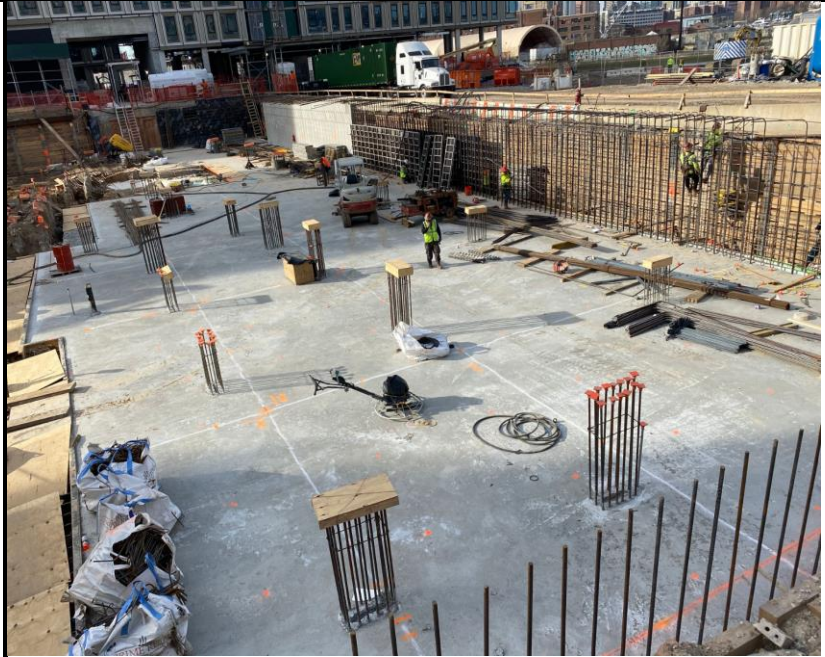
Photo 1: View of Site conditions and activities facing south.
