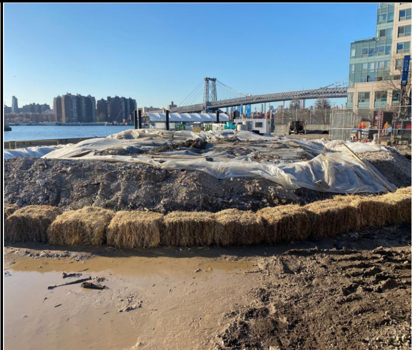
Photo 4: View of the remedial excavation stockpile.
