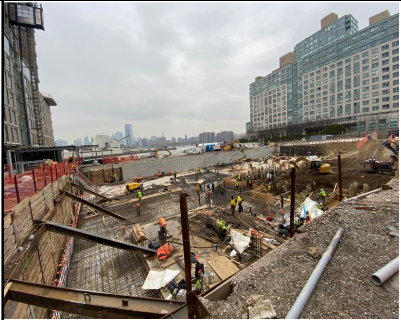
Photo 1: View of Site conditions and activities facing northwest..
