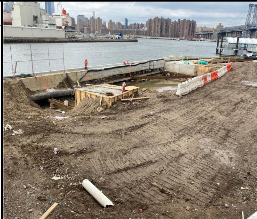
Photo 4: View of continued SOE development for the waterfront remedial excavation.
