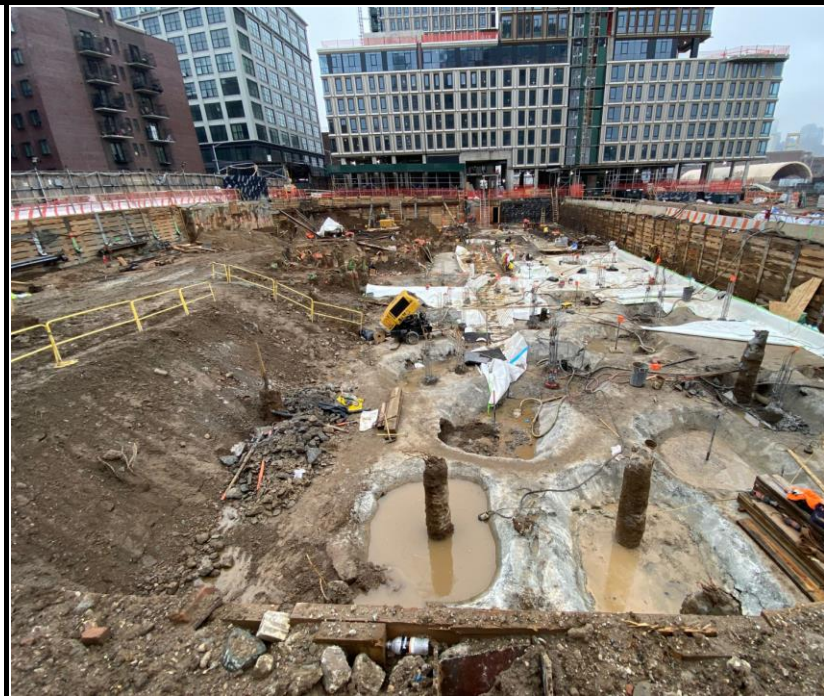
Photo 4: View of Site conditions facing south.
