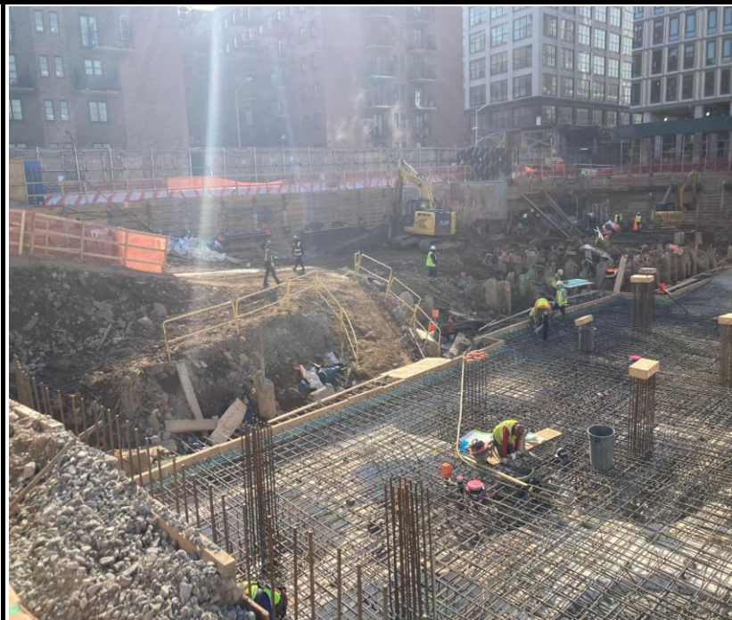
Photo 4: View of soil excavation and SOE installation facing east.
