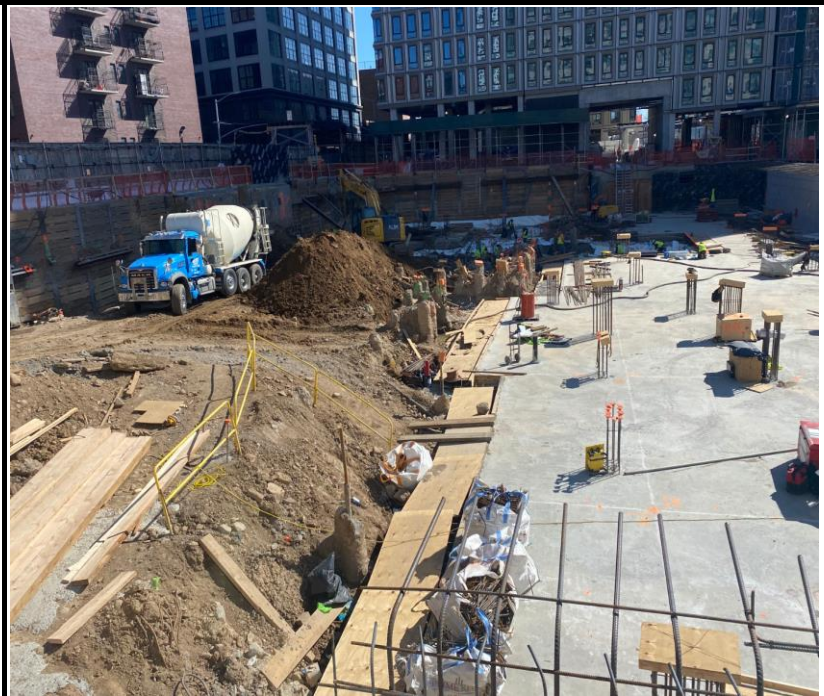
Photo 2: View of Site conditions and activities facing south.
