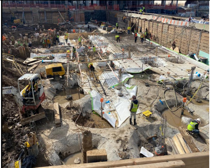
Photo 3: View of Site conditions and waterproofing and rebar installation facing south.
