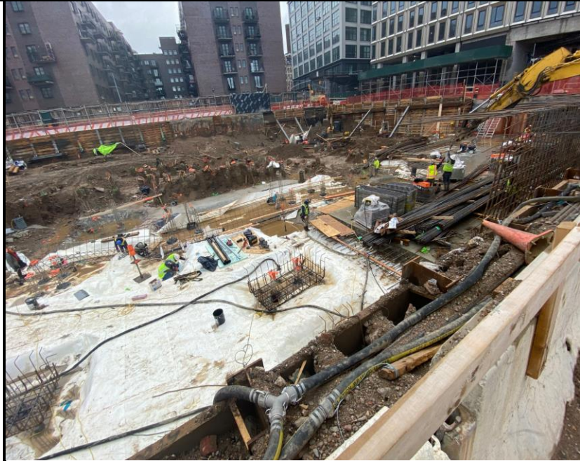
Photo 3: View of Site conditions and waterproofing and rebar installation facing southwest.
