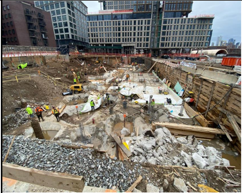
Photo 1: View of Site conditions and activities facing south.
