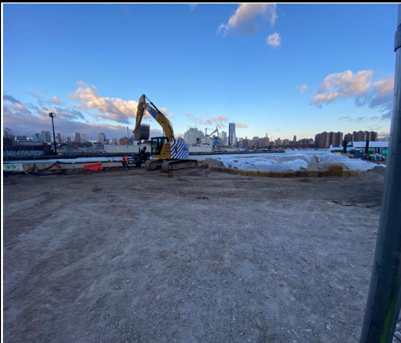
Photo 4: View of the waterfront remedial excavation.
