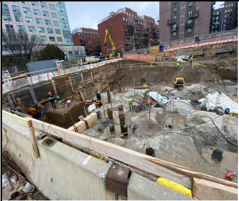
Photo 2: Site conditions and SOE installation and welding facing east.
