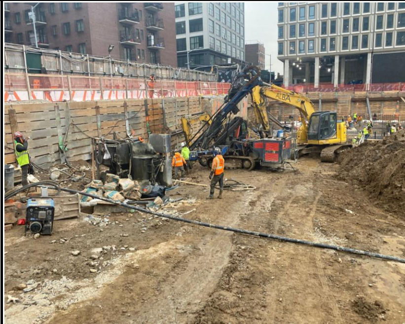
Photo 3: View of Site activities and SOE installation.
