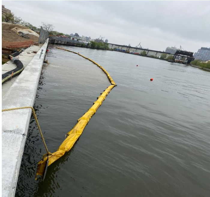
Photo 3: View of the dewatering discharge prior to being shutdown.
