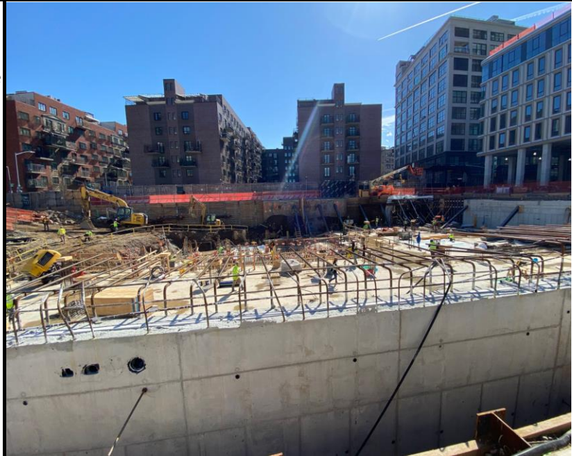
Photo 3: View of building foundation development and Site activities facing east.
