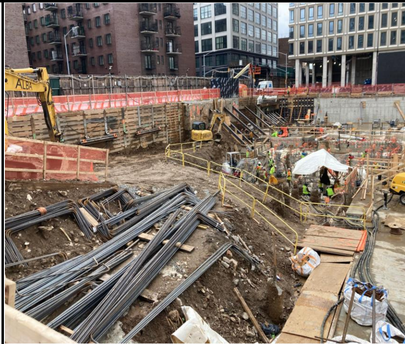
Photo 2: View of foundation development and Site conditions facing southeast.
