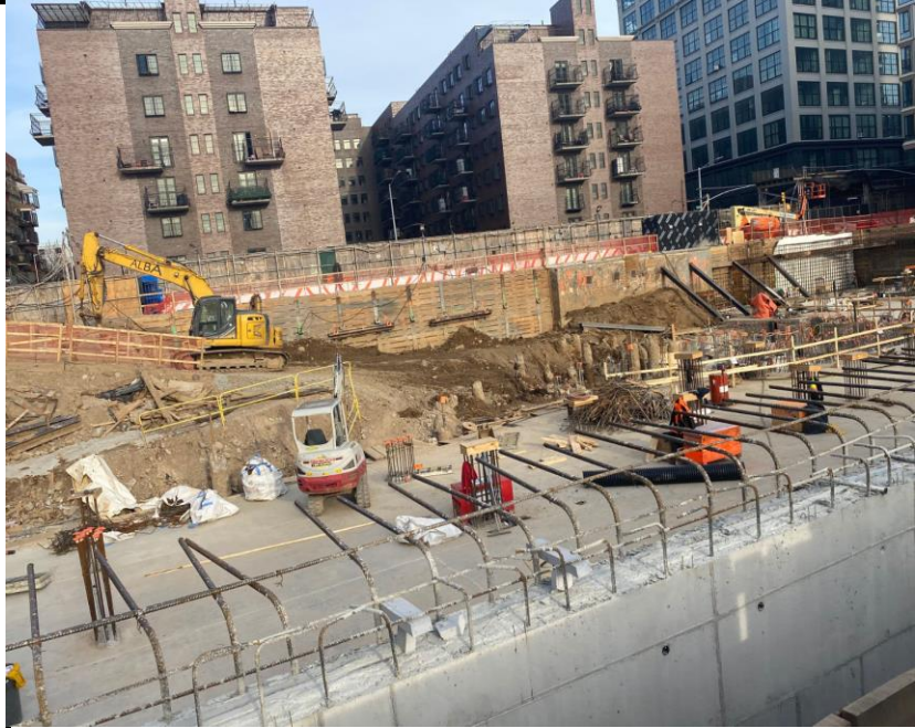
Photo 1: View of Site conditions and soil excavating facing east.
