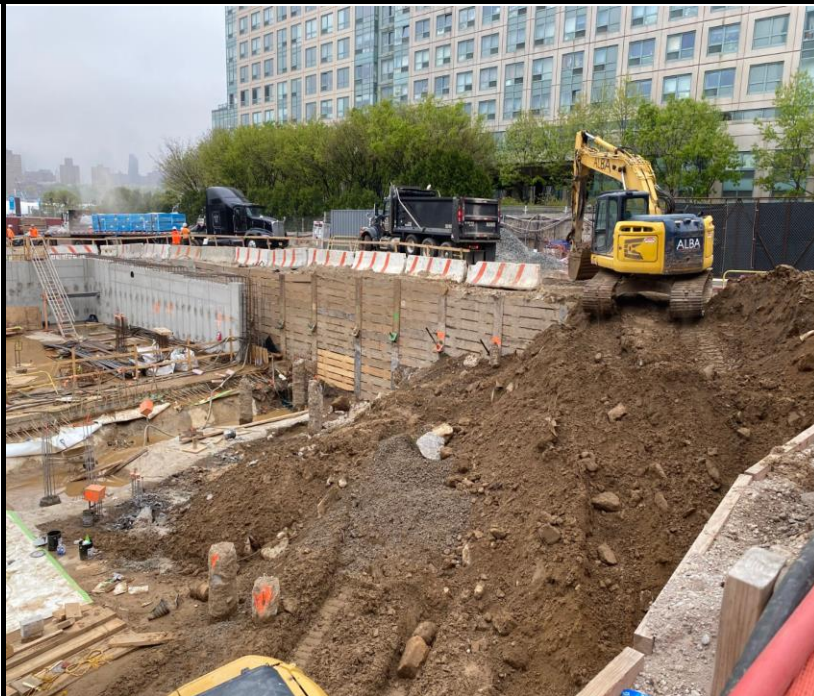
Photo 4: View of Site conditions and soil excavation facing northwest.
