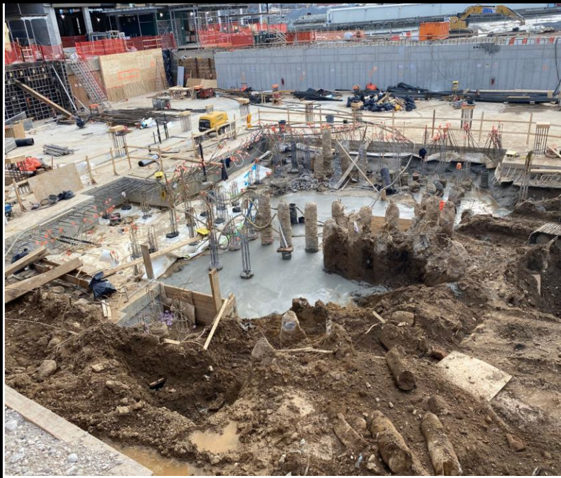
Photo 4: View of Site conditions facing west.
