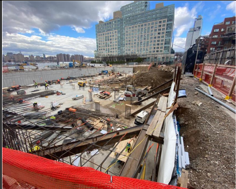
Photo 3: View of Site conditions, soil excavation and rebar installation facing northeast.
