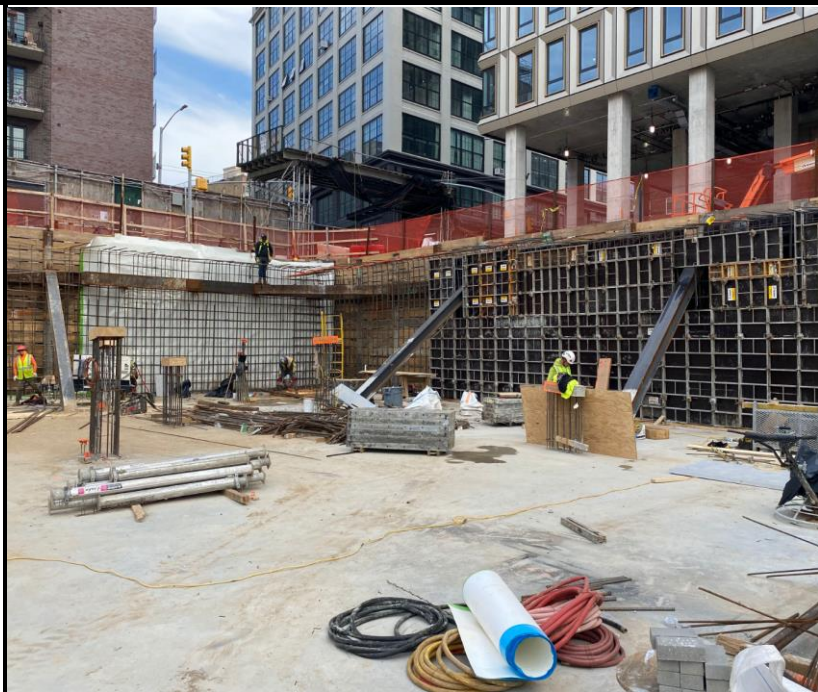
Photo 2: View of waterproofing installation.
