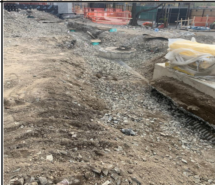
Photo 4: View of stormwater piping.
