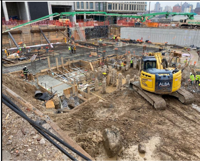
Photo 3: View of Site activities facing southwest.
