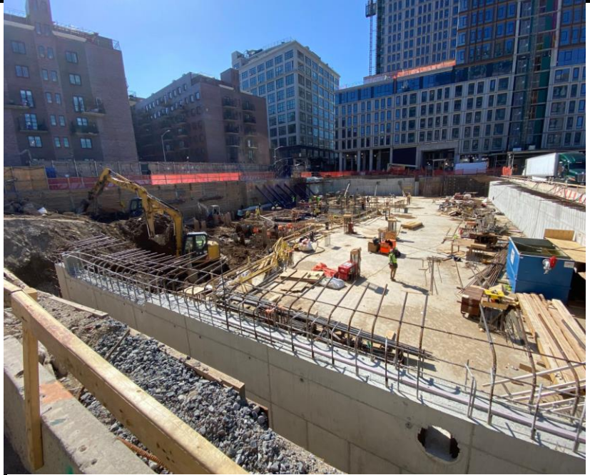
Photo 1: View of Site conditions and activities facing southwest.
