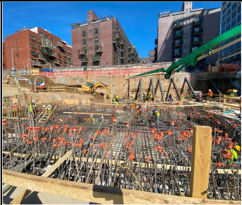
Photo 4: View of Site conditions, rebar installation and concrete pouring facing east.
