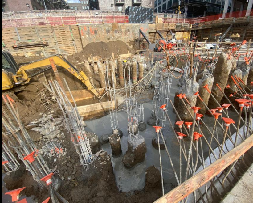
Photo 3: View of Site conditions, soil excavation and rebar installation facing east.
