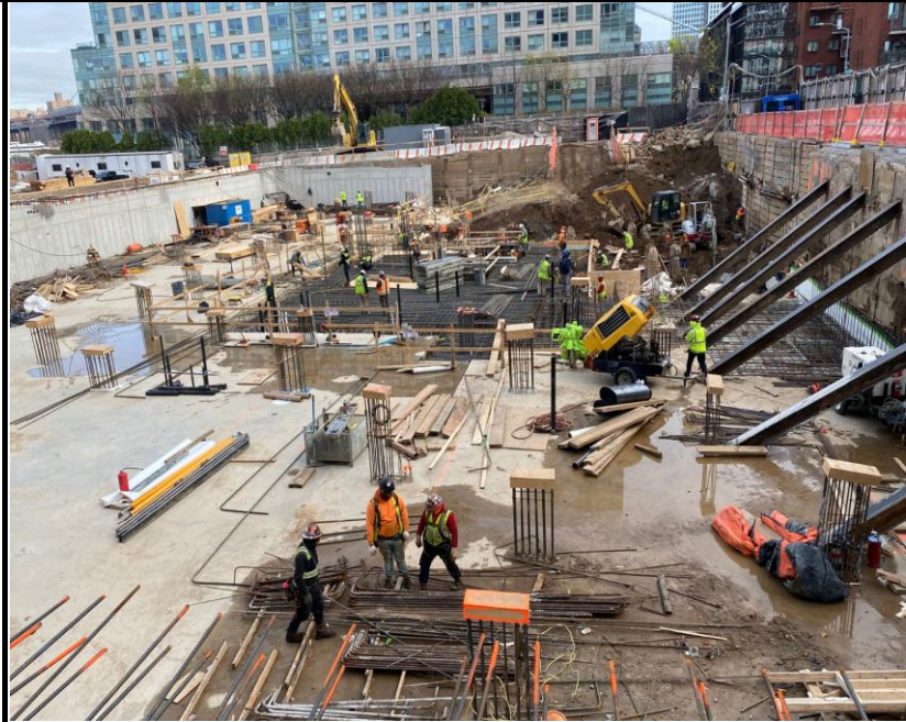
Photo 1: View of Site conditions and activities facing north.
