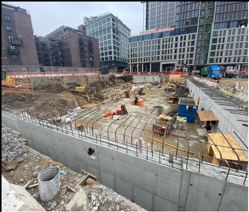
Photo 2: View of foundation development facing southeast.
