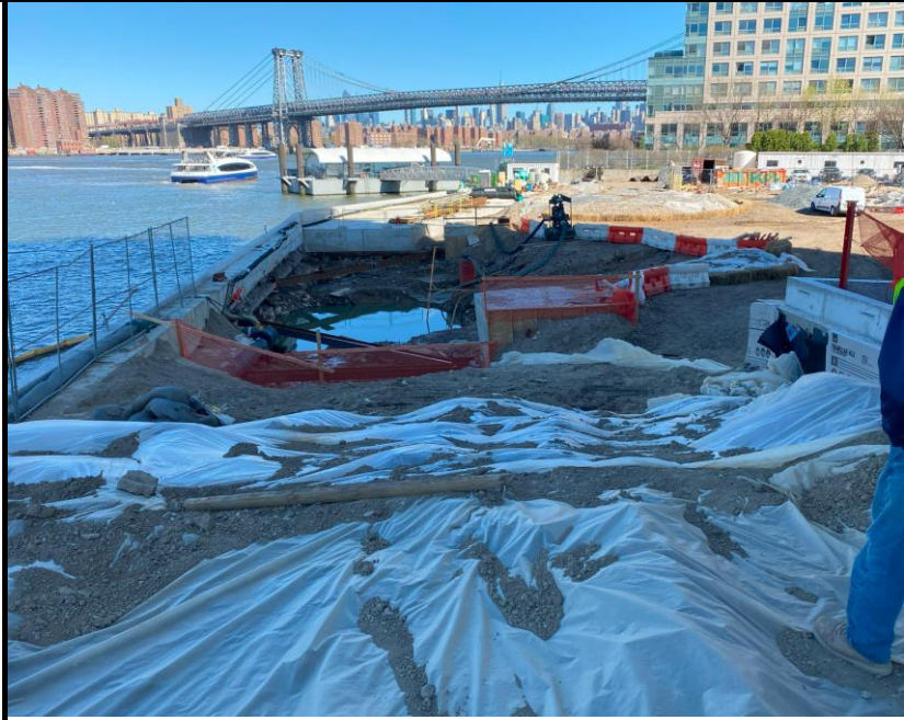
Photo 3: View of the remedial excavation facing north.
