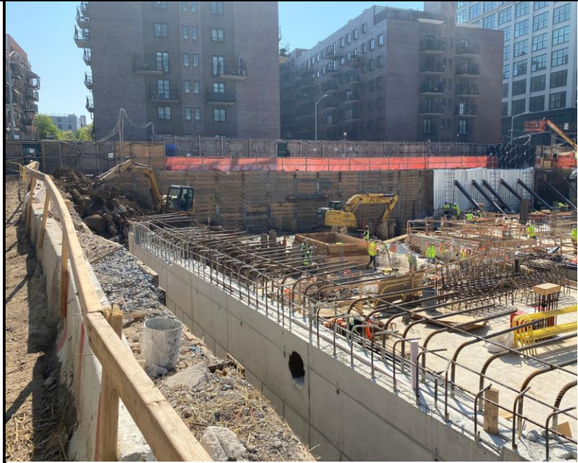
Photo 3: View of soil excavation and lagging installation facing east.
