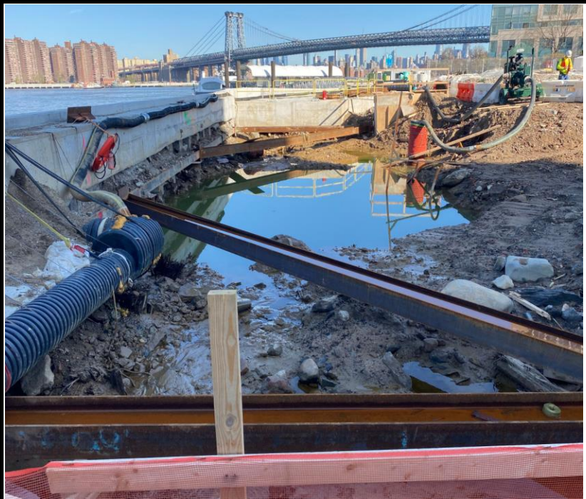
Photo 2: View of remedial excavation dewatering at the start of the workday.
