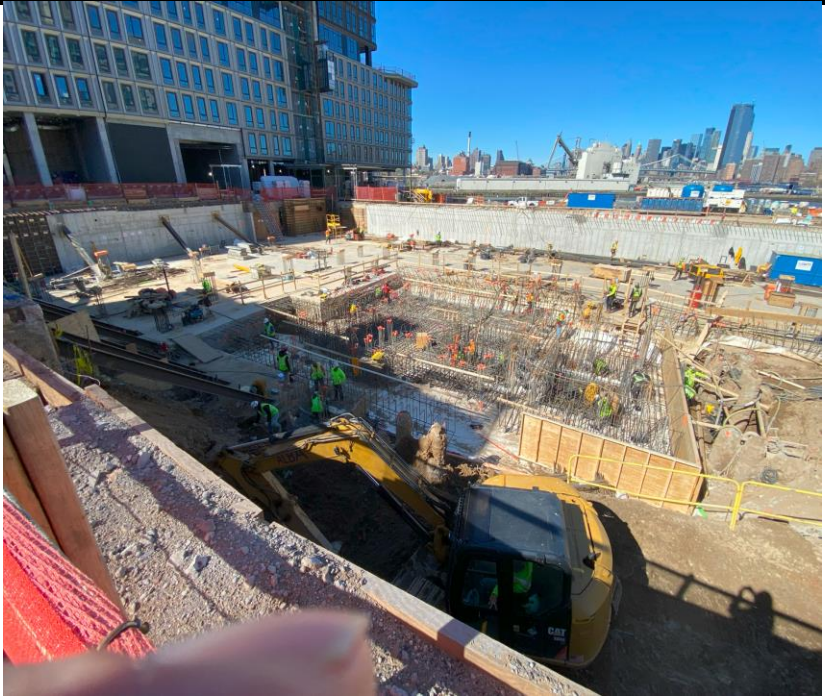
Photo 2: View of Site conditions facing southwest.
