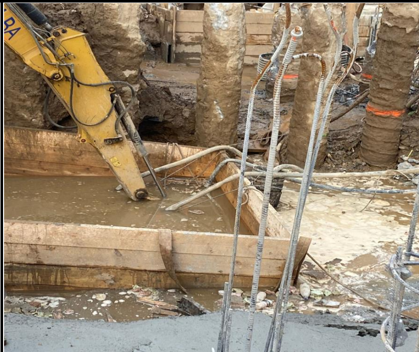
Photo 4: View of turbid water causing dewatering issue. The dewatering system was left off over night and maintenance was completed the next morning prior to restarting the system.
