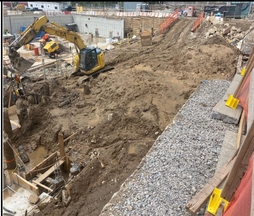
Photo 2: View of Site conditions facing northwest.
