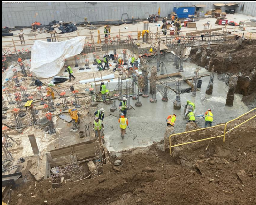
Photo 3: View of concrete pouring for continued building foundation development.
