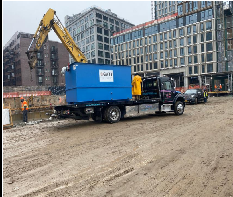
Photo 4: View of settling tank delivery.
