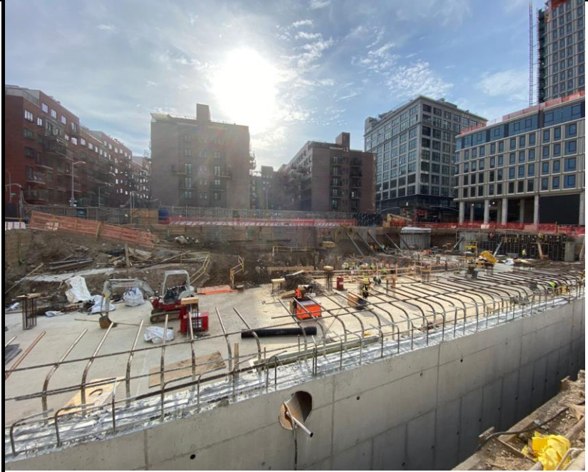
Photo 1: View of Site conditions and activities facing east.
