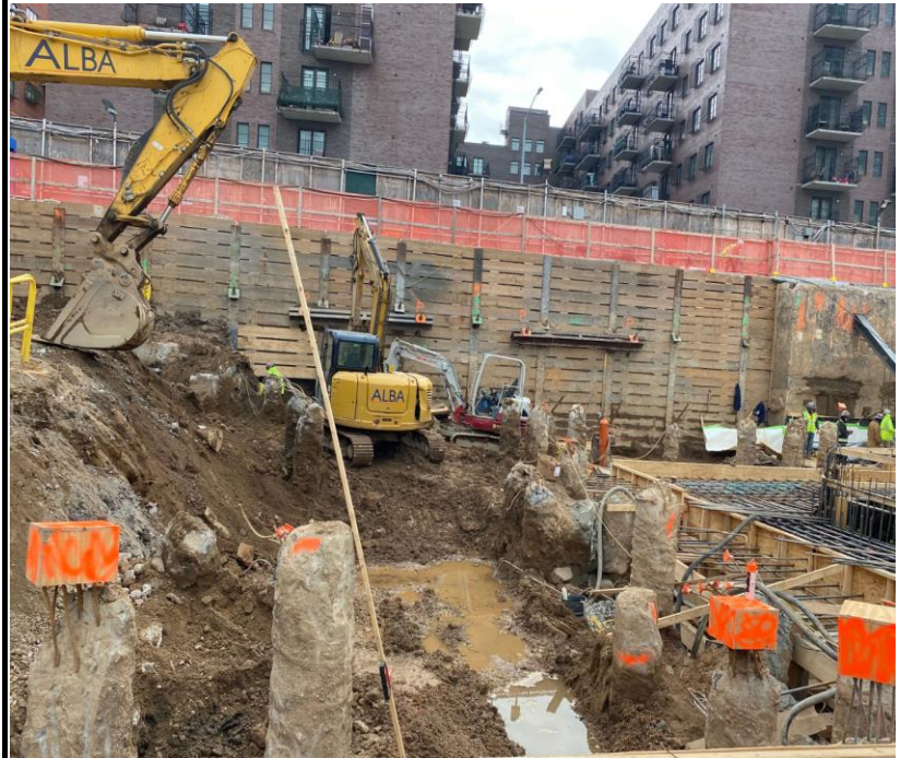
Photo 2: View of soil excavation and SOE installation.
