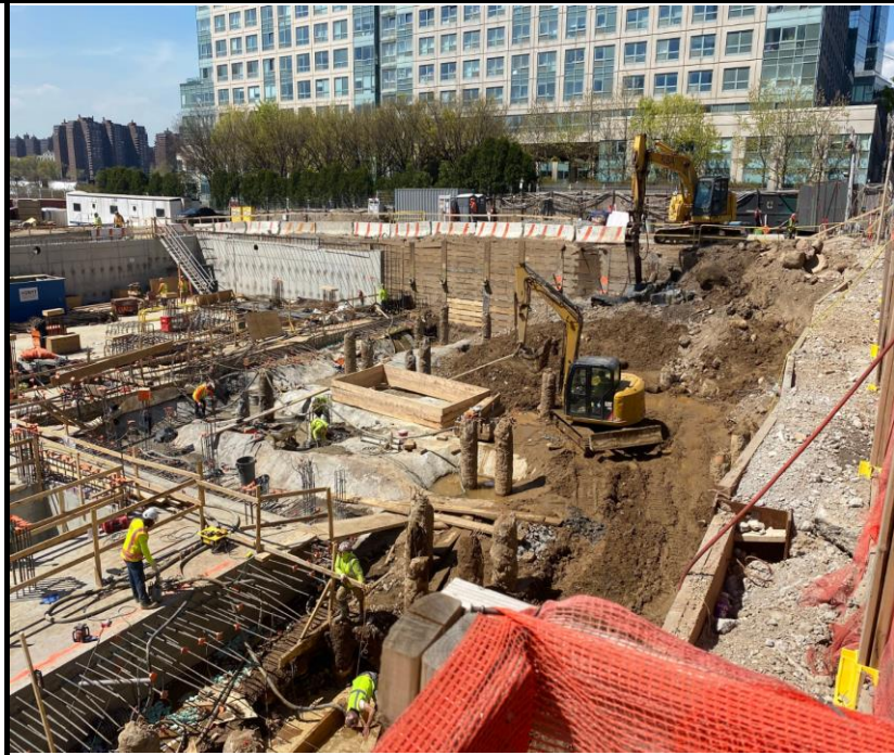
Photo 4: View of Site conditions facing northwest.
