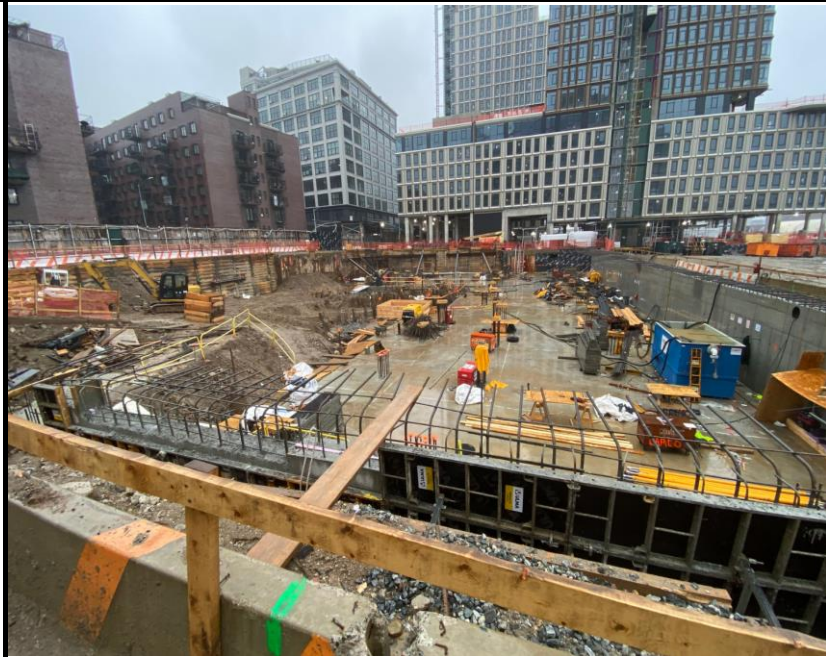
Photo 1: View of Site conditions facing south.
