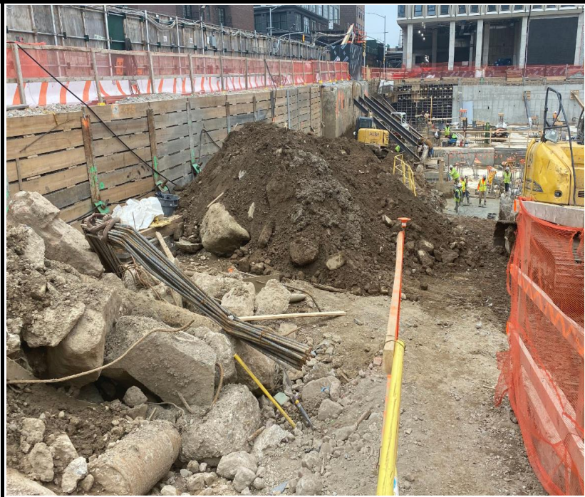
Photo 4: View of soil excavation and stockpiling.
