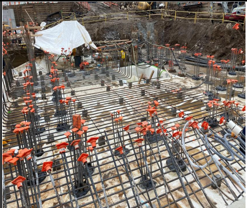
Photo 4: View of waterproofing and rebar installation.
