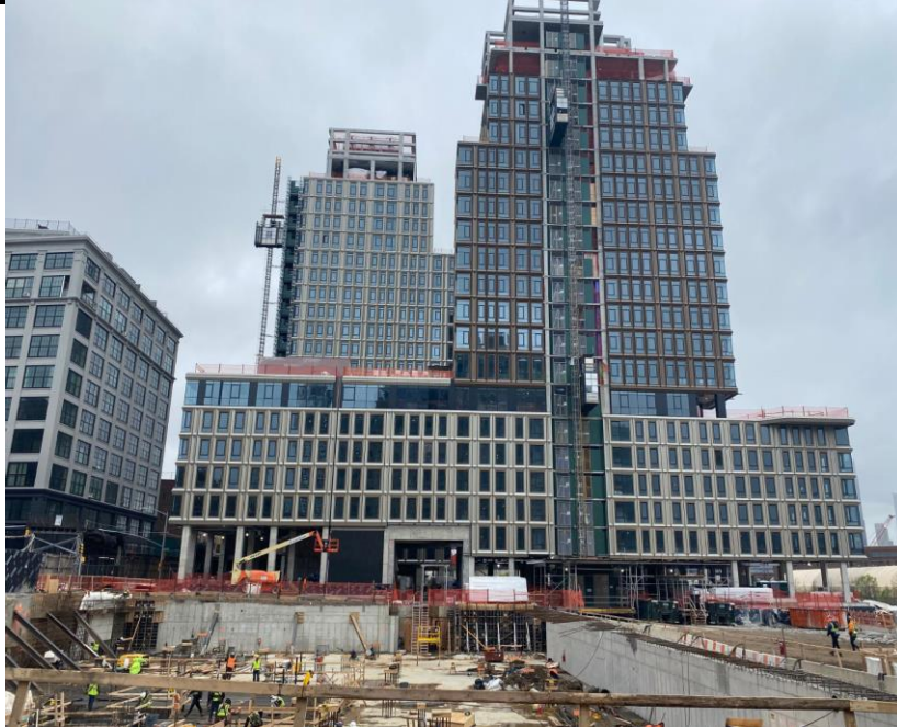
Photo 3: View of Site conditions and A1/A2 building development facing south.
