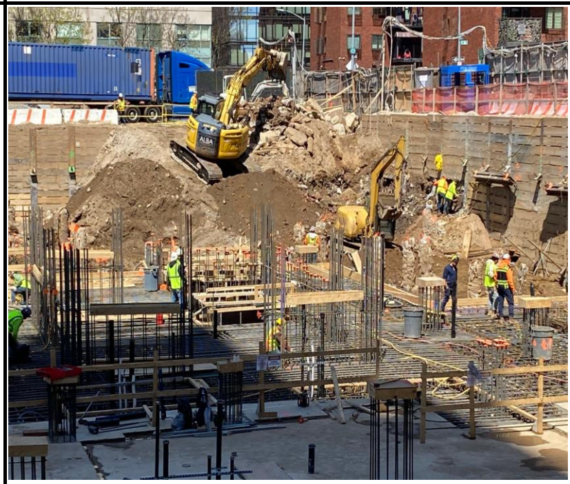
Photo 2: View of soil excavation and stockpiling.
