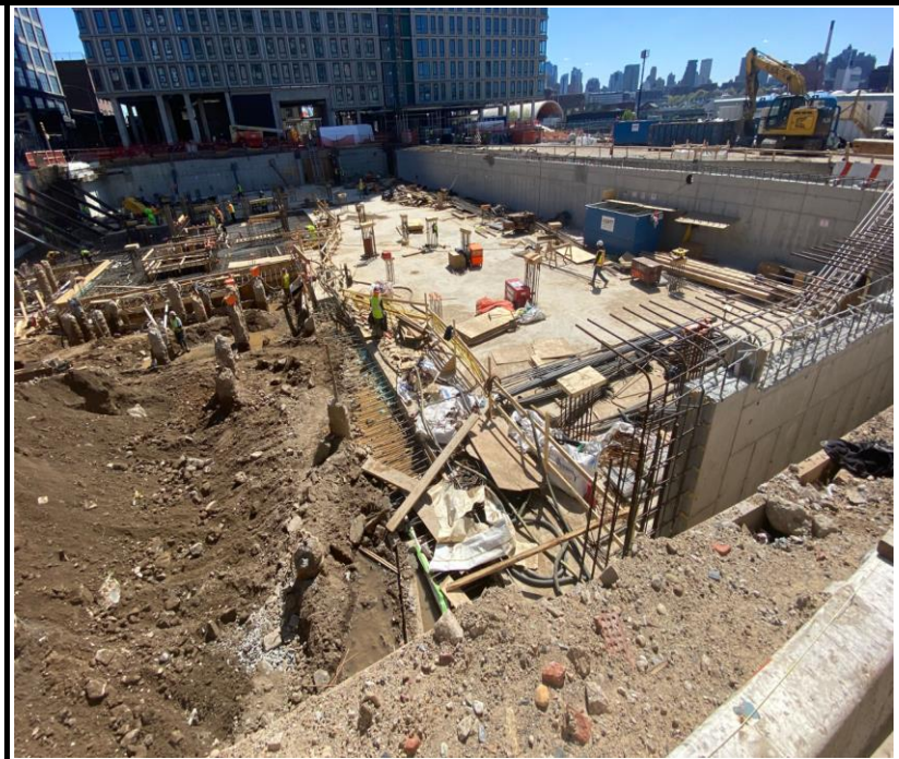
Photo 4: View of Site conditions facing southwest.
