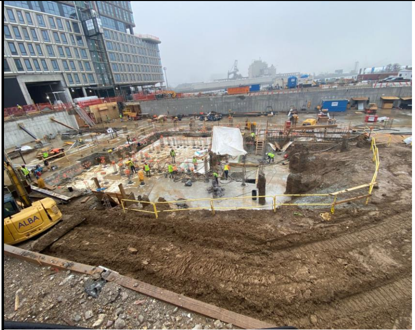
Photo 1: View of Site conditions and activities facing west.
