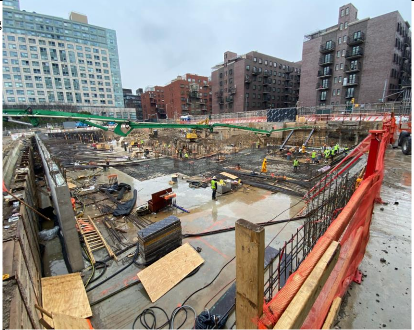
Photo 1: View of concrete pouring and Site conditions facing northeast.
