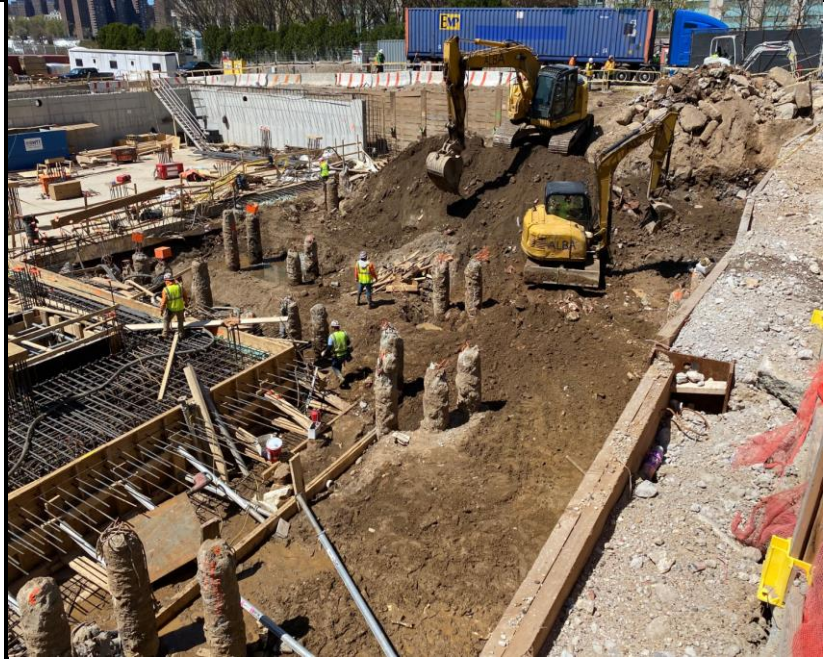
Photo 3: View of soil excavation, stocpiling and site conditions facing north.
