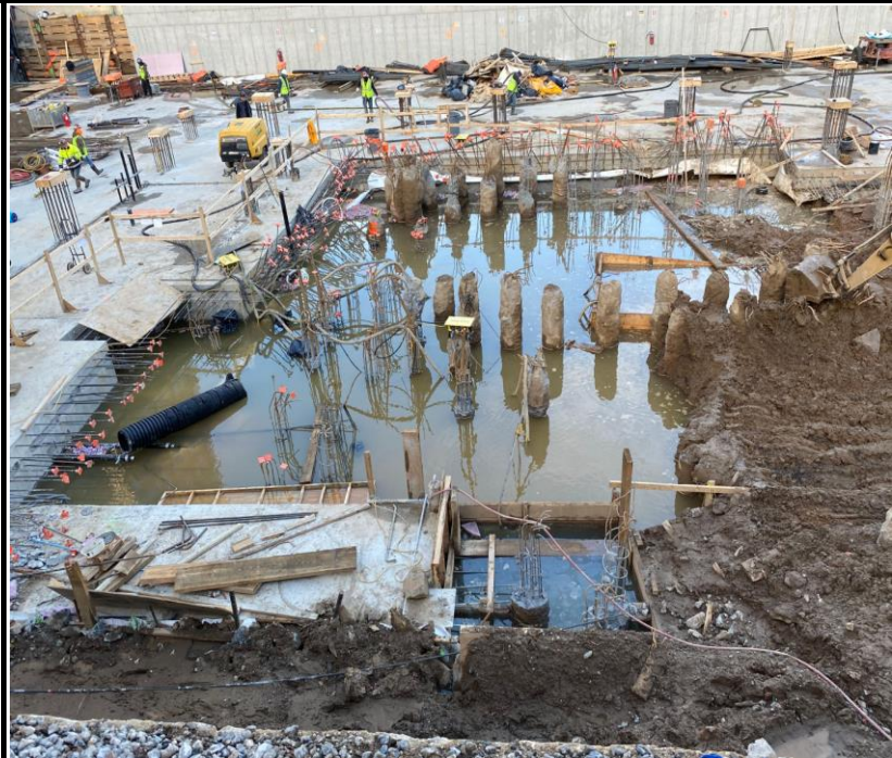
Photo 4: View of the Site prior to restarting the dewatering system.
