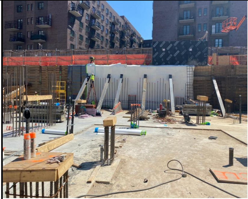
Photo 3: View of waterproofing installation facing east.
