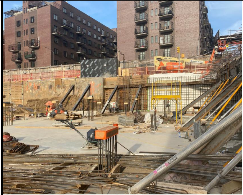
Photo 3: View of waterproofing and rebar installation facing east.
