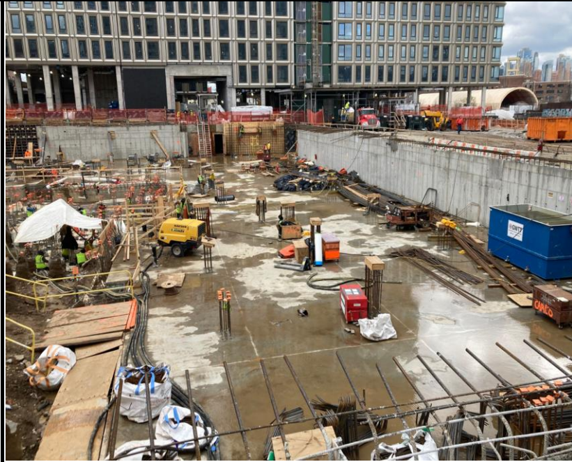
Photo 3: View of building foundation development and Site activities facing south.
