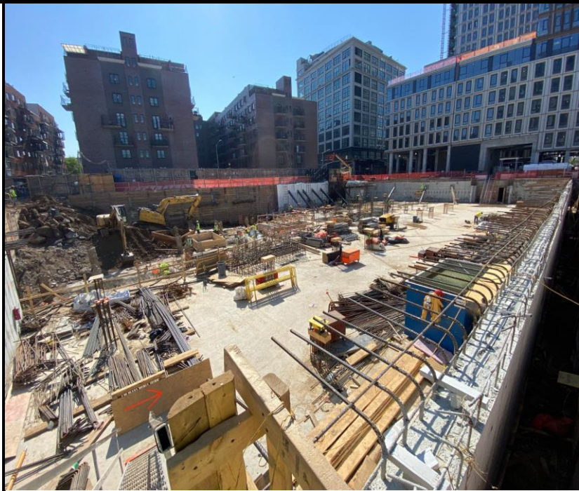
Photo 2: View of site conditions and activities facing southeast.
