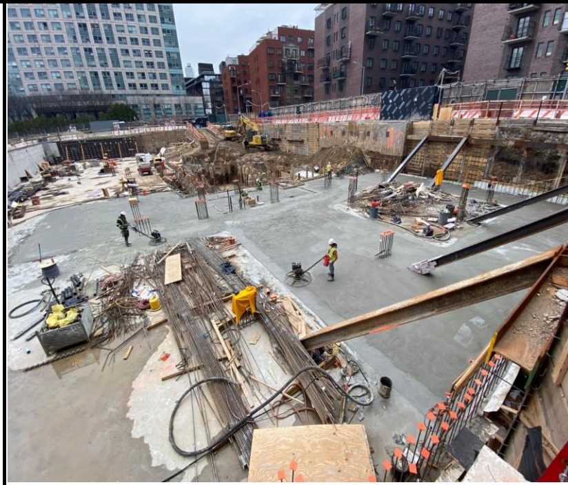
Photo 4: View of the the continued building foundation development.
