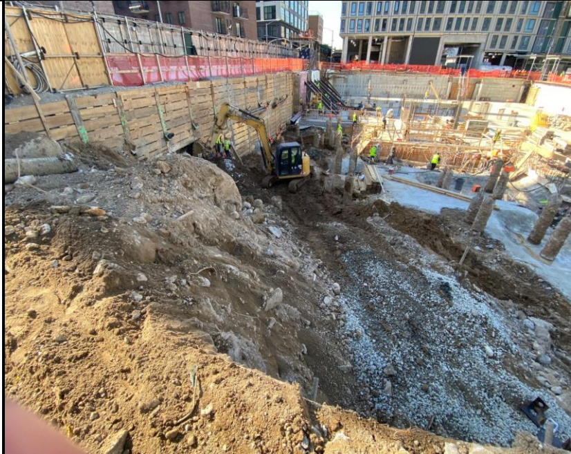
Photo 1: View of soil excavation and lagging installation.
