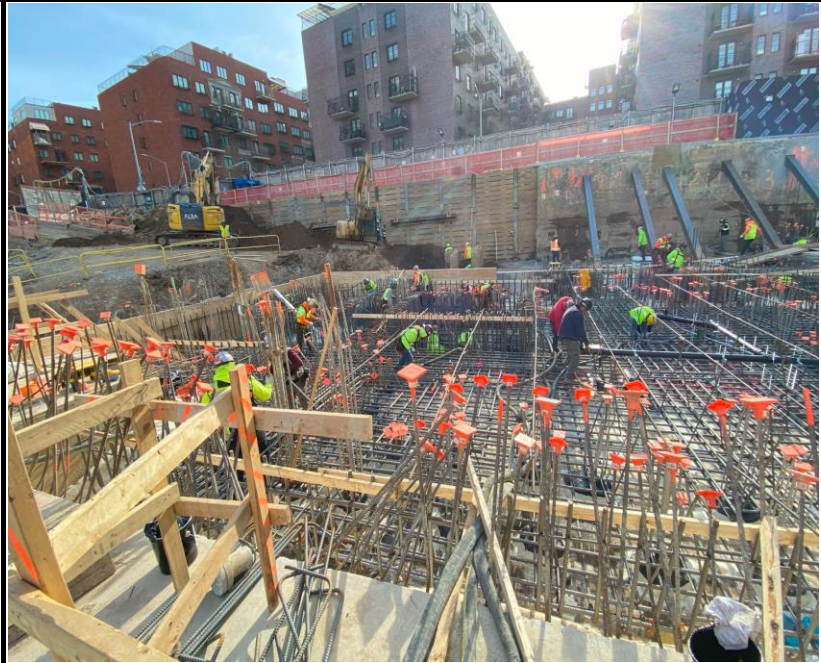
Photo 3: View of Site conditions and rebar installation facing east.
