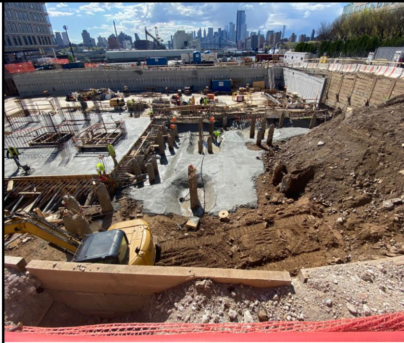
Photo 4: View of Site conditions after concrete pouring facing west.
