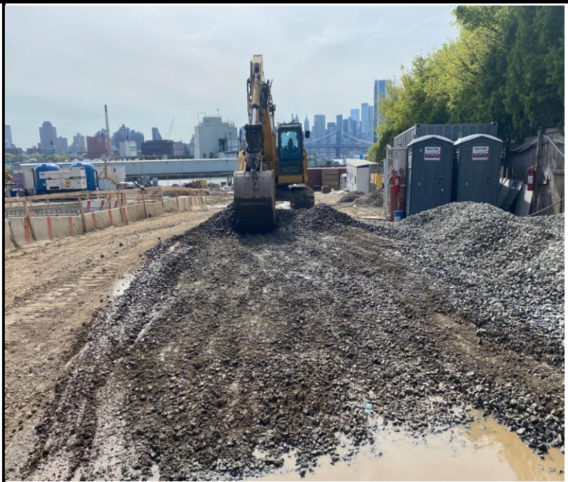
Photo 2: View of stone refreshing in truck wash pad, facing west.
