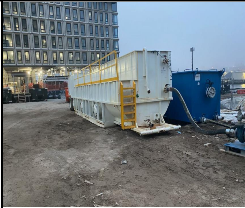
Photo 4: View of additional settling tank brought on-site by GWTT, the dewatering contractor, for additional sediment removal.
