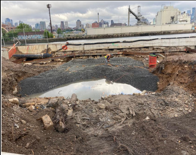
Photo 1: View of the remedial excavation facing west.
