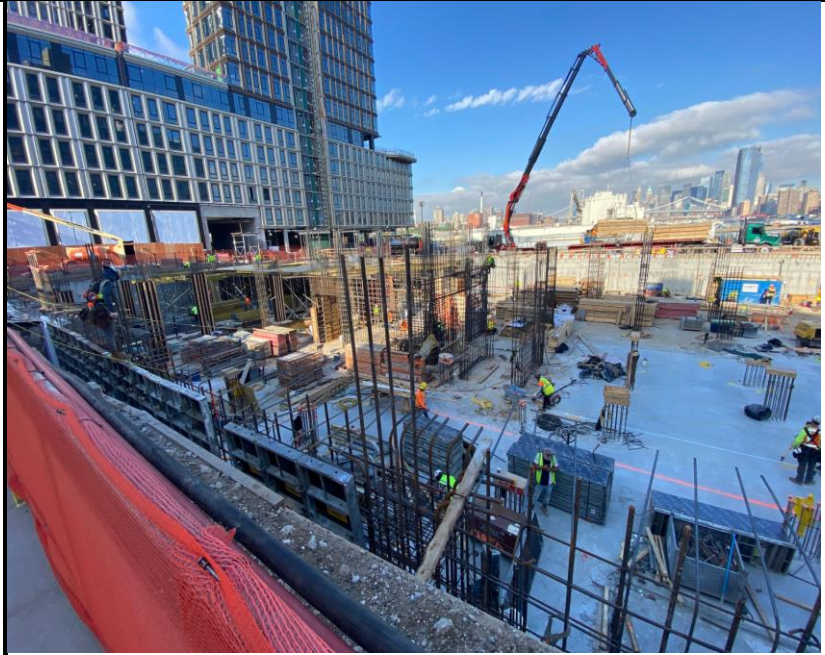
Photo 1: View of Site conditions and foundation development facing southwest.
