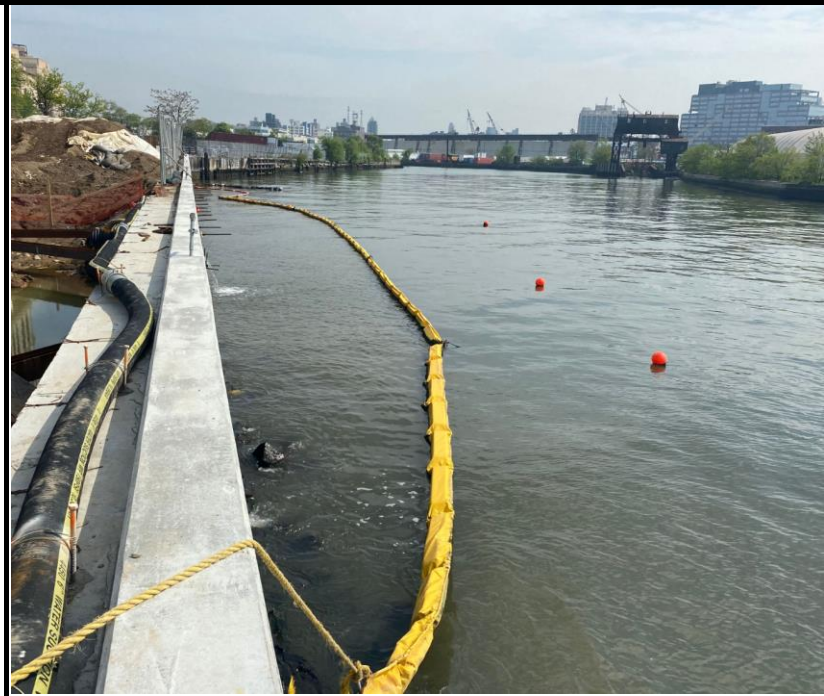
Photo 4: View of the dewatering effluent and turbidity curtain.
