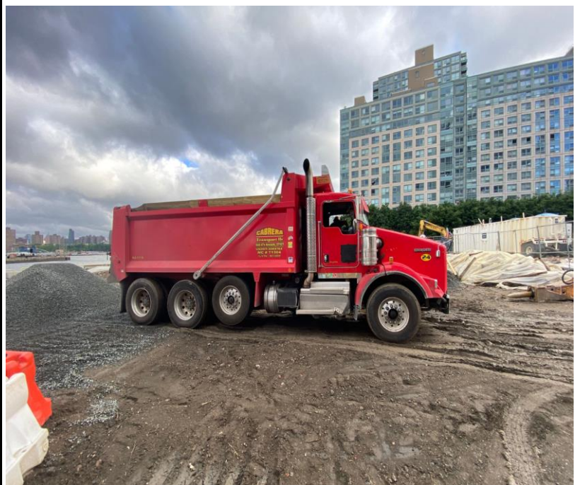
Photo 2: View of stone delivery for the remedial excavation backfilling.
