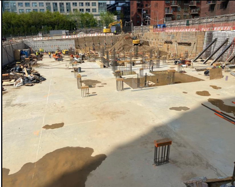
Photo 3: View of Site conditions facing north.
