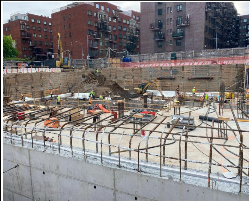
Photo 1: View of Site conditions and soil excavation facing northeast.
