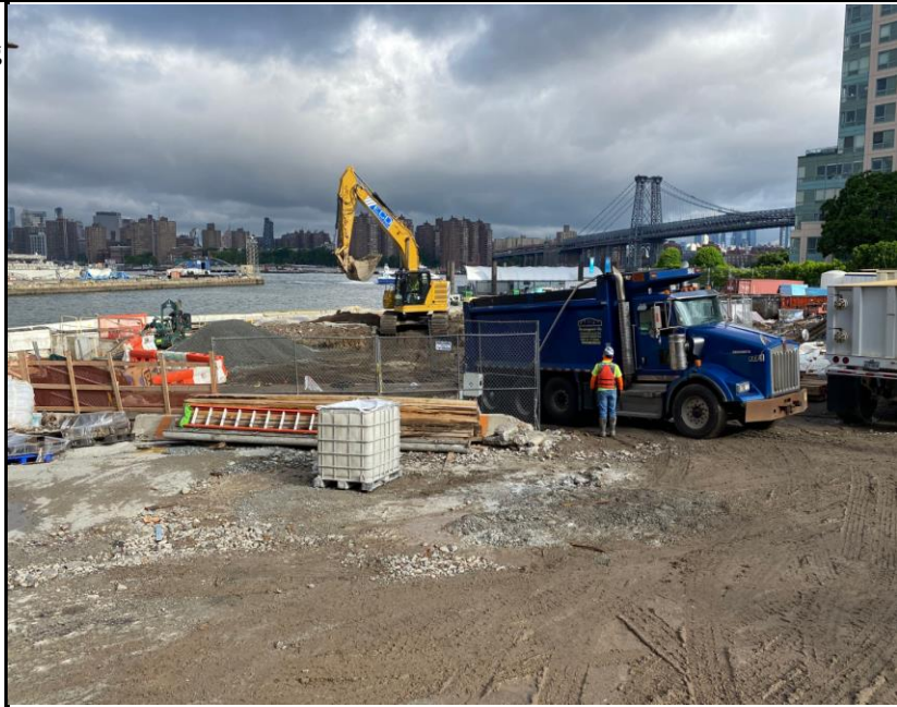
Photo 3: View of truck loading for off-site soil disposal from the remedial excavation.
