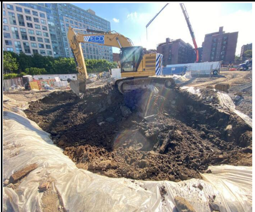
Photo 2: View of soil excavation and disposal from the remedial excavation.
