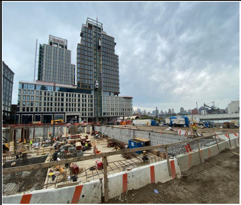
Photo 4: View of site conditions and continued A1/A2 building construction.
