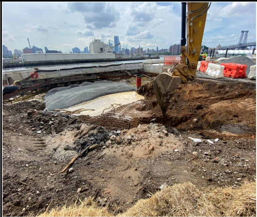
Photo 4: View of continued excavation for the remedial excavation.
