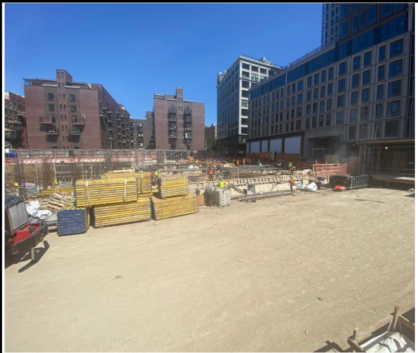
Photo 4: View of Site conditions facing east.
