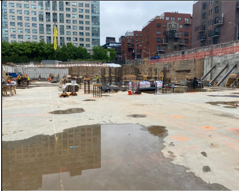
Photo 3: View of Site conditions facing north.
