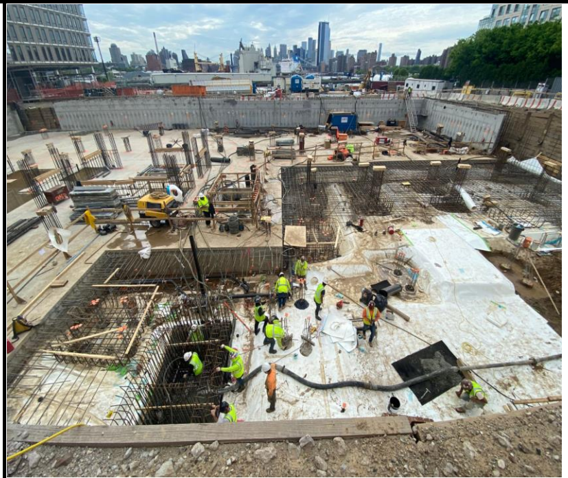
Photo 4: View of Site activities and waterproofing installation.
