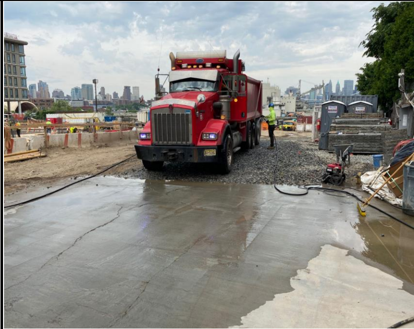
Photo 3: View of tire washing prior to trucks leaving the Site.
