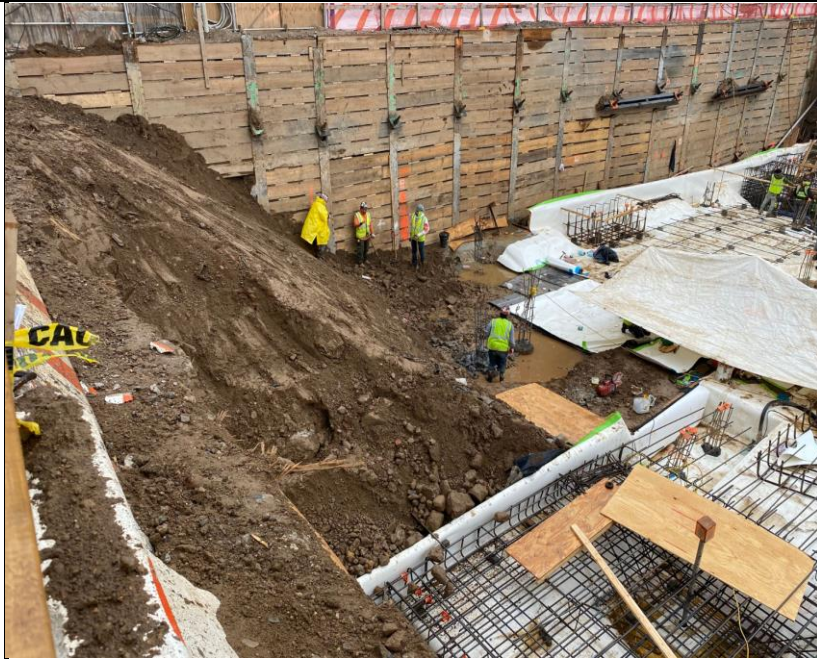
Photo 3: View of remaining soil for off-site disposal.
