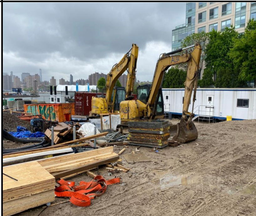
Photo 4: View of staged excavators.
