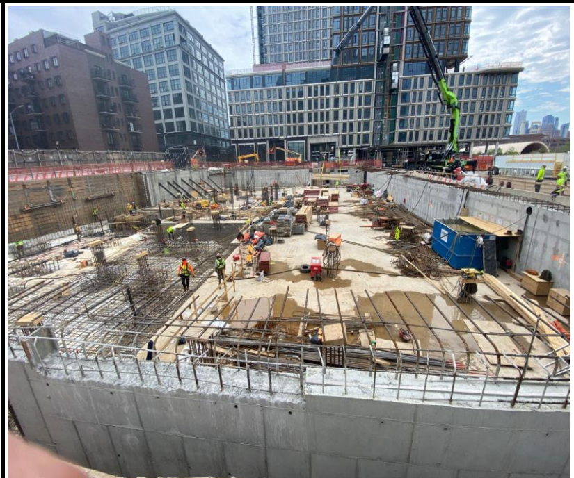
Photo 2: View of Site conditions and foundation development facing south.
