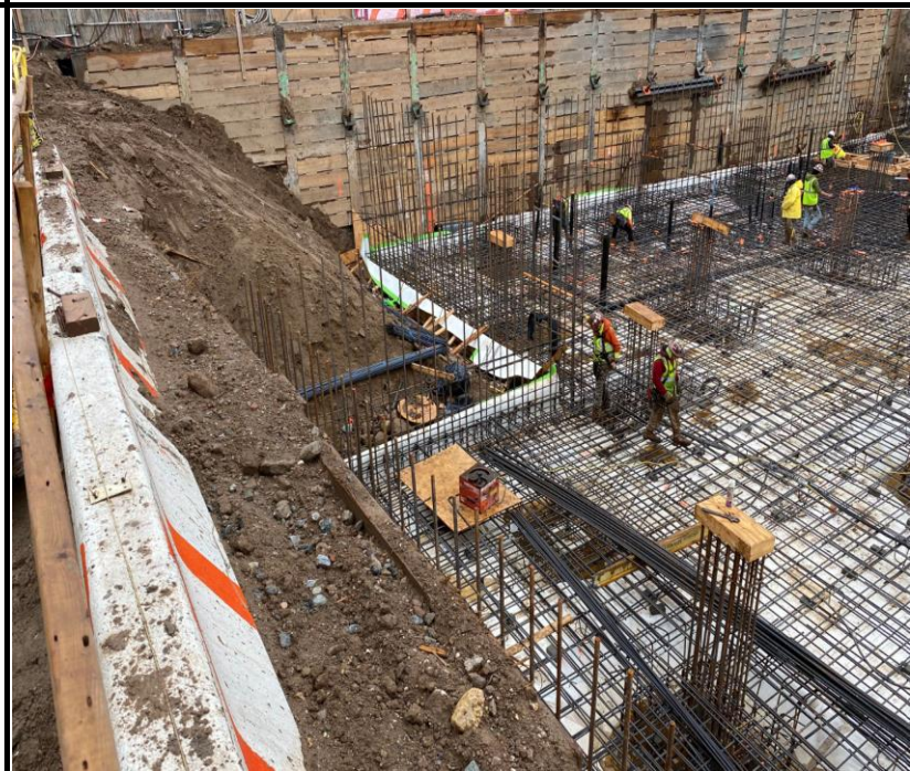
Photo 4: View of rebar and waterproofing installation.
