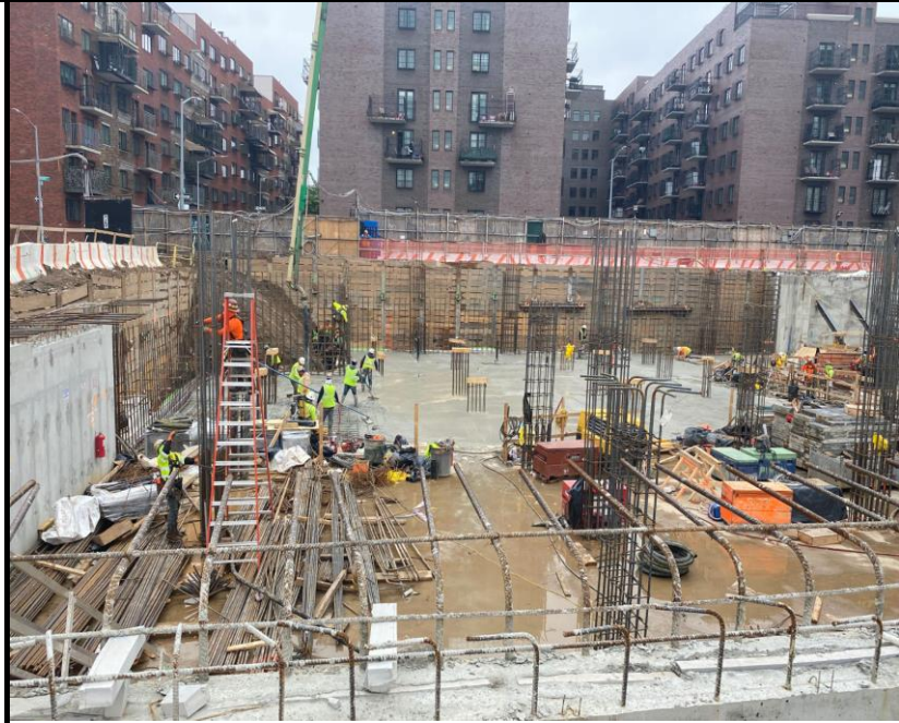
Photo 3: View of concrete pouring for concrete building slab development facing northeast.
