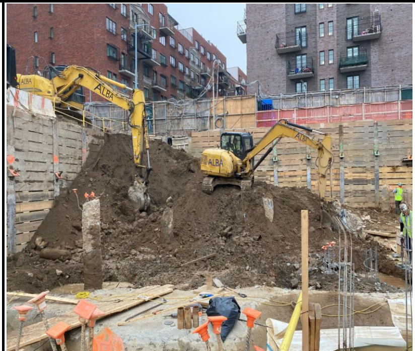
Photo 4: View of soil excavation facing east.
