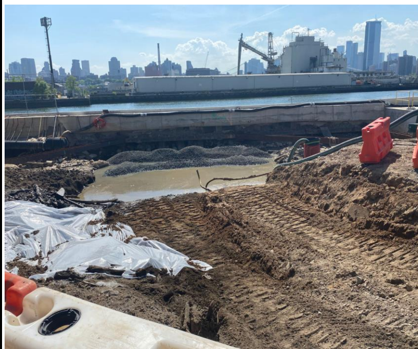
Photo 4: View of the remedial excavation facing west.
