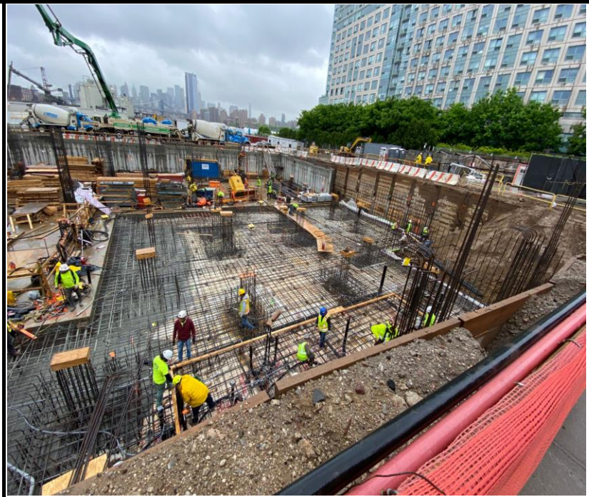
Photo 2: View of Site conditions and foundation development facing northwest.
