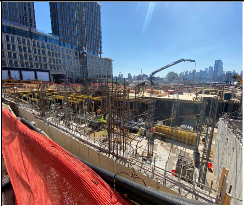
Photo 2: View of the foundation development facing west.
