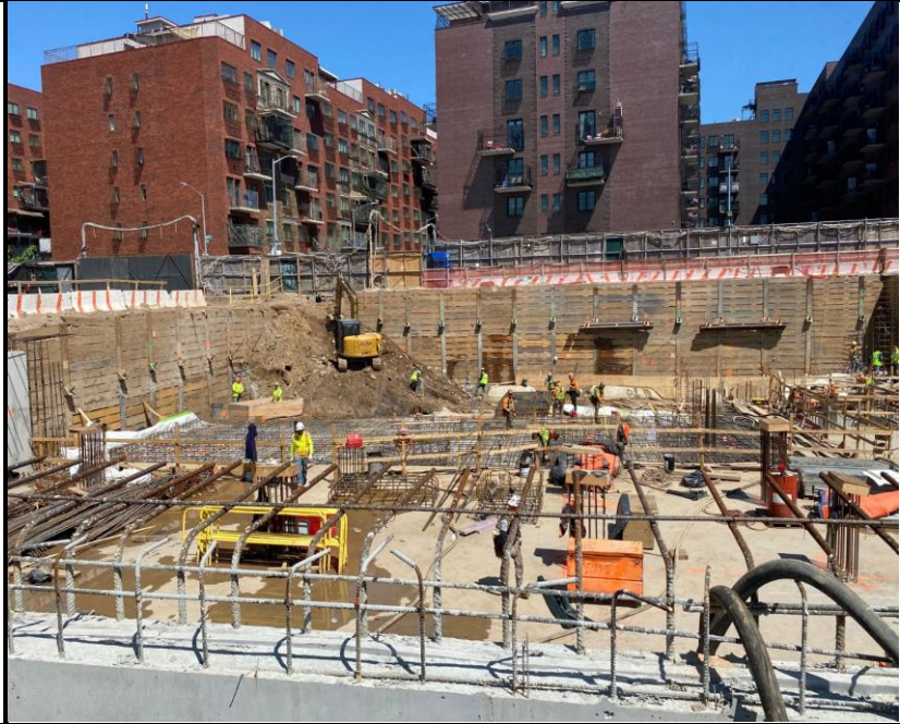
Photo 1: View of Site conditions and activities facing northeast.
