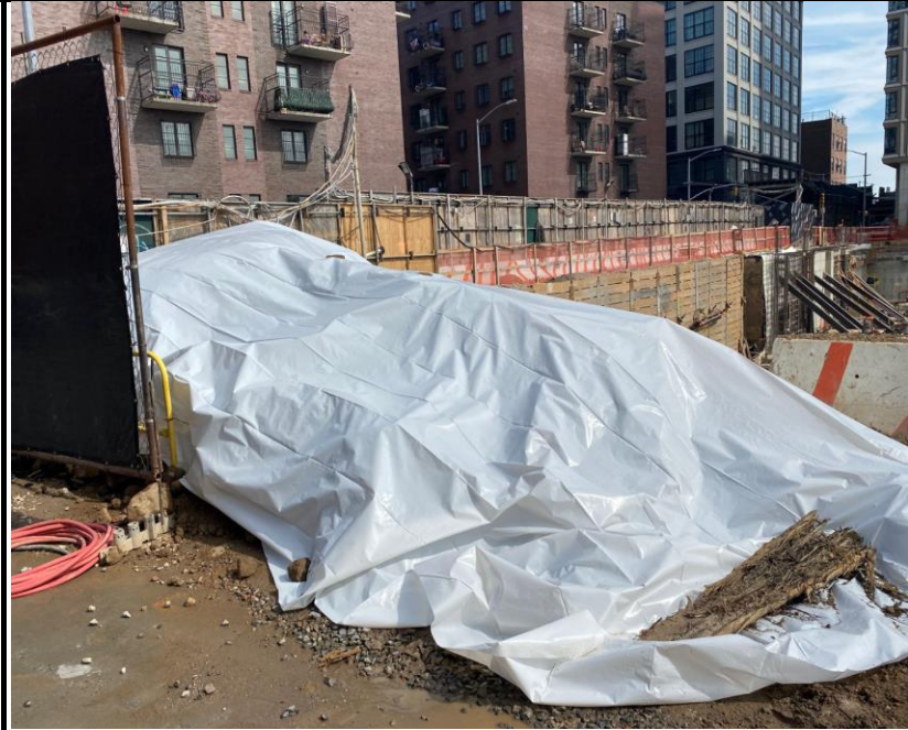
Photo 3: View of covered soil stockpile in preparation for off- site soil disposal.
