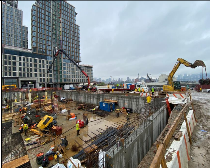
Photo 3: View of rebar installation facing southwest.
