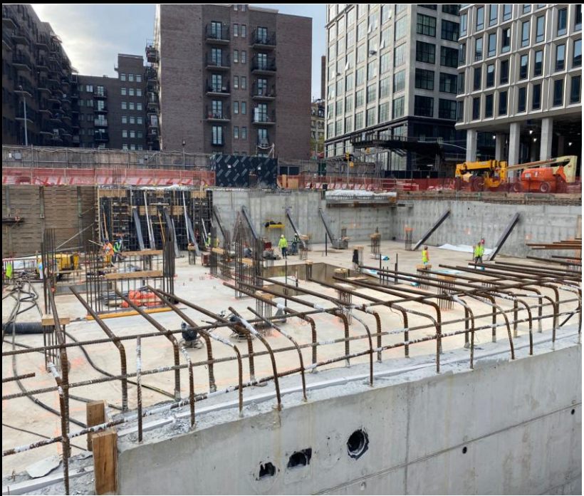
Photo 2: View of Site conditions facing east.
