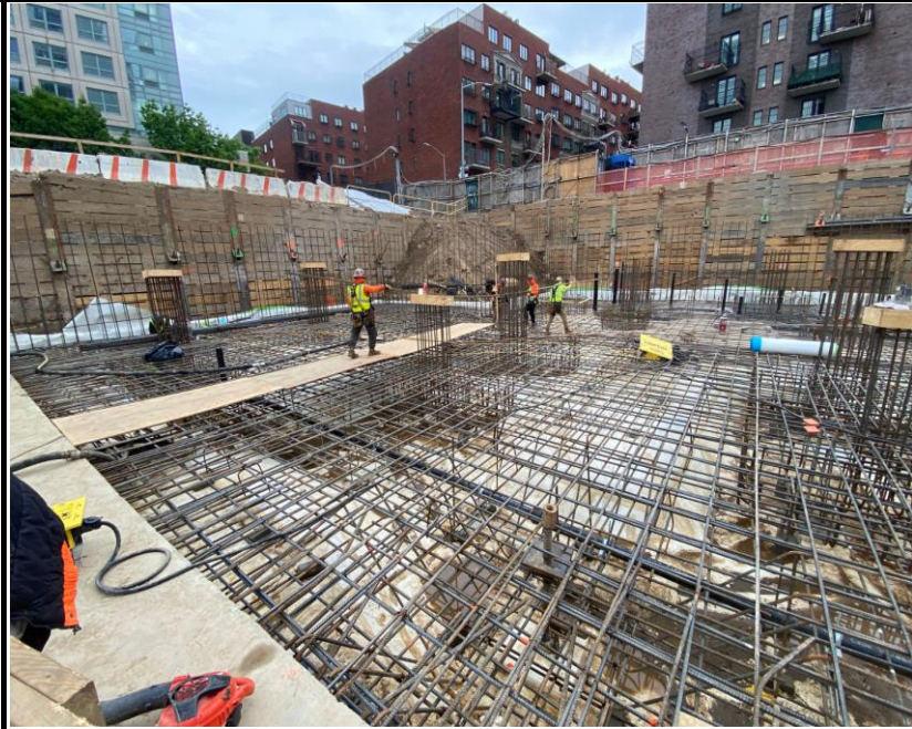
Photo 3: View of rebar installation facing northeast.
