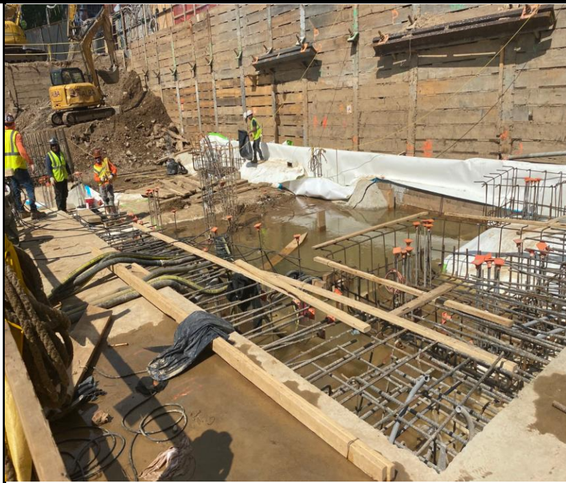
Photo 4: View of Site activities and waterproofing installation.
