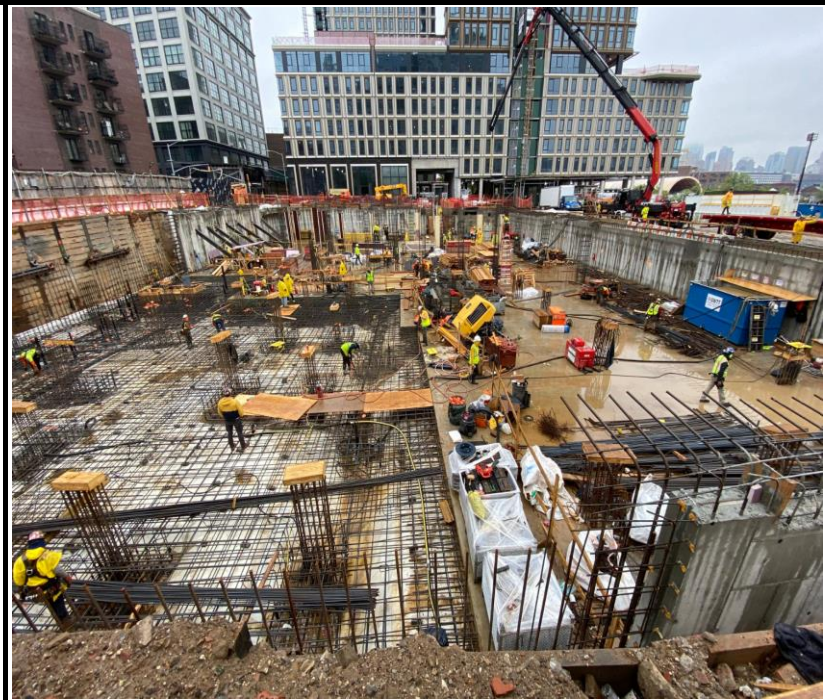
Photo 2: View of Site conditions and foundation development facing south.
