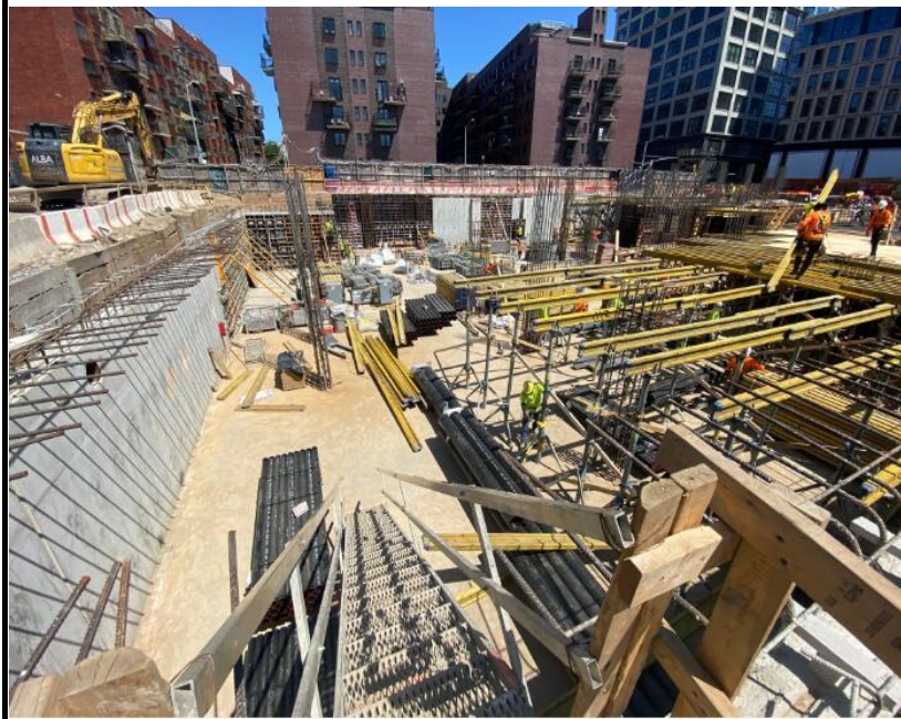
Photo 1: View of Site conditions facing east.
