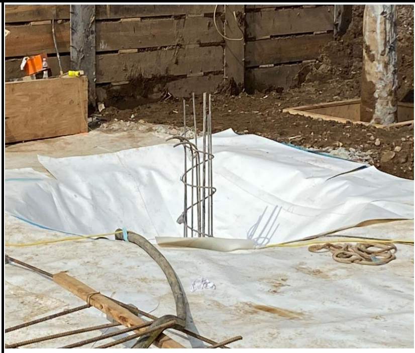
Photo 2: View of waterproofing installation.
