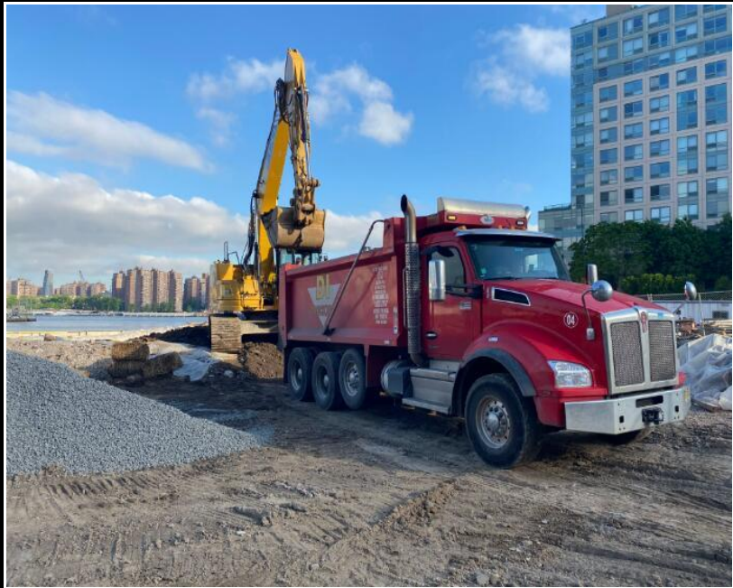
Photo 3: View of truck loading with soil from remedial excavation for off-site soil disposal.
