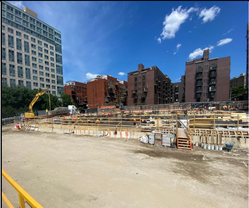
Photo 4: View of the Site and foundation development facing northeast.
