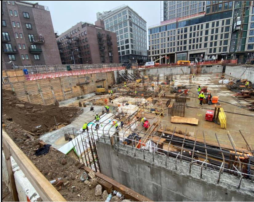
Photo 1: View of Site conditions and activities facing southeast.
