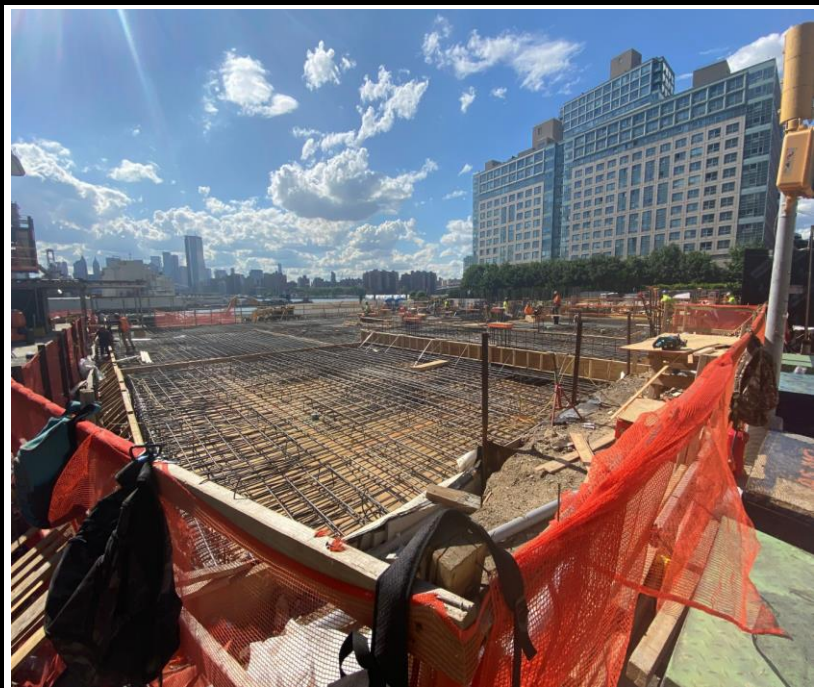
Photo 4: View of the Site and foundation development facing northwest.
