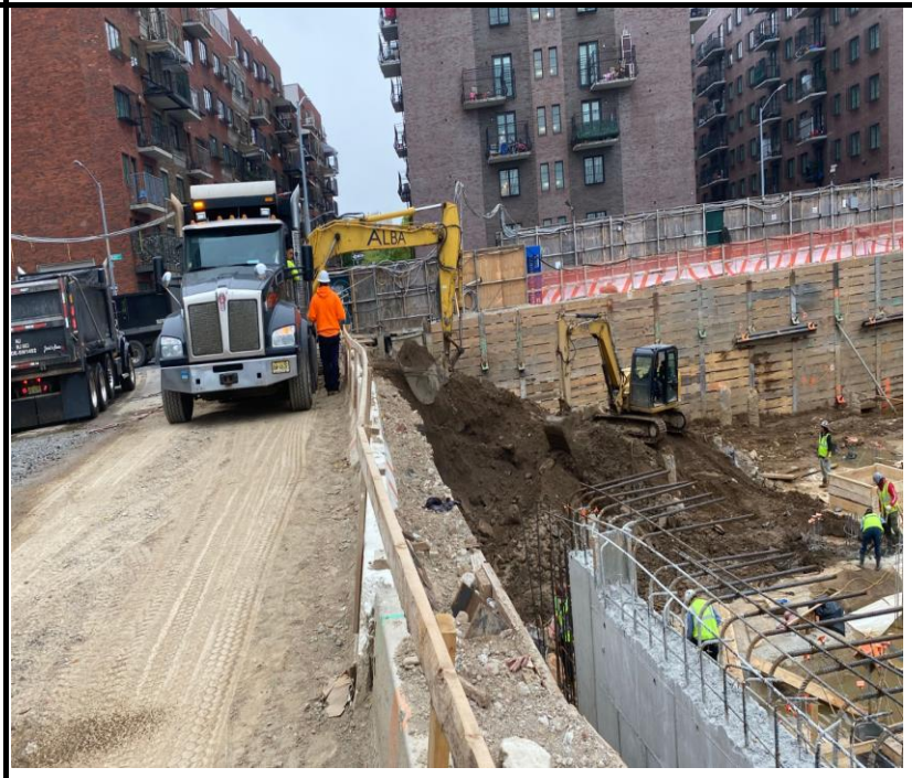
Photo 2: View of soil excavation and truck loading for off- site soil disposal.
