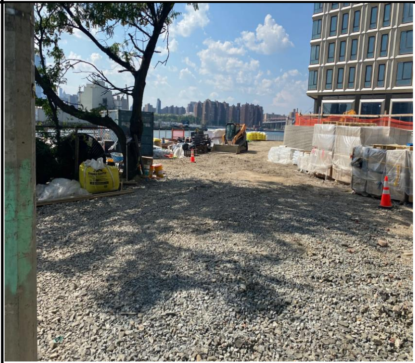
Photo 2: View of the southwest corner, facing northwest.
