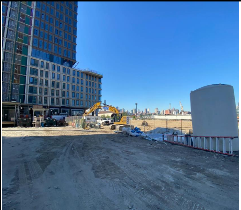
Photo 2: View of continued Site conditions facing southwest.
