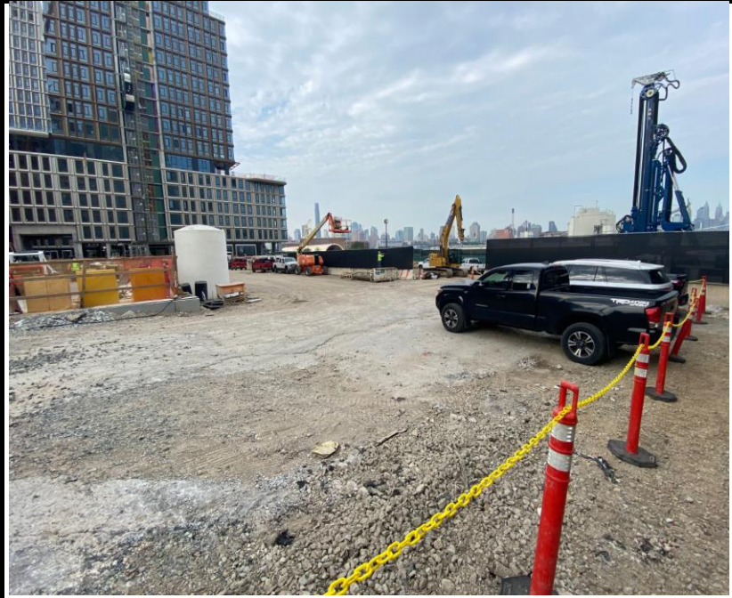
Photo 1: View of Site conditions facing west.
