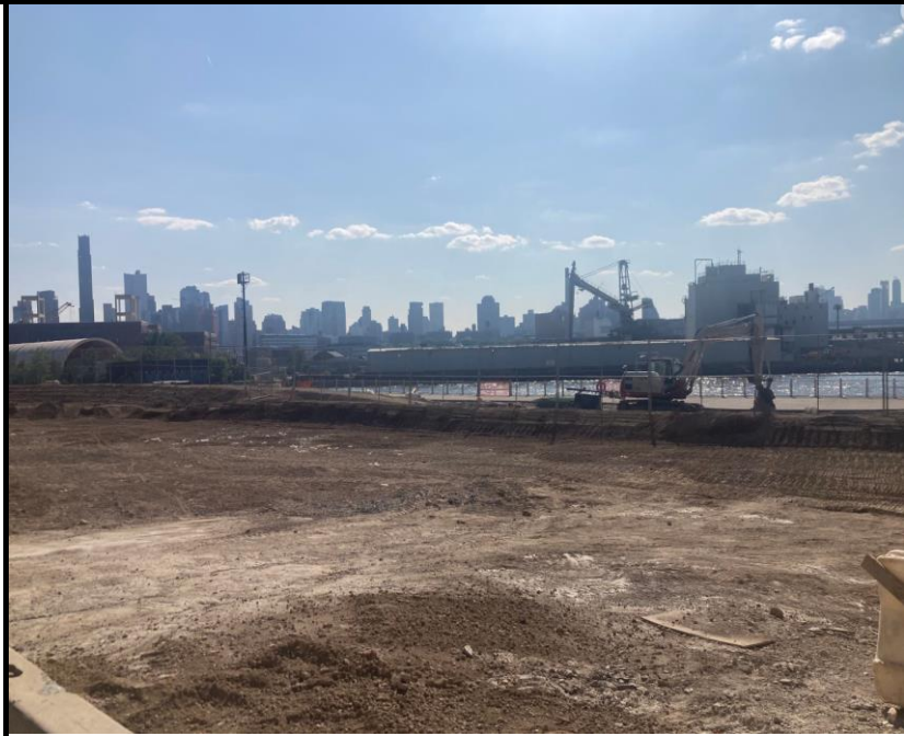
Photo 1: View of Site conditions facing west.
