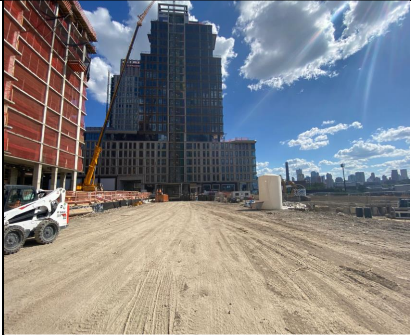
Photo 3: View of continued structure development.
