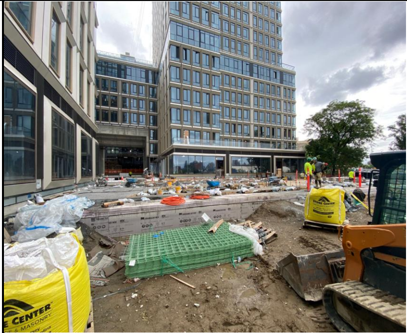
Photo 3: View of continued landscaping work in the southwest corner of the Site.
