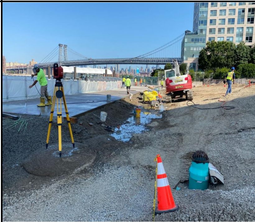
Photo 2: View of continued concrete work on the marine front.
