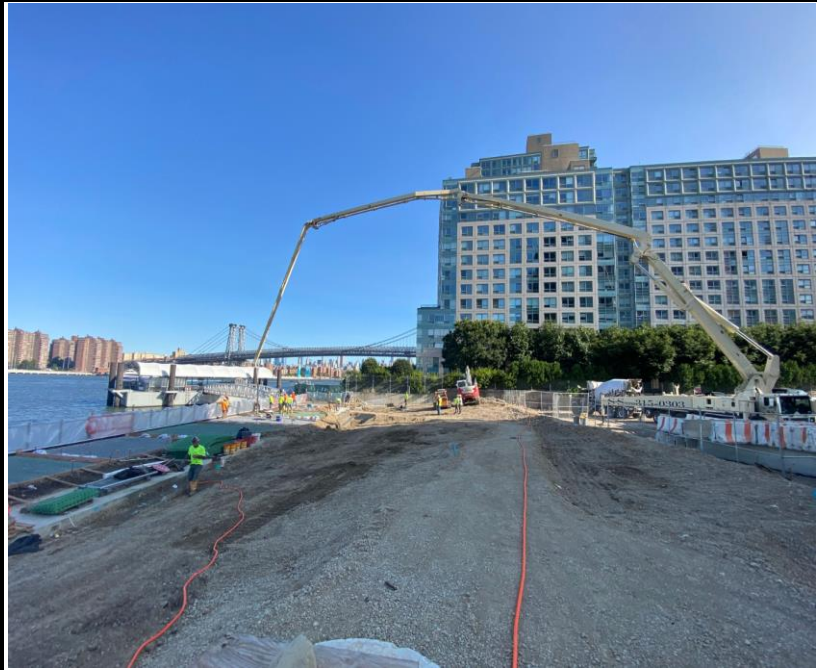
Photo 3: View of concrete pour along the marine front
