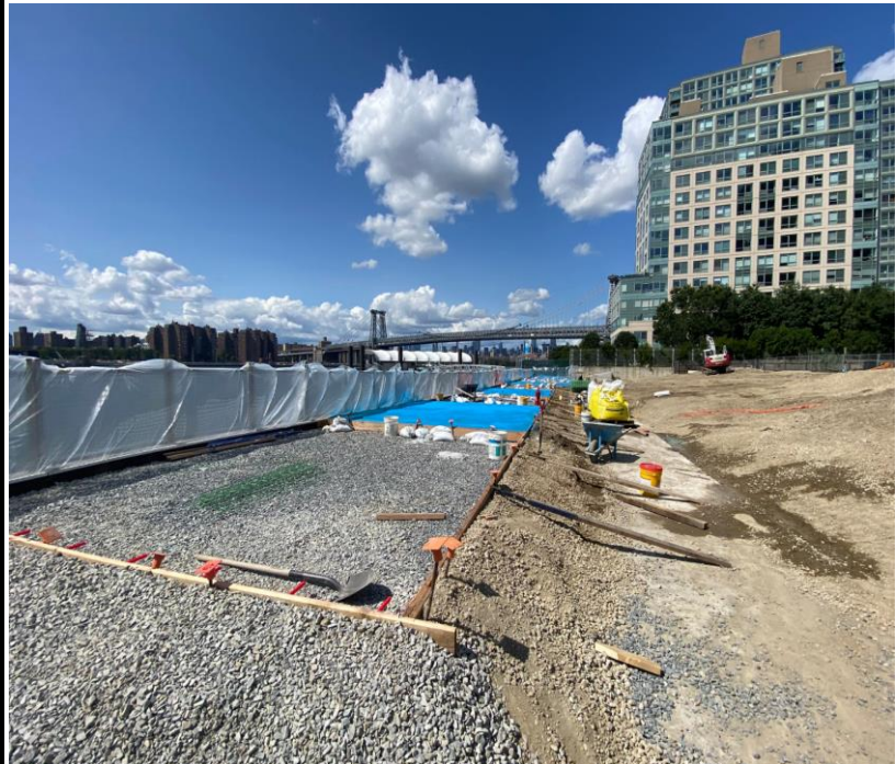
Photo 4: View of Site conditions along the marine front.
