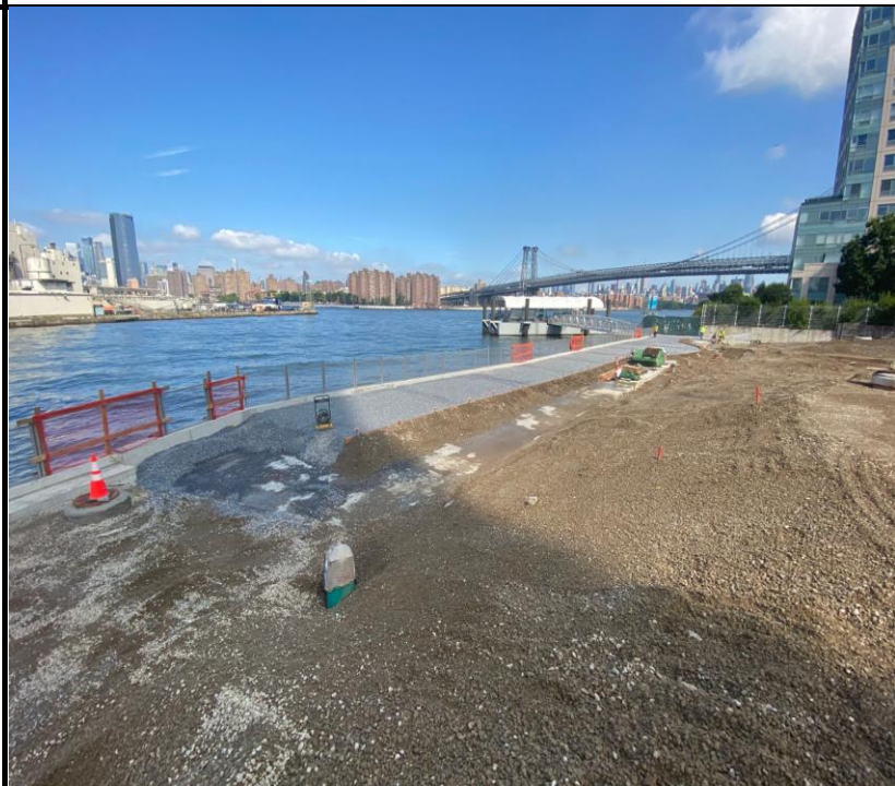
Photo 4: View of preparation for concrete pour along the marine front.
