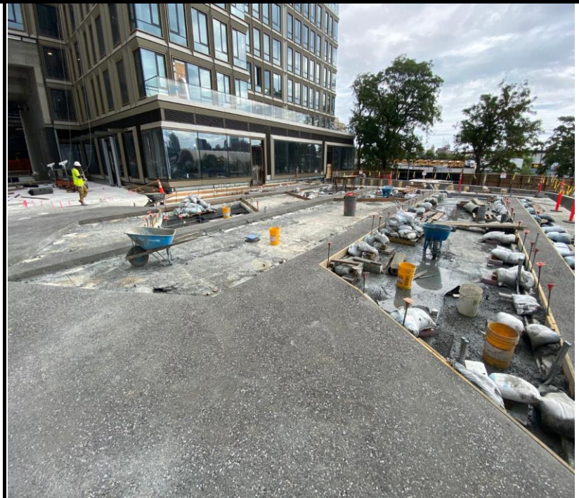
Photo 4: View of continued landscaping work in the southwest corner of the Site.
