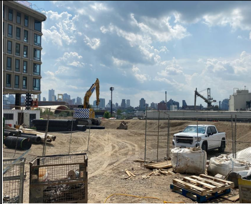
Photo 3: View of site conditions facing west.
