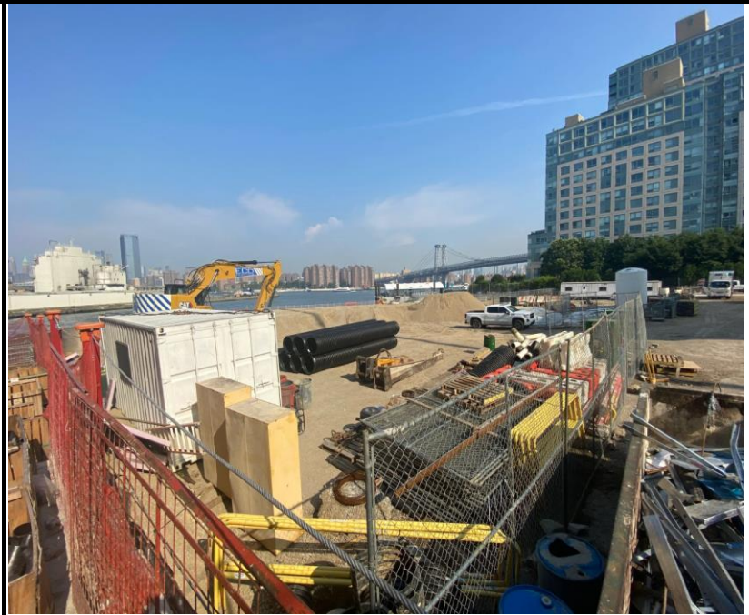
Photo 1: View of Site conditions facing northwest.
