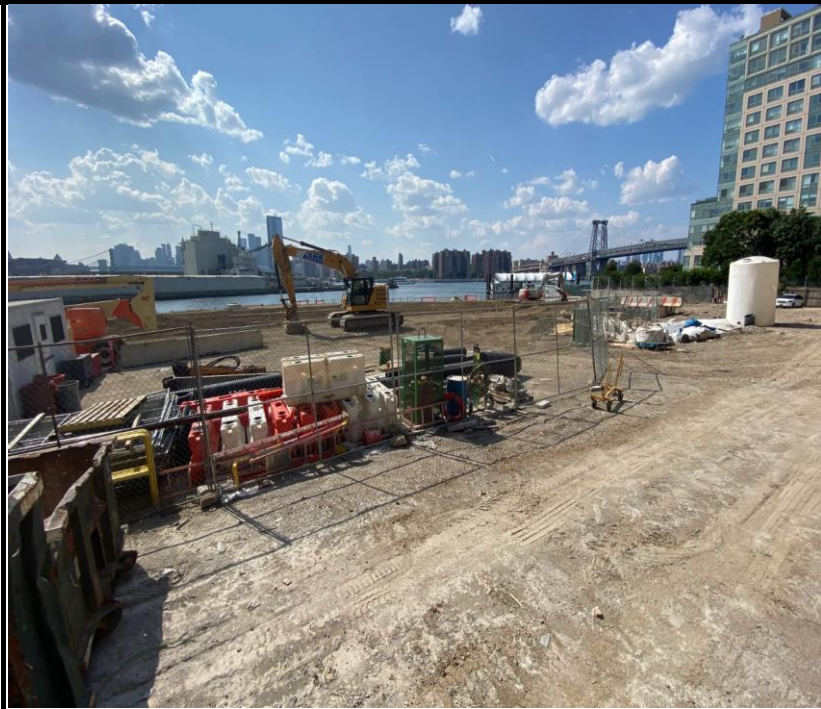
Photo 4: View of Site conditions in the marine front facing northwest.
