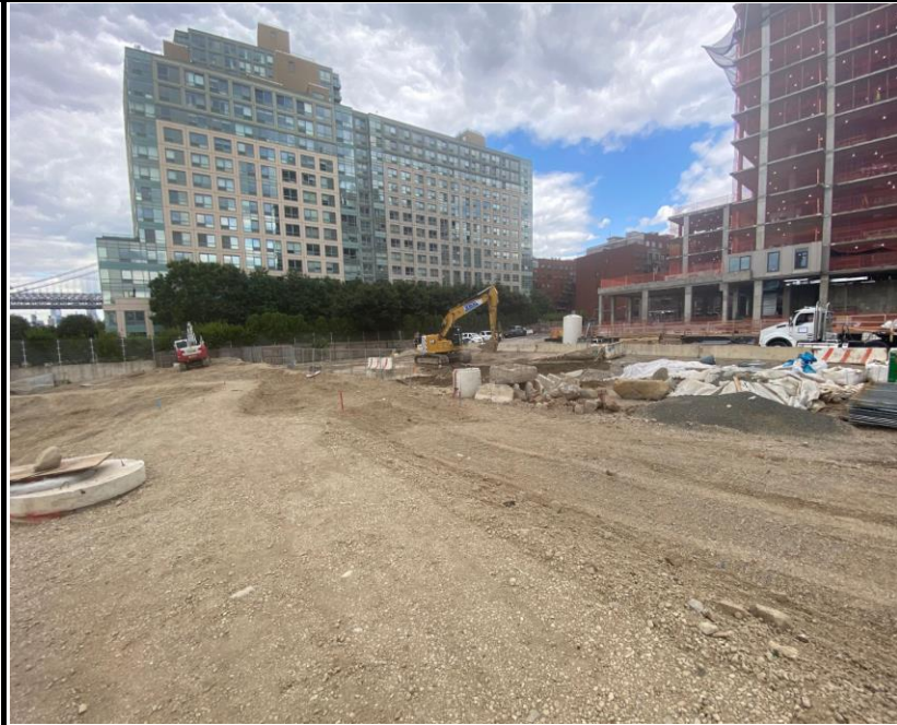
Photo 3: View of Site conditions facing northeast.
