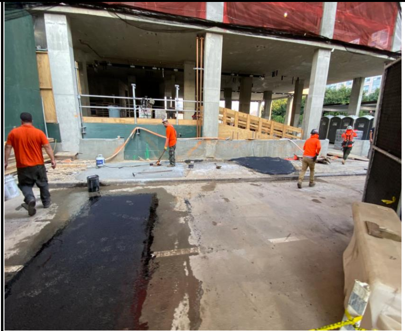
Photo 1: View of completed vault excavations along Kent Avenue.
