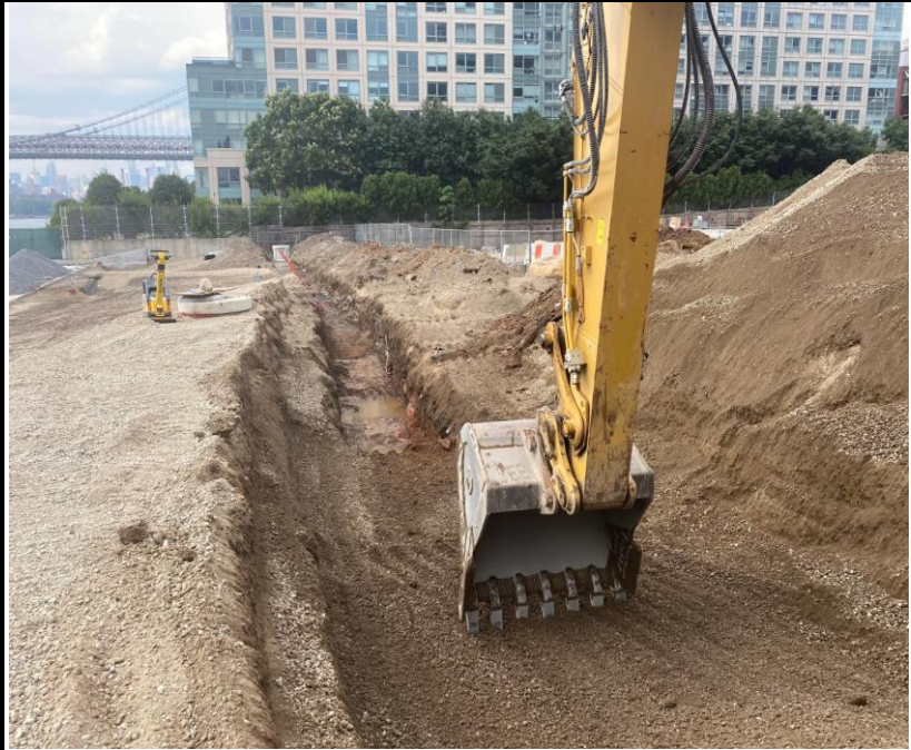
Photo 3: View of soil excavation for piping installation for the stormwater system in the marine front, facing north.
