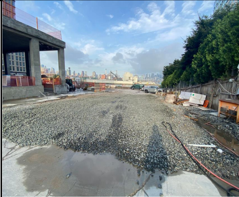
Photo 3: View of the trucking pad along Kent Avenue, facing west.
