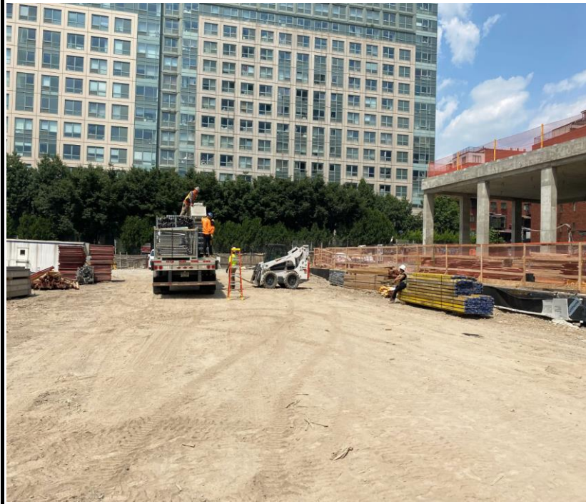
Photo 4: View of equipment mobilization and Site conditions facing north.
