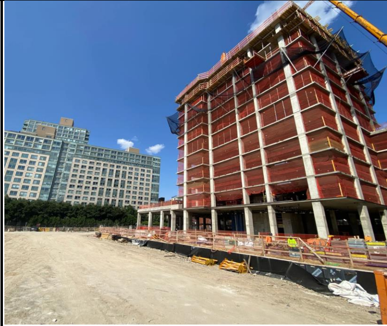
Photo 3: View of continued structure development.
