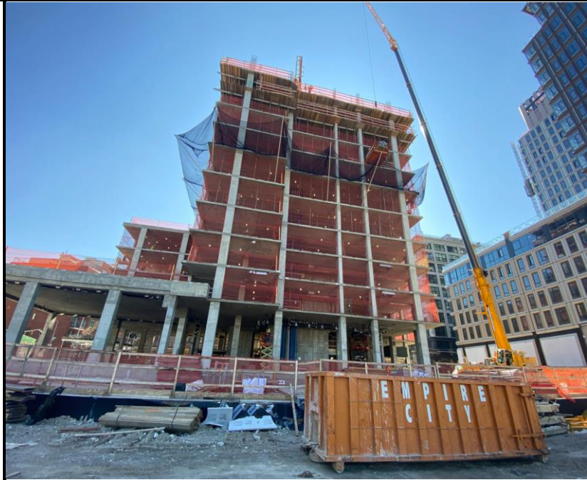
Photo 3: View of continued structure development.
