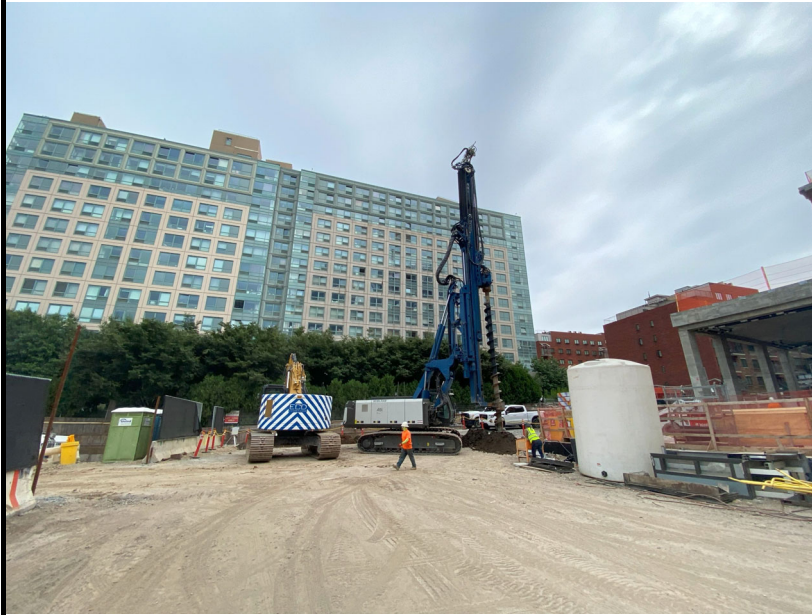
Photo 1: View of ECD continuing soldier pile installation.
