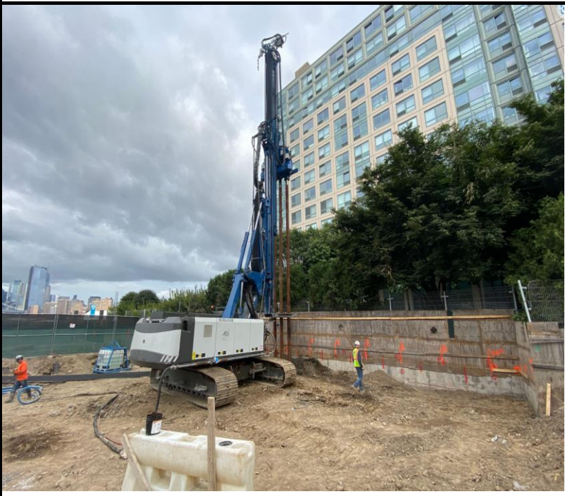
Photo 2: View of ECD completing pile installation.
