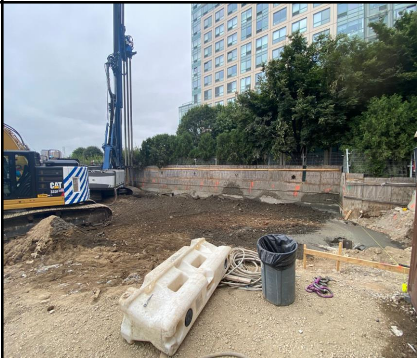
Photo 2: View of ECD completing pile installation.
