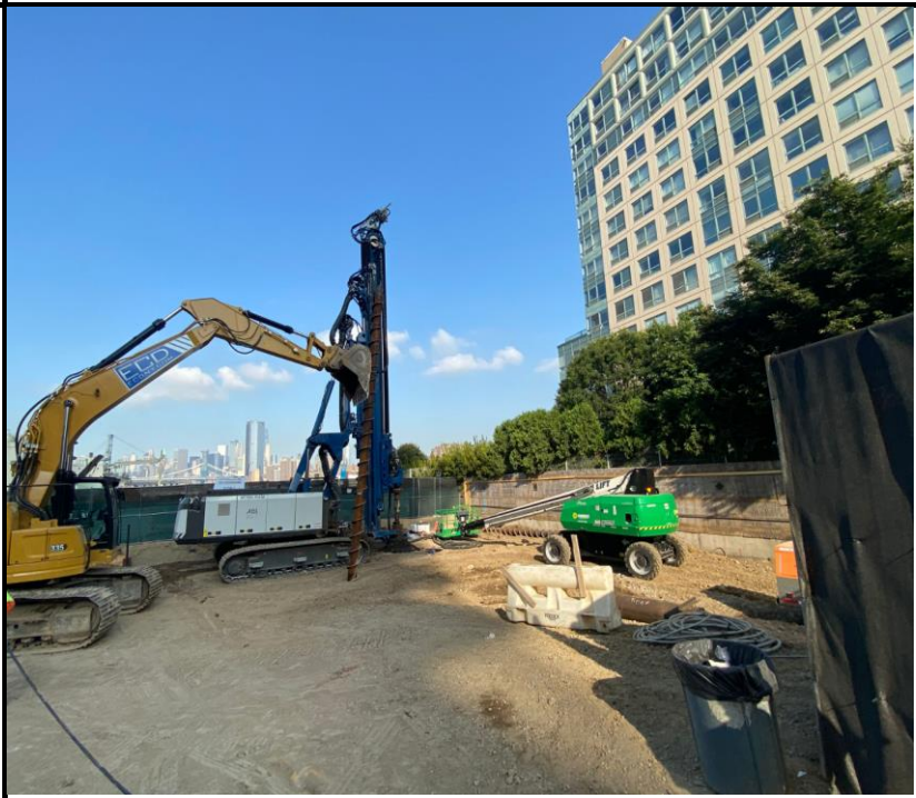
Photo 2: View of pile installation.
