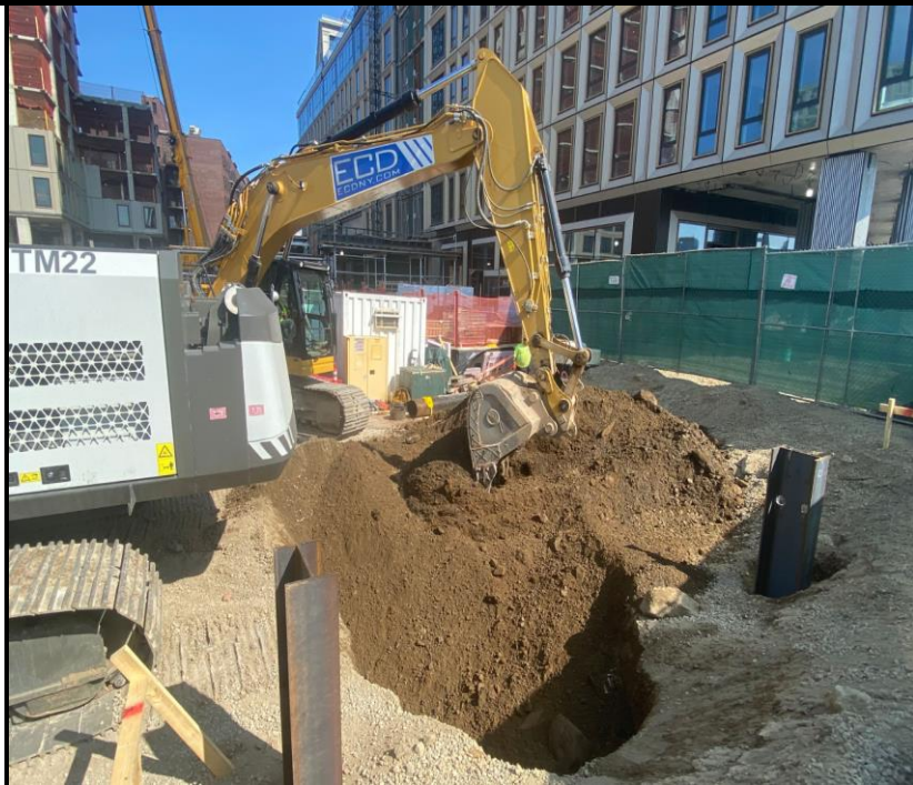
Photo 4: View of ECD completing excvaton and soldier pile installation.
