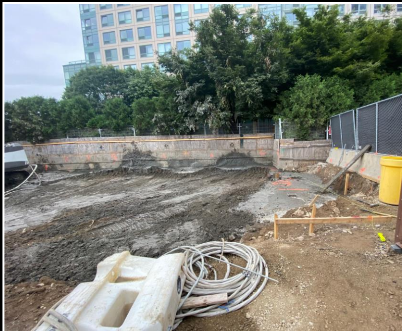
Photo 1: View of Site conditions and pile installation.
