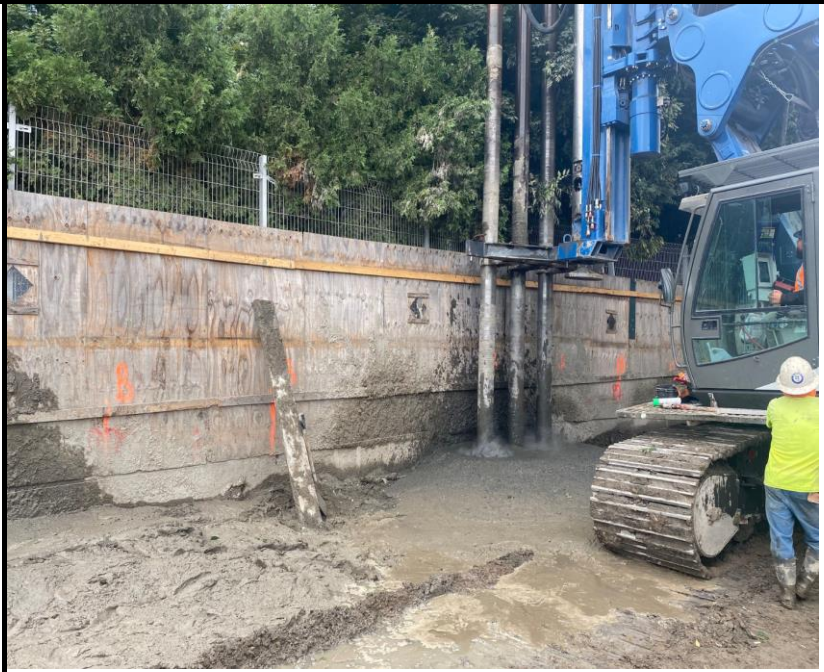
Photo 1: View of ECD completing pile installation.
