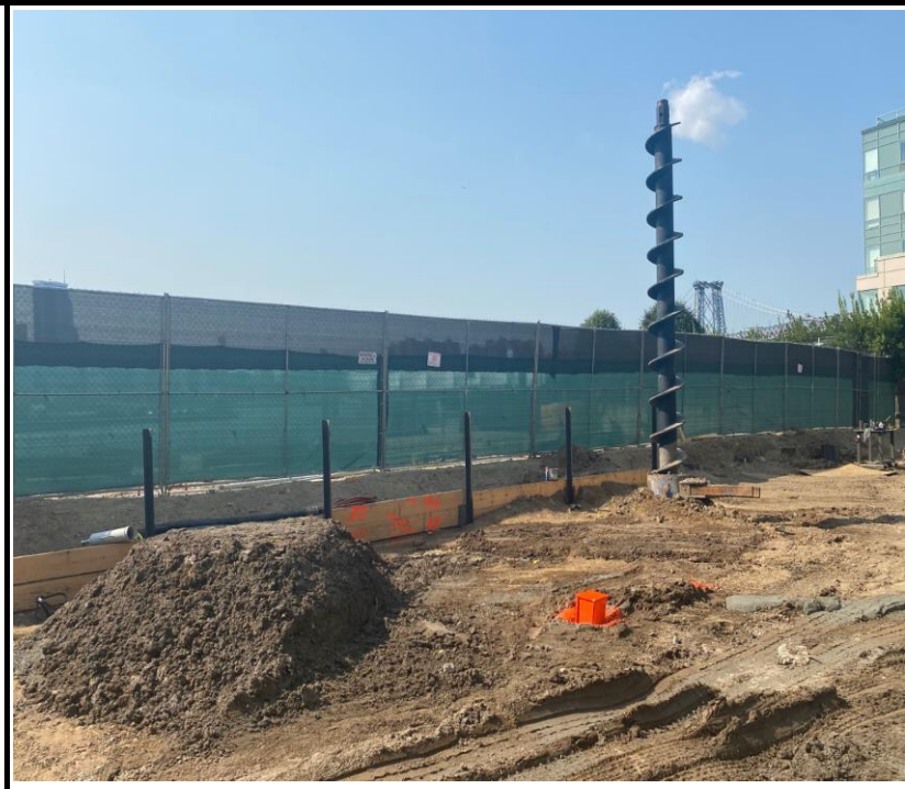
Photo 4: View of soil excavation for lagging installation.
