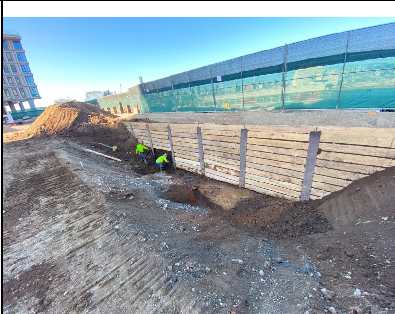
Photo 1: View of lagging installation for the SOE.
