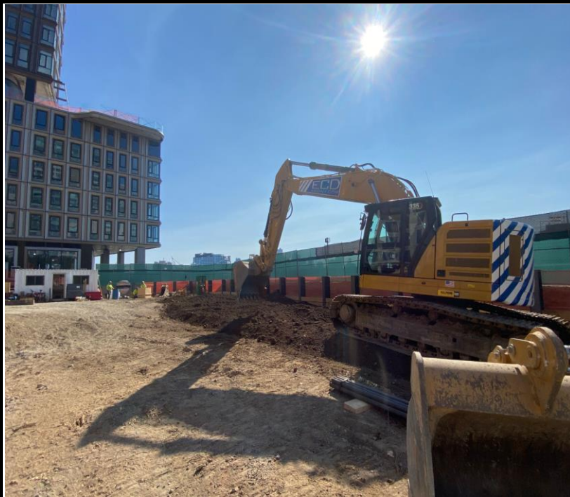
Photo 4: View of soil excavation for lagging installation.
