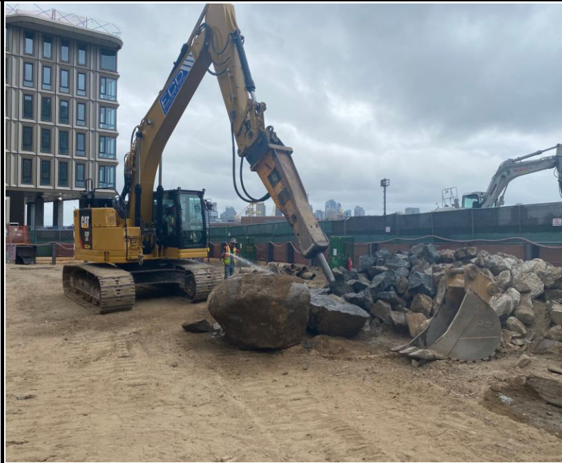
Photo 3: View of ECD hammering boulders and concrete from former building foundation.
