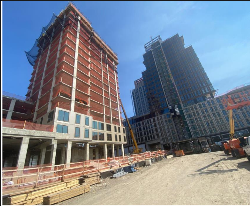
Photo 3: View of continued structural development.
