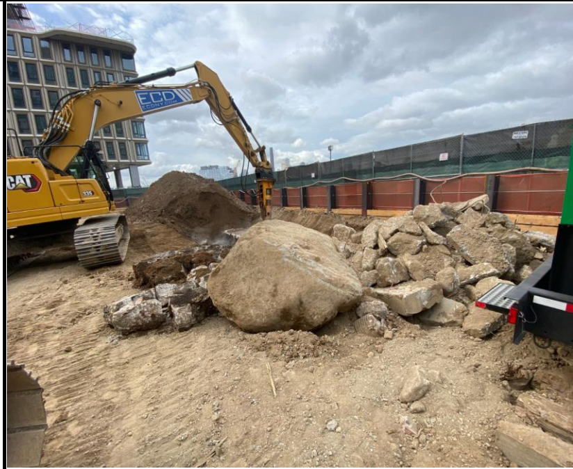
Photo 3: View of ECD breaking up boulders and concrete from former building foundation.
