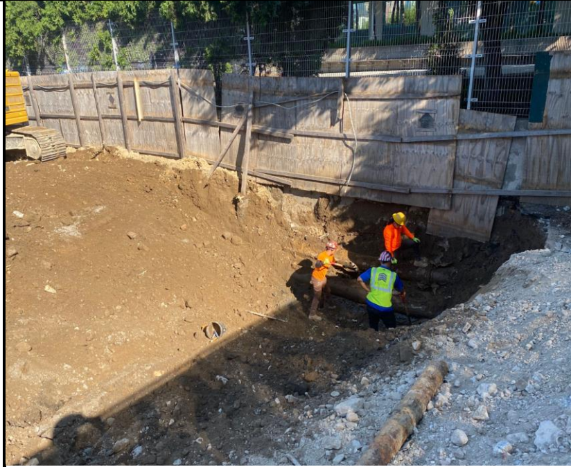
Photo 3: View of exposing pipes for testing.
