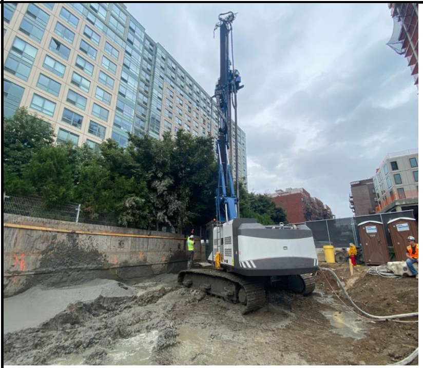
Photo 2: View of ECD completing pile installation.
