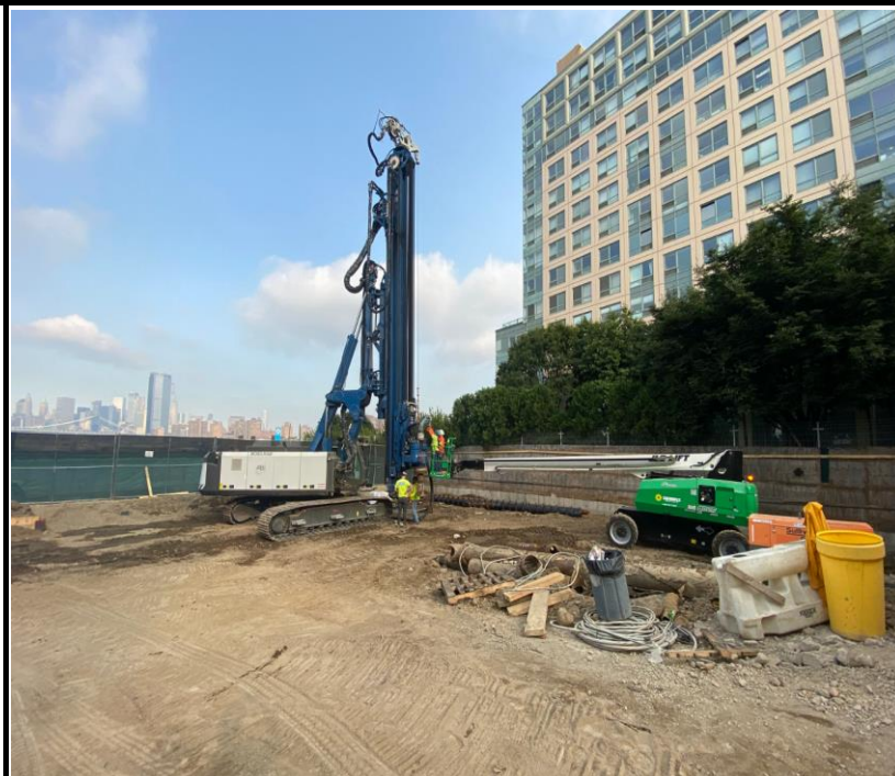
Photo 2: View of pile installation.
