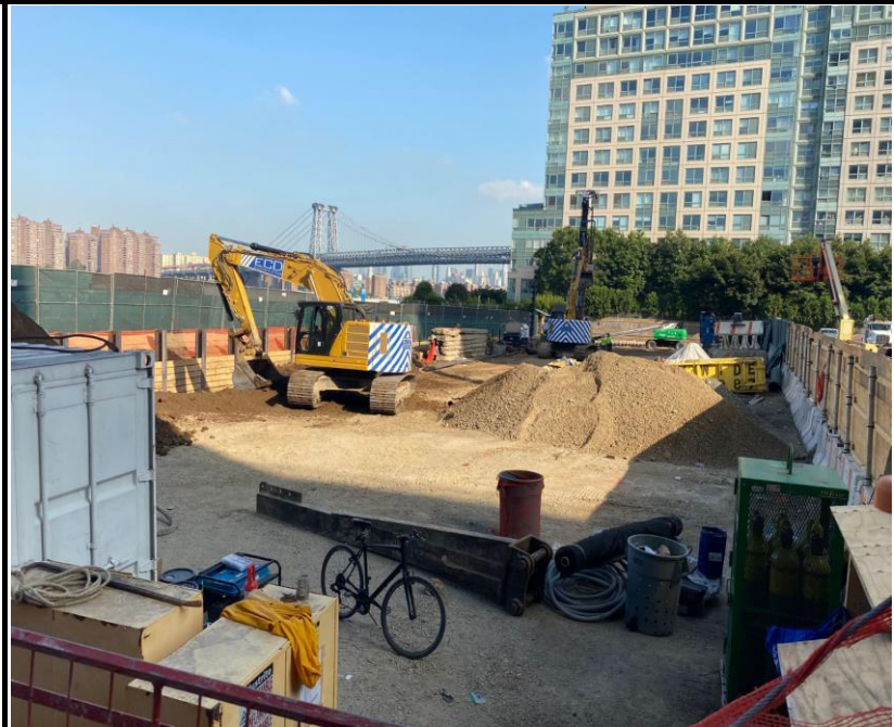
Photo 1: View of Site conditions and SOE installation.
