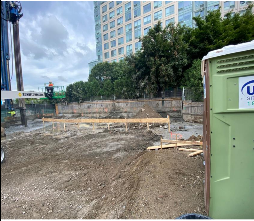
Photo 4: View of Site conditions during pile installation and grouting.
