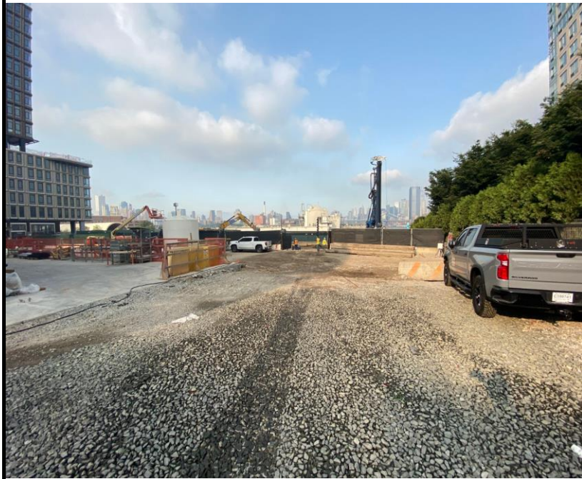
Photo 1: View of the Site facing west.
