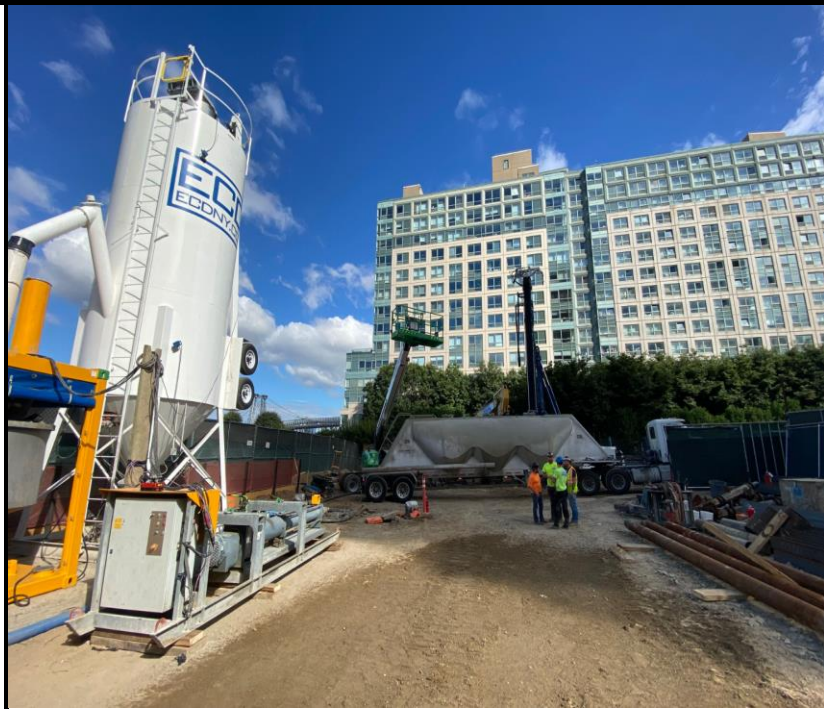
Photo 4: View of Site conditions and ECD equipment for grouting.
