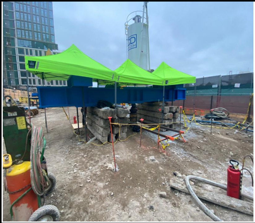
Photo 2: View of ECD completing load testing.
