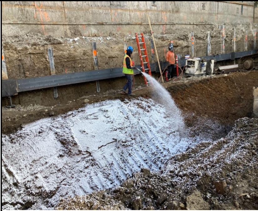
Photo 1: View of ECD spraying odor suppressing foam in the remedial excavation.
