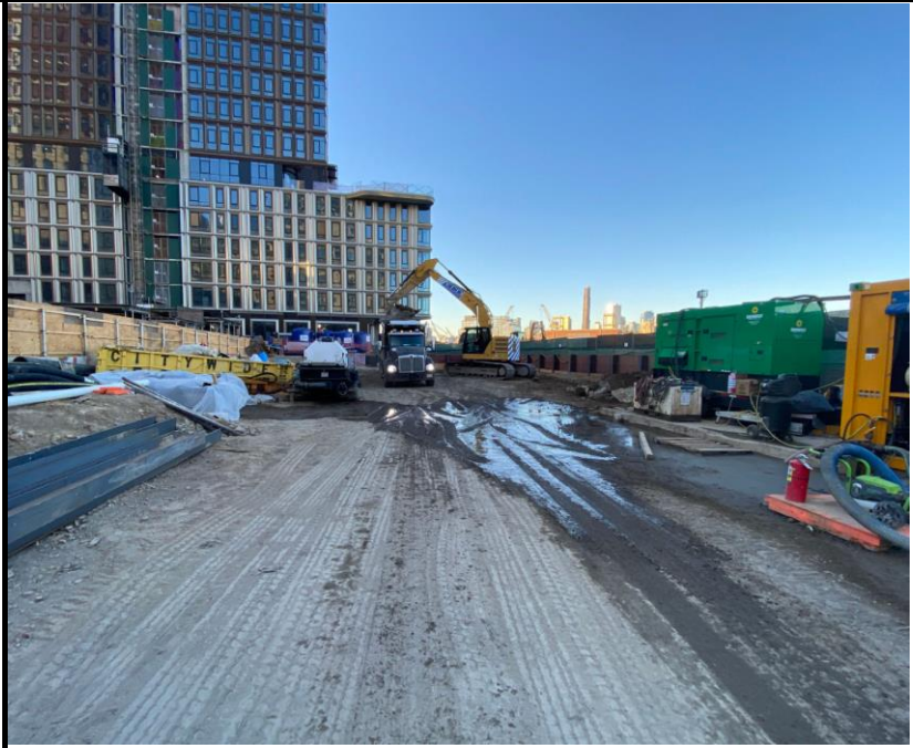
Photo 1: View of truck loading for off-site soil disposal.
