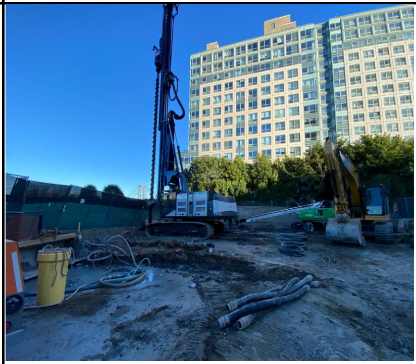
Photo 4: View of continued pile installation.
