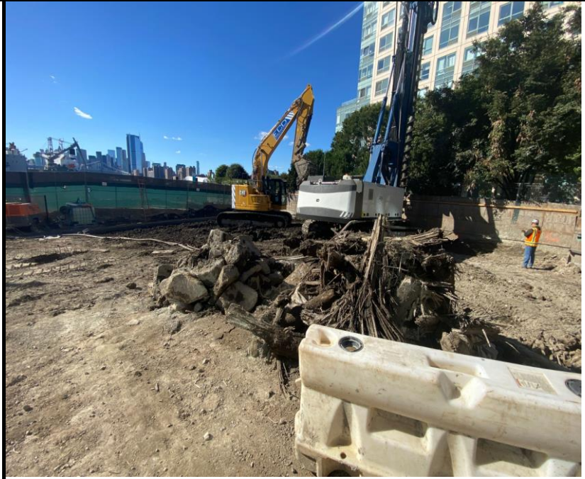
Photo 1: View of pile installation facing northwest.
