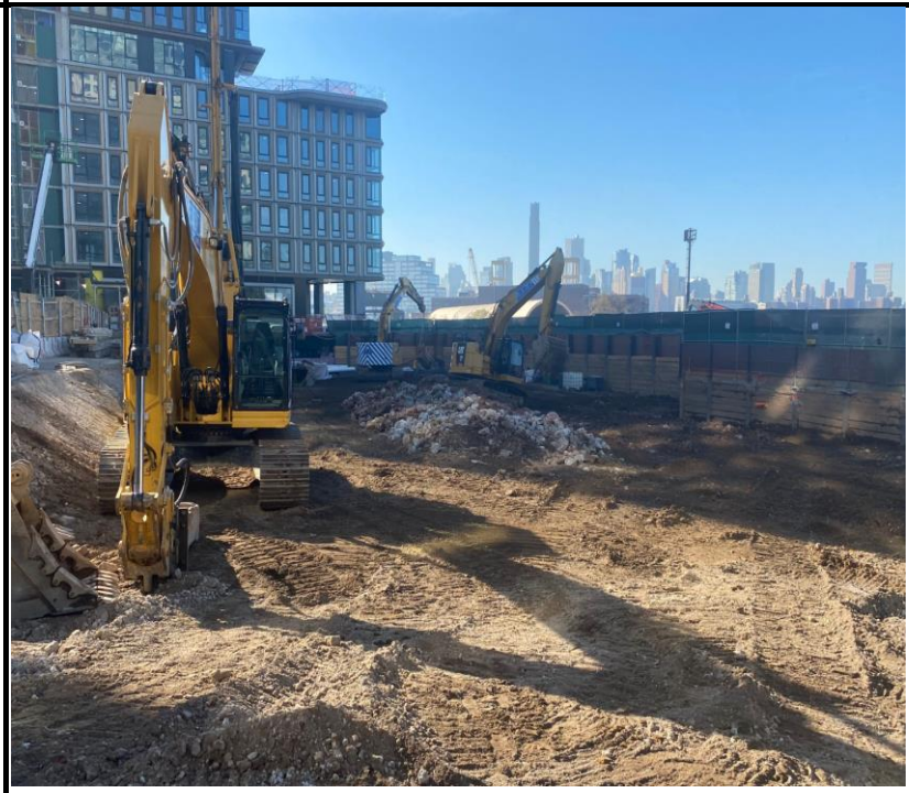
Photo 2: View of Site conditions and continued excavation and SOE installation.
