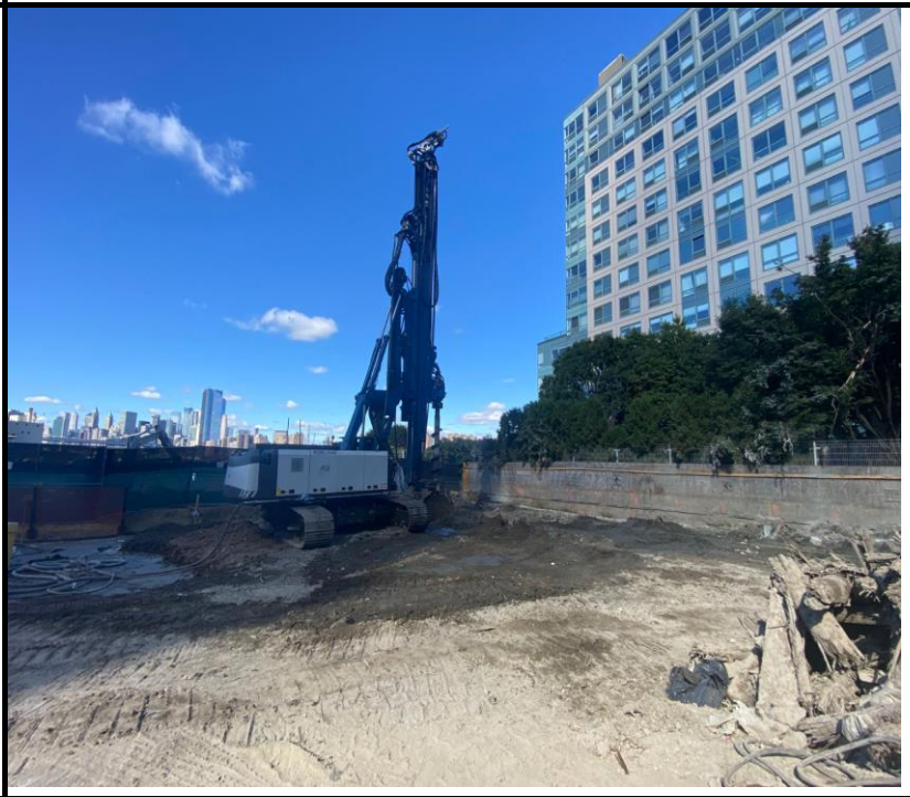
Photo 2: View of drilling for pile installation facing northwest.
