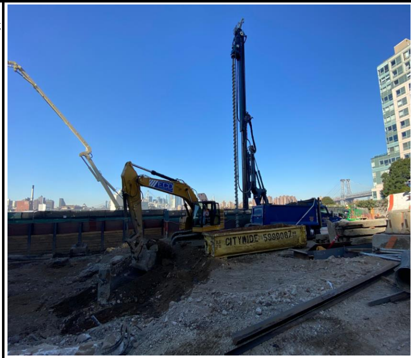
Photo 4: View of truck loading for off-site soil disposal
