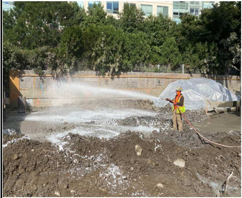
Photo 1: View of ECD spraying odor suppressing foam.
