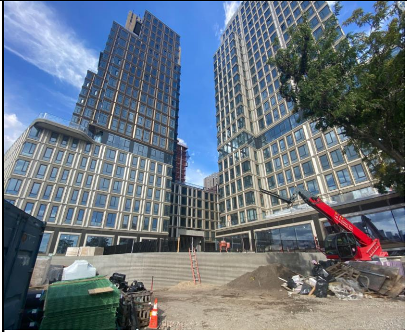
Photo 3: View of continued development of A1 and A3 structures.
