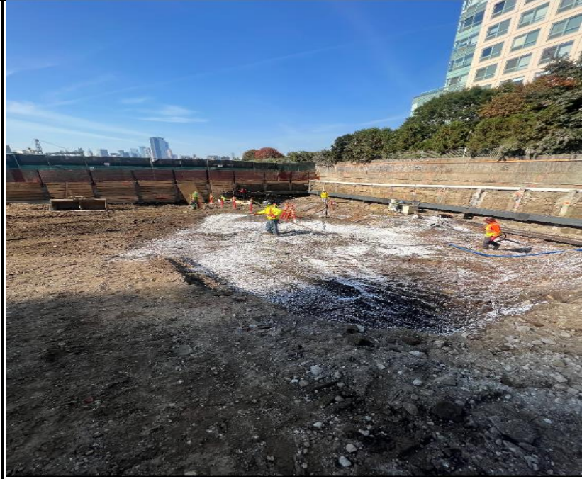
Photo 3: View of ECD spraying odor suppressing foam to continue excavation.
