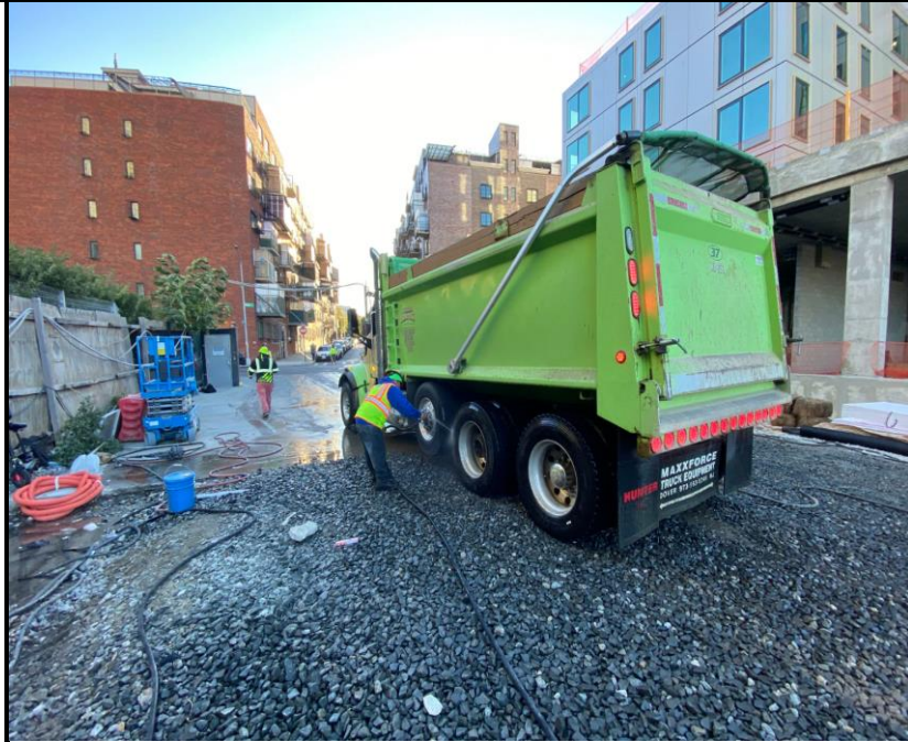
Photo 3: View of truck washing prior to leaving the Site.
