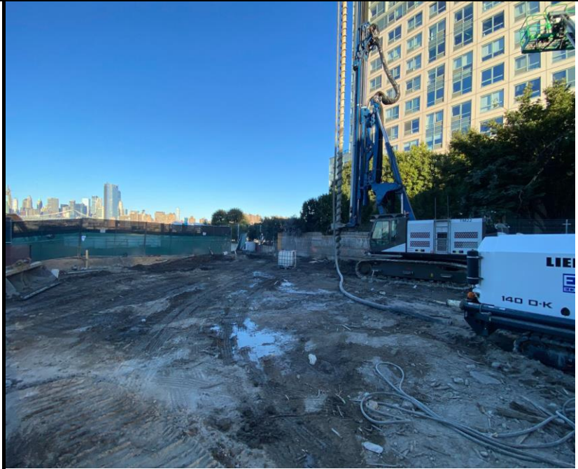
Photo 1: View of continuation of drilling and grout mix wall installation.
