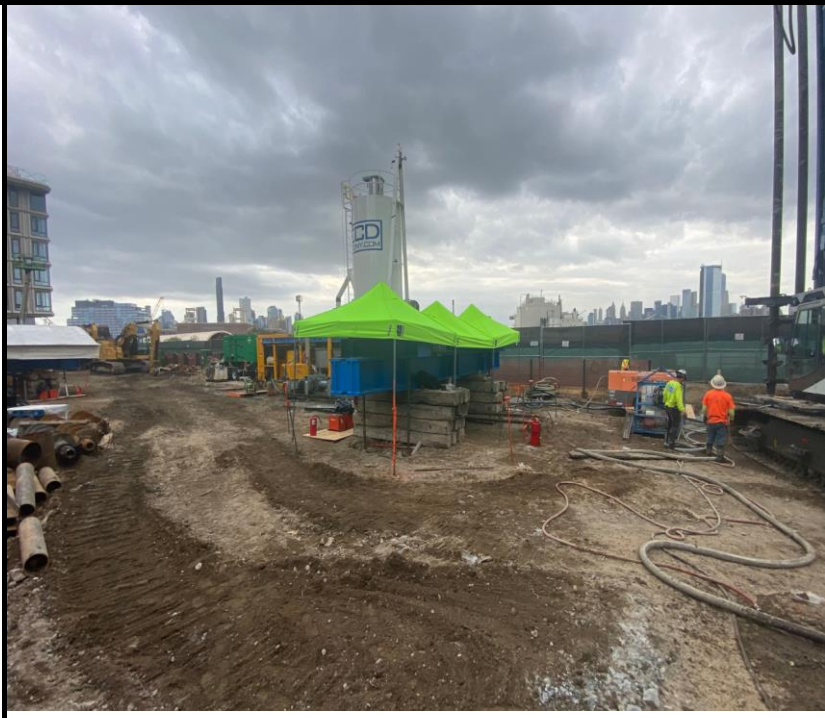
Photo 2: View of ECD completing 24-hour load testing.
