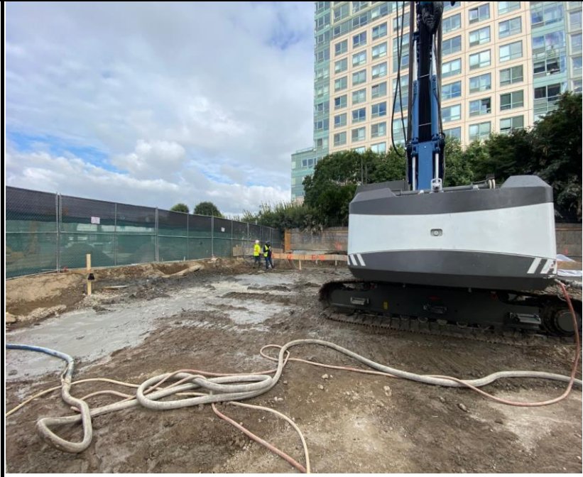
Photo 3: View of Site conditions and pile installation.
