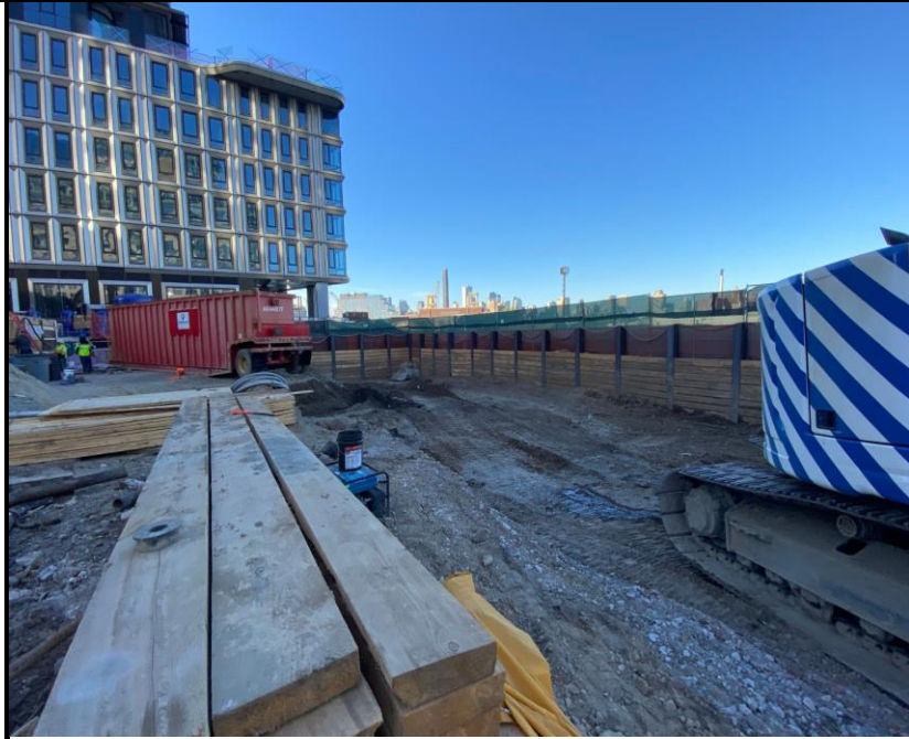
Photo 3: View of lagging installation for SOE.
