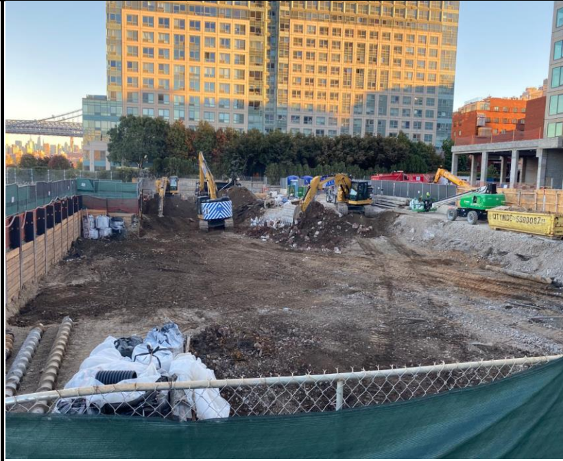
Photo 3: View of site conditions and soil excavation facing north.
