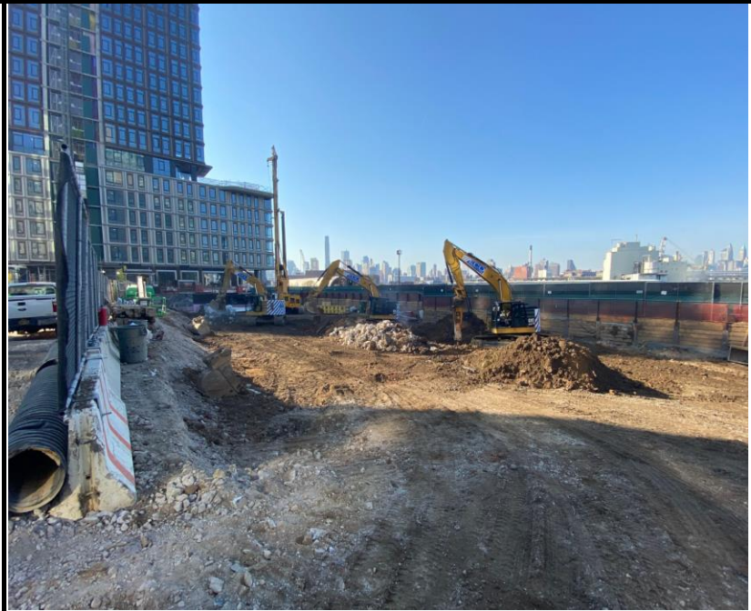
Photo 1: View of Site conditions, excavation and concrete demolition.
