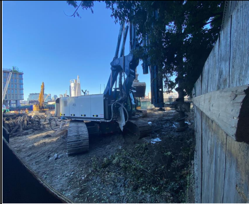
Photo 3: View of pile installaton along the northern perimiter of the Site.
