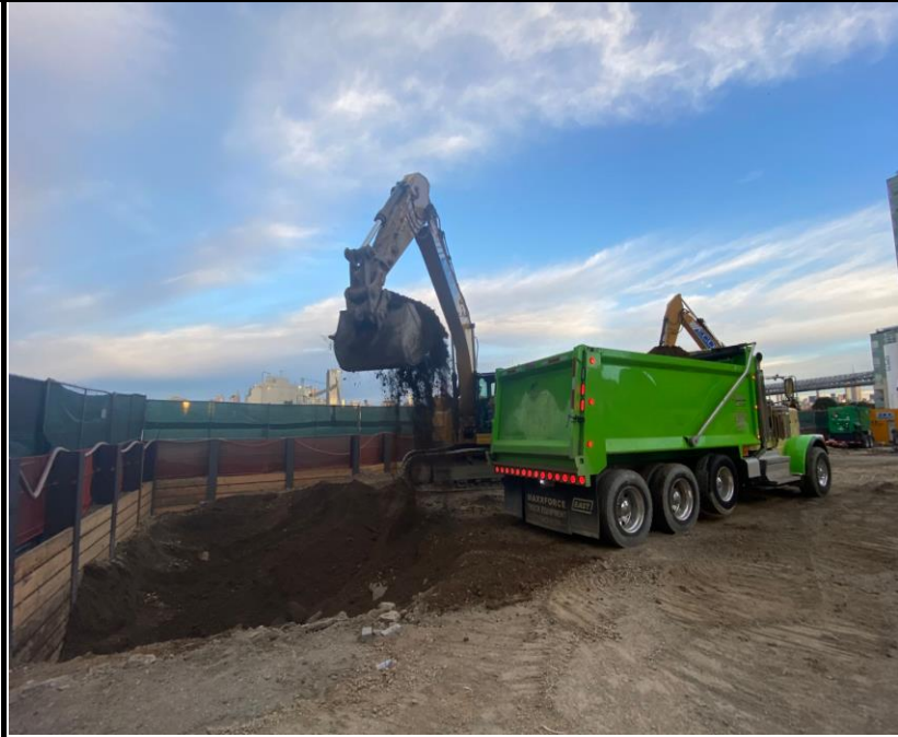
Photo 3: View of soil excavation and truck loading for off-site disposal.
