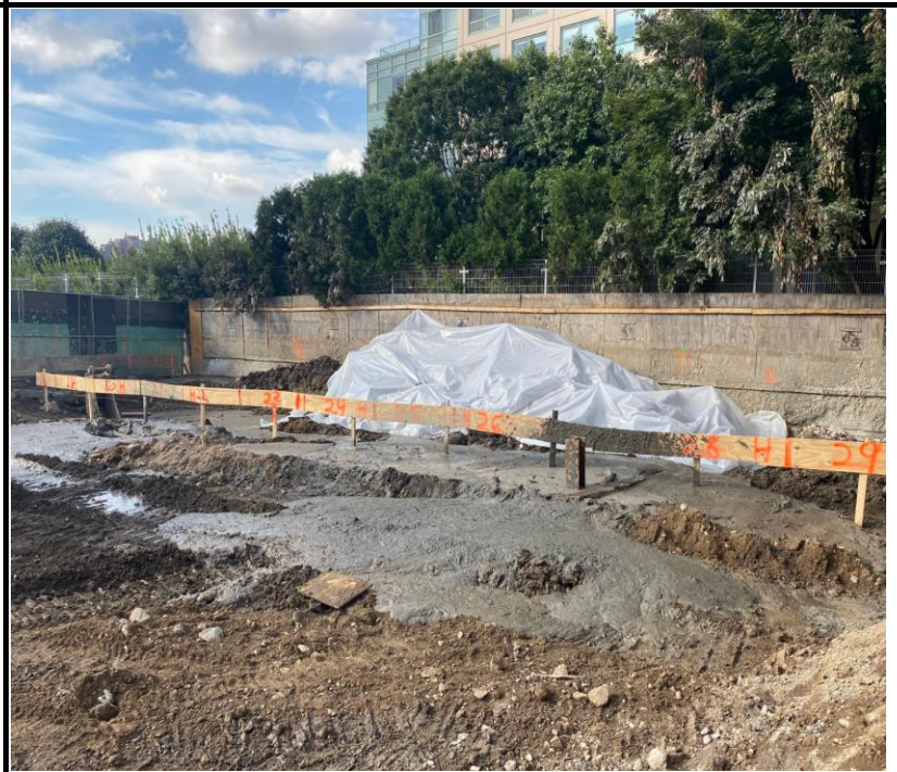
Photo 2: View of covered remedial excavation at the end of the workday.
