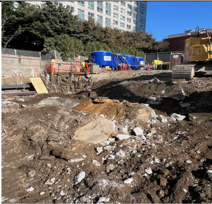
Photo 2: View of the tanks prior to removal.
