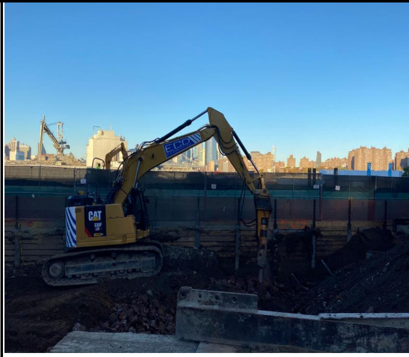
Photo 4: View of hammering former foundation elements.
