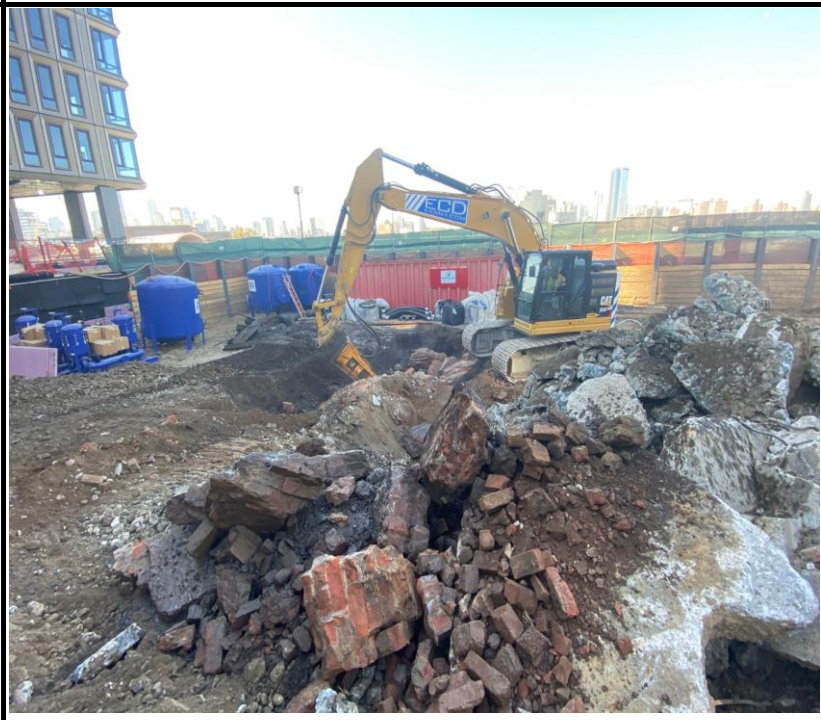
Photo 4: View of demolition of former foundations below grade.
