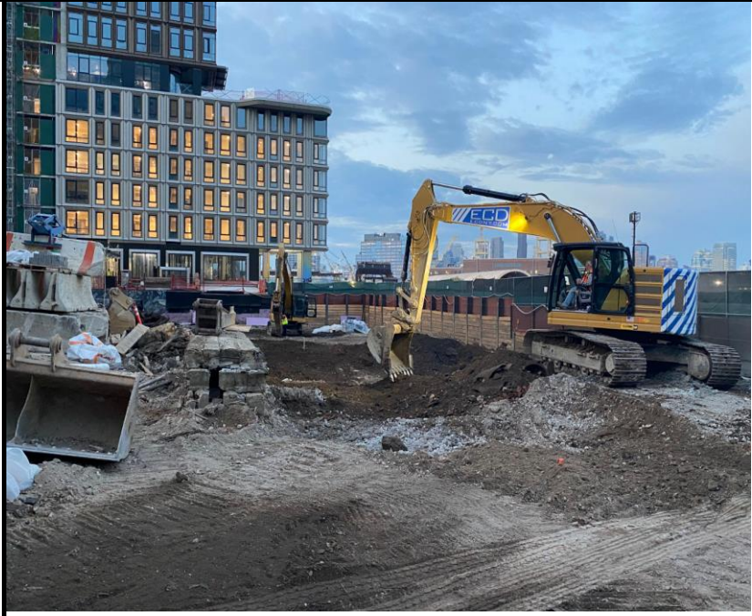
Photo 1: View of soil excavation and site conditions facing south.
