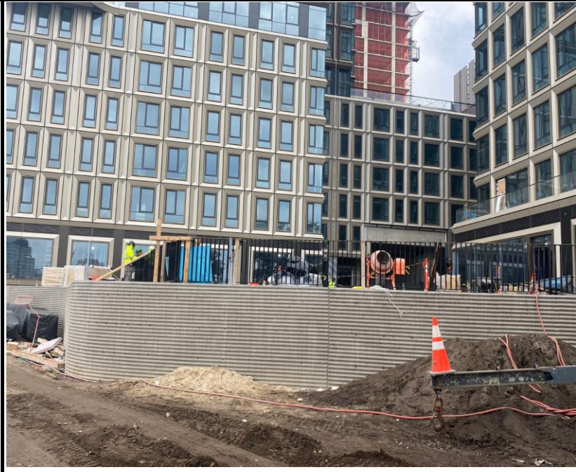
Photo 3: View of continued patio development.
