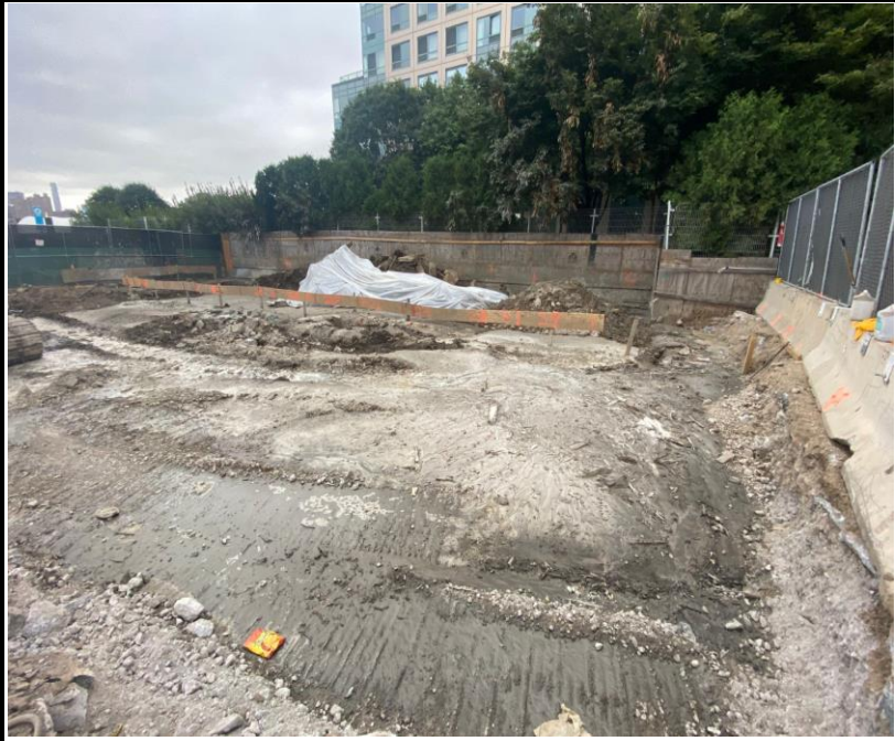
Photo 3: View of Site conditions facing northwest.
