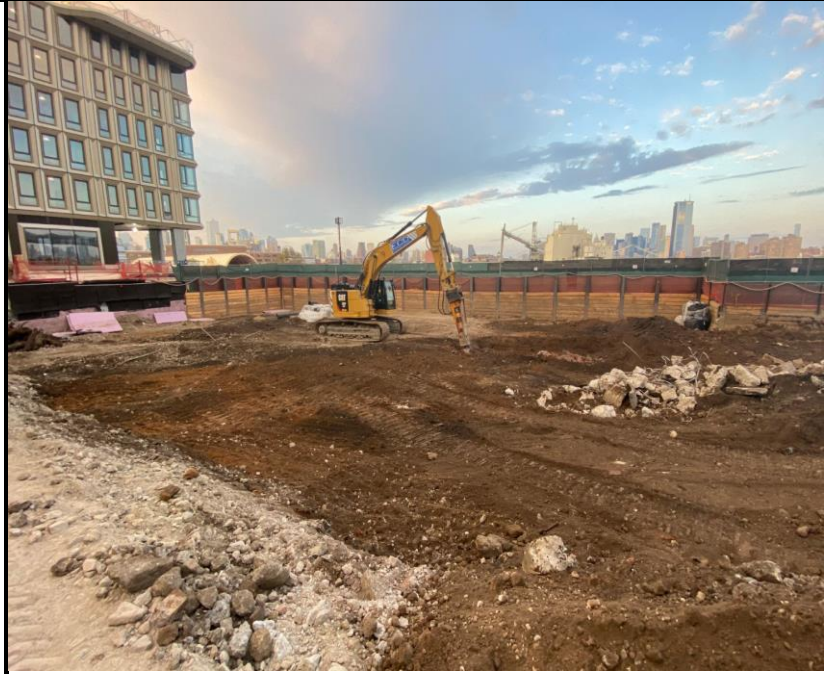
Photo 3: View of hammering former foundation elements.
