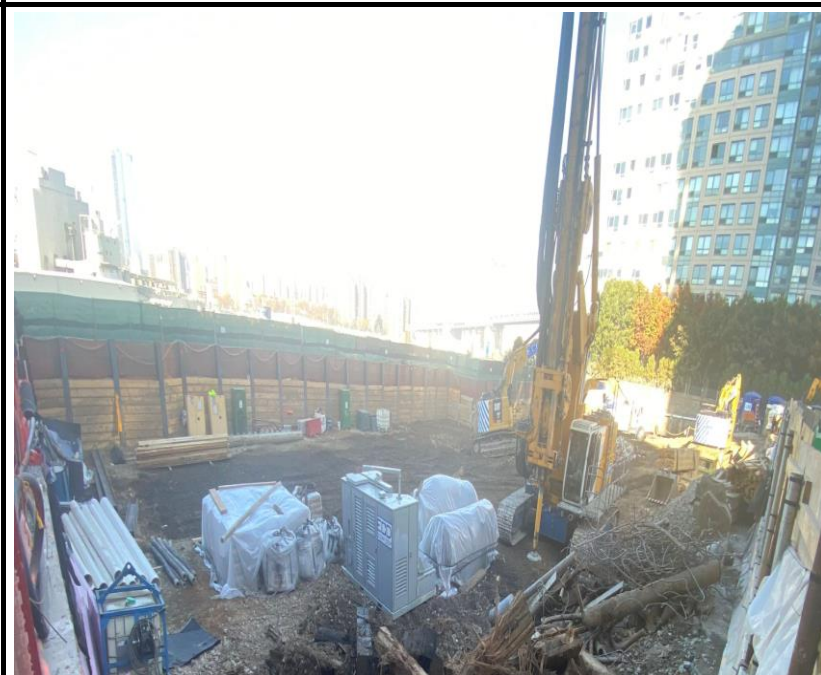
Photo 4: View of Site conditions and tanks contained in poly sheeting.
