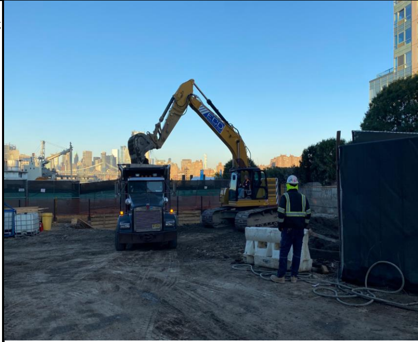
Photo 3: View of truck loading for off-site soil disposal.
