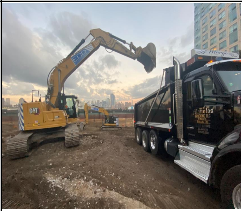
Photo 2: View of truck loading for off-site soil disposal.
