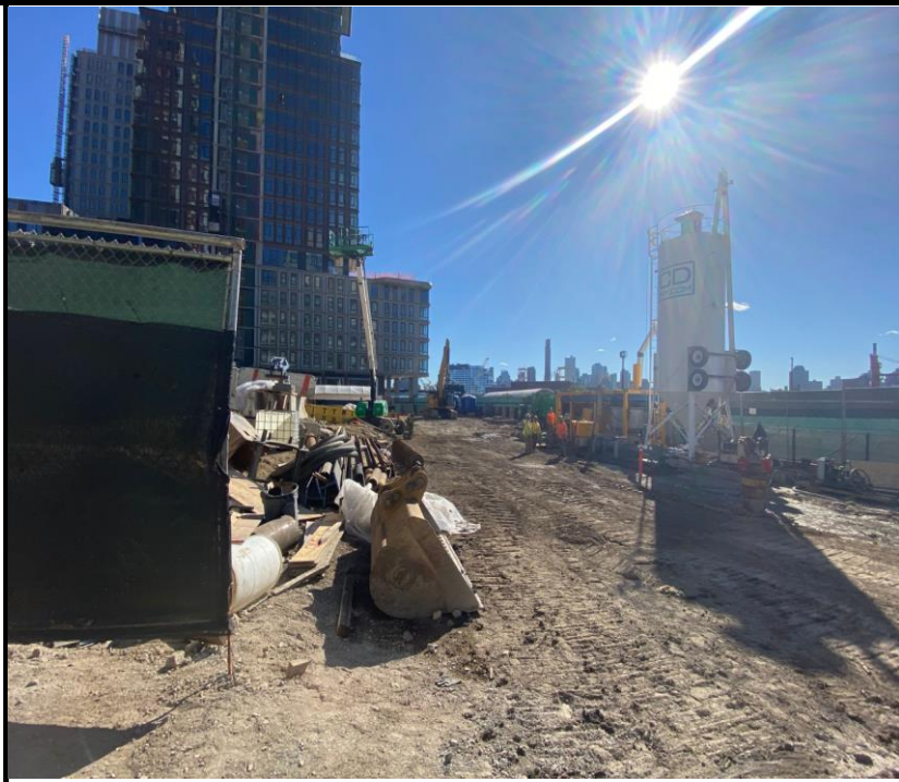
Photo 2: View of Site conditions facing southwest.
