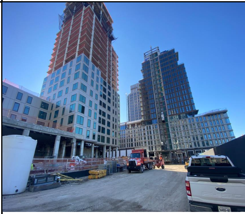
Photo 4: View of continued development of A1, A2 and A3 buildings.
