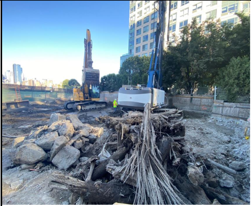
Photo 1: View of site conditions and pile installation facing northwest.
