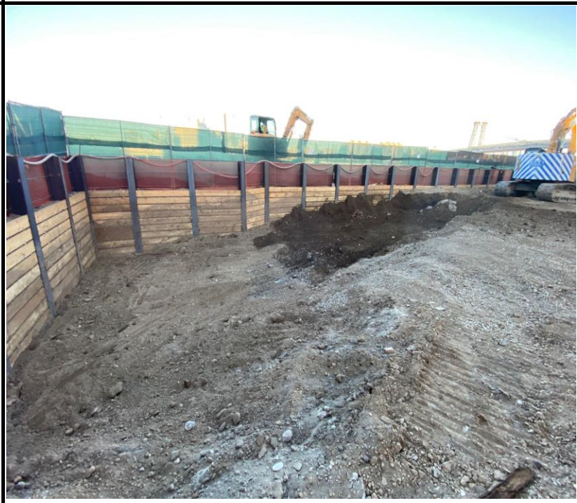
Photo 2: View of soil excavation.
