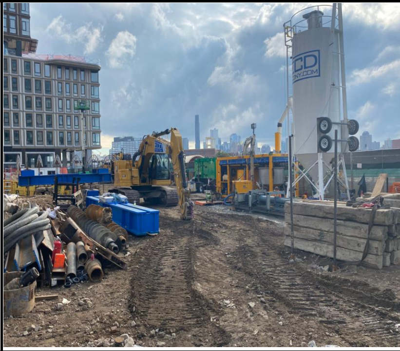
Photo 4: View of Site conditions facing southwest.
