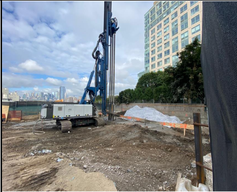
Photo 1: View of pile installation.
