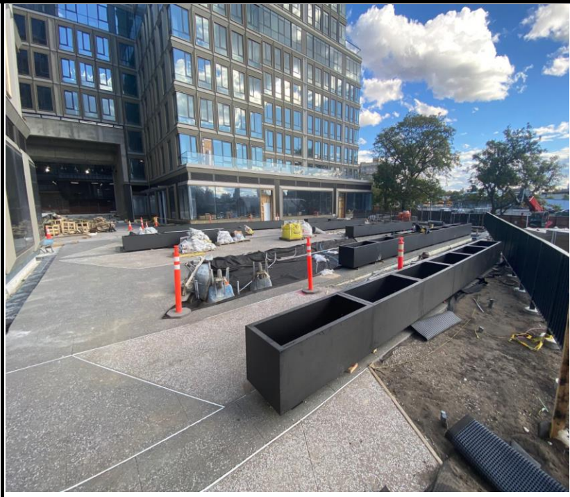
Photo 4: View of continued patio development.
