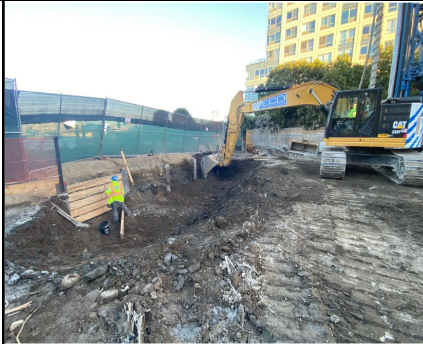
Photo 3: View of lagging installation for SOE.
