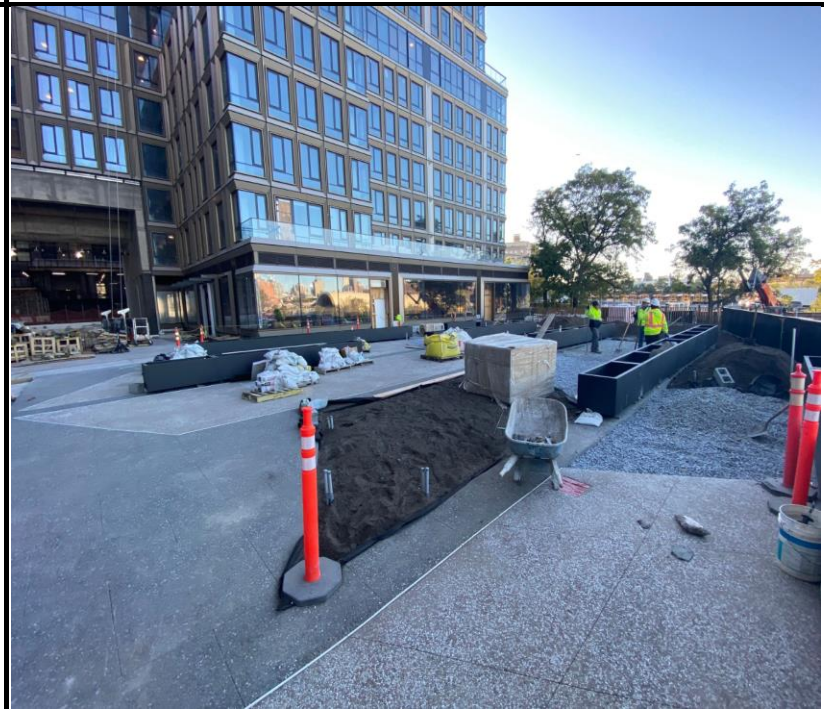
Photo 4: View of continued patio development.
