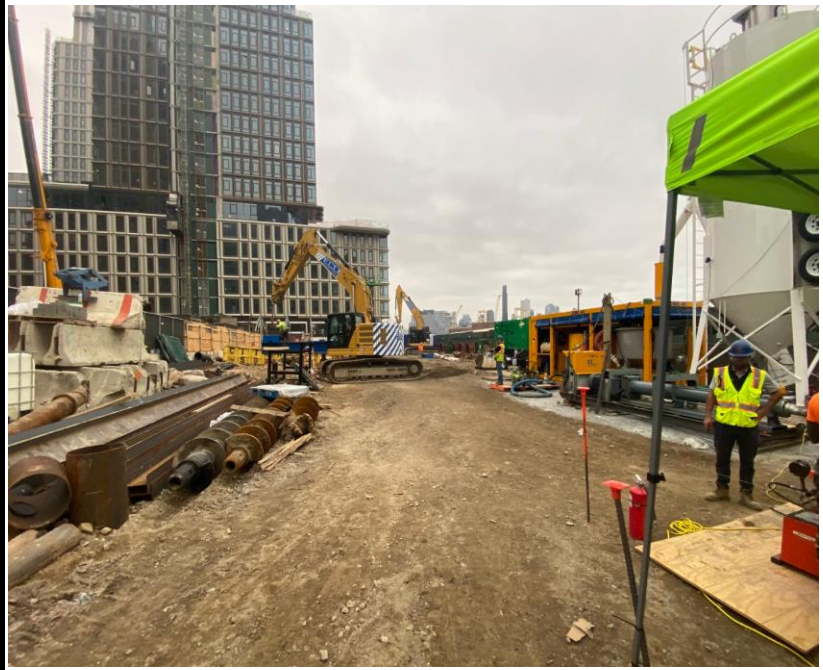
Photo 1: View of site conditions facing southwest.
