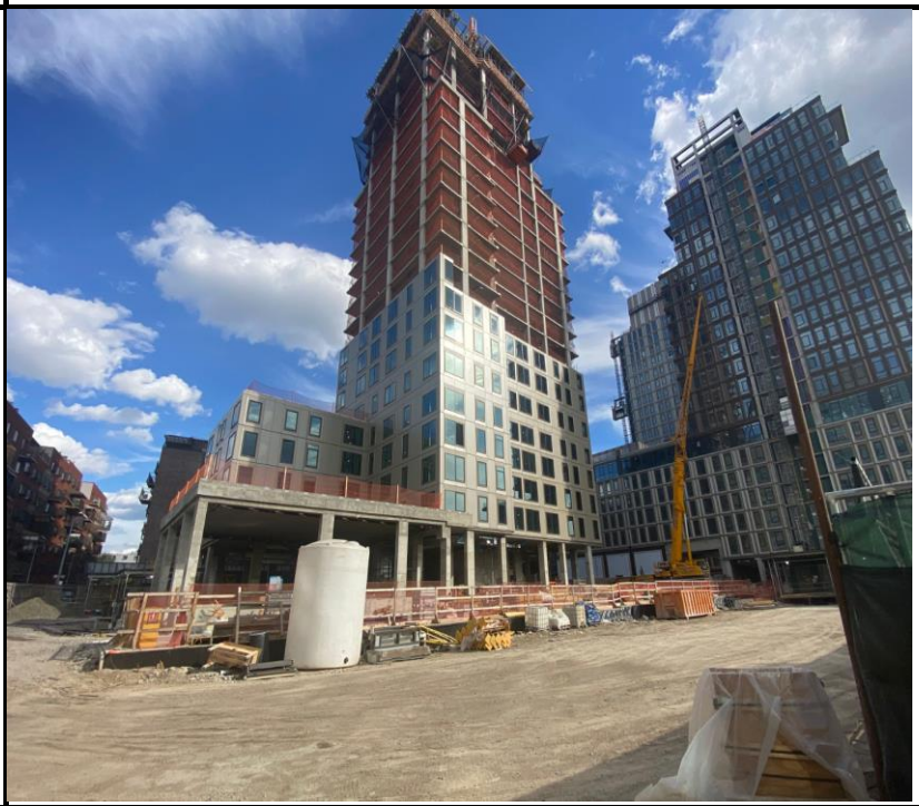
Photo 2: View of continued development of A3 building.
