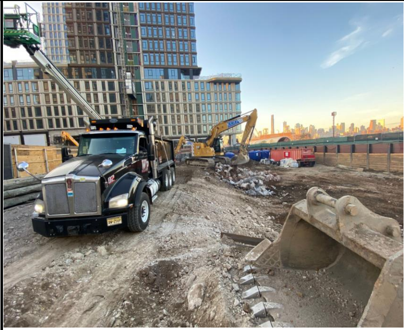
Photo 3: View of truck loading for off-site concrete disposal.
