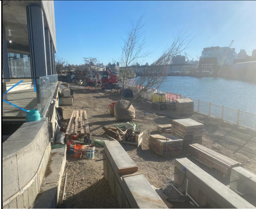
Photo 3: View of landscaping and site conditions in the marine front.
