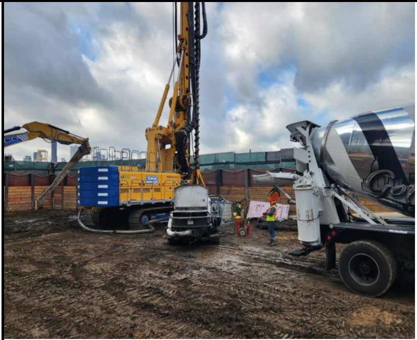
Photo 1: View of ECD completing pile installation.
