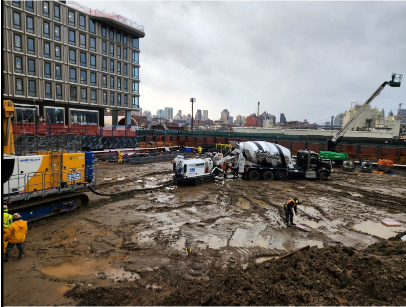
Photo 1: View of Site conditions and activities, facing southeast.
