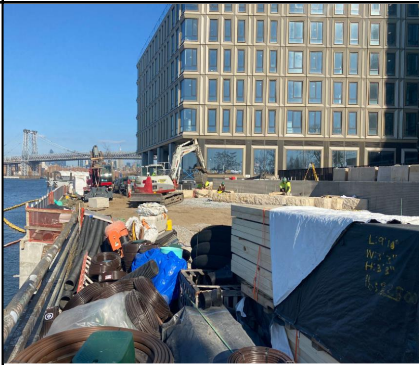
Photo 2: View of Site conditions in the marine front facing north.
