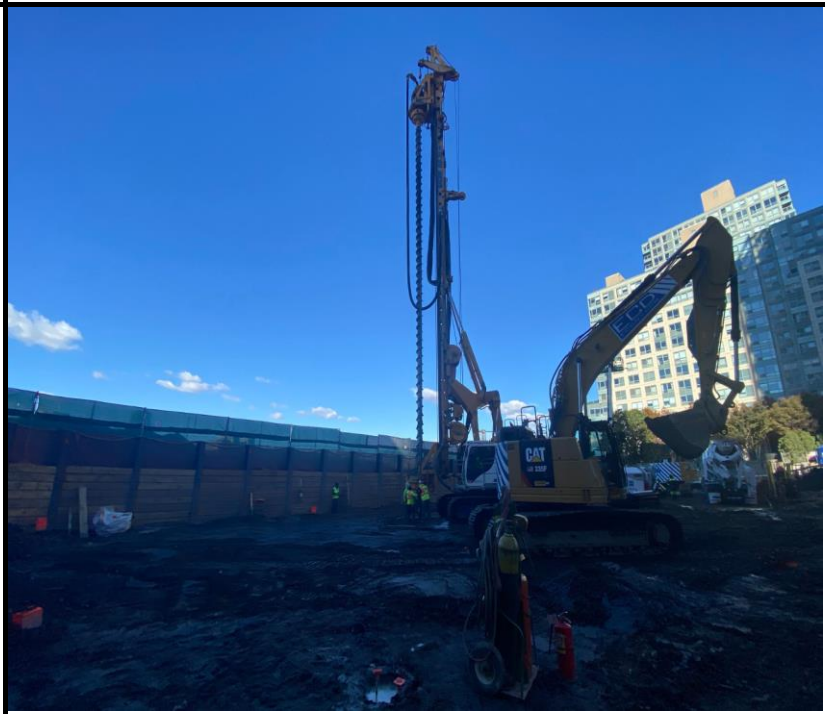
Photo 2: View of pile installation.
