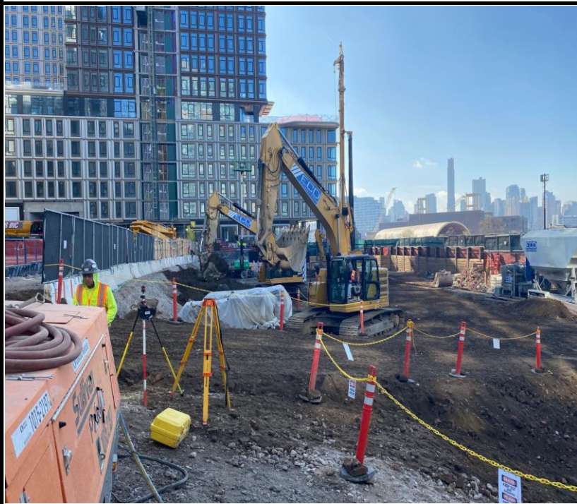
Photo 2: View of Site conditions facing south.
