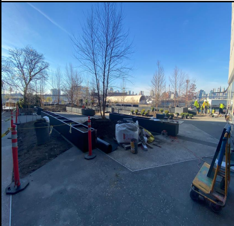
Photo 2: View of the continued landscaping and patio work along the marine front.
