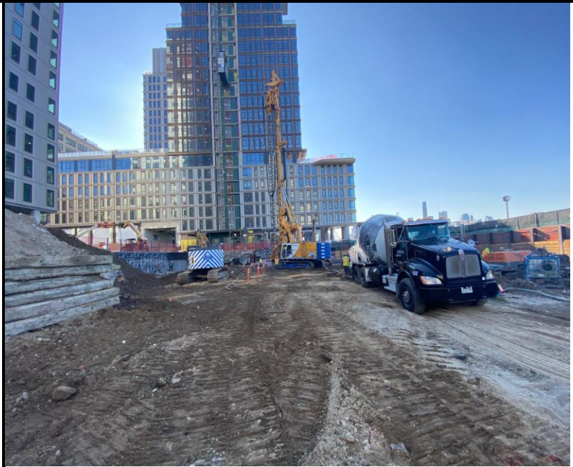
Photo 1: View of drilling activities facing south.
