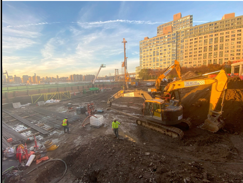
Photo 1: View of Site conditions and activities, facing northwest.
