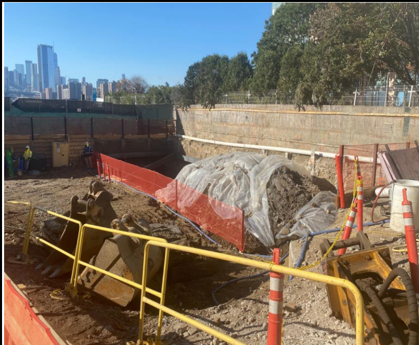
Photo 3: View of the northern remedial excavation.
