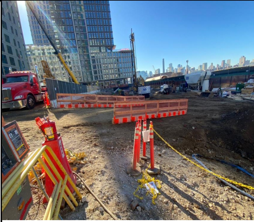
Photo 4: View of Site conditions facing south.
