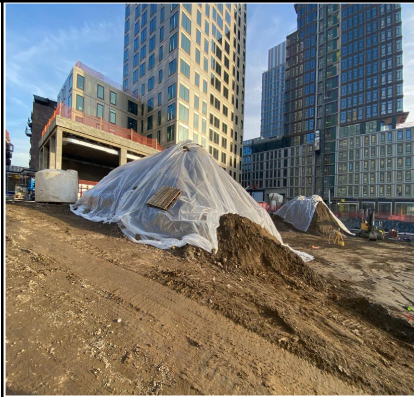
Photo 4: View of soil stockpiled in preparation for off- site disposal.
