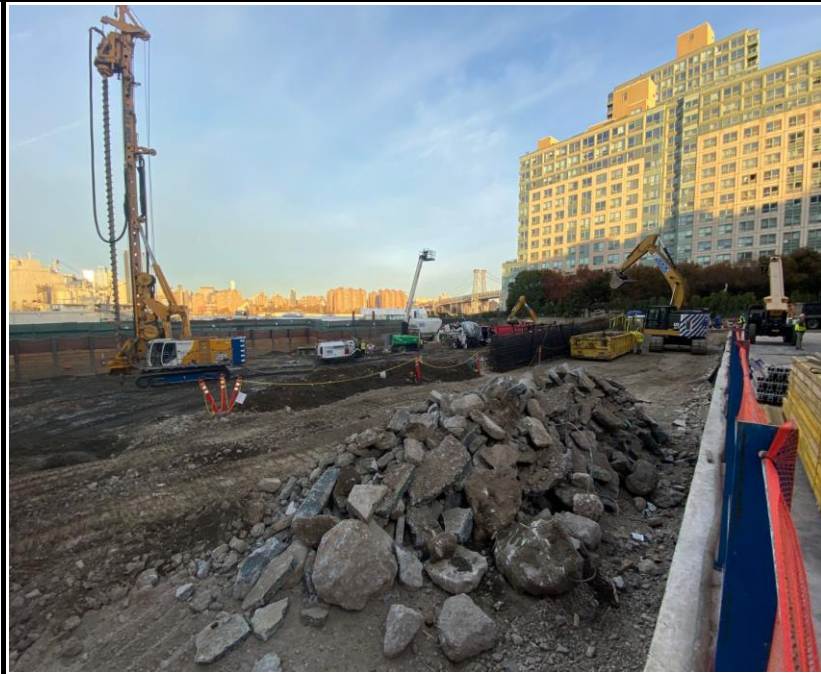
Photo 3: View of Site conditions and pile installation facing northwest.
