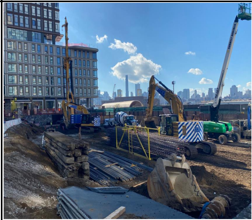
Photo 2: View of Site conditions facing southwest.
