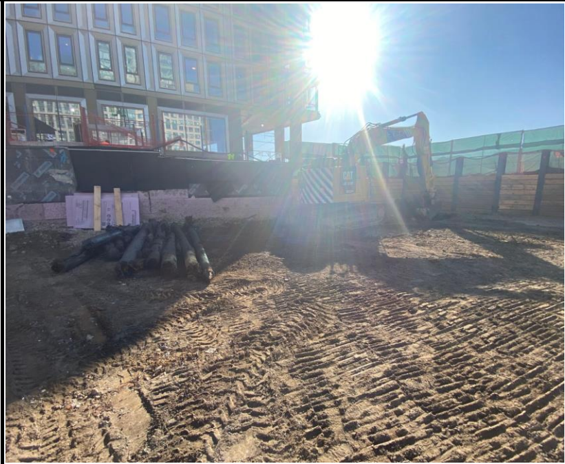
Photo 3: View of excavation facing southwest.
