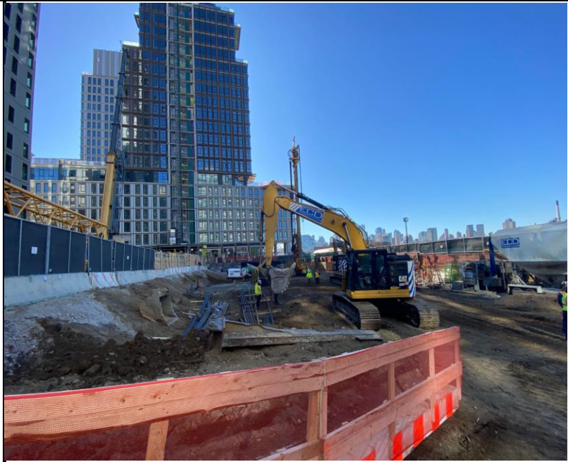
Photo 3: View of Site conditions facing south.
