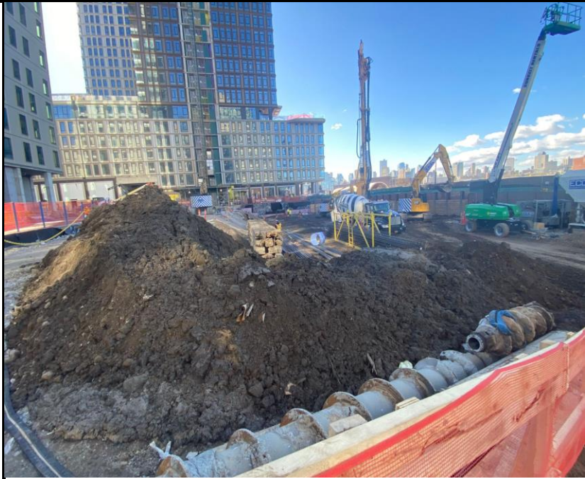
Photo 1: View of Site conditions facing southwest.
