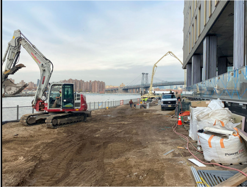
Photo 1: View of Site conditions and activities, facing north.
