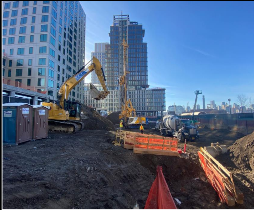
Photo 1: View of Site conditions facing south.
