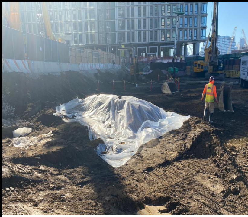
Photo 4: View of sand from tanks covered in poly in preparation for off- site disposal.
