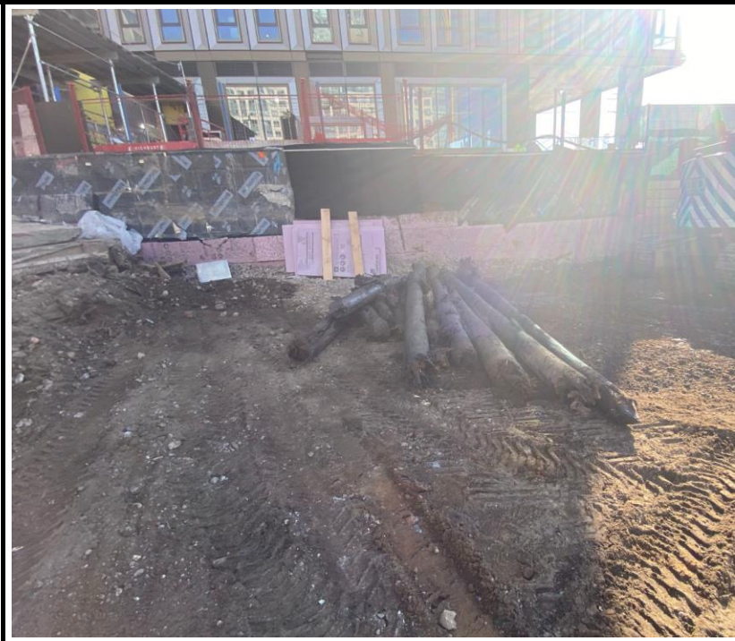
Photo 4: View of wood piles removed from excavation stockpiled for off-site disposal.
