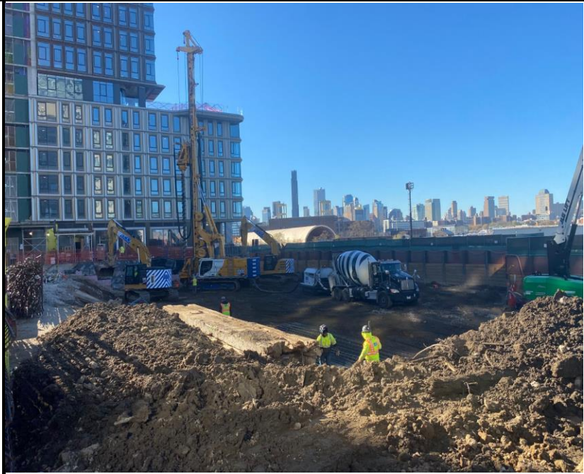
Photo 1: View of Site conditions facing southwest.
