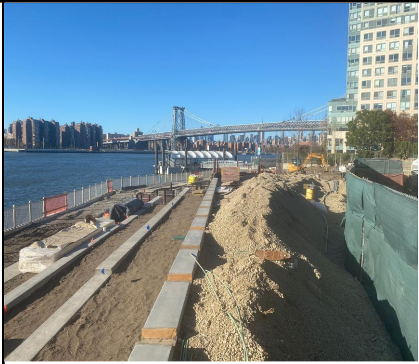
Photo 4: View of Site conditions in the marine front facing north.
