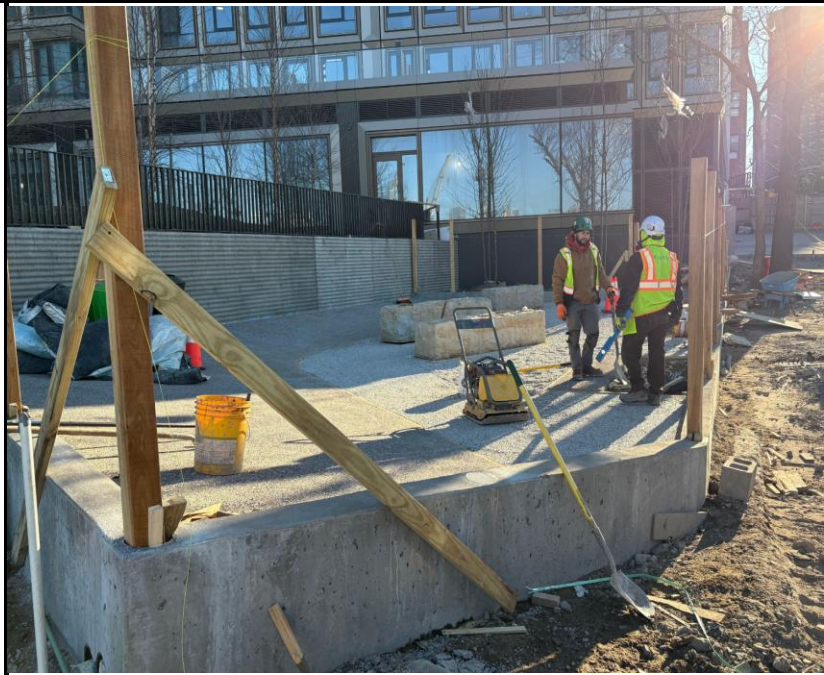
Photo 3: View of the continued marine front development.
