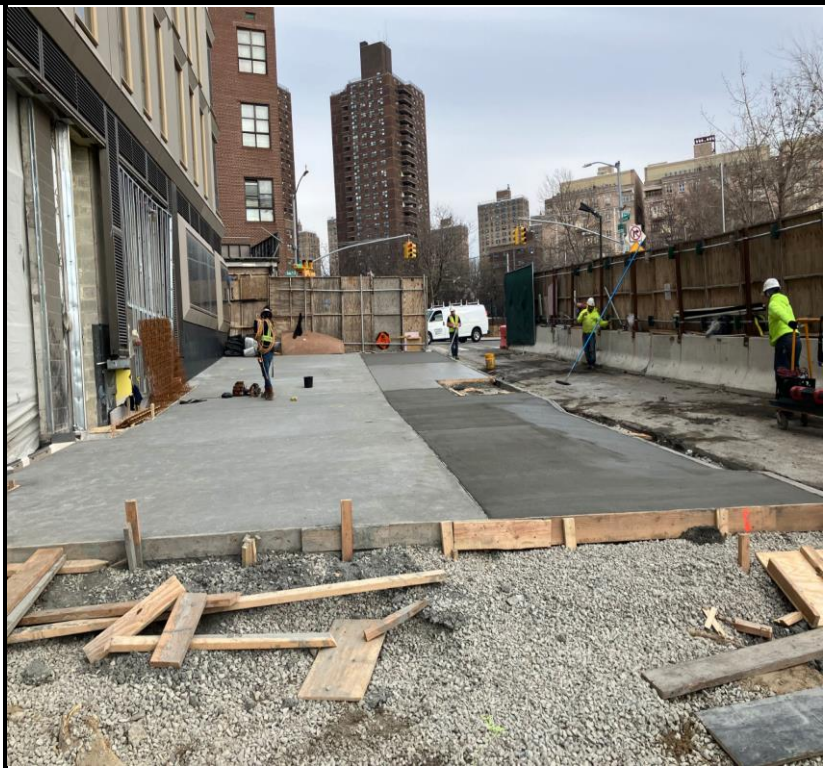
Photo 2: View of sidewalk development for building A1 along Division Avenue.
