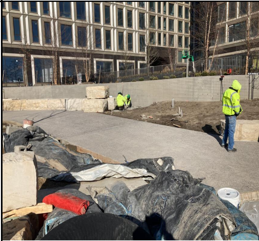
Photo 2: View of continued landscaping development facing east.
