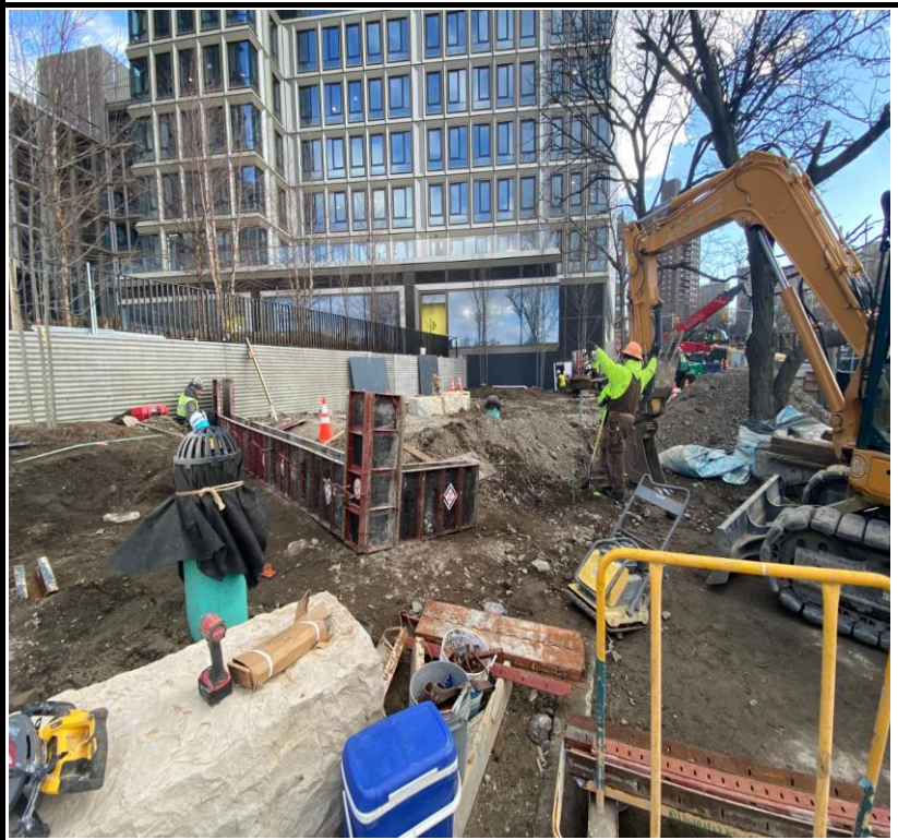
Photo 2: View of continued landscaping development facing east.
