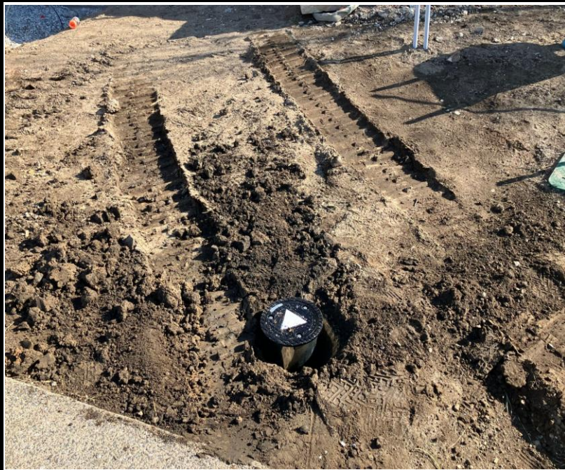
Photo 1: View of monitoring well installation.
