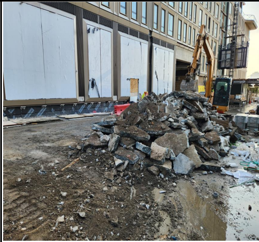
Photo 4: View of concrete removal between buildings A2 and A3.
