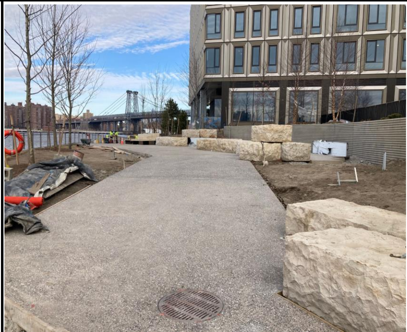
Photo 1: View of the landscaping development facing north.
