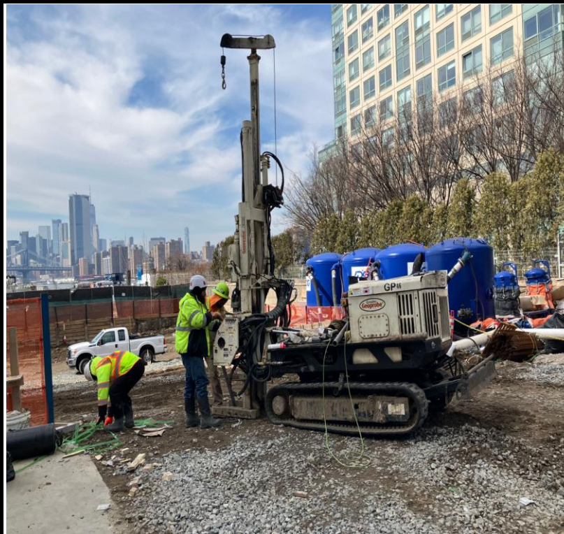
Photo 2: View of soil boring advancement for soil characterization of future utility trench.
