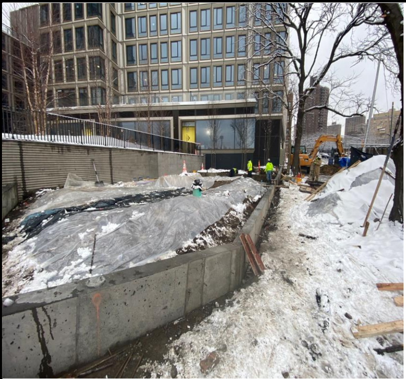
Photo 2: View of continued landscaping development facing east.
