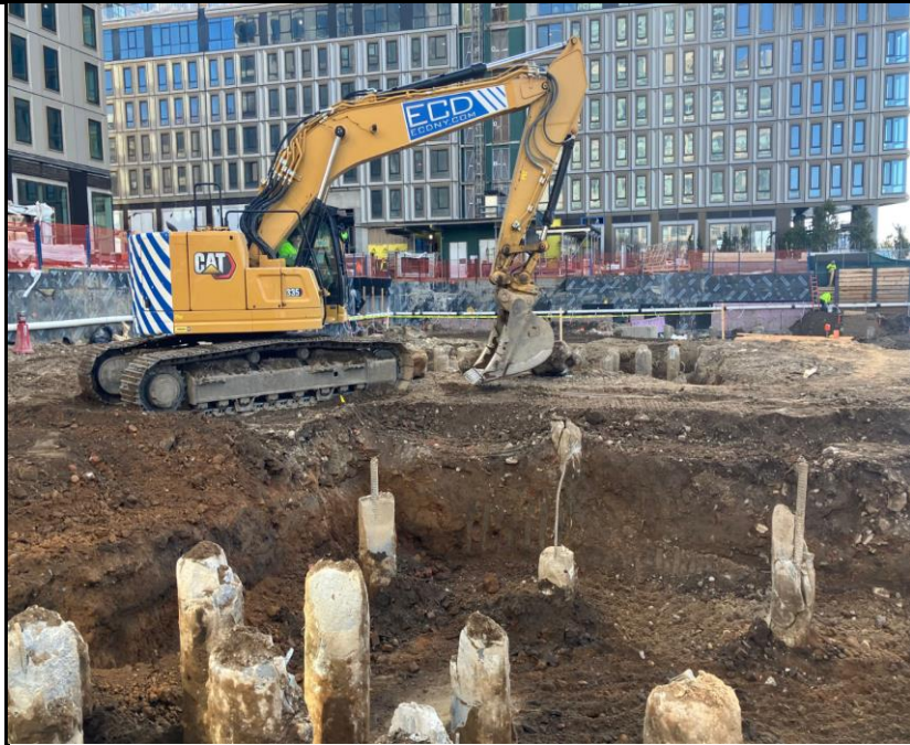
Photo 3: View of the Site facing south.
