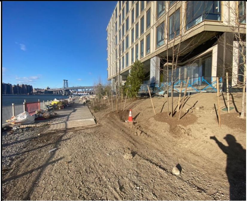
Photo 1: View of the landscaping development facing north.
