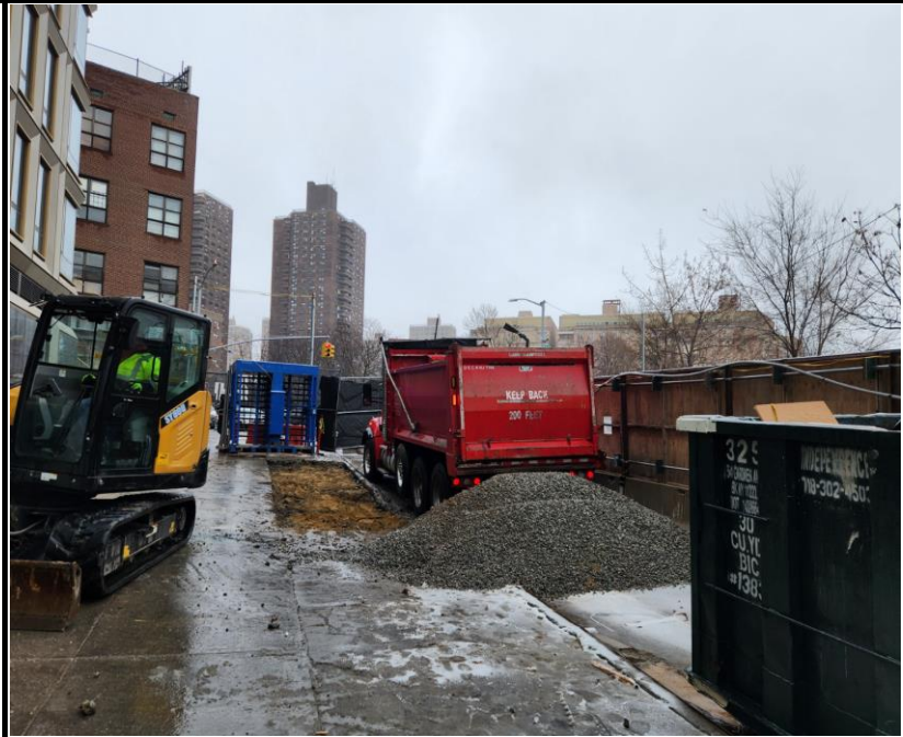
Photo 1: View of stone delivery for grading.
