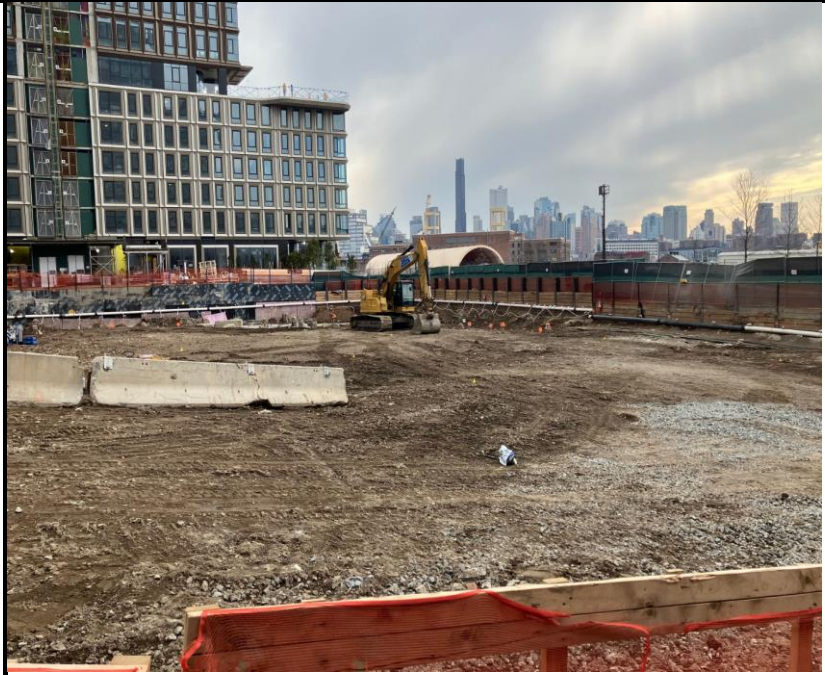
Photo 1: View of the Site facing southwest.
