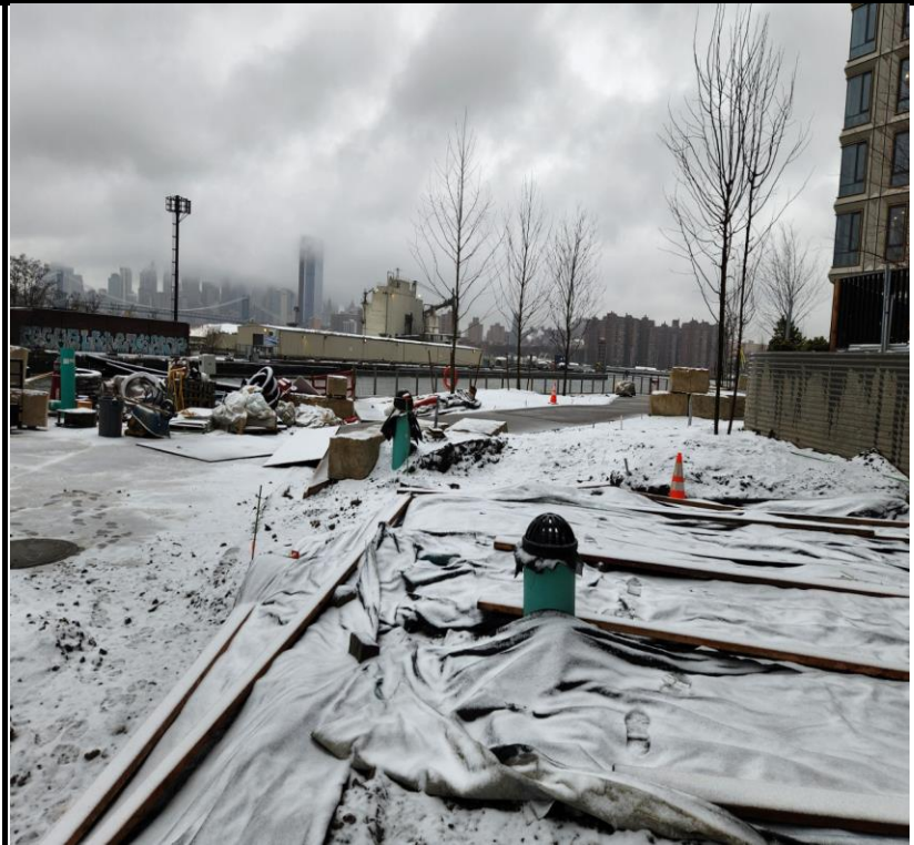
Photo 2: View of continued landscaping area conditions facing northwest.
