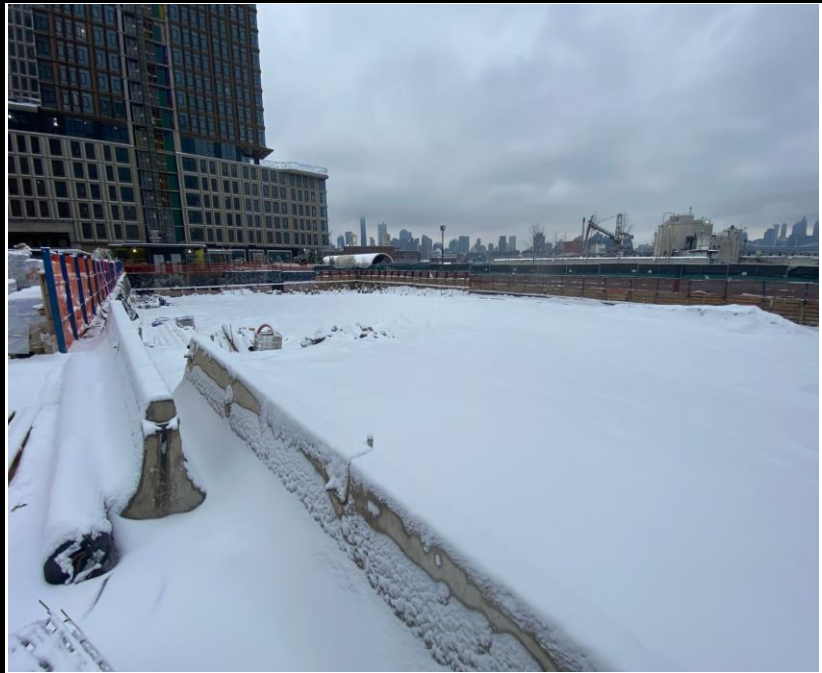
Photo 1: View of the Site facing southwest.
