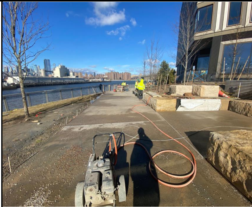
Photo 3: View of continued landscaping development facing north.
