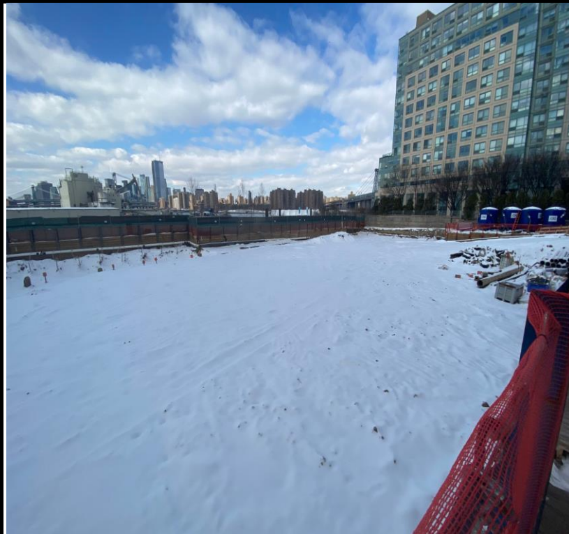
Photo 2: View of Site conditions facing northwest.
