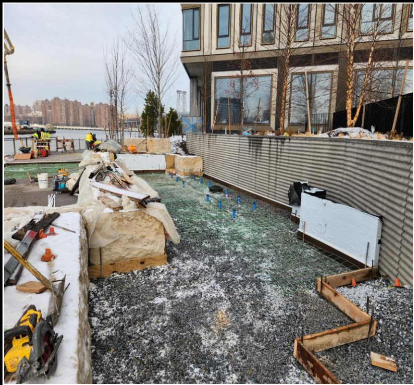
Photo 2: View of continued landscaping development facing northwest.
