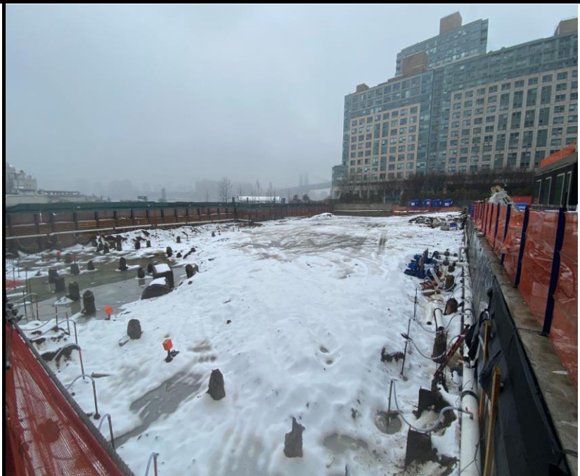
Photo 1: View of the Site facing north.
