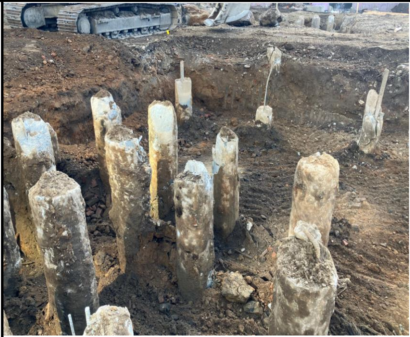
Photo 1: View of pile caps in remedial excavation.
