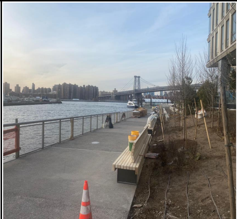
Photo 2: View of continued landscaping development facing east.
