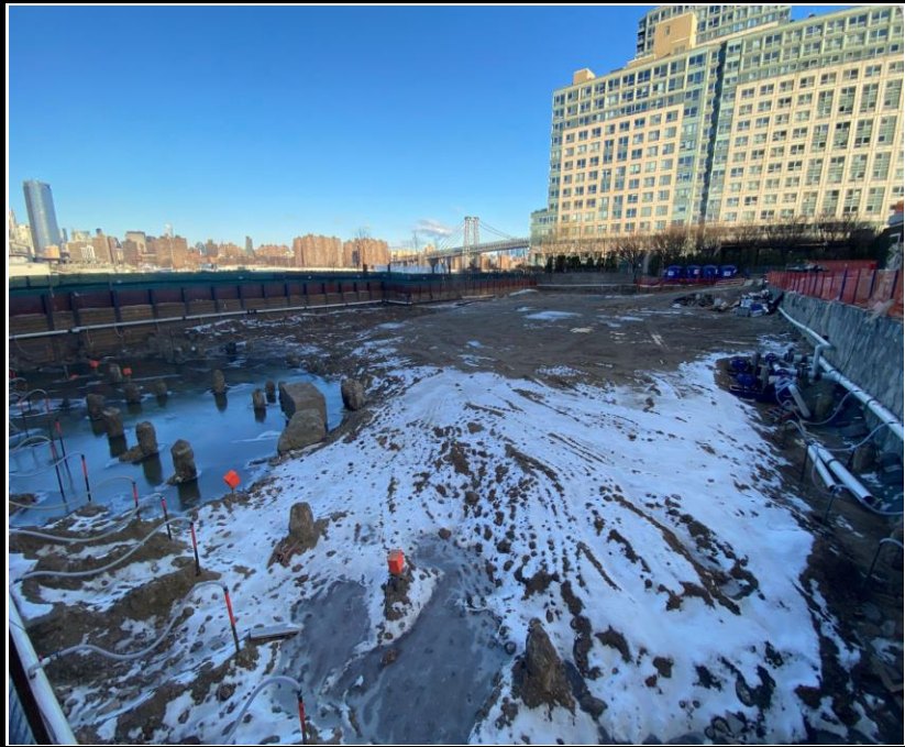
Photo 1: View of the Site facing north.
