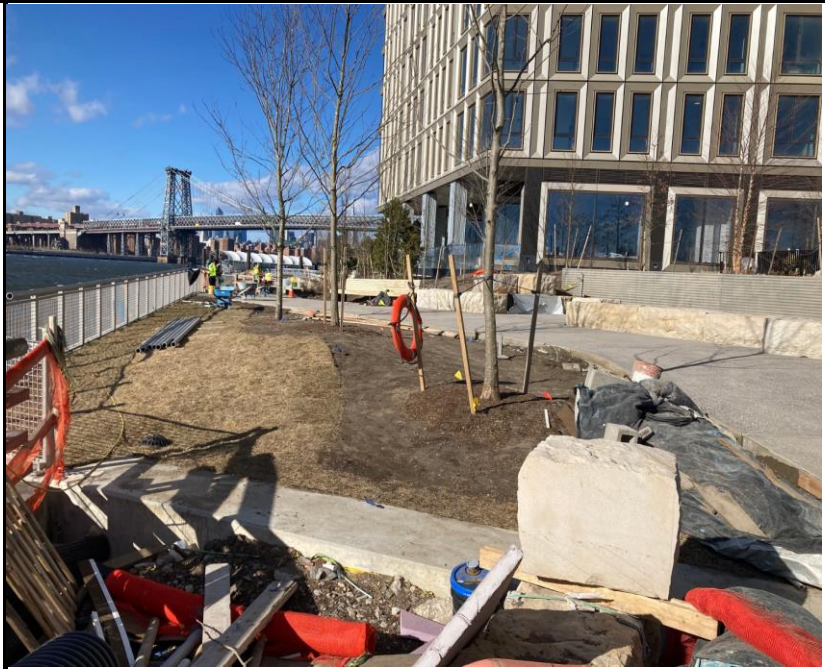
Photo 1: View of the landscaping development facing north.
