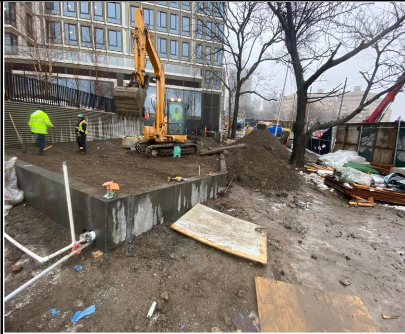
Photo 3: View of continued landscaping development facing east.
