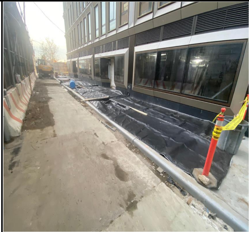
Photo 4: View of sidewalk development along Kent Avenue.
