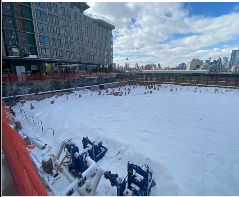
Photo 1: View of Site conditions facing southwest.
