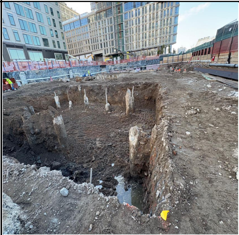
Photo 2: View of the Site facing south.
