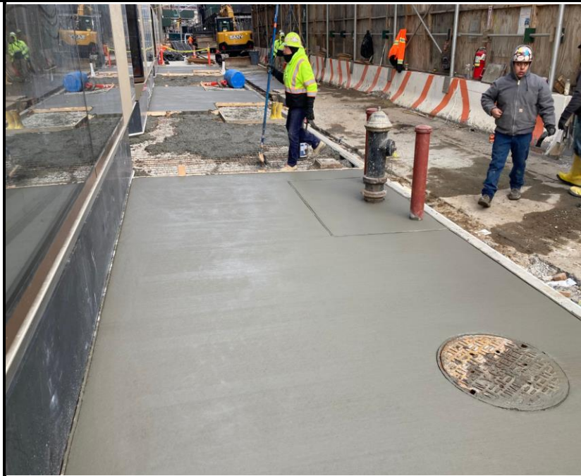
Photo 3: View of sidewalk development along Kent Avenue.
