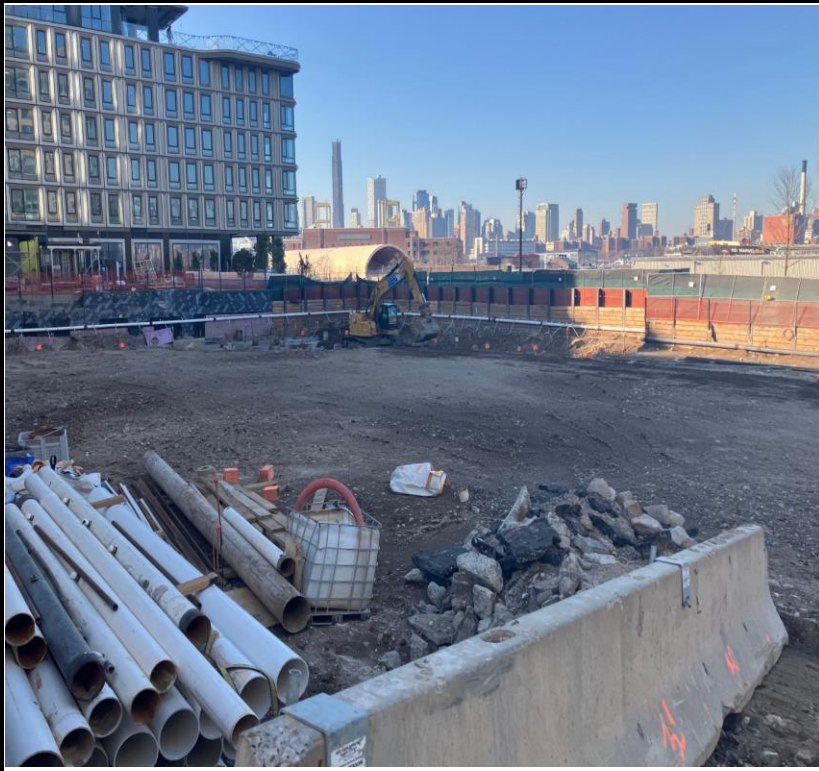
Photo 4: View of Site conditions facing southwest.
