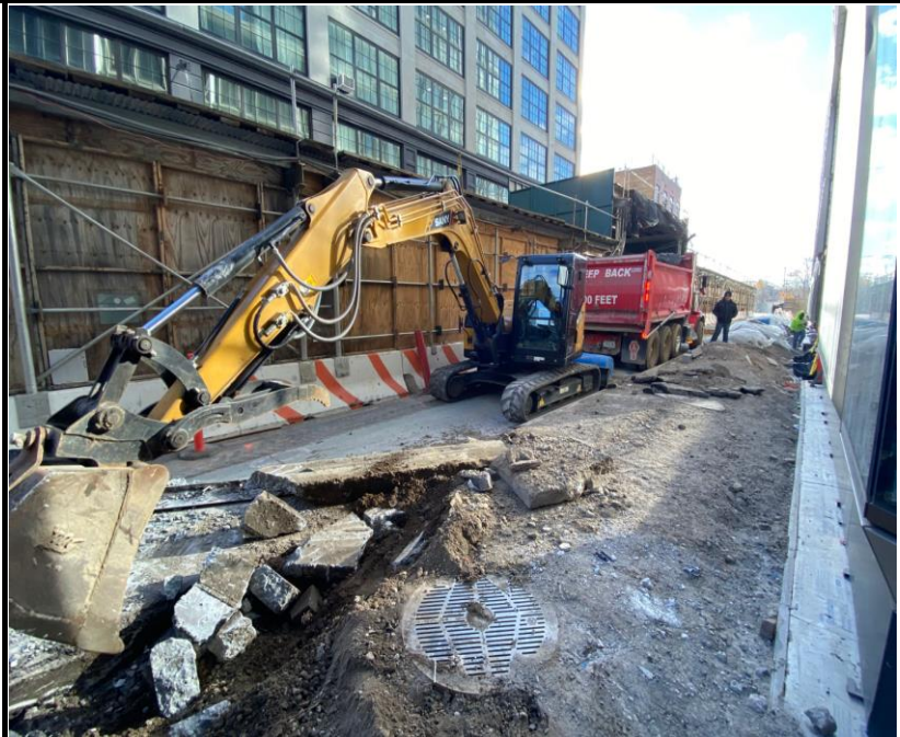
Photo 3: View of continued sidewalk development along Kent Avenue and the A2 building.
