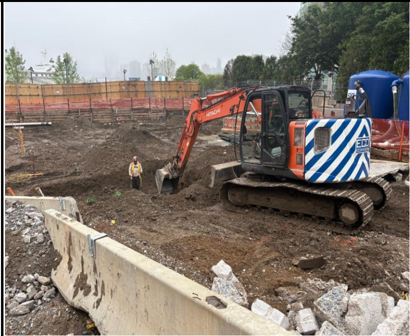
Photo 1: View of ECD completing survey.
