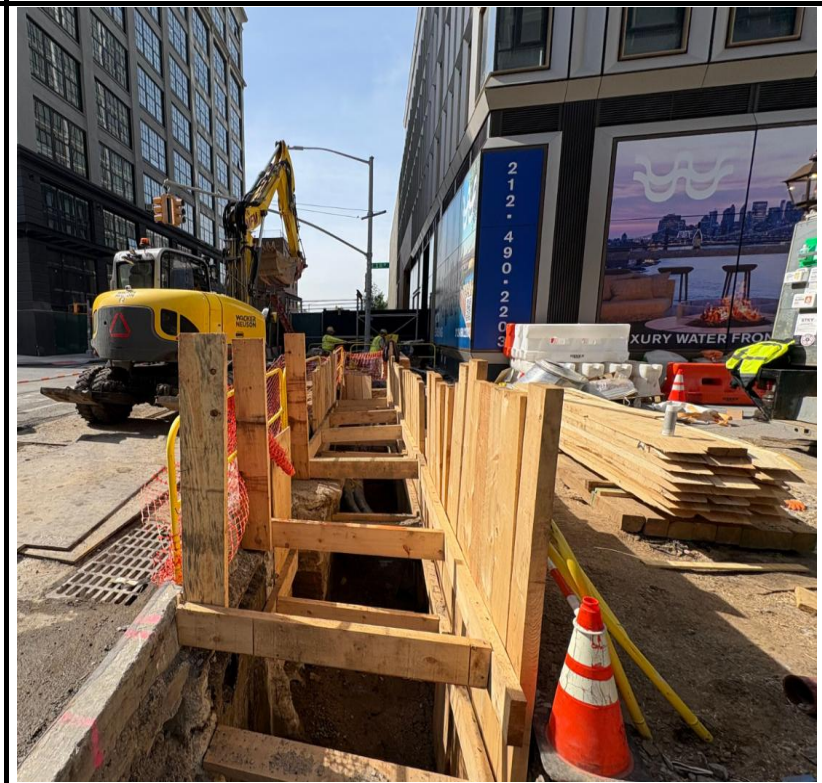
Photo 4: View of continued trench work for water line.
