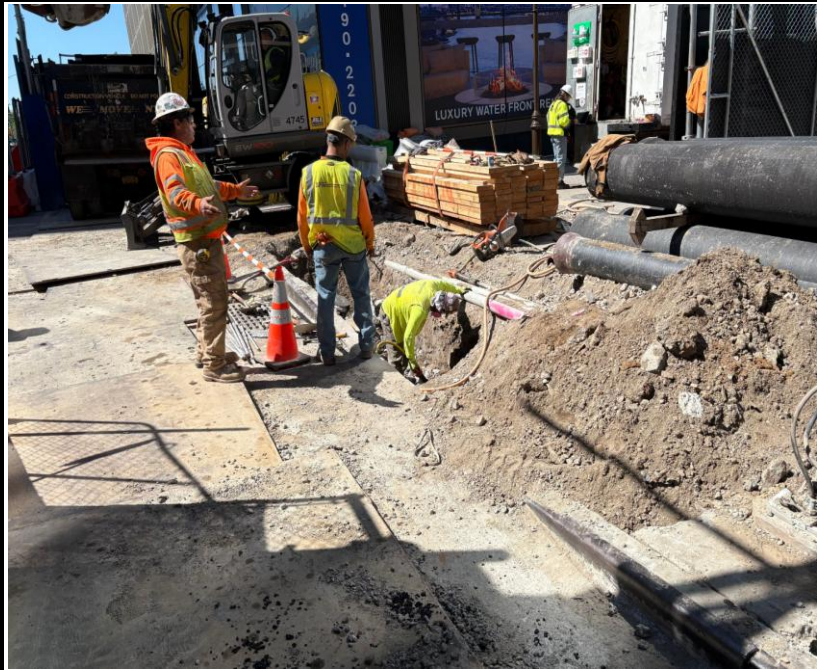
Photo 3: View of continued trench work for water line.
