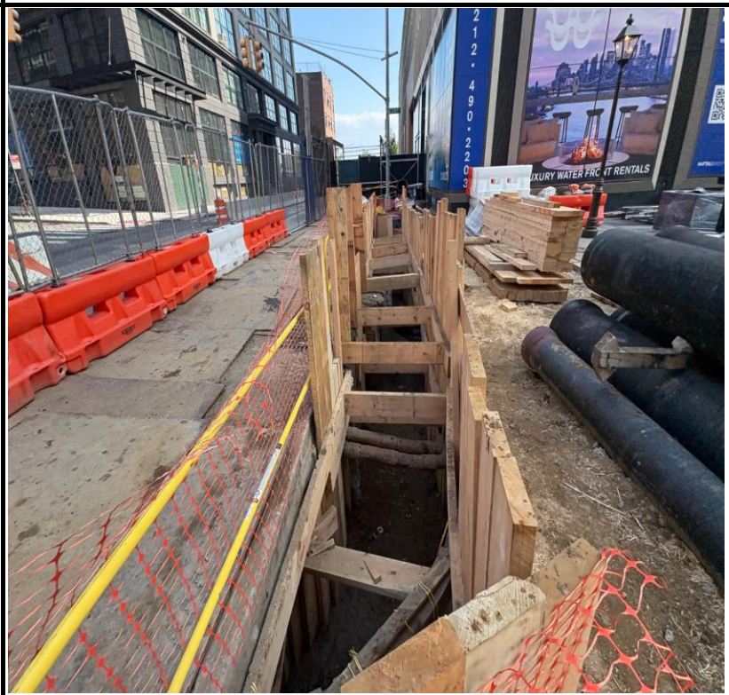
Photo 4: View of ECD completing pile installation.
