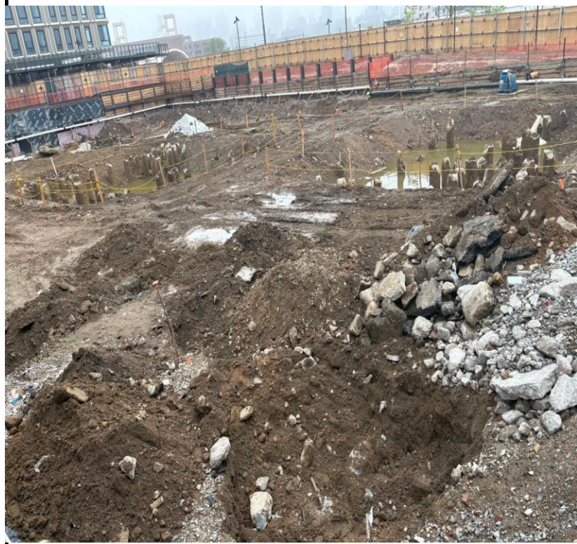
Photo 2: View of the Site facing west.
