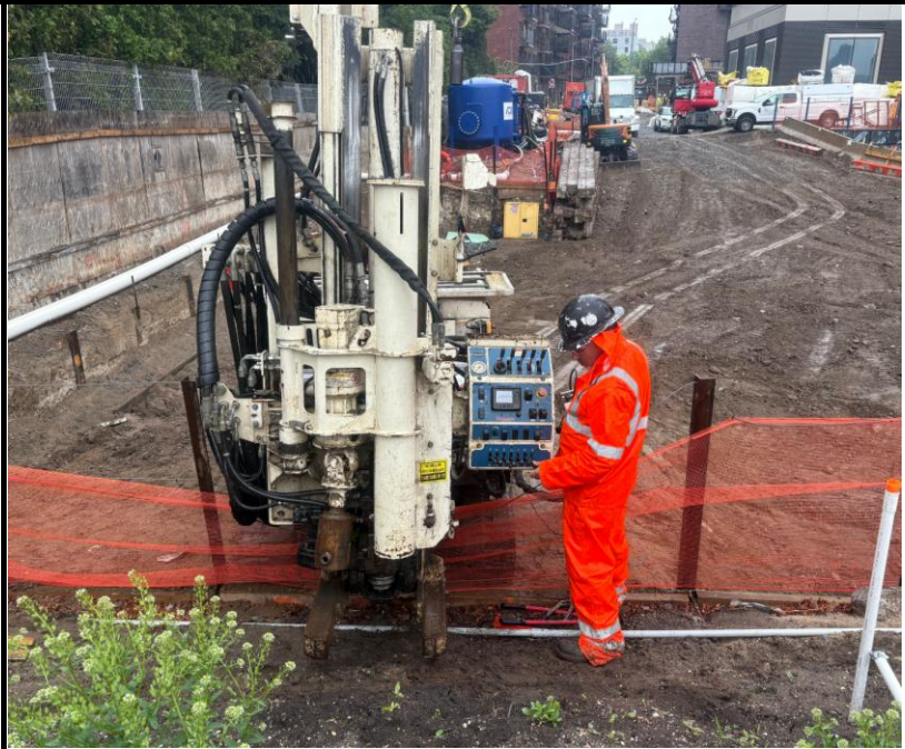
Photo 3: View of soil boring advancement.
