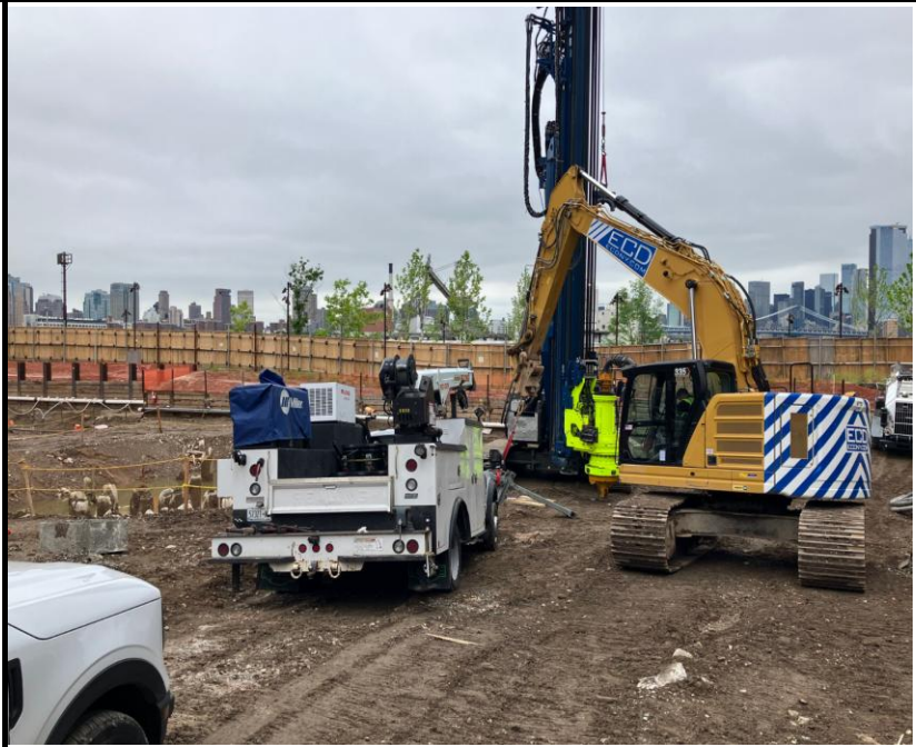
Photo 1: View of ECD mobilizing to begin additional pile installation.
