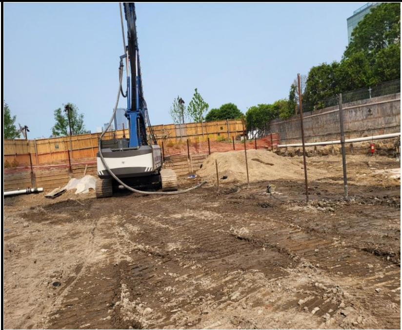
Photo 1: View of Site conditions and staged drill rig facing west.
