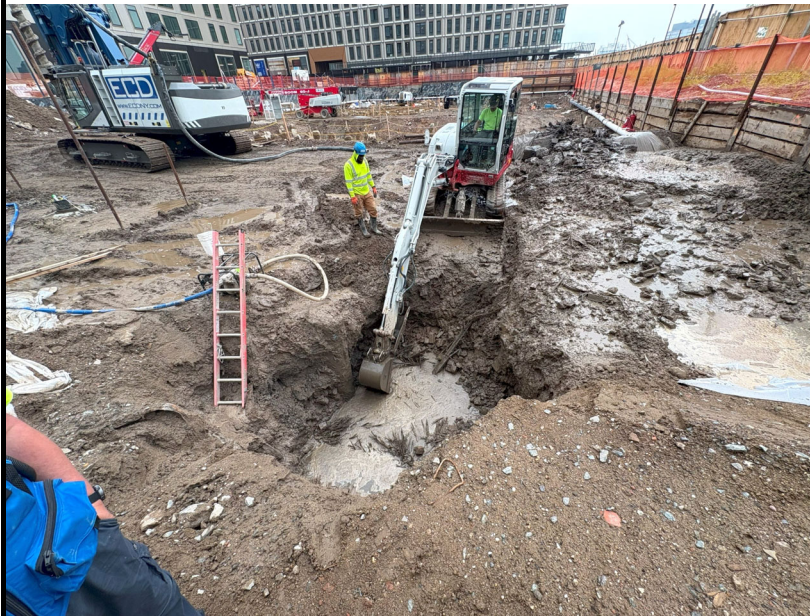
Photo 3: View of excavation.
