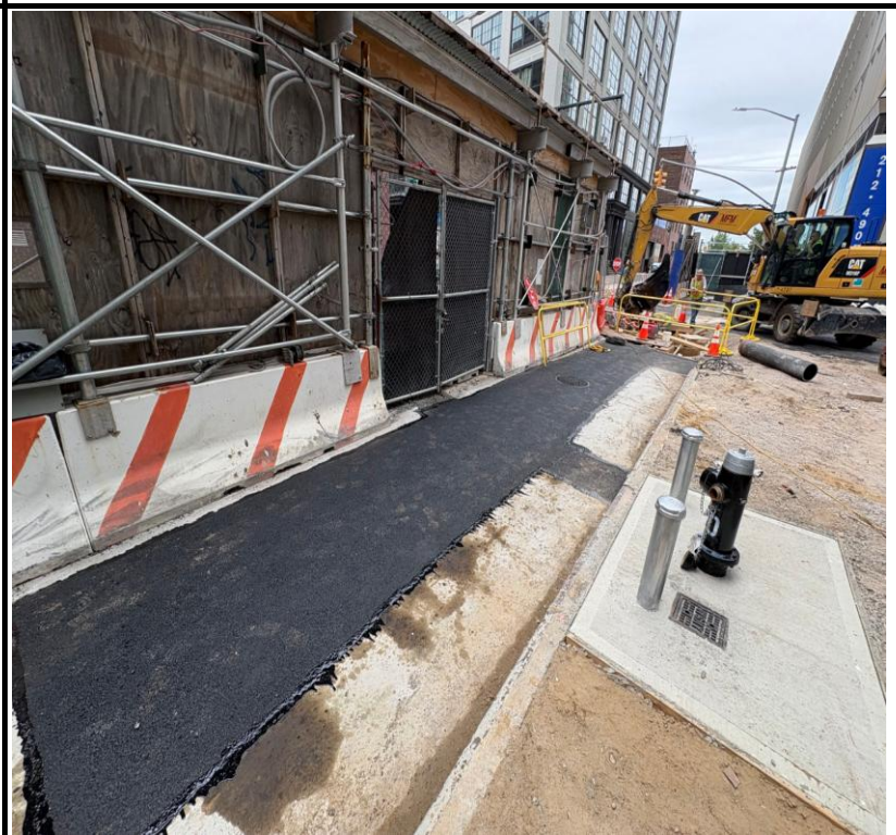
Photo 2: View of continued water line installation along Kent Avenue.
