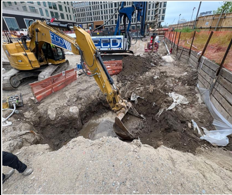
Photo 3: View of additional soil excavation in the west sidewall of PWS 27.
