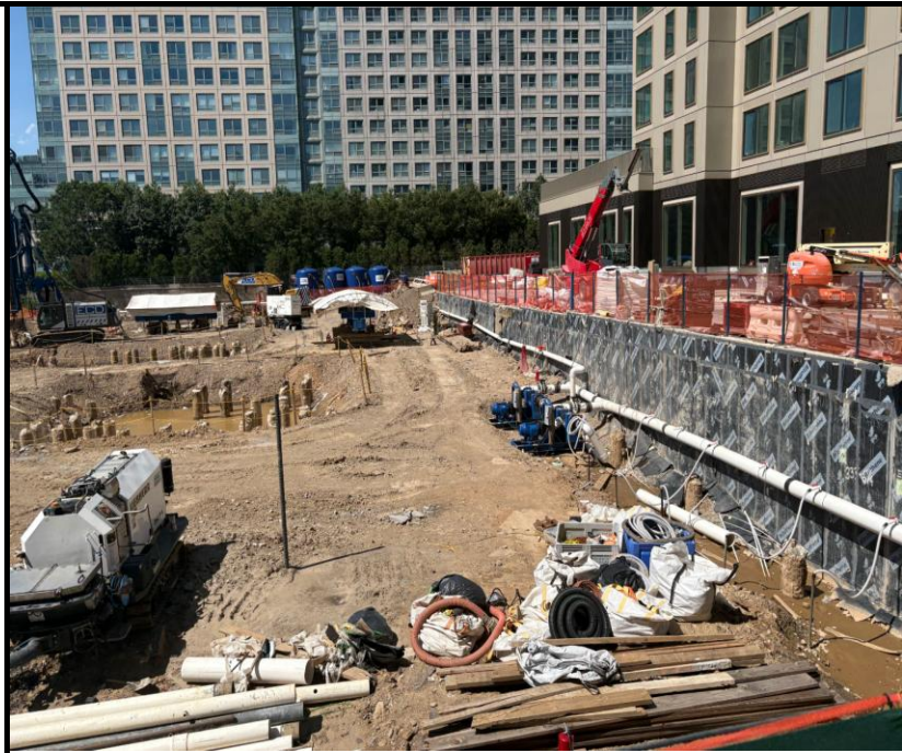
Photo 3: View of the Site facing northeast.
