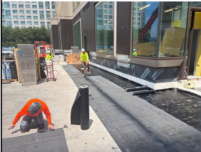
Photo 4: View of waterproofing installation in the courtyard.
