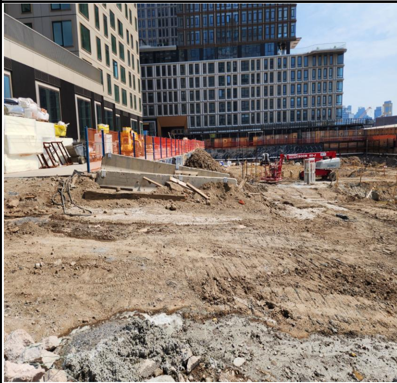
Photo 4: View of Site conditions facing south.
