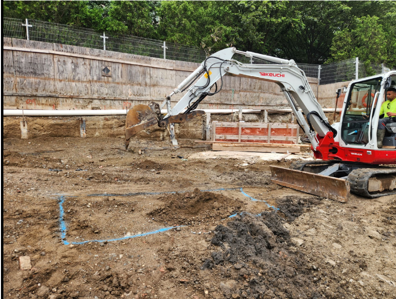
Photo 1: View of markout for test pit.
