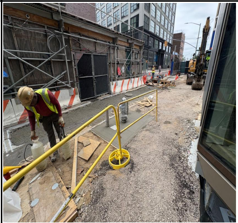
Photo 2: View of continued water line installation and new concrete for fire hydrant.
