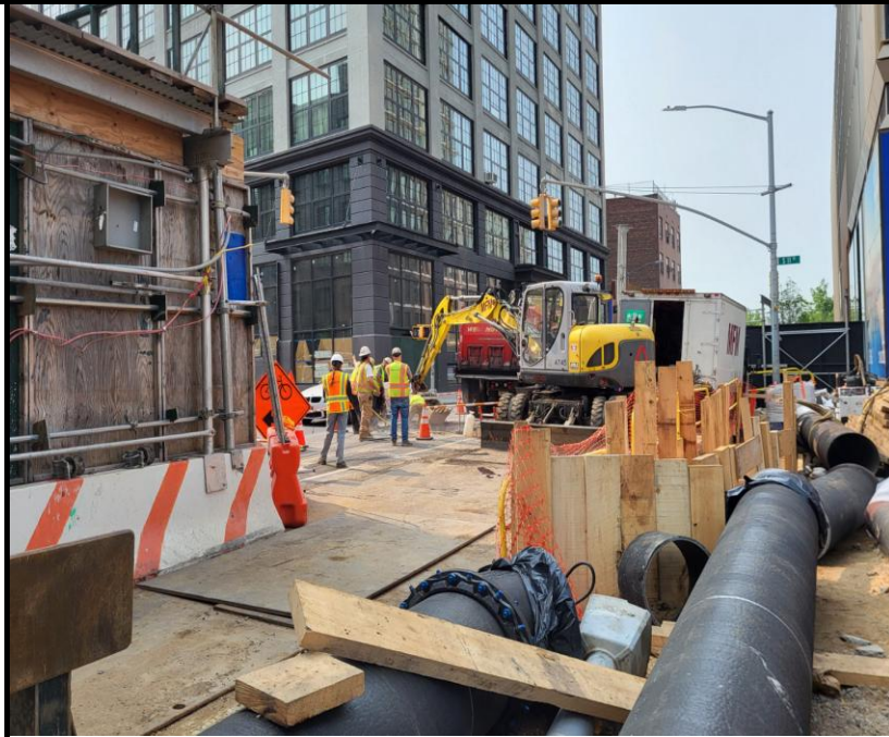
Photo 3: View of continued water line installation.
