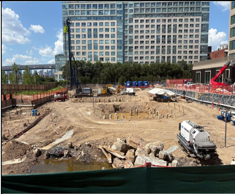
Photo 1: View of the Site facing north.
