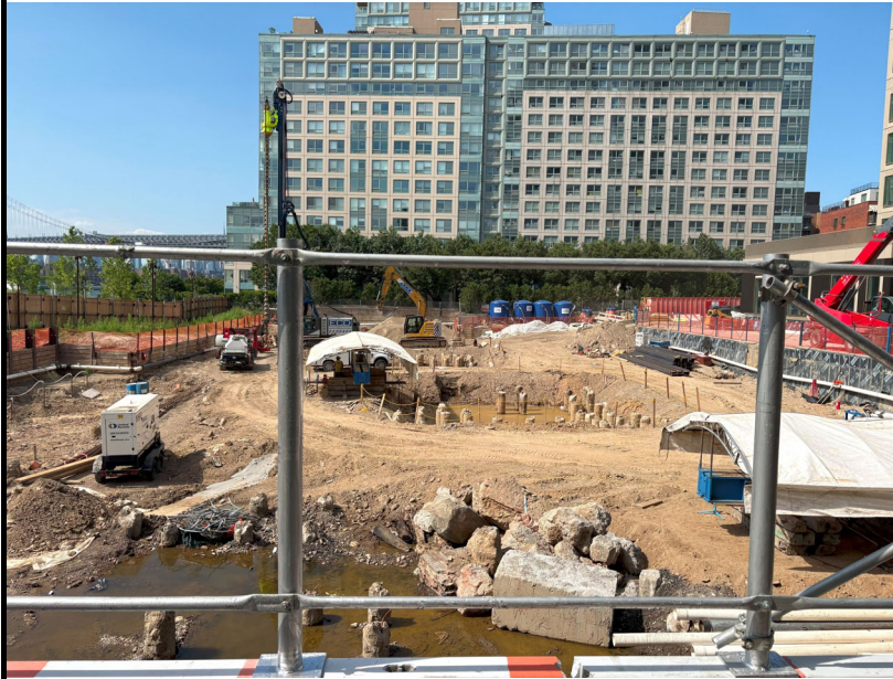
Photo 1: View of the Site facing north.
