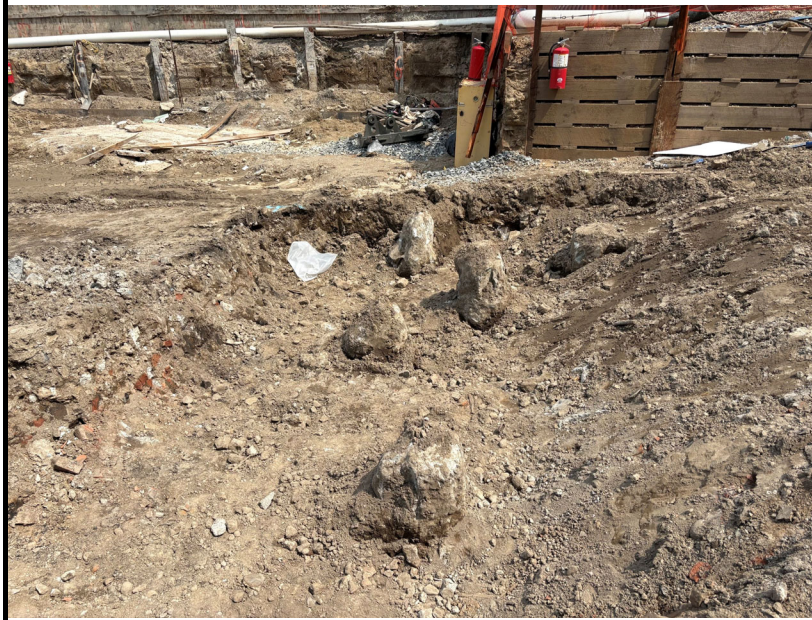
Photo 3: View of UST grave excavation, looking north.
