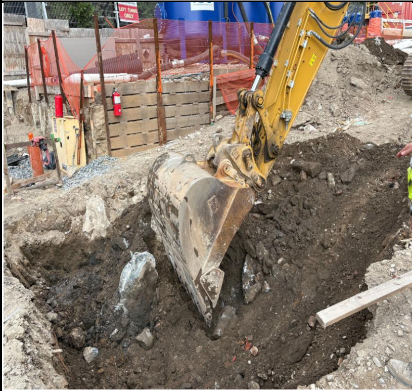
Photo 4: View of additional soil excavation in the tank grave.
