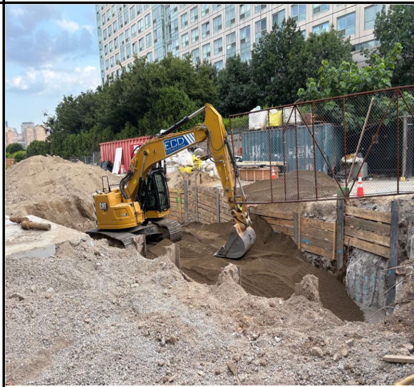
Photo 2: View of RCA cap grading.
