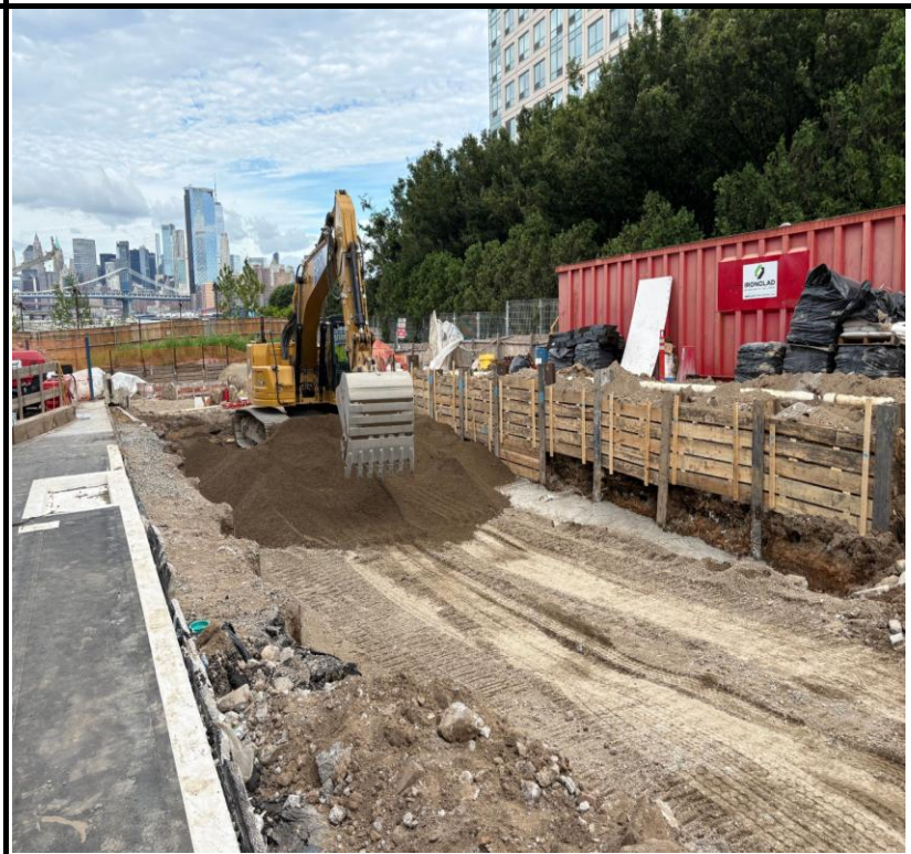
Photo 2: View of RCA cap grading.
