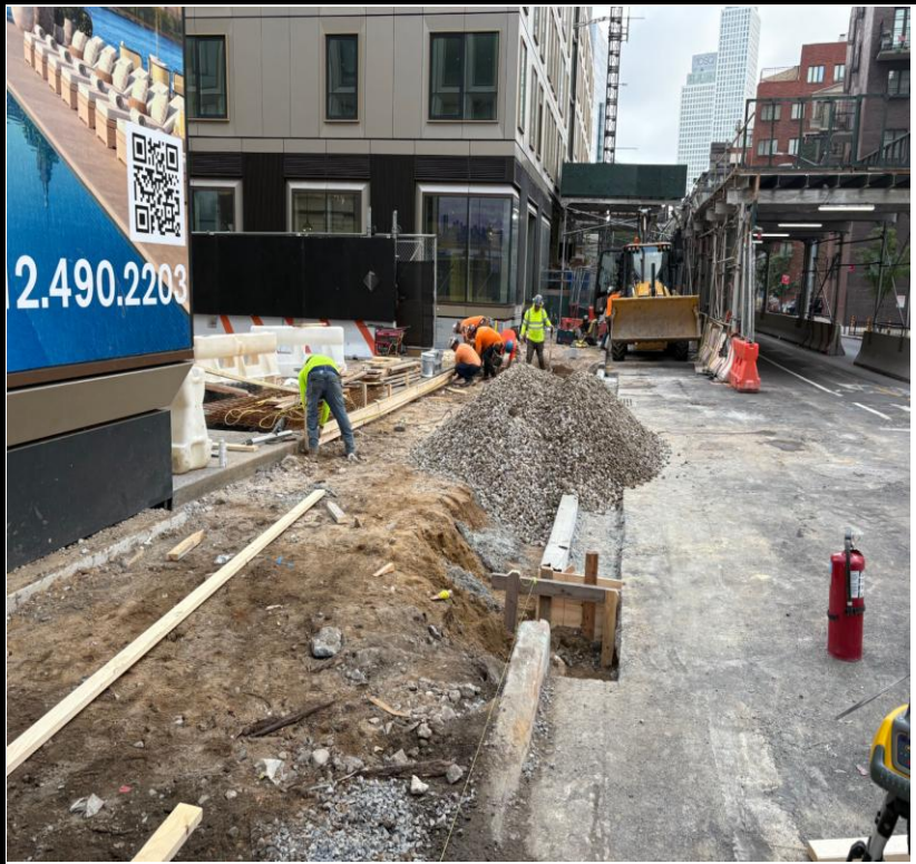
Photo 2: View of curb installation along Kent Avenue.
