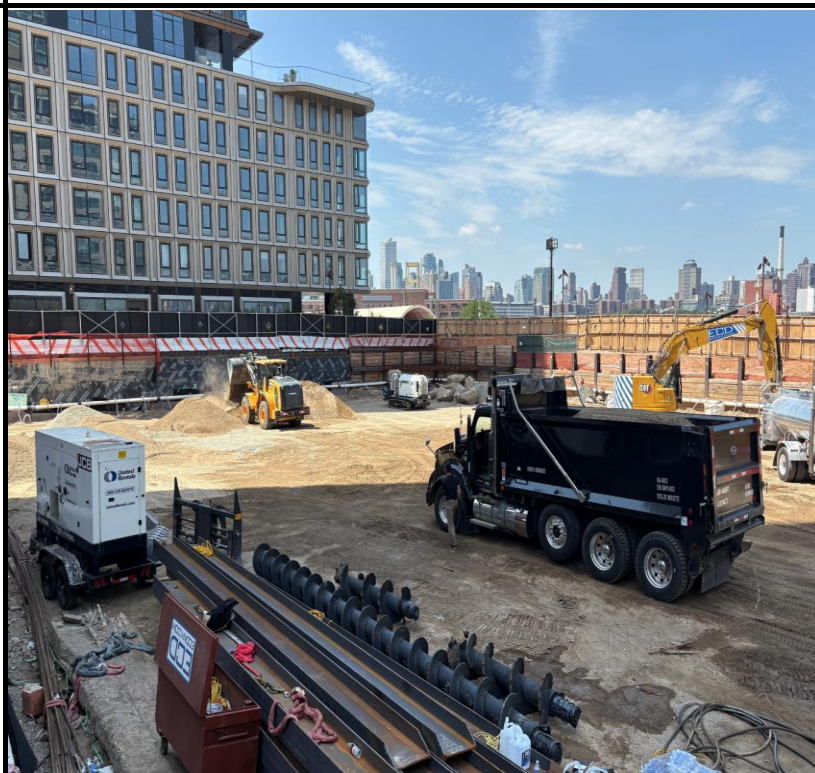
Photo 2: View of RCA cap placement.
