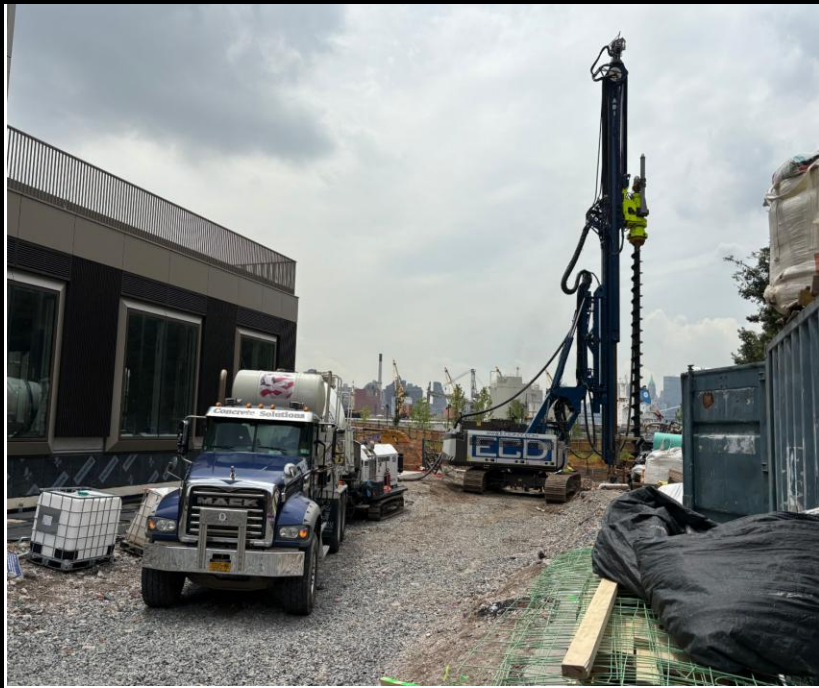
Photo 3: View of pile installation for SOE in the utility driveway area..
