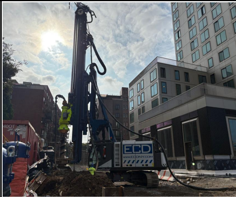
Photo 3: View of pile installation for SOE in the utility driveway area.
