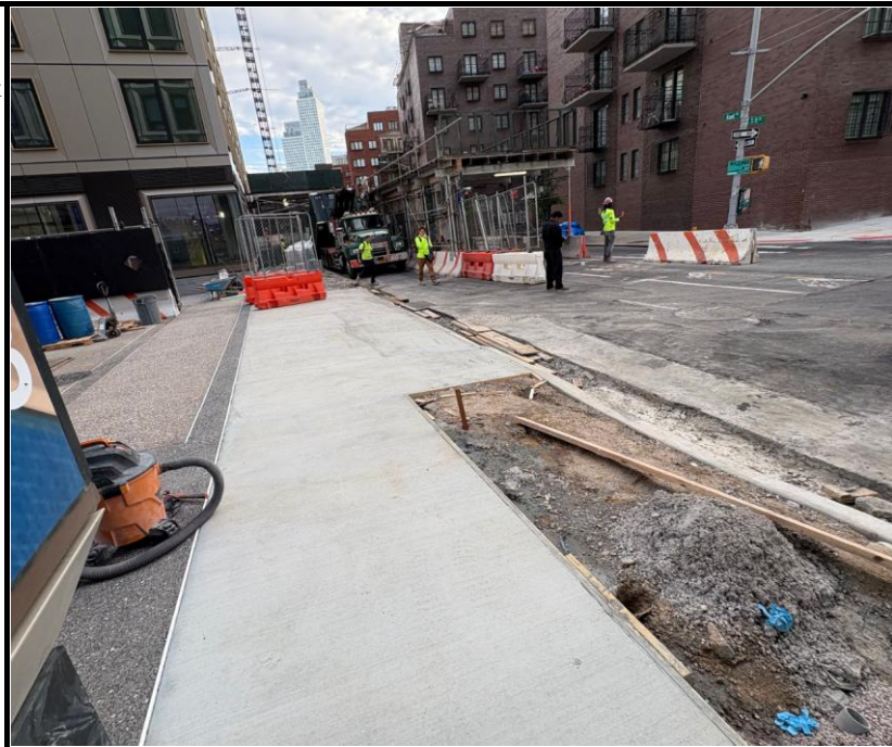
Photo 3: View of continued curb installation work along Kent Avenue.
