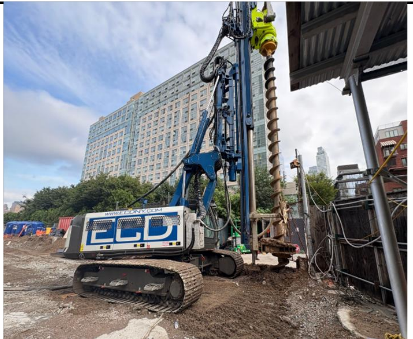
Photo 1: View of pile installation for SOE in the utility driveway area.
