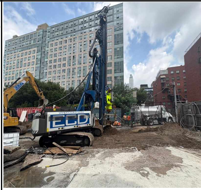
Photo 4: View of pile installation for SOE in the utility driveway area.e.
