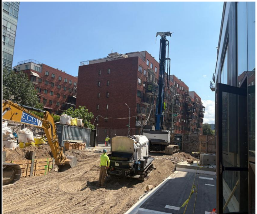
Photo 1: View of pile installation.
