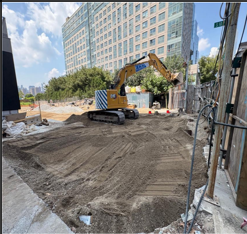
Photo 4: View of continued cap installation and grading.
