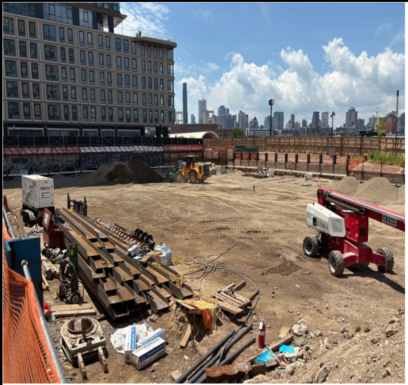
Photo 2: View of RCA cap placement and grading.
