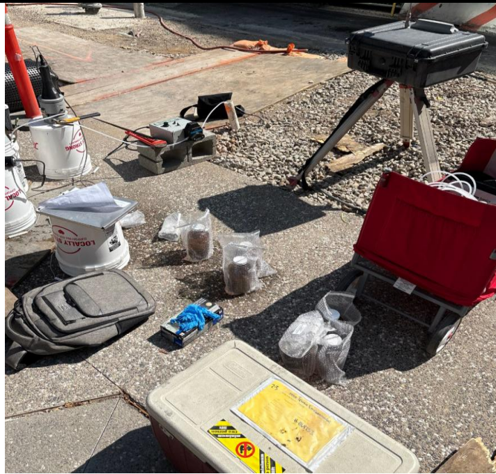
Photo 3: View of groundwater sampling.
