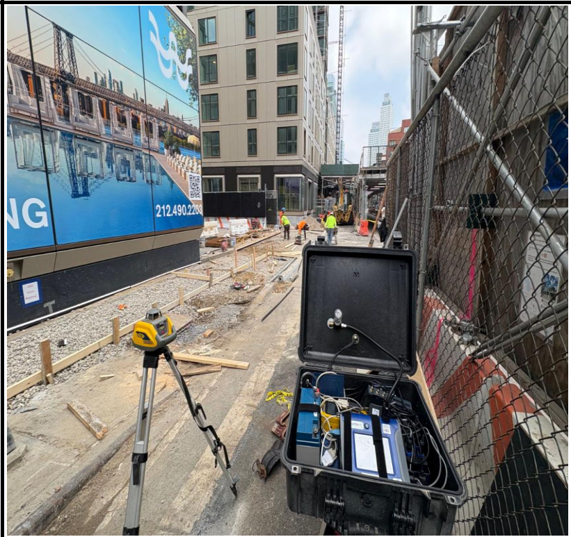
Photo 4: View of curb installation along Kent Avenue.
