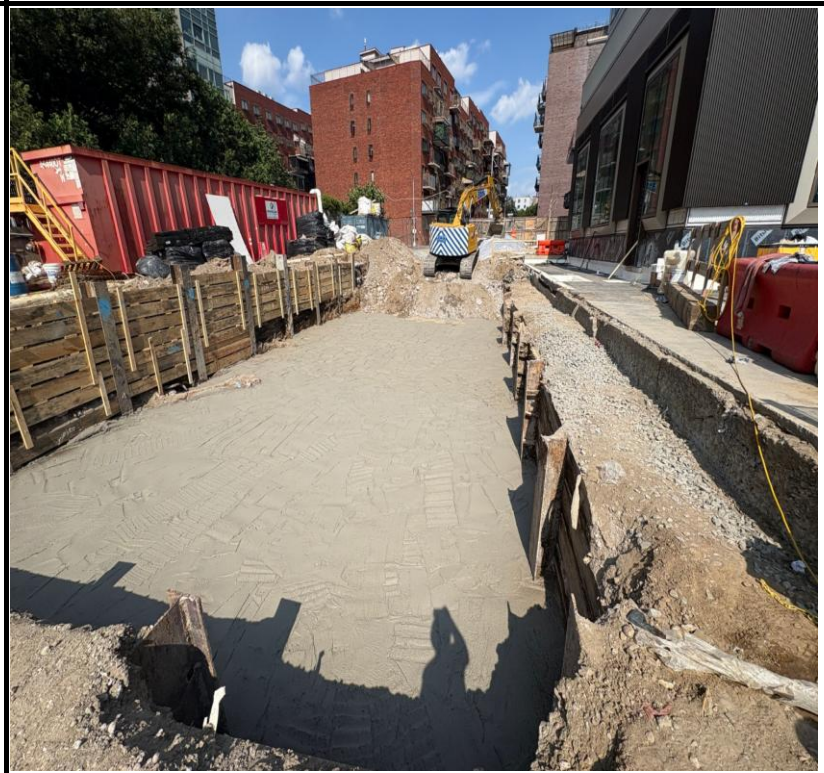
Photo 4: View of cap in the utility driveway.
