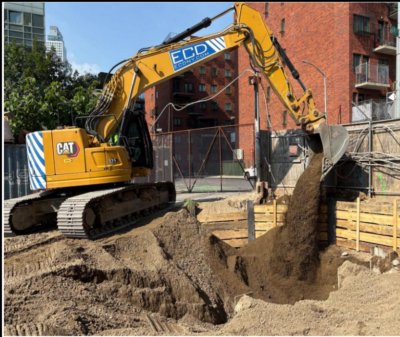
Photo 3: View of continued RCA cap installation and grading.
