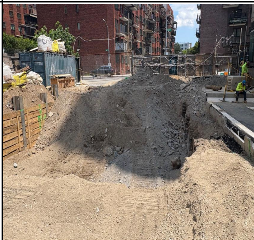
Photo 2: View of RCA cap grading.
