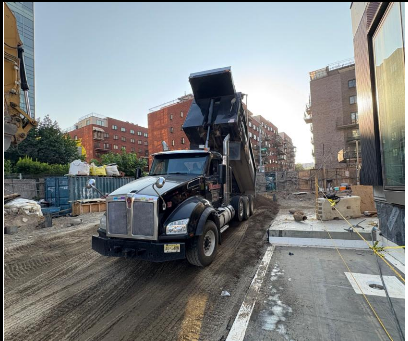
Photo 3: View of RCA import for continued cap installation and grading.
