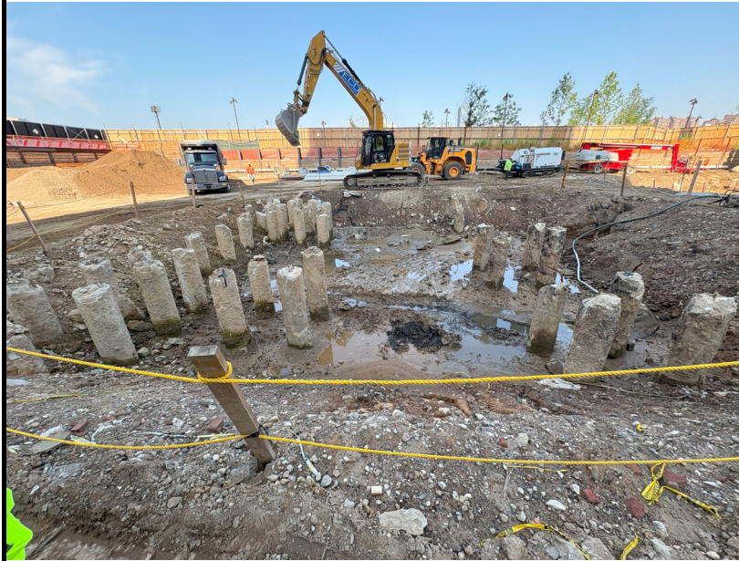
Photo 1: View of PWSB-21 following dewatering and prior to backfill placement.
