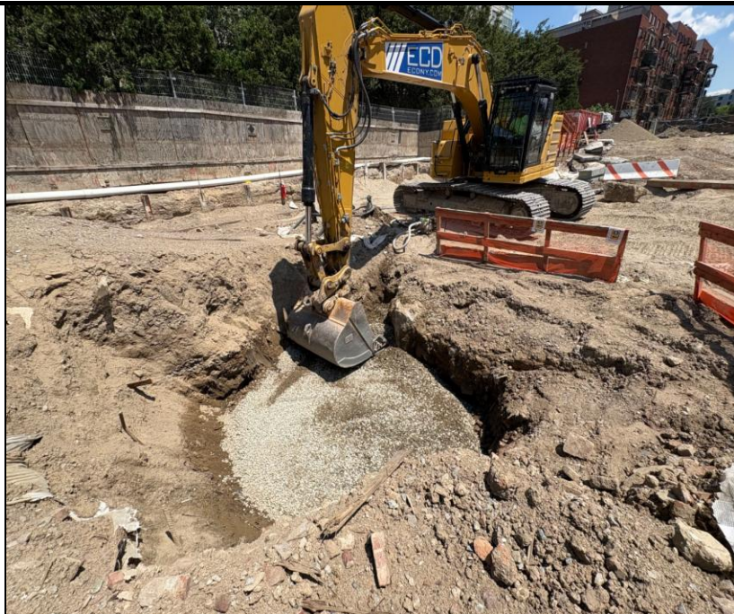
Photo 1: View of PWSB-27 sidewalk backfilling.
