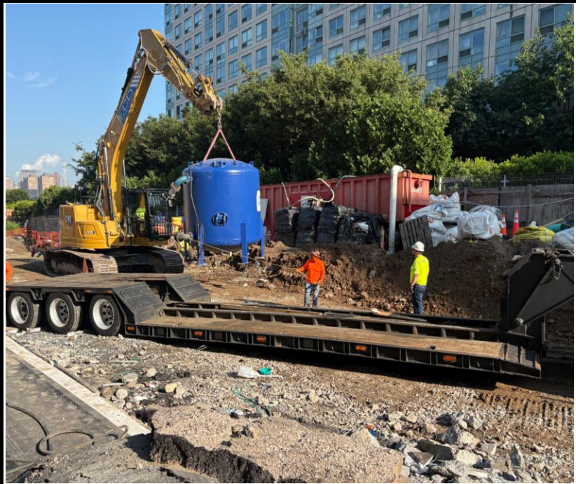
Photo 1: View of dewatering system component demobilization.
