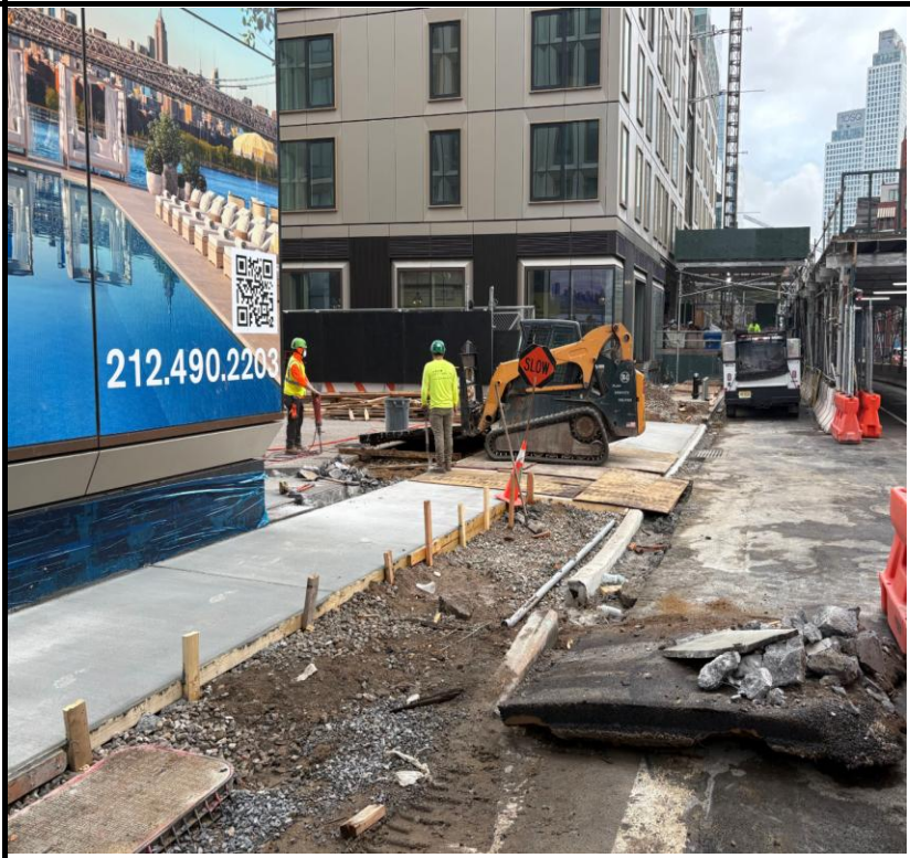
Photo 2: View of curb installation along Kent Avenue.
