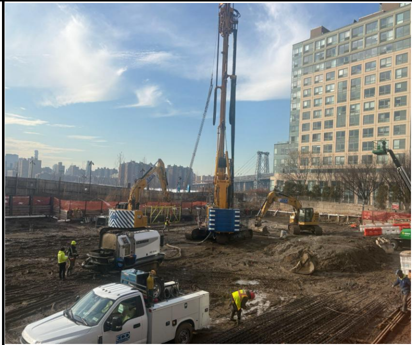
Photo 3: View of pile installation and site conditions facing northwest.
