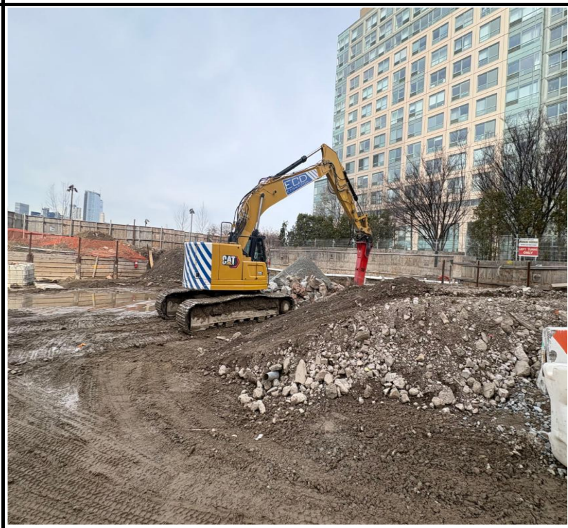
Photo 2: View of soil excavation and concrete hammering facing northwest.
