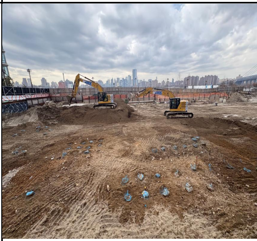
Photo 4: View of soil excavation and site conditions facing west.
