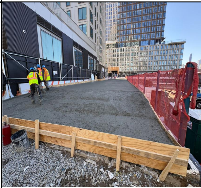
Photo 4: View of concrete pour for patio development
