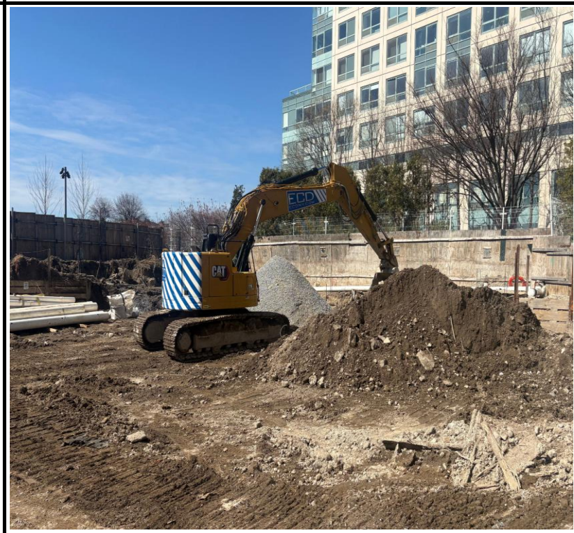
Photo 4: View of RCA stockpile for off-site disposal.
