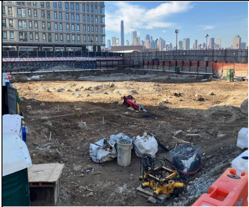
Photo 1: View of site conditions facing southwest.
