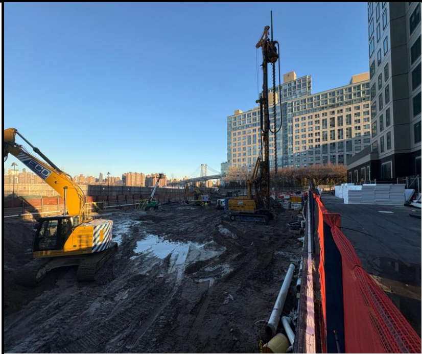
Photo 1: View of pile installation and Site conditions facing northwest.
