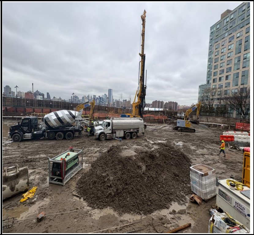
Photo 2: View of pile installation and site conditions facing west.
