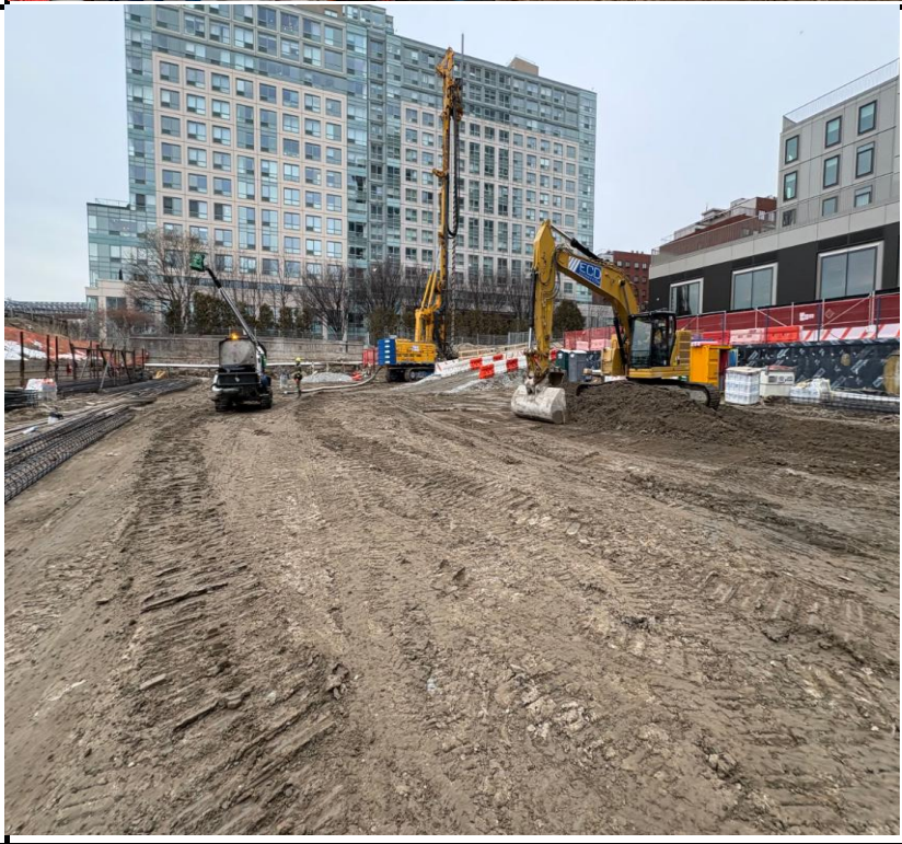
Photo 4: View of pile installation and site conditions facing north.
