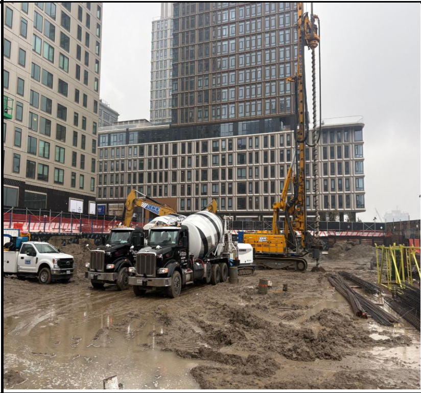
Photo 2: View of pile installation and site conditions facing south.
