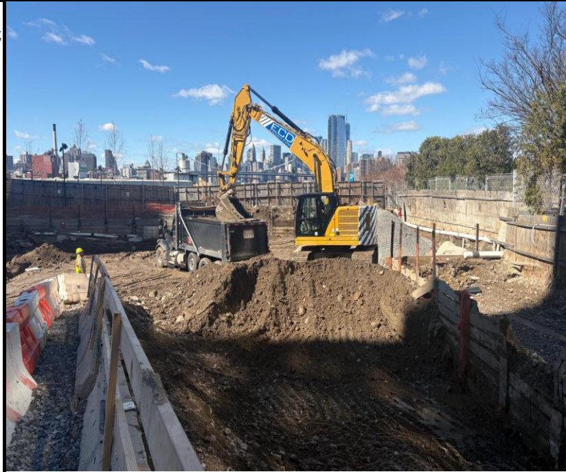
Photo 3: View of truck loading for off-site disposal of RCA cap.
