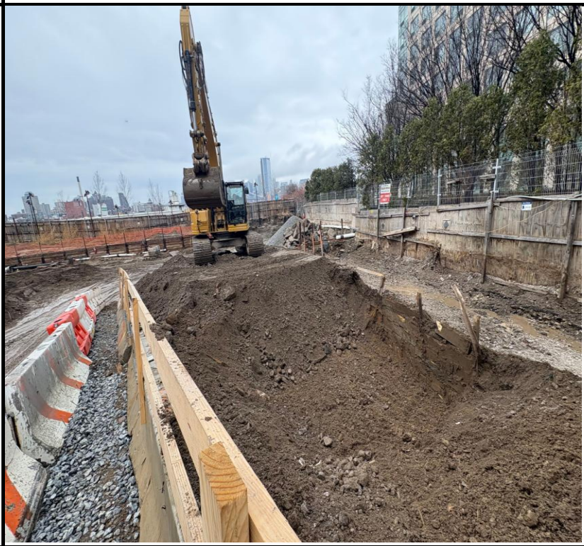
Photo 2: View of soil cap excavation and concrete facing west.
