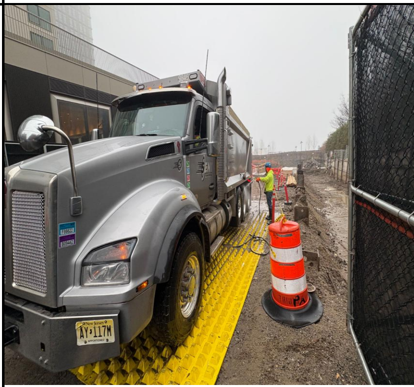
Photo 4: View of truck washing prior to trucks leaving the Site.
