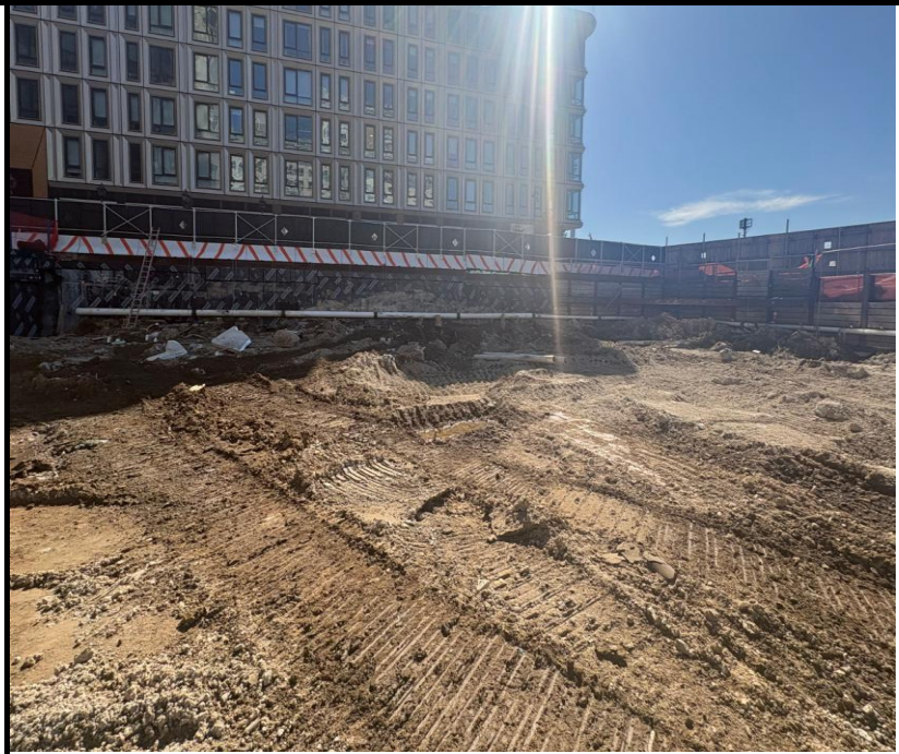
Photo 3: View of dewatering pipe installation.
