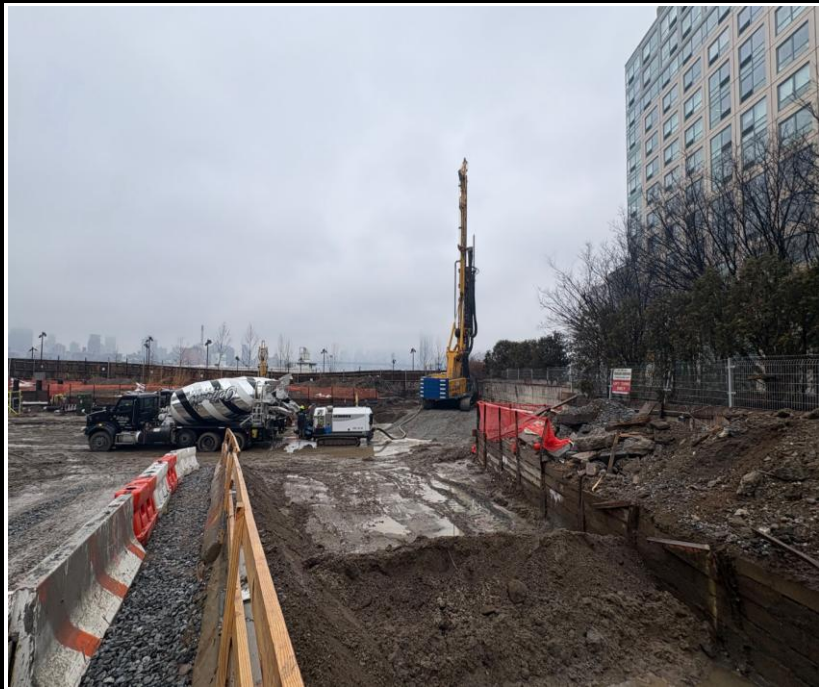
Photo 3: View of pile installation and site conditions facing west.
