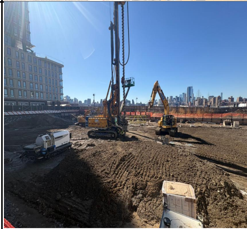
Photo 4: View of pile installation and site conditions facing west.
