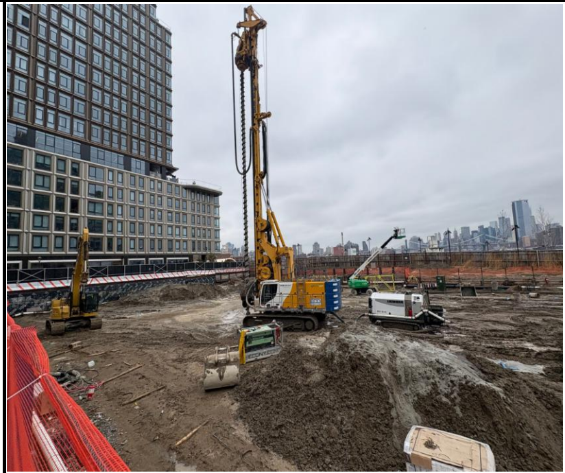
Photo 3: View of pile installation and site conditions facing southwest.
