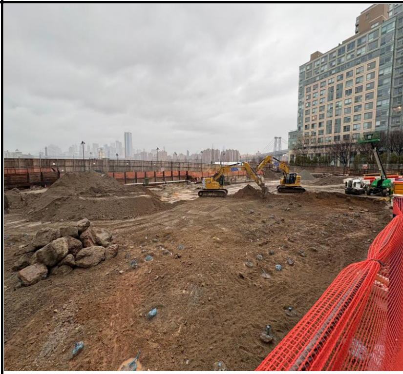
Photo 2: View of soil excavation and site conditions facing northwest.
