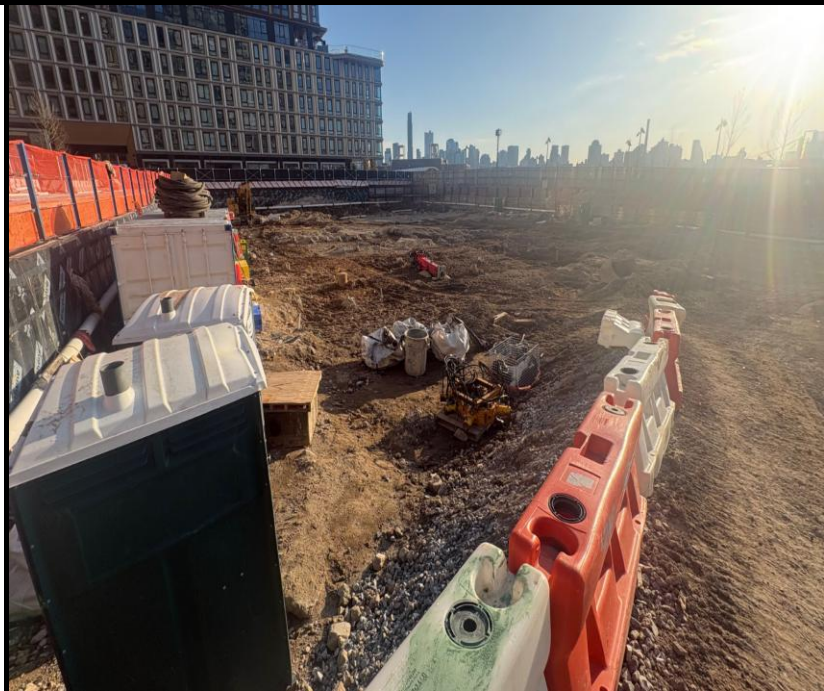
Photo 3: View of site conditions facing southwest.
