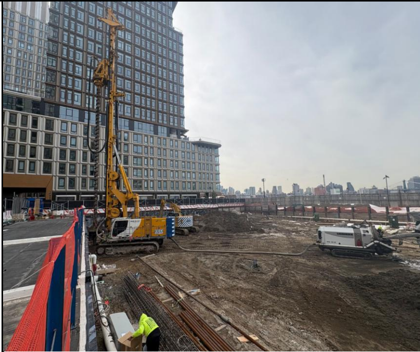
Photo 1: View of the Site and pile installation facing southwest.
