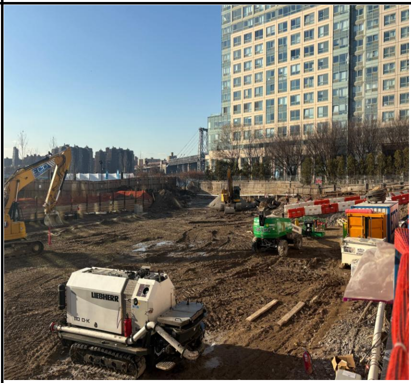
Photo 2: View of pile installation and site conditions facing northwest.
