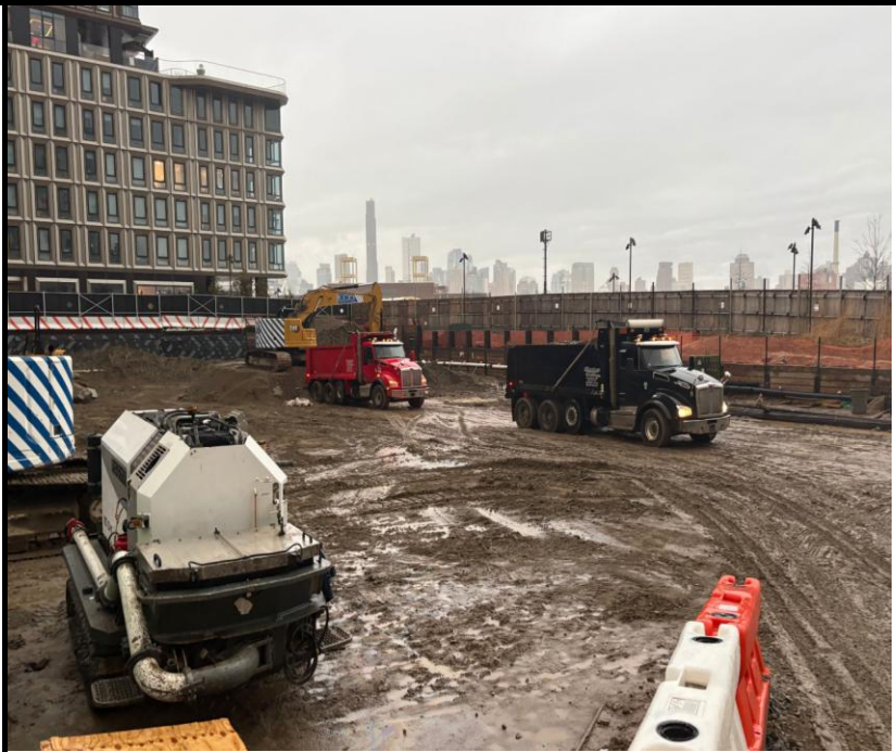
Photo 1: View of truck loading for off-site soil disposal.
