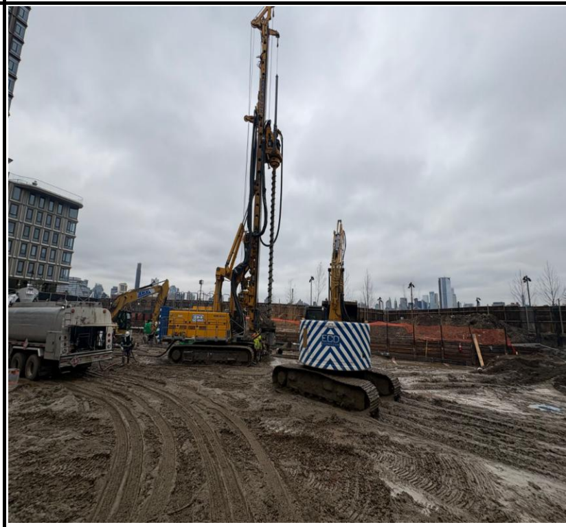
Photo 4: View of pile installation and site conditions facing west.
