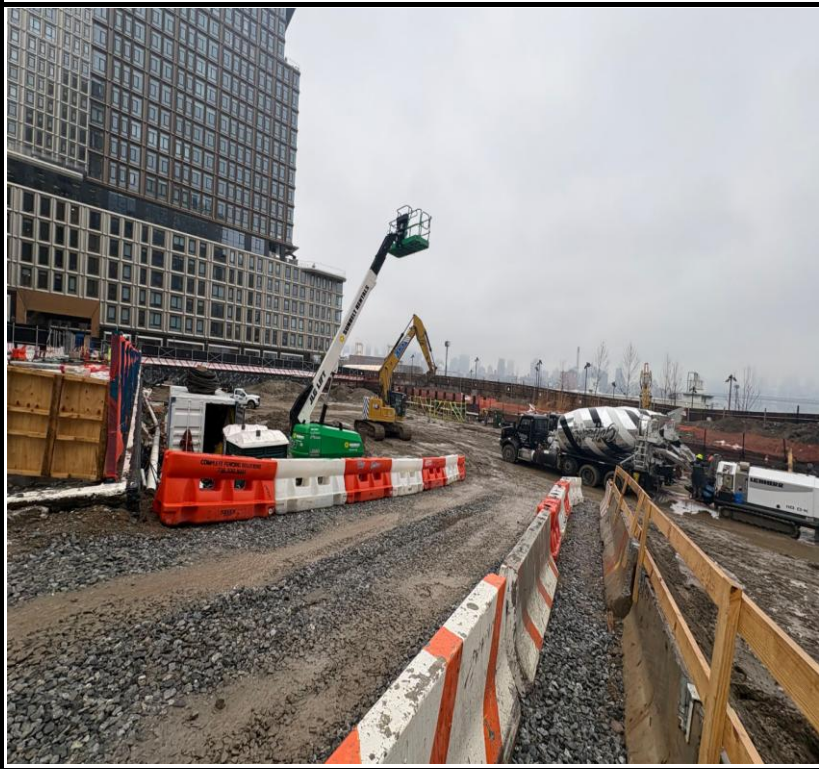
Photo 4: View of pile installation and site conditions facing southwest.
