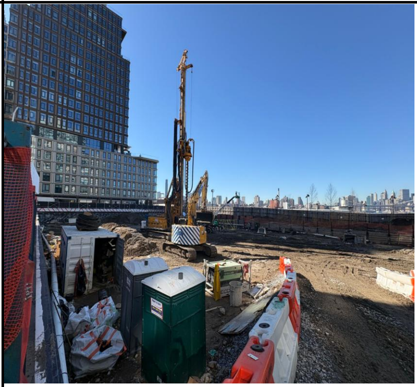
Photo 2: View of pile installation and site conditions facing southwest.
