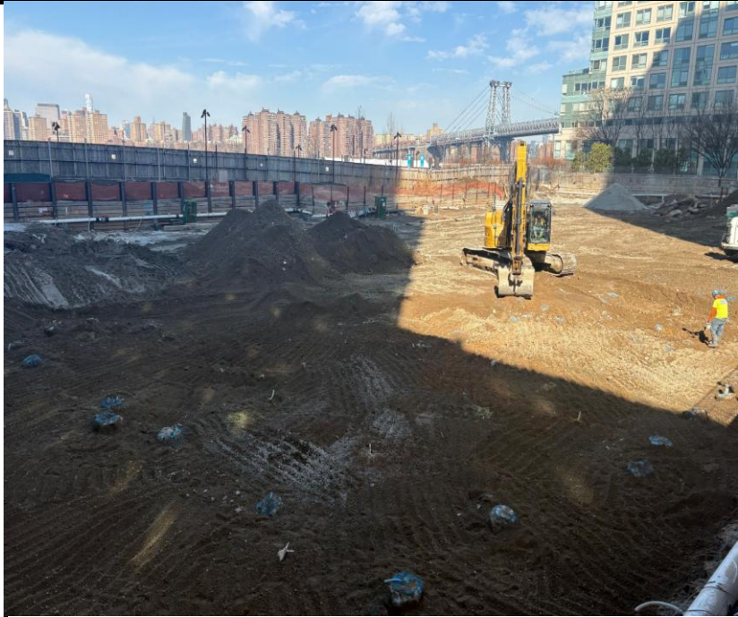
Photo 3: View of soil excavation and site conditions facing northwest.
