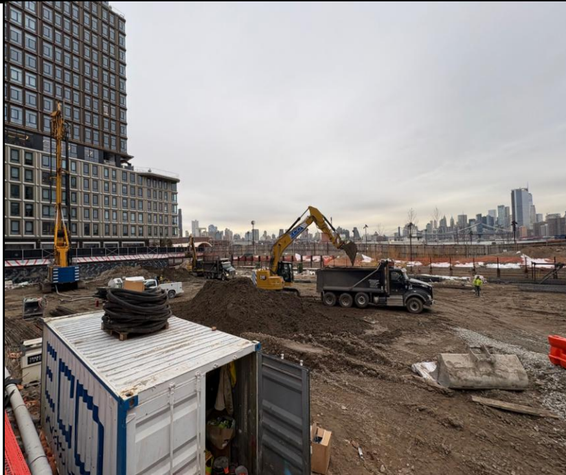
Photo 3: View of pile truck loading for off-site soil disposal.
