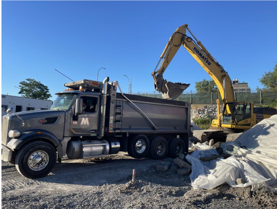
Photo 1: Kingdom loading a permitted tri-axle truck with non-hazardous soil in the southwestern part of Sackett Place (facing southeast)
