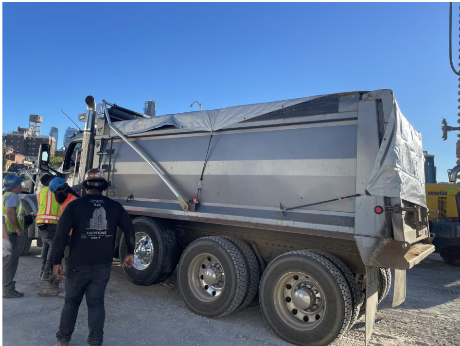
Photo 2: Kingdom applying a tight-fitting cover to a truck prior to exporting soil for off-site disposal (facing north)
