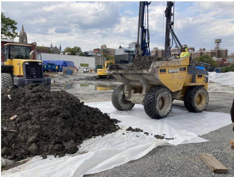
Photo 2: Kingdom stockpiling drilling spoils on polyethylene sheeting in the southeastern part of Sackett Place (facing northwest)
