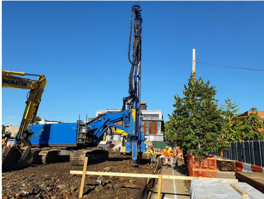
Photo 1: Kingdom installing a soldier pile in the northern part of Society Brooklyn (facing west)
