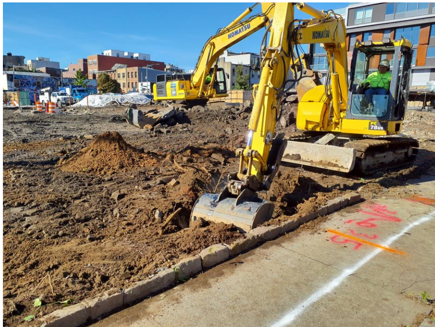
Photo 2: Kingdom excavating in the northern part of Society Brooklyn to pre-clear obstructions prior to soldier pile installation (facing southwest)
